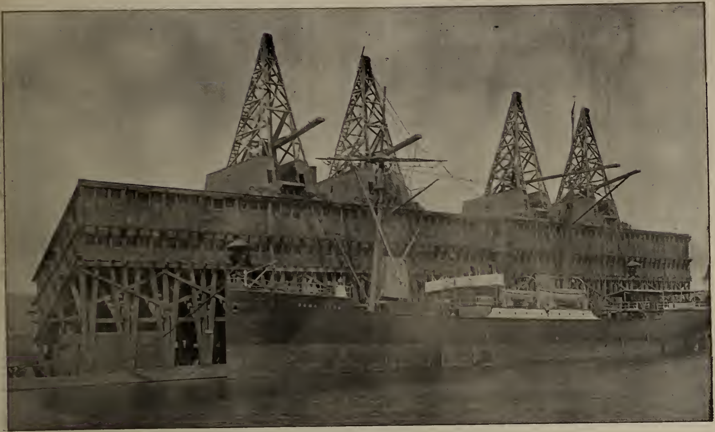
New Coal Handling Towers at Point St. Charles, Montreal.
