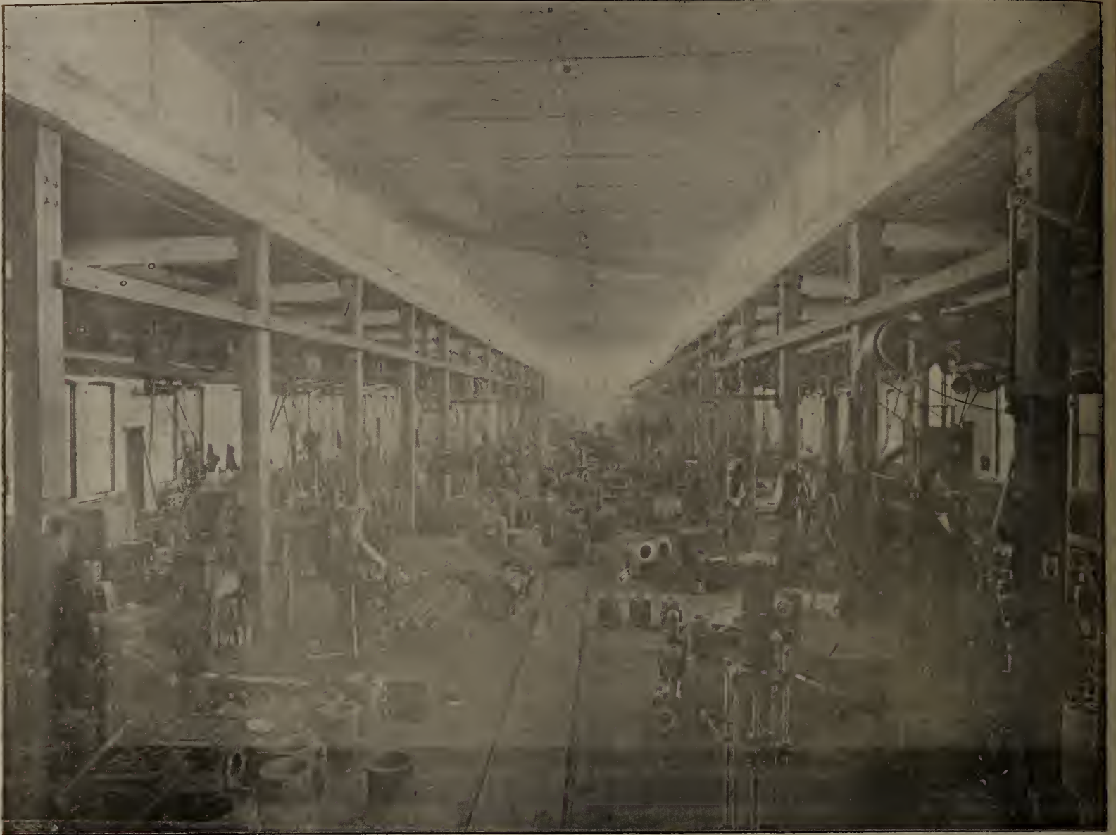
Works of the Northey Manufacturing Co. Ltd. at Toronto.—Interior of Pump Works.
