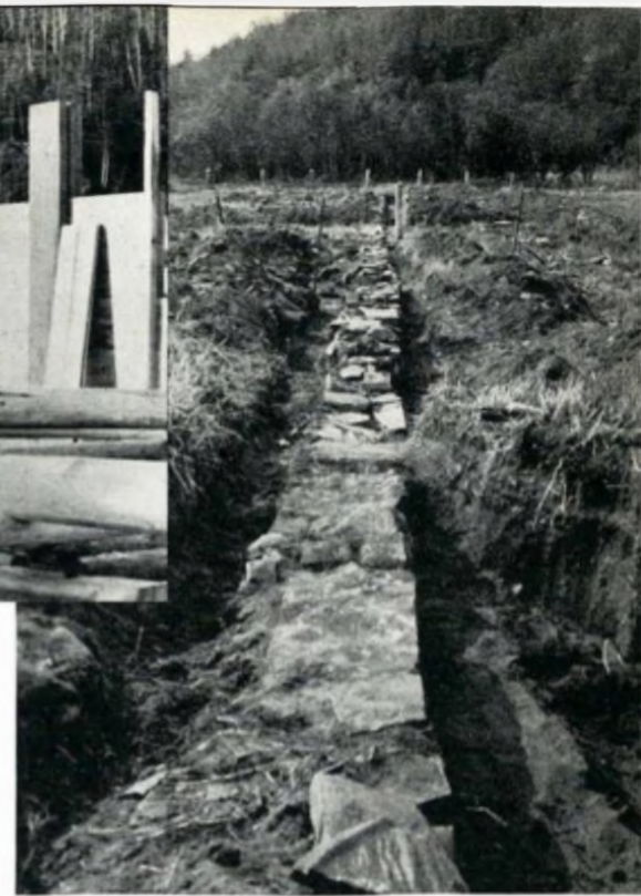
Original foundation of main hall, 95x30 feet.
