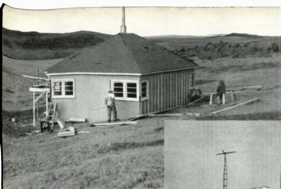
Building the new dwelling at Holman Island, north of latitude 70°. Plasterboard paper is being laid over the first coat of plywood, before the second coat is applied. Though the stormy winds do blow—at 50° below zero—the finished house stays snug and warm.
