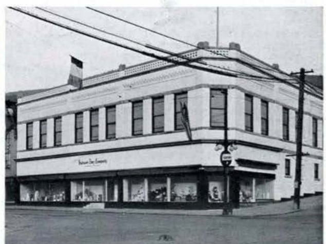
The Nelson store, built in 1899, also had its face lifted and the interior thoroughly modernized. A centre entrance was provided, and new fixtures installed on the ground floor. The two out-moded store buildings were made into one by removing a brick and masonry wall and substituting columns and beams. Such architectural feats are readily accomplished by the Superintendent of Buildings' staff.
