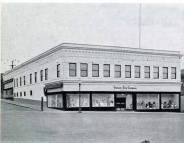
The Company's post in Kamloops was established in 1821. Today's retail store was remodelled this year. High transom windows were taken out, and modern show windows installed with black tile and chromium as a frame for display. Inside, both floors were remodelled for customer convenience and the display of merchandise.
