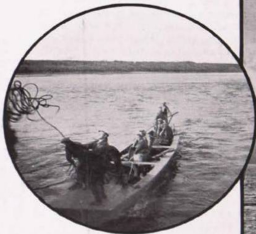
Cable scow about to tie up to large vessel after fastening cable to "dead man" on bank.
