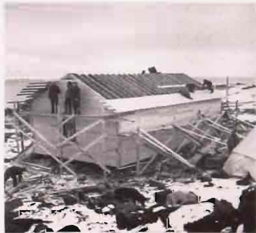
Construction of Fort Ross; the warehouse. Everybody digs in.
