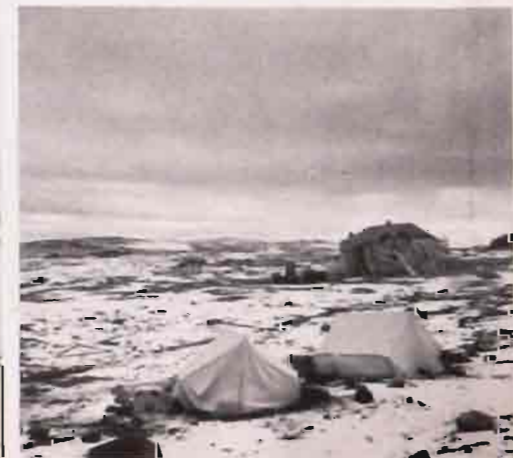
Construction of Fort Ross; the dwelling, with cook and temporary storage tents in foreground.
