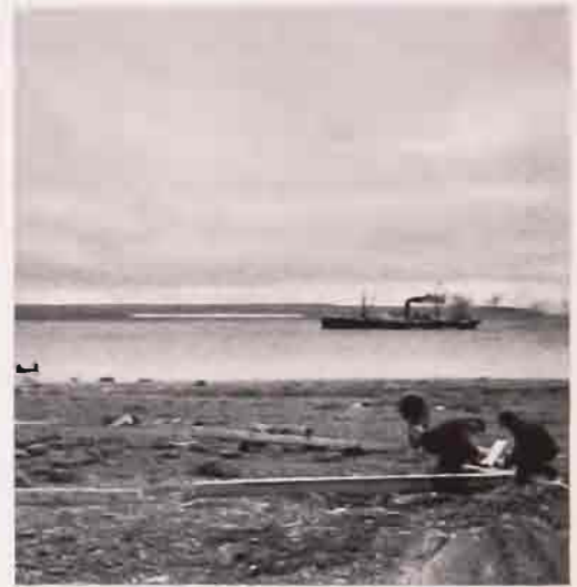
Laying the foundation for Fort Ross.
