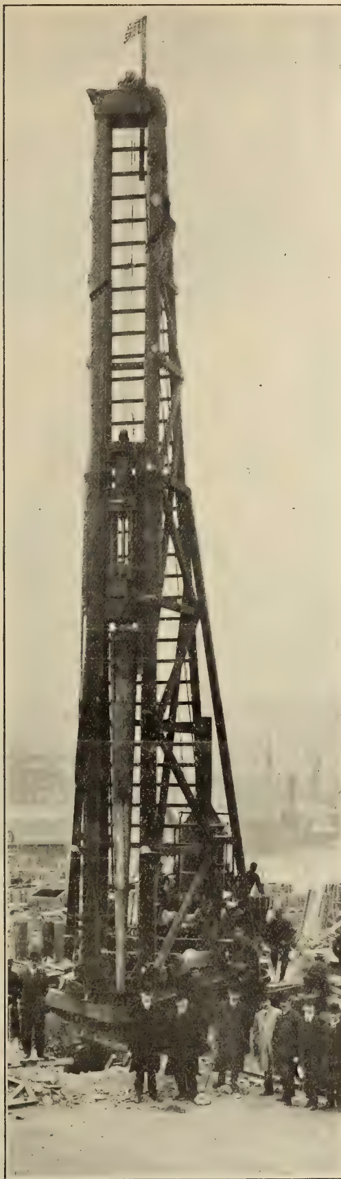
The core and shell of a Raymond concrete pile preparatory to placing. By means of the core the shell is driven to refusal. The core is then withdrawn and the shell filled with concrete.
