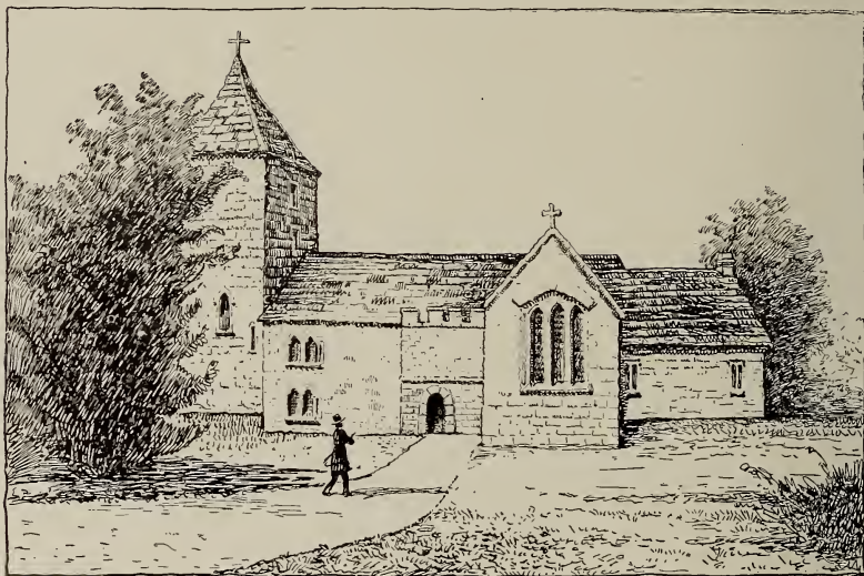
DUNKESWELL PARISH CHURCH BEFORE RESTORATION.
