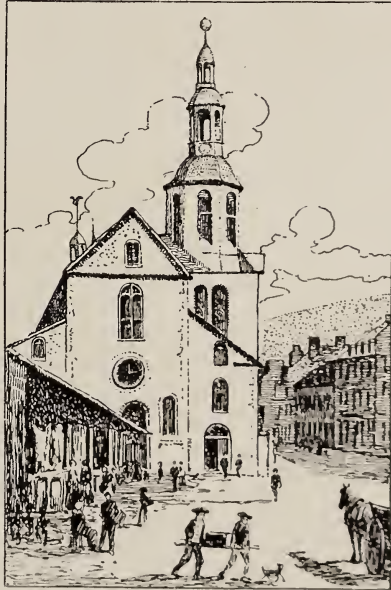
THE CATHEDRAL, QUEBEC, AS RESTORED.
