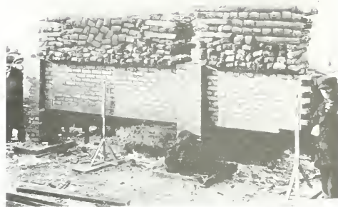
LOAD 12,512 LBS. TO THE PIER AND 6,750 TO THE RIGHT
