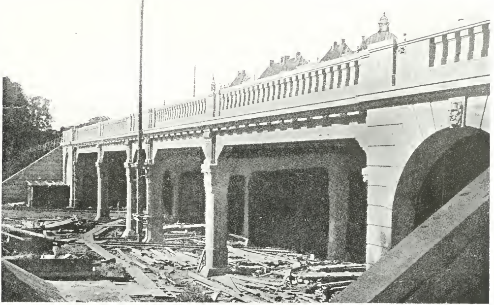
FIG. V.—ATTEMPT TO CONCEAL NATURE OF MATERIAL USED IN CONSTRUCTION
