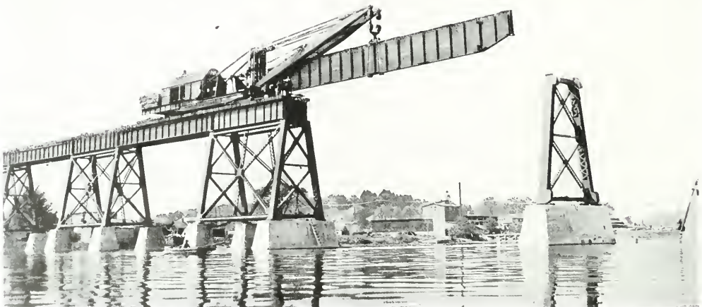
NO. 11.—THE 114-FOOT GIRDER CARRIED OUT BY DERRICK CAR.
