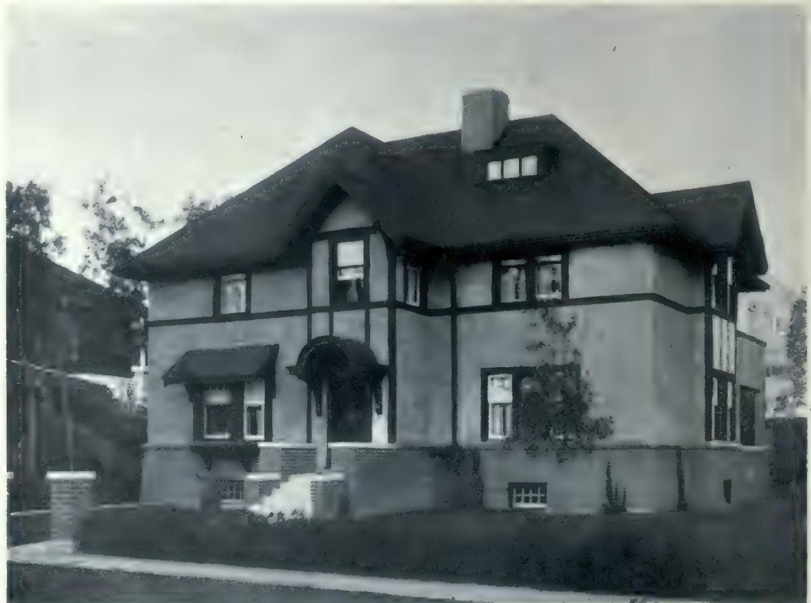
Residence of Mr. F. Christie, Betourney street. One of Winnipeg's many cement stucco houses, in which the plaster is applied directly to metal lath, thus making it a durable and permanent type of construction. J. D. Atchison, Architect.
