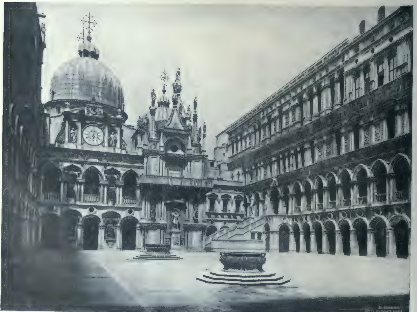
Ducal Palace, Venice. View showing Inner Colonnade and General Architectural Treatment of Court-yard Elevations. CONSTRUCTION, JUNE, 1910.
