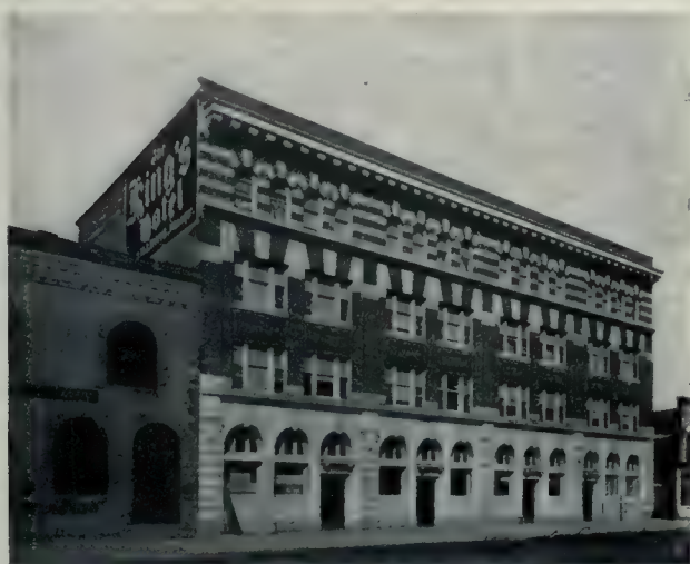
King's Hotel, Regina's $200,000 hostelry, which is the most modernly appointed building between Winnipeg and the Coast. Storey & Van Egmond, Architects.
