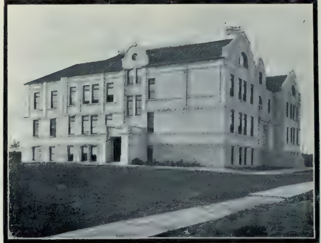
La Verendrye School, Winnipeg, Most Recently Erected and Elaborately Equipped School Building, Built of Sand-Lime Brick. Designed by Commissioner of School Buildings J. B. Mitchell.
