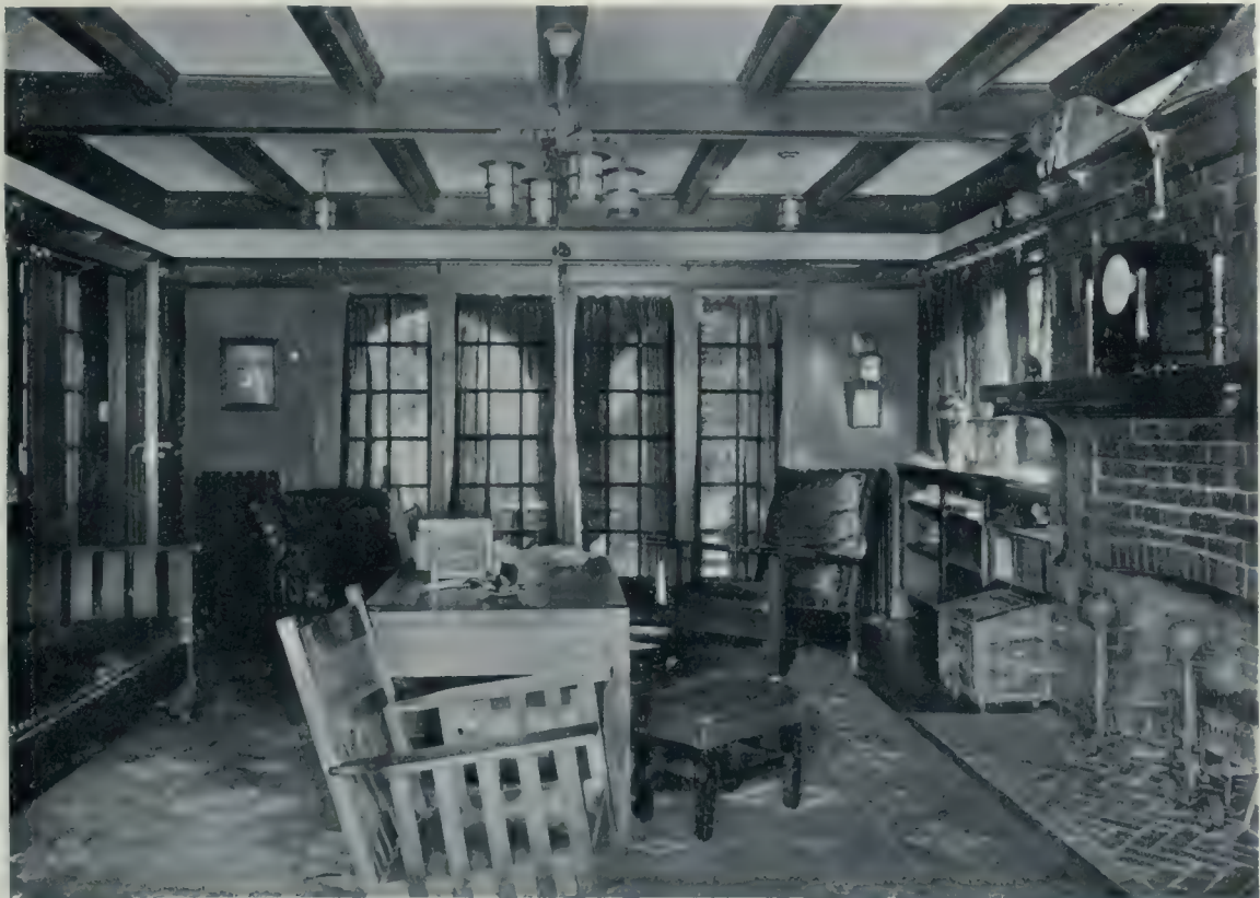
View of Same Room, Looking Towards the Front of House. Built-in Conveniences are Found in the Form of Book Shelves and the Fixed Seat which Conforms to the Large Bay Window. The Fireplace is of Vitrified Crucible Brick, and the Lighting Fixtures are Designed to be Consistent with the General Scheme. Chadwick and Beckett, Architects.
