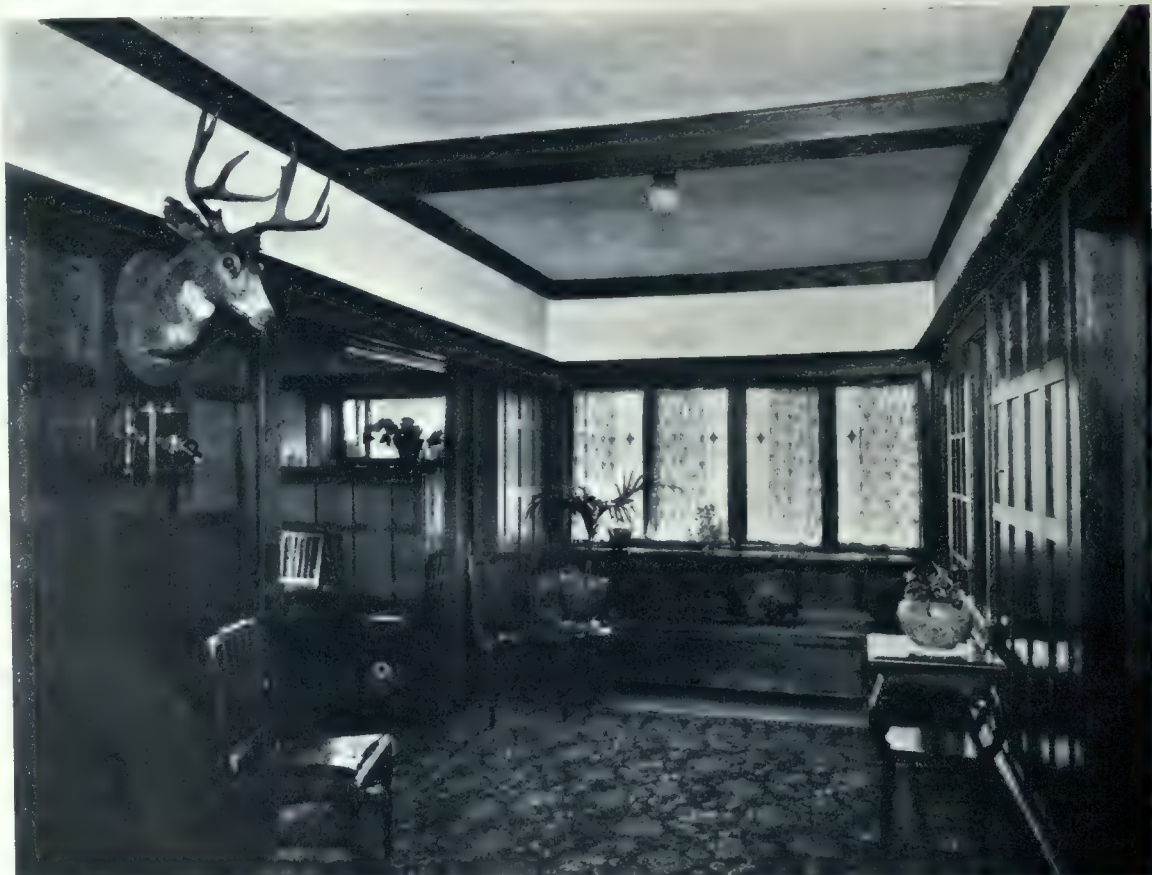
Hallway, Residence of Fred J. Calvert—With its Built-in Window Seat and High Wall Panelling, a Similar Wall Scheme Being Seen in the Dining Room Through the Opening on the Left. E. Stanley Mitton, Architect.
