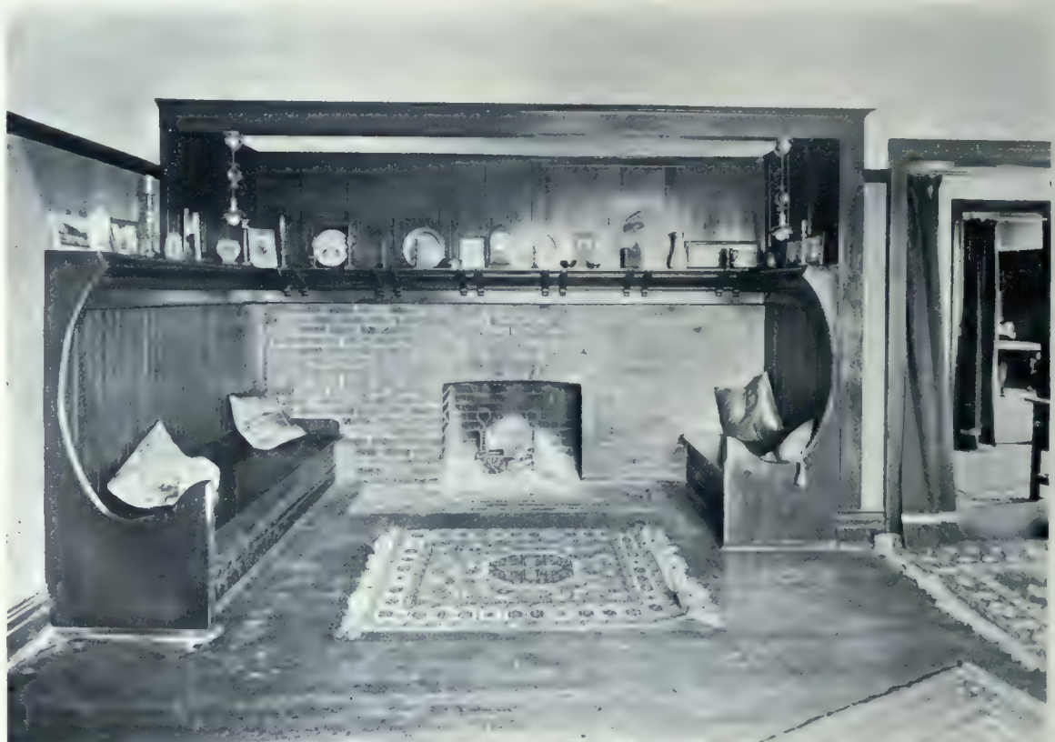
Living Room Ingle, Residence of Howard Bovell, Western Avenue, Toronto. Built of Ontario Paving Brick, with Hinged Seats on Either Side to Form Fuel Boxes. Chadwick and Beckett, Architects.
