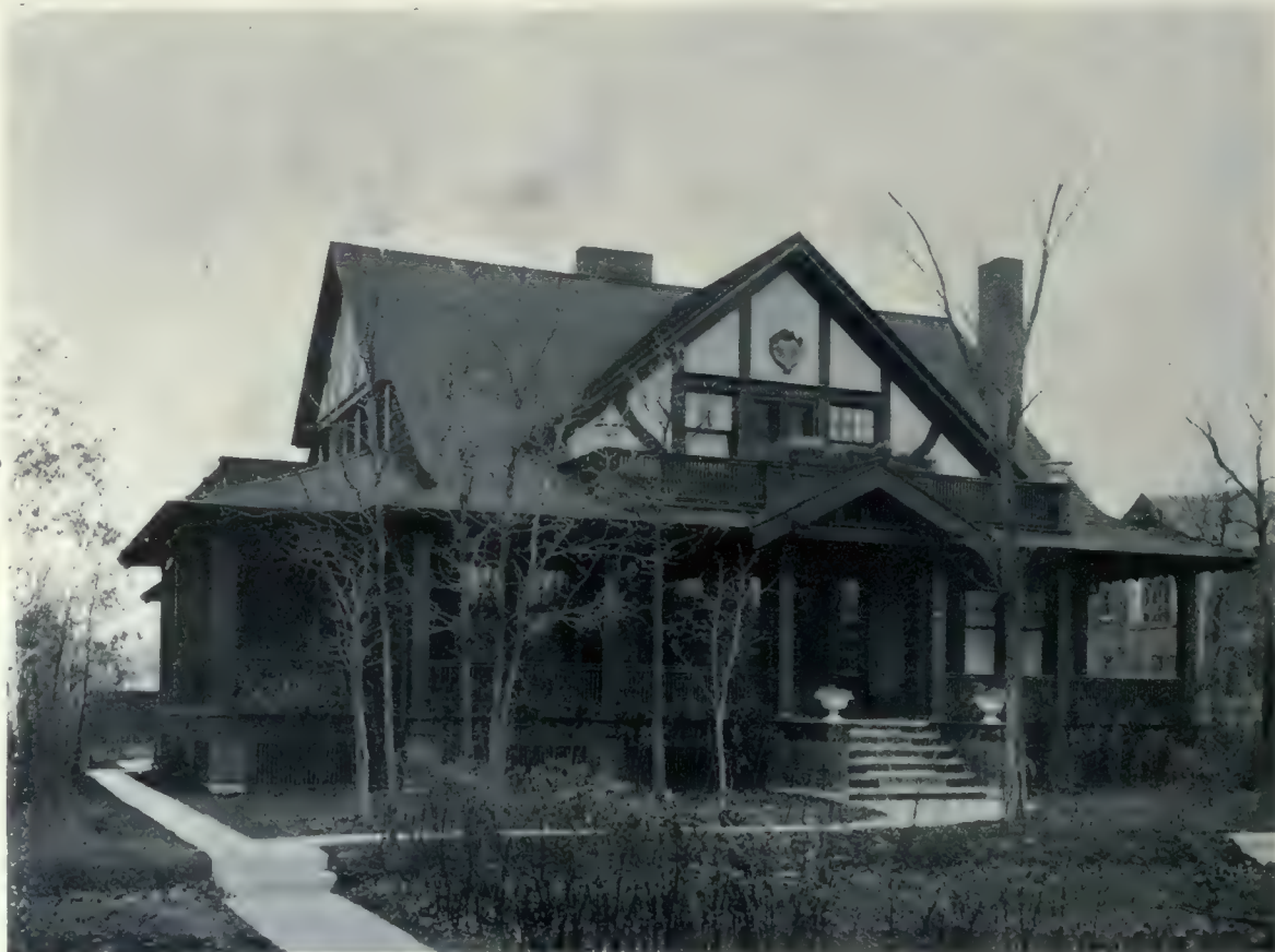
Bungalow of F. W. Pace, Wellington crescent, Winnipeg. The graceful lines, half timbered gables, and soft brown tone of woodwork, serves to give this little abode a pleasing individuality and homelike appearance. J. H. G. Russell, Architect.
