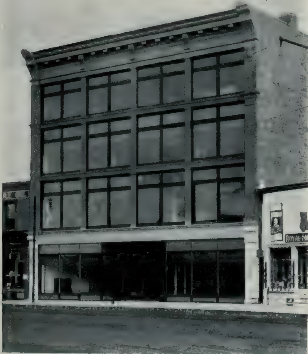
Store and warehouse of the Blower-Henry Company, Edmonton. R. Percy Barnes, Architect.
