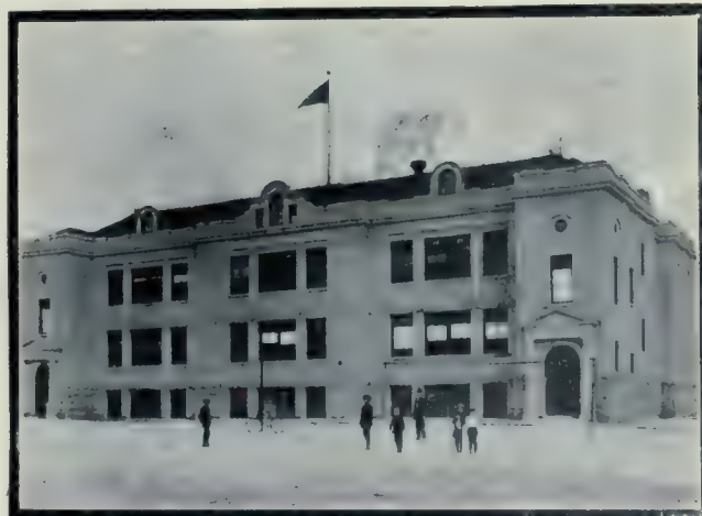
Lord Selkirk School—One of Winnipeg's Several Important Educational Buildings, in Which the Entire External Wall Construction is Executed in Sand-Lime Brick. Designed by Commissioner of School Buildings J. B. Mitchell.
