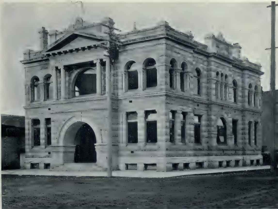
Public Library Building, Victoria, B.C. A Substantially Built Structure, Having British Columbia Granite Exterior Walls. Thos. Hooper, Architect.
