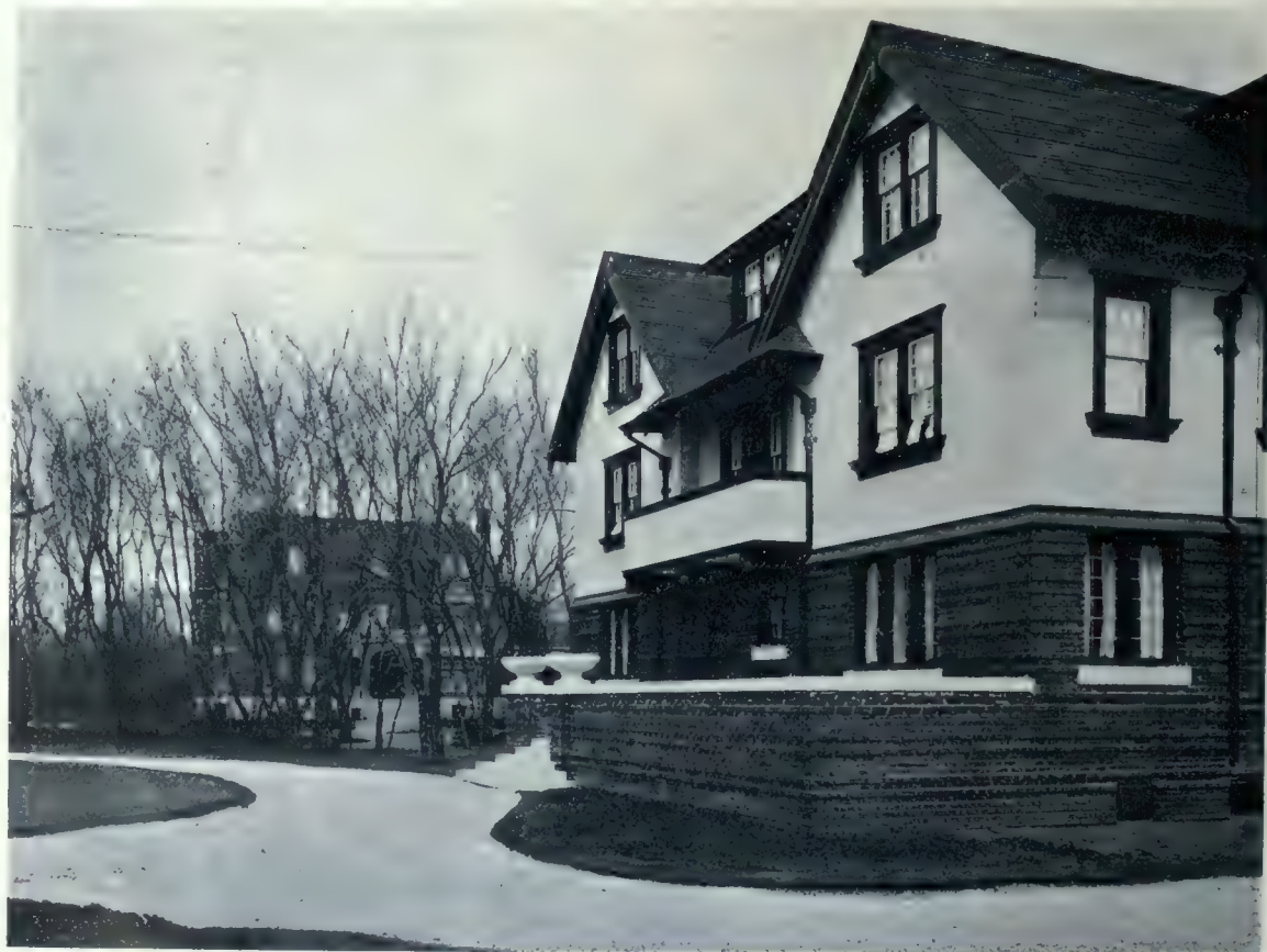
Residence of Hugh F. Osler, Winnipeg. The walls of this Residence are Built of Concrete Blocks, Veneered with Copper Color Vitrified Brick for the Lower Storey and Finished with Cement Plaster above. The Tone of the Woodwork is Brown, save the Window Sashes, which are Painted White. This View Shows the Main Approach, and gives a Fair Idea of the General Character of the Surroundings. Herbert B. Rugh, Architect.
