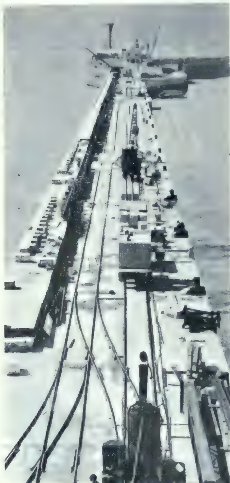
BUILDING THE ADMIRALTY PIER.
