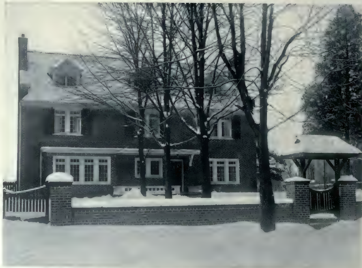
Residence of Thomas Baker, 630 Talbot Street, London, Ont. F. S. Baker, F.R.I.B.A., Architect.
