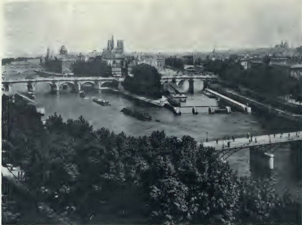
General View of the Older Portion of Paris on the Island Known as the Cite, Showing Pont Neuf, built 1578-1604, with a Portion of Pont des Arts in the Foreground, and Pont Au Change, Pont Arcole and Other Bridges in the Upper Left of Picture.
