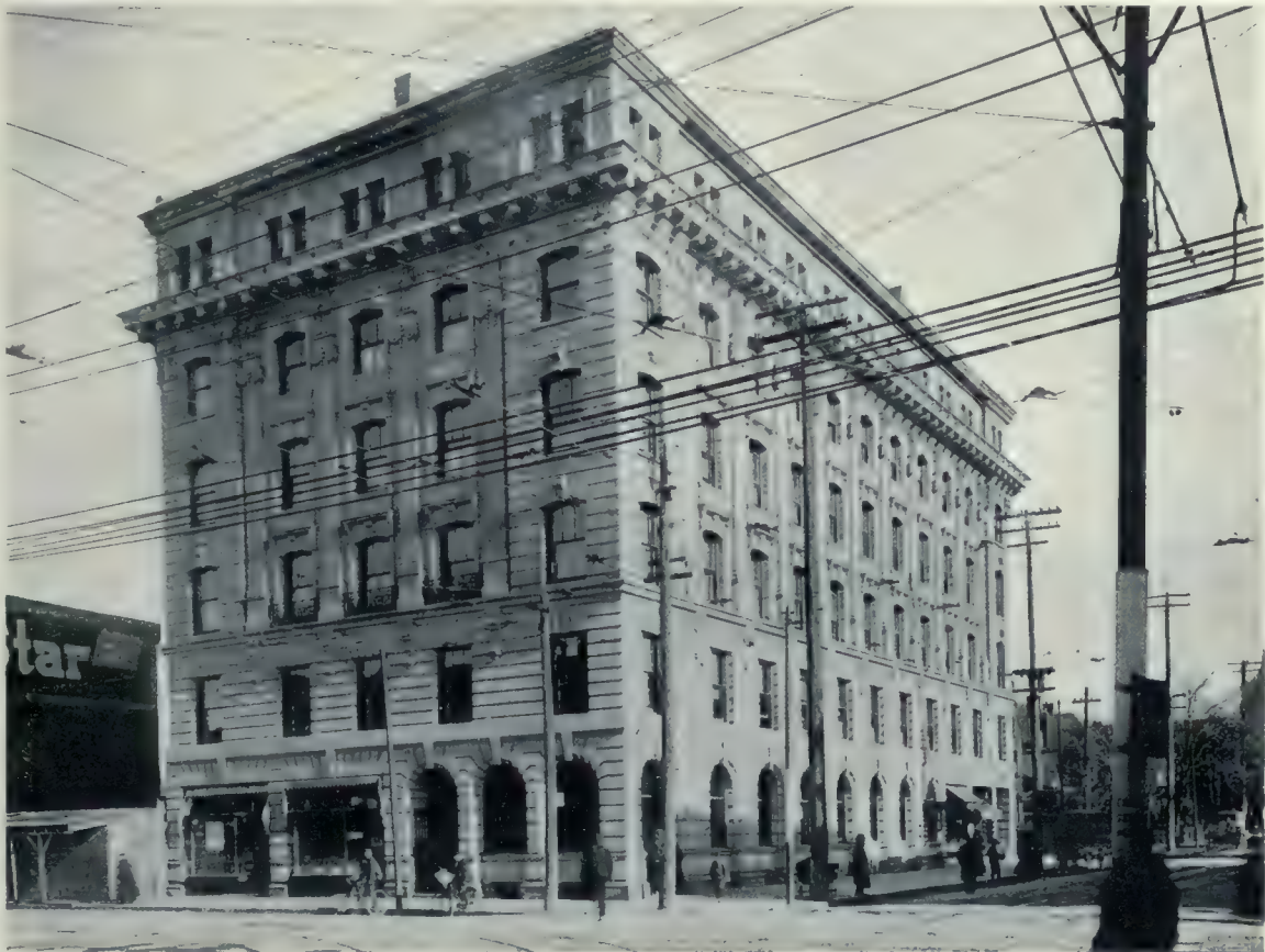
Traders Bank Apartments, cor. Yonge and Bloor Sts., Toronto. F. S. Baker, F.R.I.B.A., Architect.
