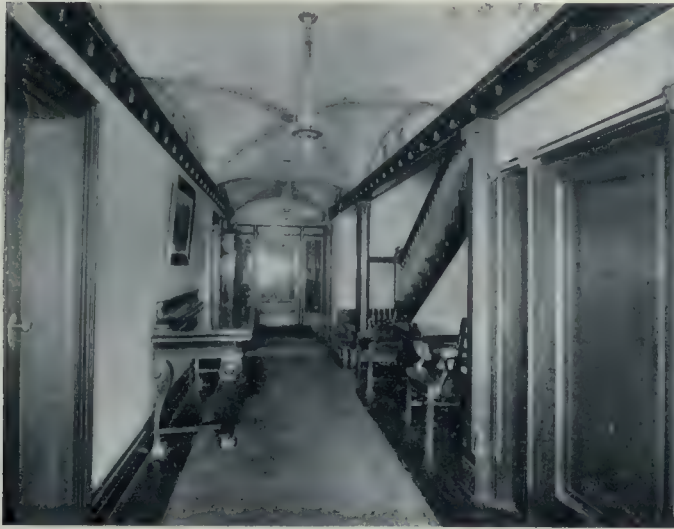
Main Hall, Looking Toward Entrance.
