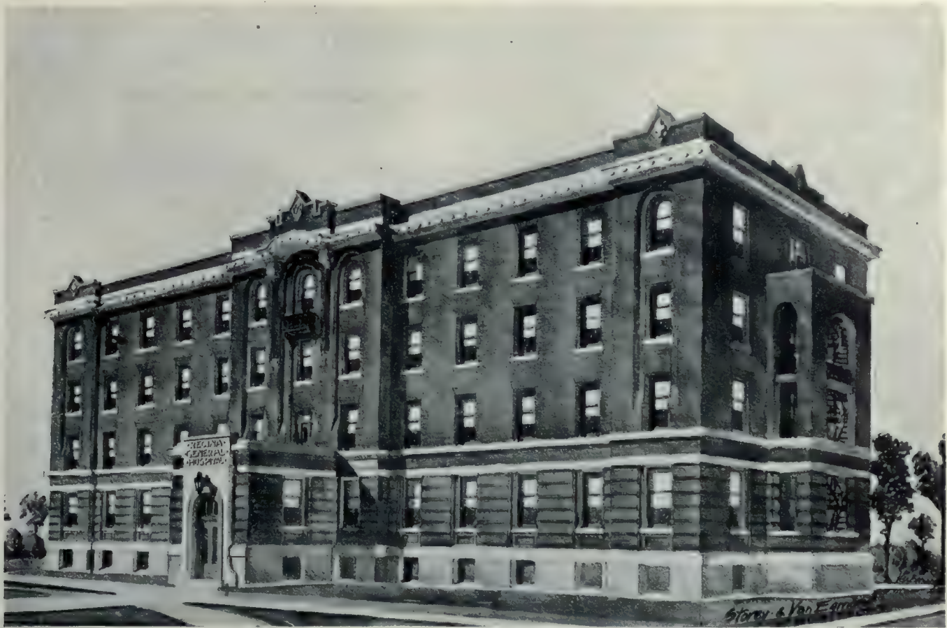
Regina's New General Hospital, now being built at a cost of $105,000. Although the building is to be entirely fireproof in its construction, an additional precautionary measure is provided in an enclosed outside iron stairway, placed at end of the structure. Storey & Van Egmond, Architects.
