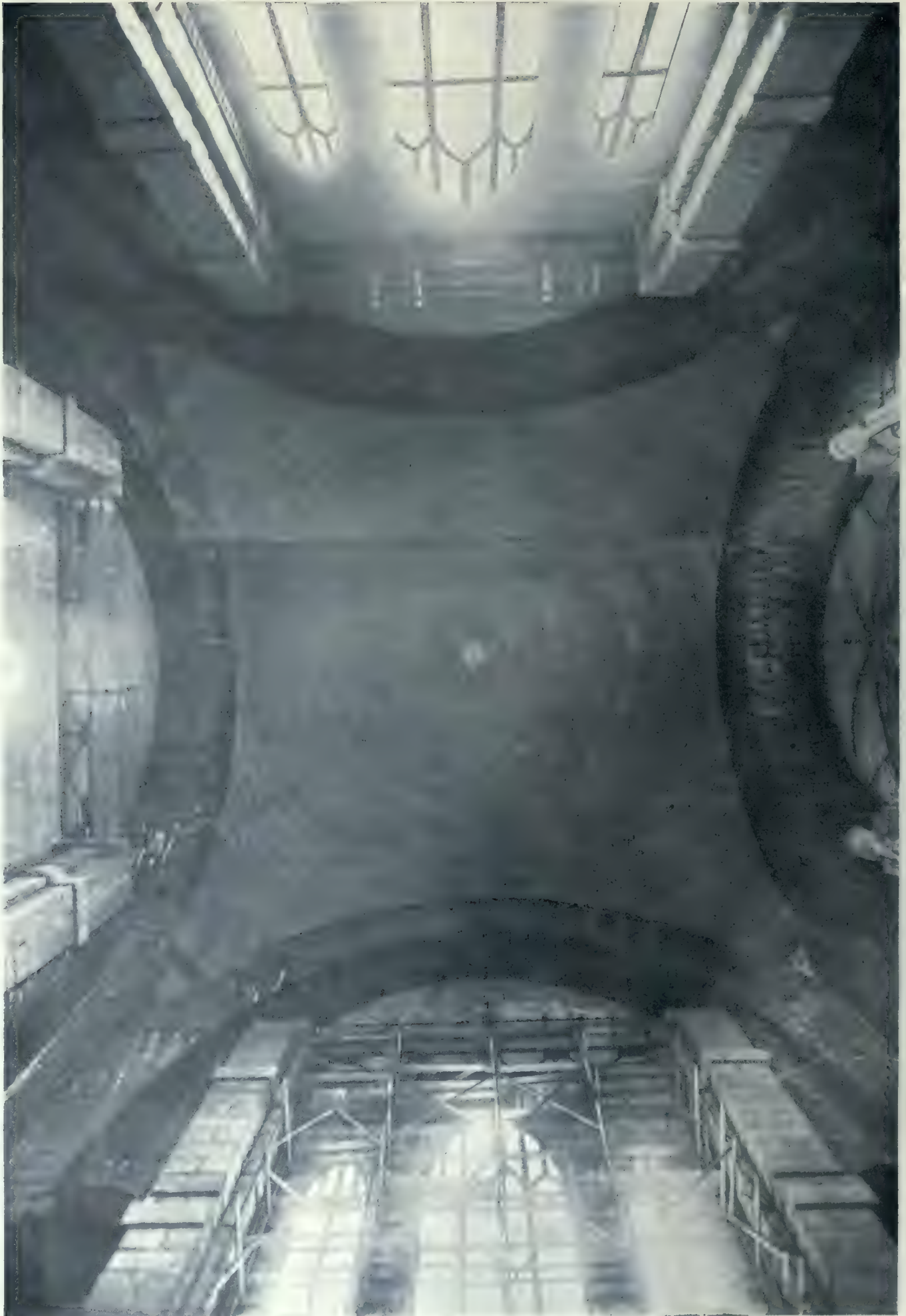
Looking up into the immense dome. Cathedral of St. John the Divine, New York City, the construction of which, being carried out in defiance to all accepted theories of engineering of this kind, is entirely without precedent. It was built without either false work or scaffolding, and is the third largest dome in the world, being 135 feet in diameter, or 7 feet less than the dome of the Pantheon in Rome.
