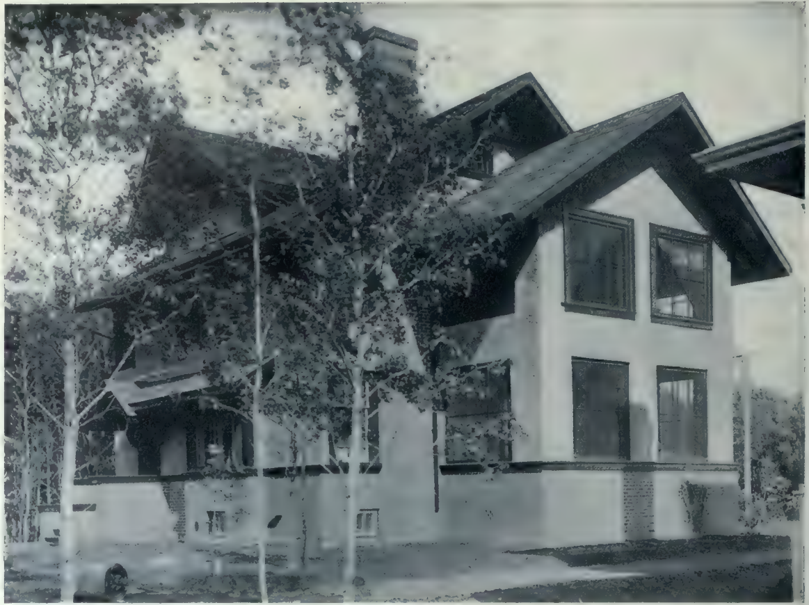
Residence of George Stephen, Winnipeg. A modern cement stucco house with straight lines and pleasing gables, and attractively set off by red sand mould brick up to the first floor window sills. Herbert B. Rugh, Architect.
