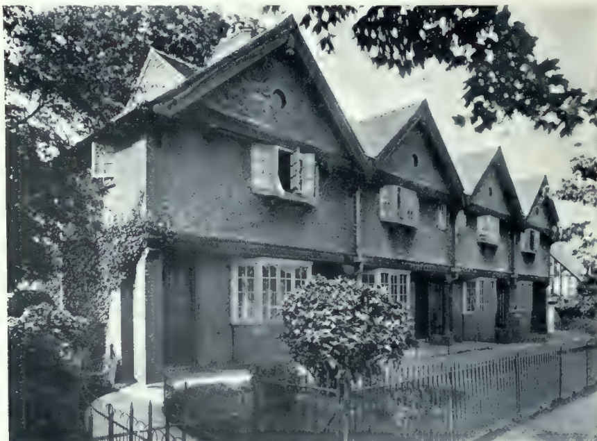
Wood Street, Port Sunlight. In this Row of Cottages the Walls are of Brick, Rough-casted in the Upper Portion and Finished with Decorative Plaster Work in the Gables.
