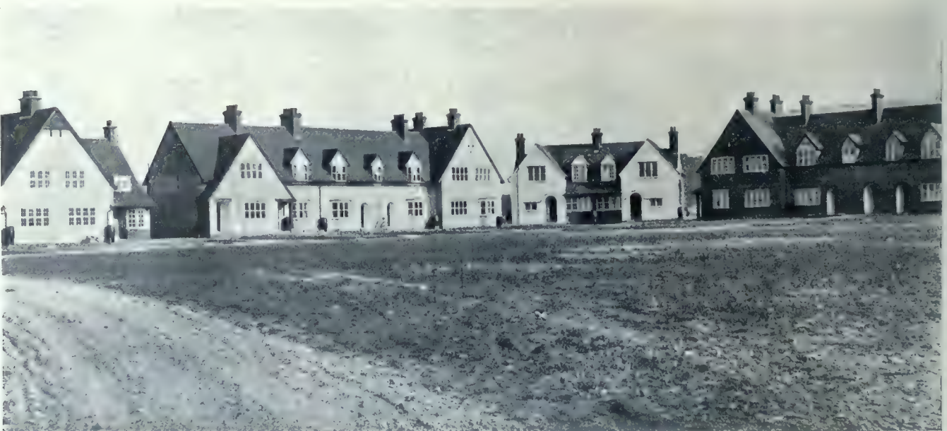
Cottages at Westholm, Letchworth. In Most Cases, the Houses are Built of Brick and Covered with Roughcast Color-washed a Light Cream. The Facing Brickwork is of a Warm Red Color and the Roof is of Hand-made Sand-faced Tile Toned Down to be in Harmony with the Cheerful but Restful Appearance of the Walls.
