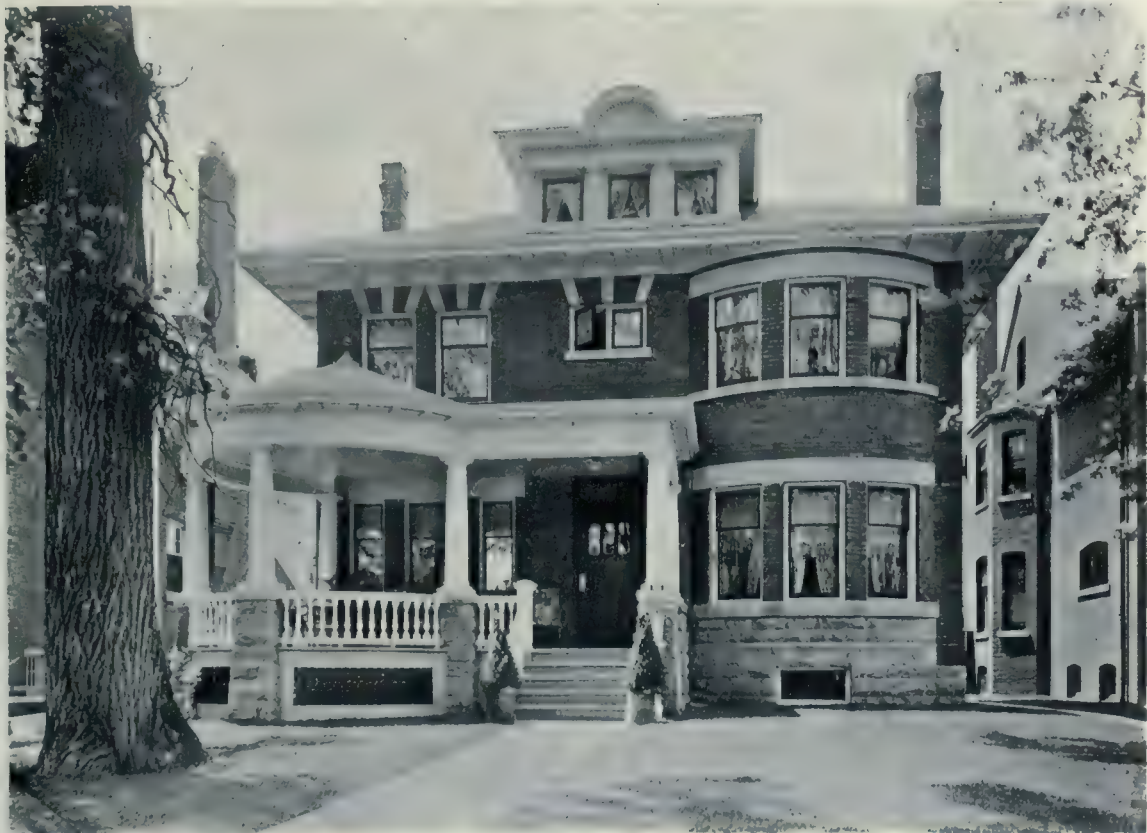
Home of H. Horseman, 185 Crescent Road, Toronto. A Residential Structure Designed along Modern Lines, with Red Brick Walls, Grey Stone Trimmings and White Painted Woodwork. Ellis & Connery, Architects.
