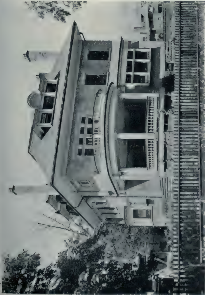
Residence of John H. Eyre, 58 Avenue Road.
