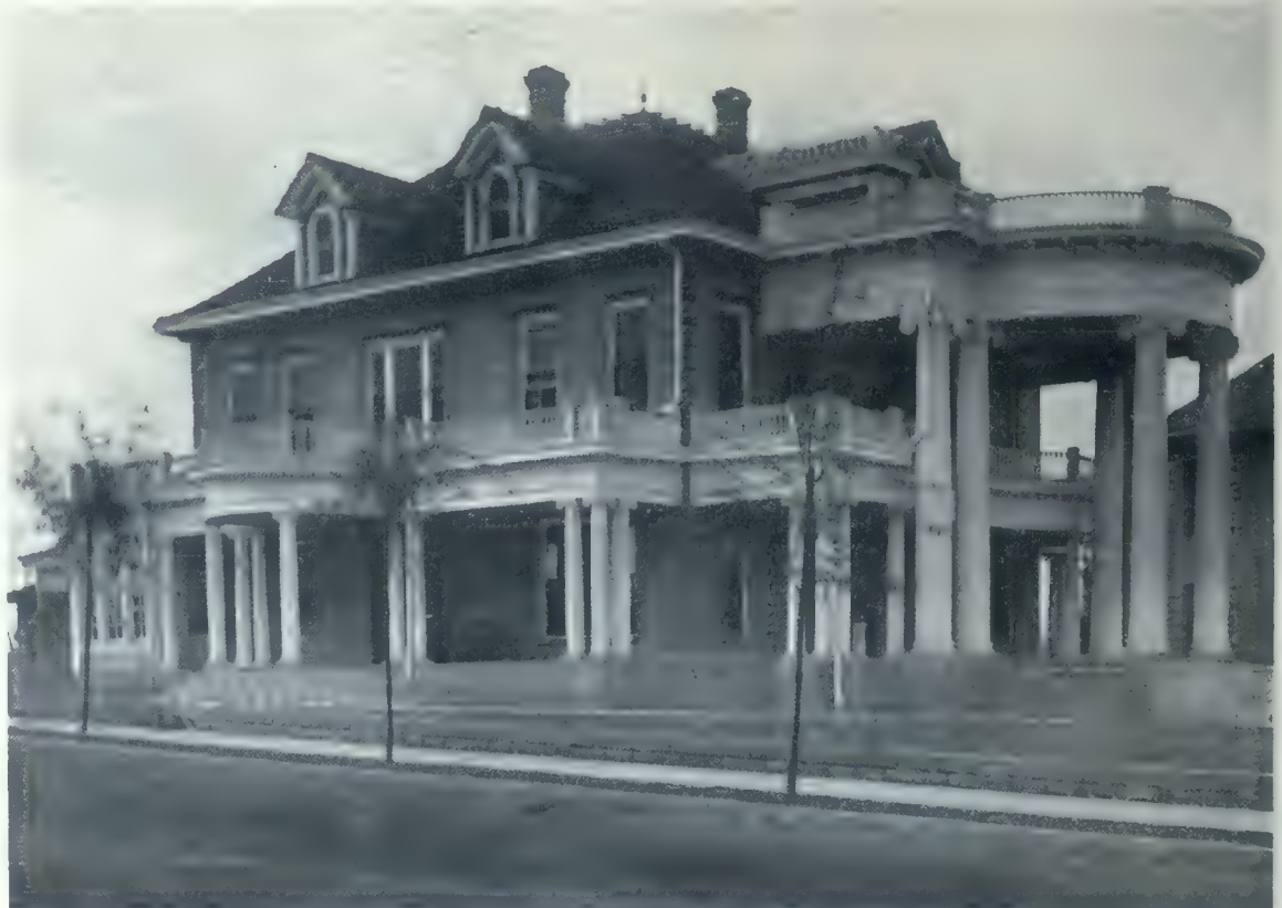
Residence of Dr. Dickerson, McComb, Mississippi. An attractive Dwelling Structure in which the Walls are Constructed of Plain Concrete Blocks with Bevel Block Trimmings.
