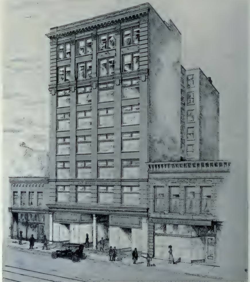
The Bower Building, an Eight Story Fireproof Store and Office Structure now in Course of Erection on Granville Street, Vancouver, B.C. The Frame Work of the Building is of Steel Encased in Concrete—this Latter Material Also Being Used for the Curtain Walls—While the Front is Faced with Bedford Indiana Limestone of a Blue Tone. Thos. Hooper, Architect.
