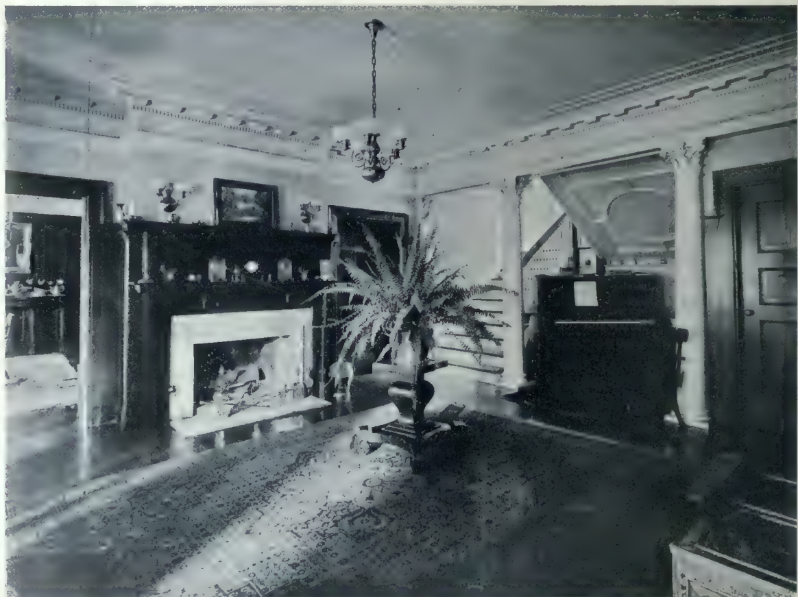
Main Hall, Residence of Miller Lash, Lowther Avenue, Toronto. This Interior is in Character with the General Style of the House. The Plan is Square and Roomy, and the Walls to a Height of Five Feet are panelled in Oak, Stained a Rich Brown, in Keeping with the Other Woodwork. Sproatt and Rolph, Architects.
