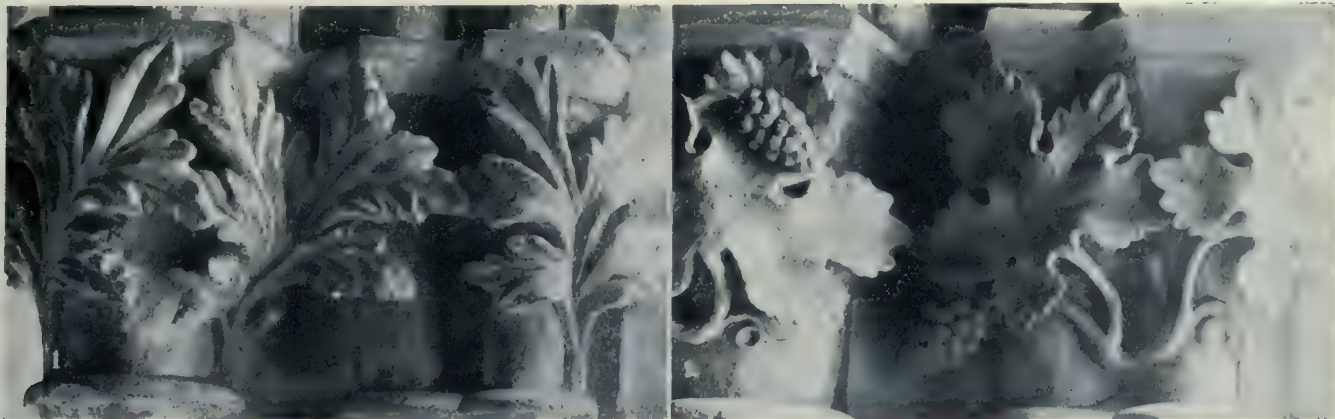
Capitals of Columns in Vestibule to Cloister.
