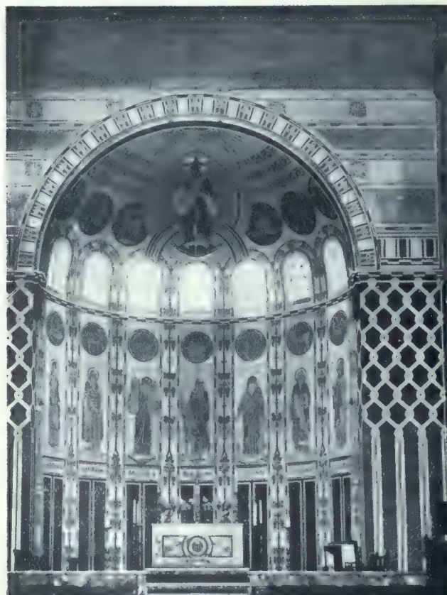
Beautiful decorations in Sgraffito, as seen in the Apse of St. Agatha's Church, Portsmouth.
