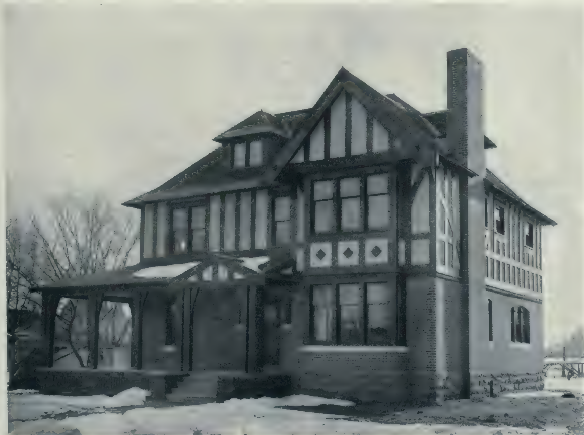
Rectory of Holy Trinity Church, Pembroke, Ont. The Red Brick and Half Timbered Treatment give this House a Simple English Feeling. It is very pleasantly situated, being Located on Elevated Grounds, Overlooking the Ottawa River. C. P. Meredith, Architect.
