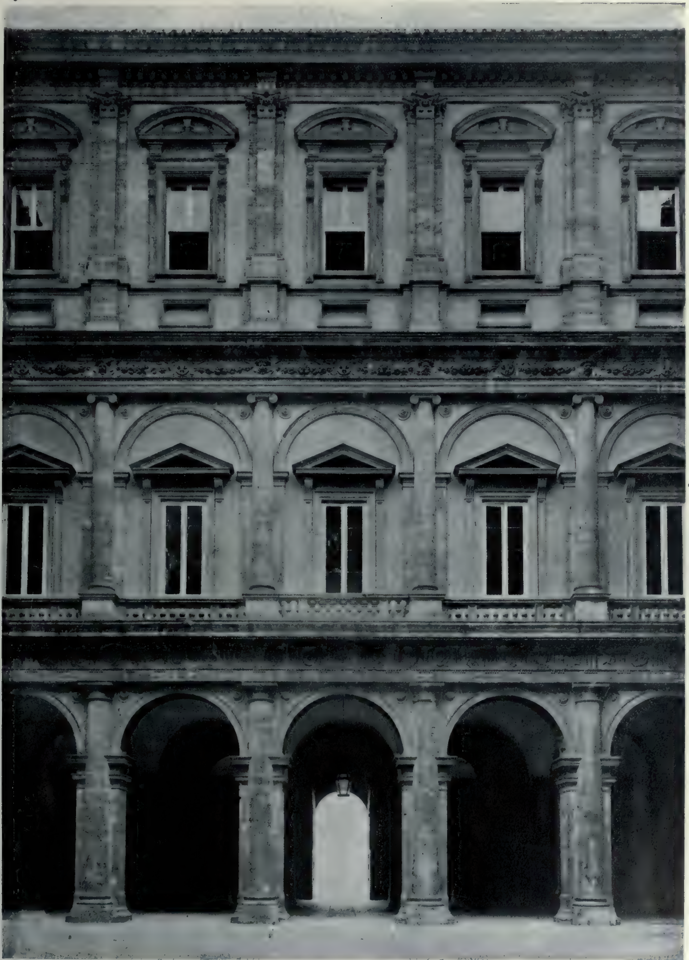
Court of Farnese Palace, showing the Doric, Ionic and Corinthian Columns which decorate the piers in the respective stories as they rise, and the general treatment of window scheme and cornices.
