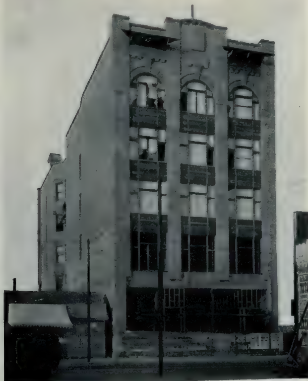
Store and office building for Mr. A. J. Samis, which is now being completed on Eighth avenue east, Calgary. Dowler & Michie, Architects.
