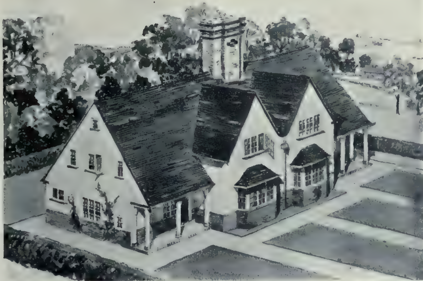
(E)—Plan of Cottages, Holmstead Road, Hampstead, Which Cost About $2,500 to Build. In this Structure Roughcast is Used on the External Walls, the Roof Being of Tile. Note the Balance of the Design and the Single Bold Chimney. J. Gordon Allen, Architect.
