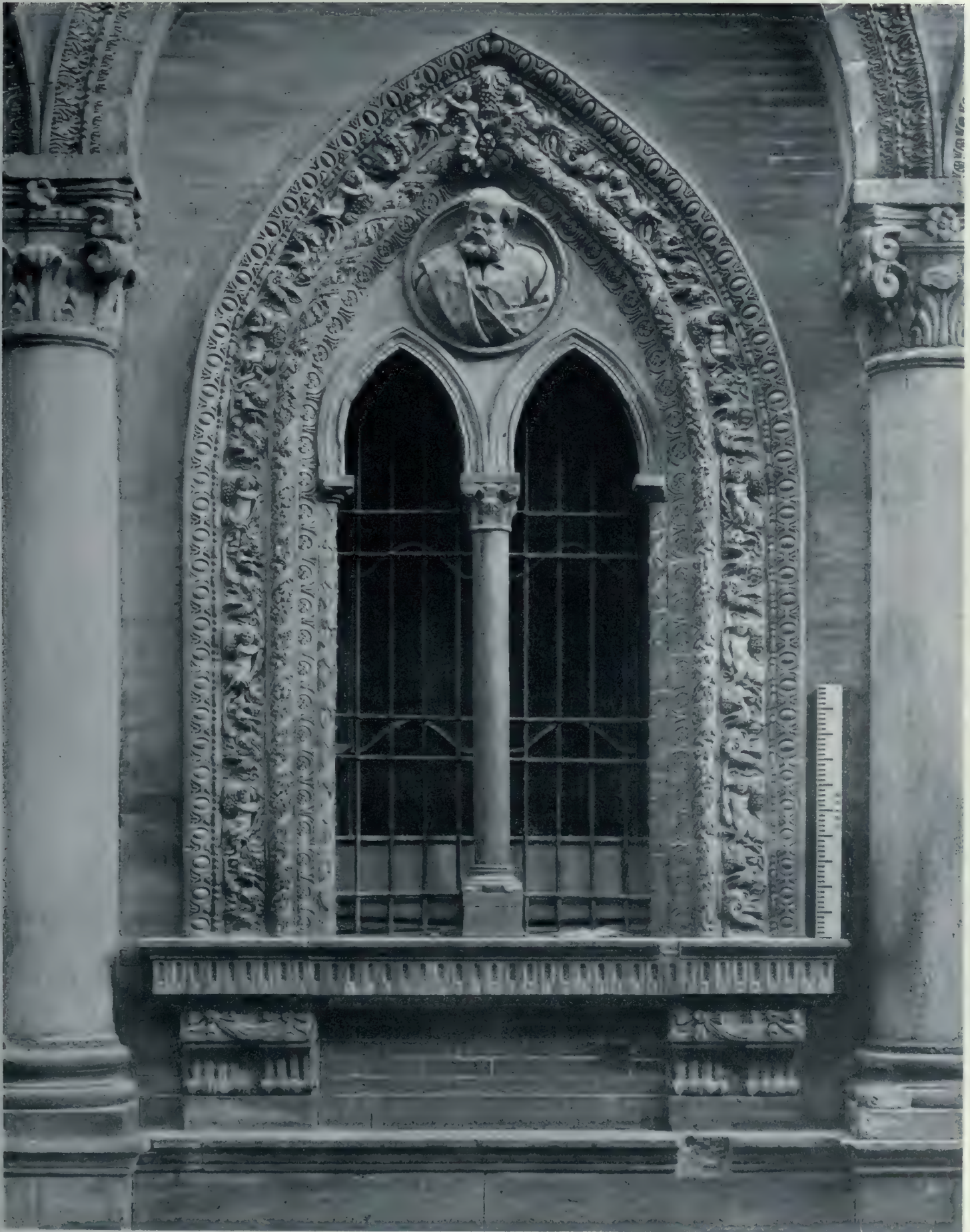
Detail of one of the lower pointed windows of the Maggiore Hospital, Milan, showing bi-secting columns supporting the sham arches. The common frame work with its elegant decorations above all with the narrow space of fine leaves interspersed with exquisite birds. The head in the window shown here gives some idea of the freshness and sharpness of the work, which is most realistic in style, as is demonstrated in the flowing and detailed beard in the medallion.
