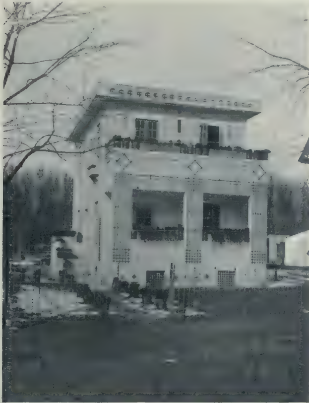
Two-Storey Concrete House erected at Brantwood, Maryland. The walls are 8 inches in thickness and the floors are 4½ inch slabs reinforced in both directions. This was the first house constructed with standard section moulds, and it was built to demonstrate the possibilities of reinforced concrete in low priced, sanitary, fireproof residences. Milton Dana Morrill, Architect.
