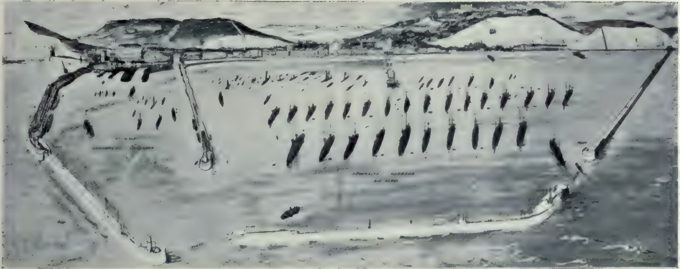
The new Harbor at Dover, as seen from the English Channel, the greatest artificial enclosure for war vessels and merchantmen ever constructed. Some idea of the magnitude of the undertaking may be gathered from the fact that the outer masonry walls alone measure 2½ miles in length, and necessitated in their construction over a quarter of a million barrels of Portland cement.
