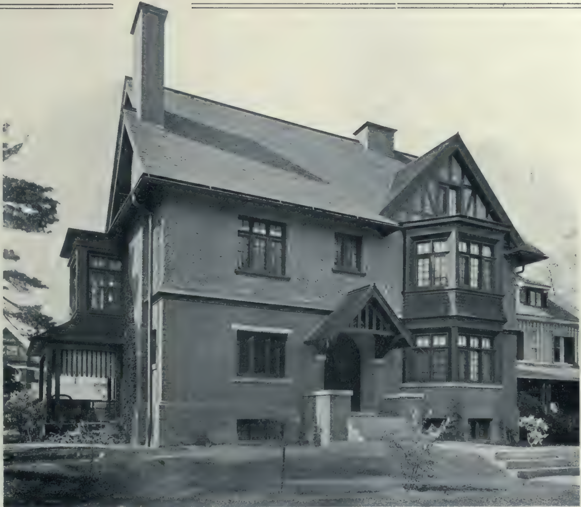
Residence of H. H. Beck, Clarendon Crescent, Toronto. Both in Design and Situation this house possesses a strong Domestic Interest. The Walls are of Red Brick for the Lower Storey, with Rough Plaster Cement above, the Wood Work and Gable Timbers being painted Brown. Charles P. Band, Architect.
