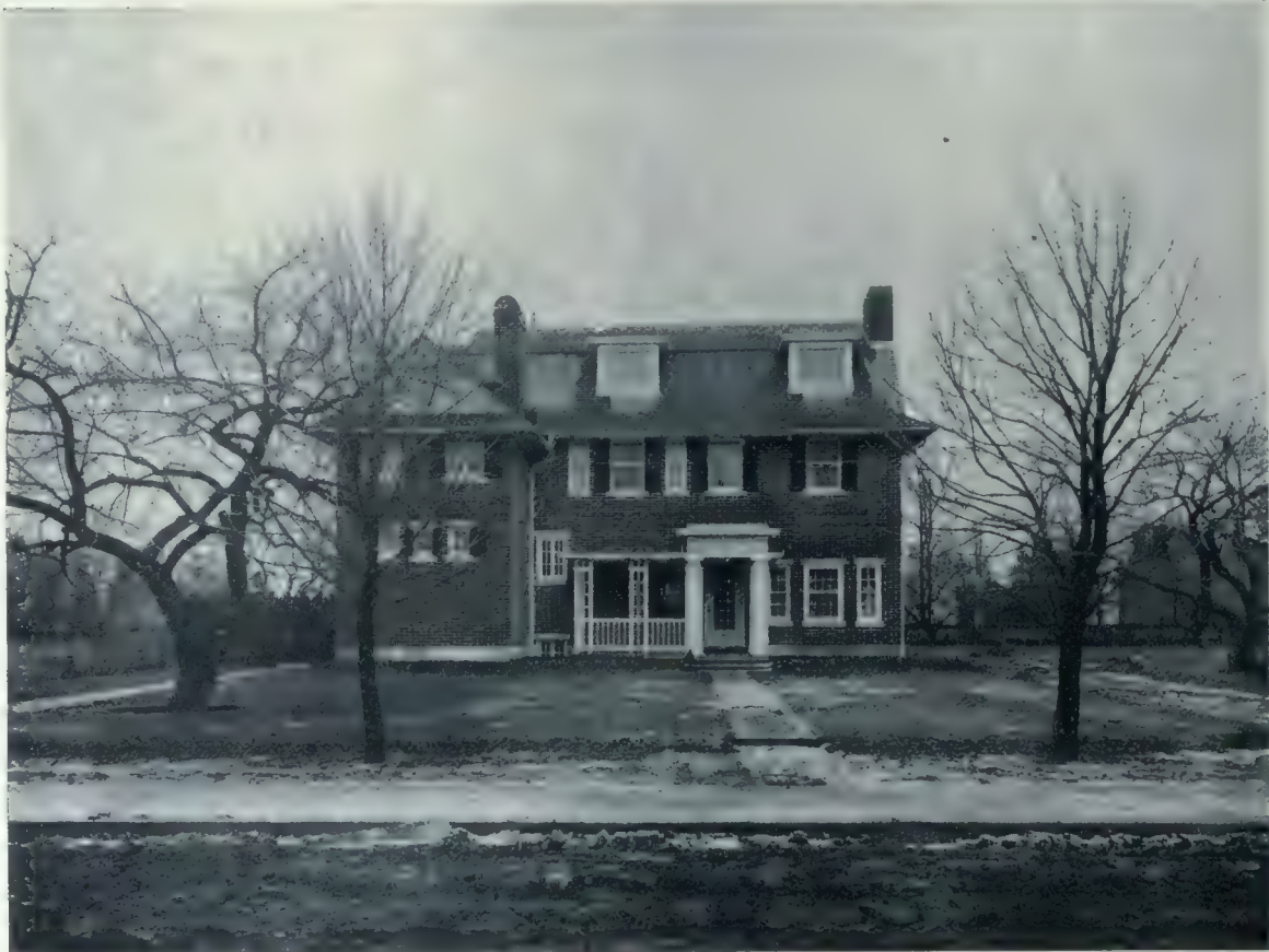
Residence of E. R. Rolph, of the firm of Sproat & Rolph, Architects, on Jackes avenue, Toronto. An interesting Georgian house with walls of ordinary red brick laid in a double stretcher bond, so jointed with false vertical joints of the same colors as to take on the appearance of Roman brick.
