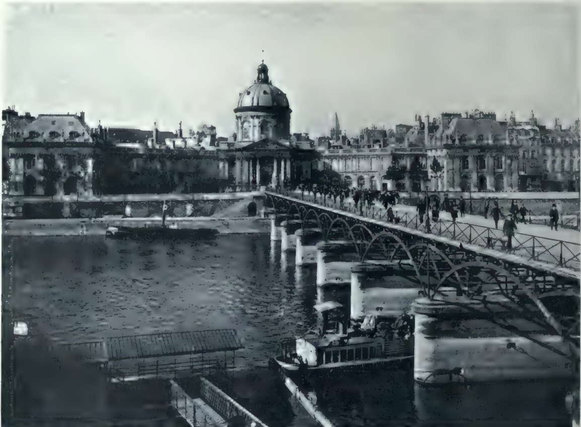
Pont des Arts—Built in 1802-04. This Bridge is Built of Cast Iron and is Used by Pedestrians Only.
