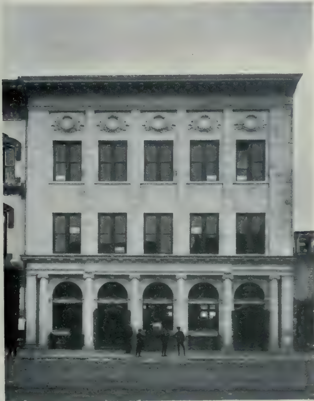
Main branch of the Traders Bank of Canada, Winnipeg, built of Tyndall stone, a peculiarly beautiful whitish grey, brown veined, stone quarried a few miles south of the city. F. S. Baker, Architect.
