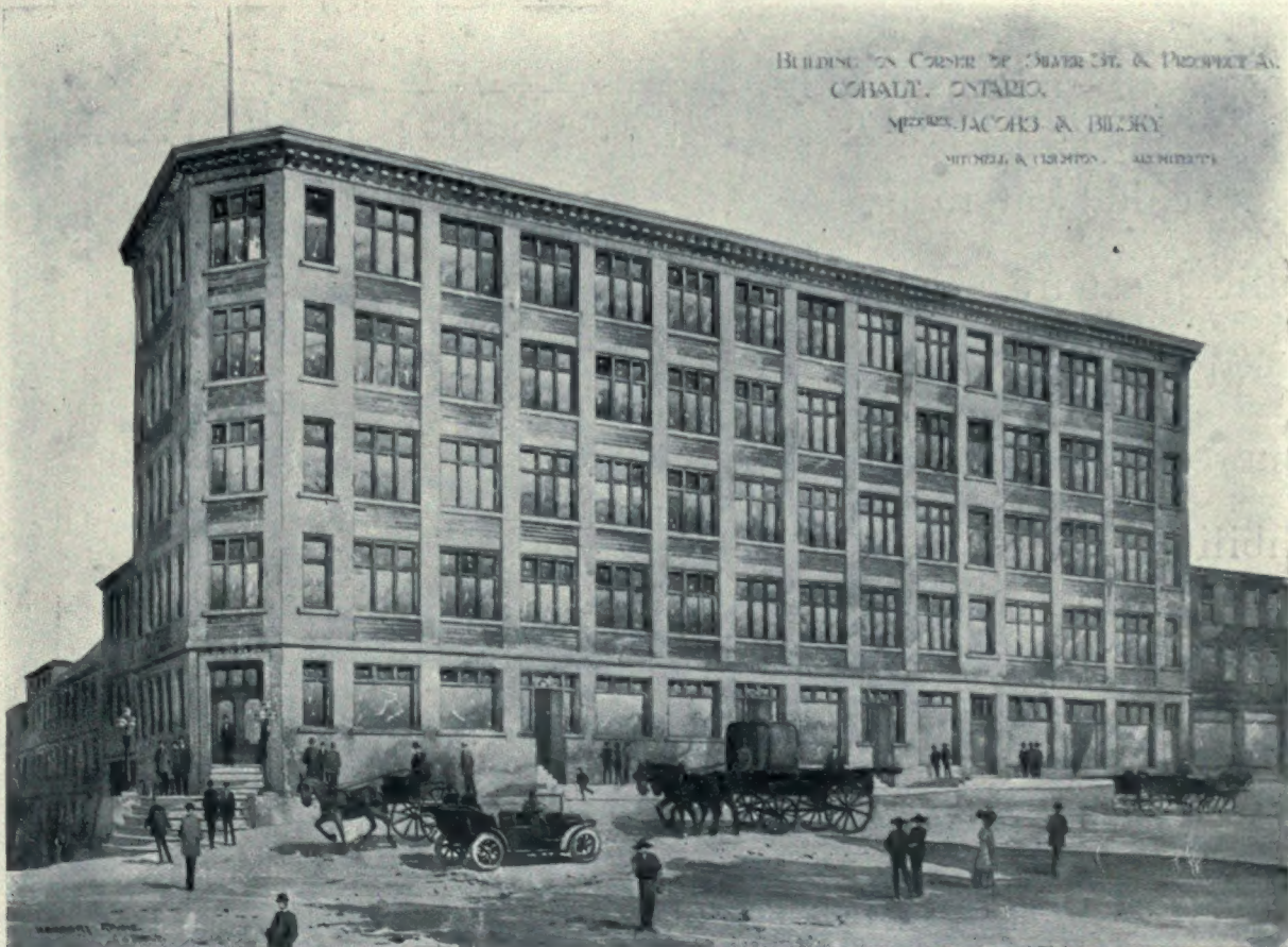
FIREPROOF OFFICE BUILDING, OF RE INFORCED CONCRETE, COBALT, ONT. Owner, Jacob A. Jacobs. Architects, Mitchell & Crighton. Contractors, Bishop Construction Co. Kahn System of Reinforcement used.
