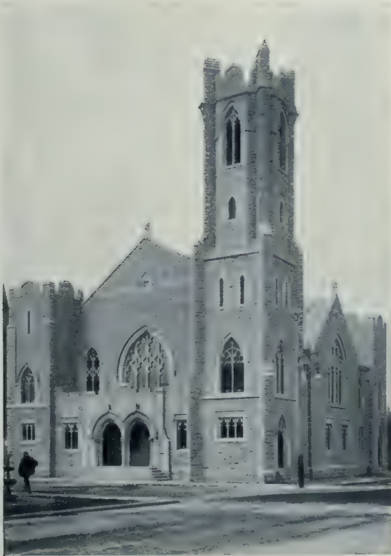
St. Andrew's Presbyterian Church, Fort William, Ont. Hood and Scott, Architects.
