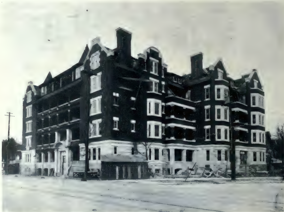
Roslyn Court, Roslyn Road, Winnipeg. One of the recently completed apartment buildings, a noteworthy feature of which is the scheme of outside balconies, with doorways opening from each suite. Wm. Wallace Blair, Architect.
