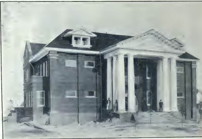
The Above Fluted Columns which are 36 inches in diameter at base of shaft, and 26 feet in height, were manufactured by us
