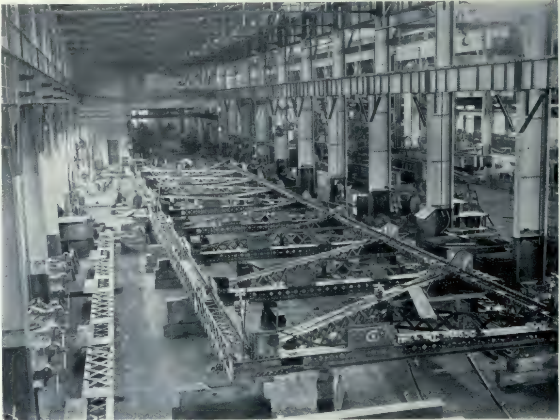
St. Andrew's Rapids Dam. View showing method of assembling and reaming trusses in shop before shipment. H. E. Vautelet, Consulting Engineer.
