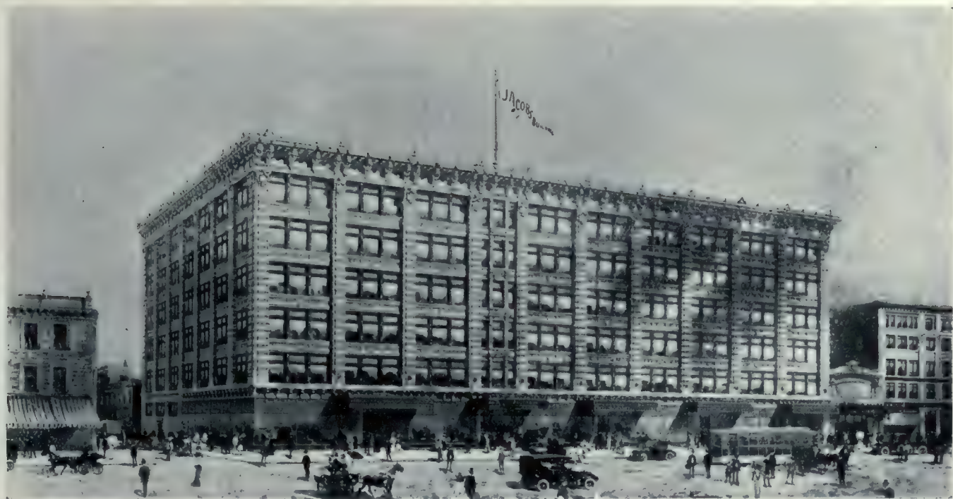
The new Jacobs Building, the largest reinforced concrete building in Canada, which is now nearing completion at the corner of St. Catherine and St. Alexander streets, Montreal. Mitchell and Creighton, Architects.
