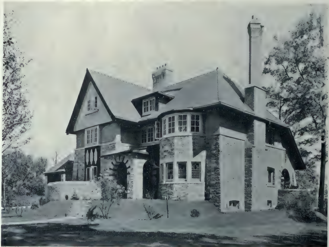
"Seven Oaks," the Home of Charles H. Fleming, Castle Frank Crescent, Toronto.—An Exceptionally Noteworthy Residence Which Exhibits a Feeling that is Strongly akin to the Rare Homelike Charm so Characteristic of the English Country House. The Beauties of the Site are Deserving of Especial Note, as are Also the Texture and Treatment of the Walls. The Stone Work, which is Built of Credit Valley, Blue Owen Sound, and Water-Rusted Lake Shore Stone, Lacks the Cold Grey Monotone So Often Seen in Residential Work and Unites with the Red Tile Roof and Verdant Tones of the Ground and Foliage to Make a Most Perfect Domestic Composition. Chadwick and Beckett, Architects.
