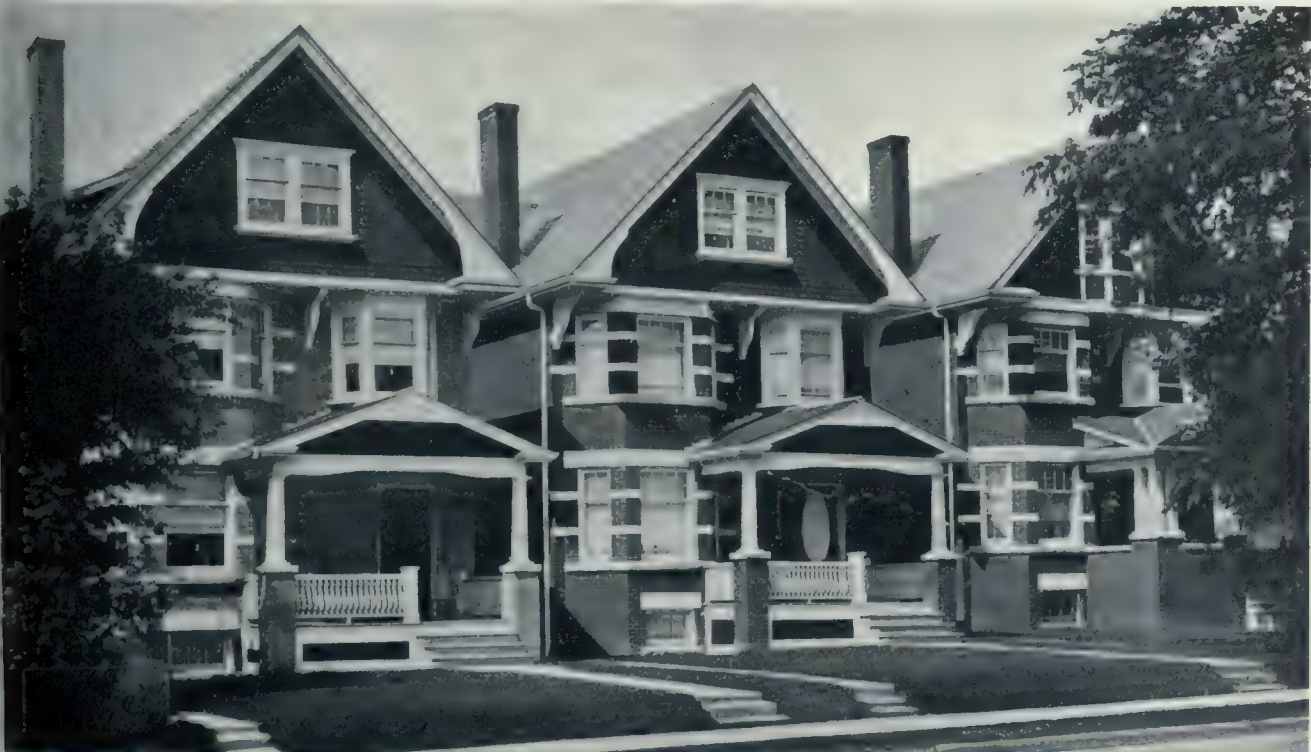
Dwellings, 276-278-280 Roncesvalles Avenue, Toronto. These buildings illustrate the possibilities of ROMAN STONE for trimmings on the moderate-priced dwelling.
