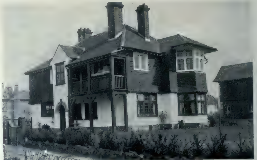
House at Parklangley, Beckenham. One of the Type of Houses Now Being Built According to the Garden Suburb and Town Planning Idea, on a Wooded Estate About Twelve Miles from London, for Families of the Middle Class. Reginald Fry, Architect.
