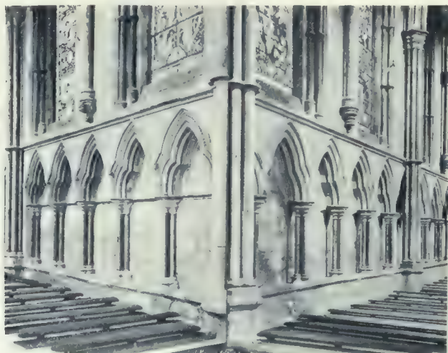
Vail Arcade, South Side, and Nave Arcade, North Side.
