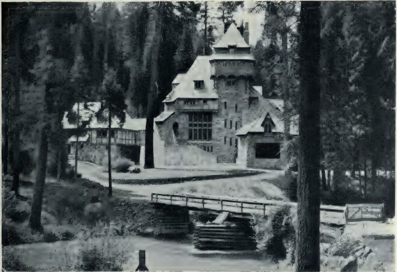
"Mytoon"—"A Mediæval Castle" Designed for a Summer House for Mrs. Phoebe Hearst in the Primeval Forest of Northern California. Note How Perfectly the Architect has Succeeded in Creating a Design that Conforms with the Site and Harmonizes with the Clusters of Giant Trees that Surround it. The Crowning Walls on the Tower and Main Building as Well as the Projecting Attics Were Necessary Because of the Heavy Snowfall. Maybeck & White, Architects.
