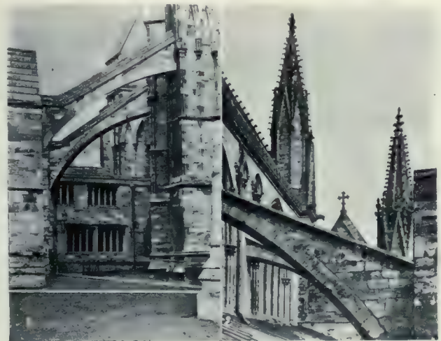
1. Flying Buttress of Chapter House. 2. Flying Buttress Connected on Exterior of Clerestory to Resist the Thrust of the Stone Vaulting.
