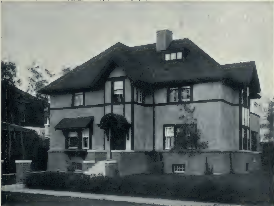
Residence of Mr. F. Christie, Winnipeg. J. D. Atchison, Architect. Herringbone Metal Lath used in these outside walls.
