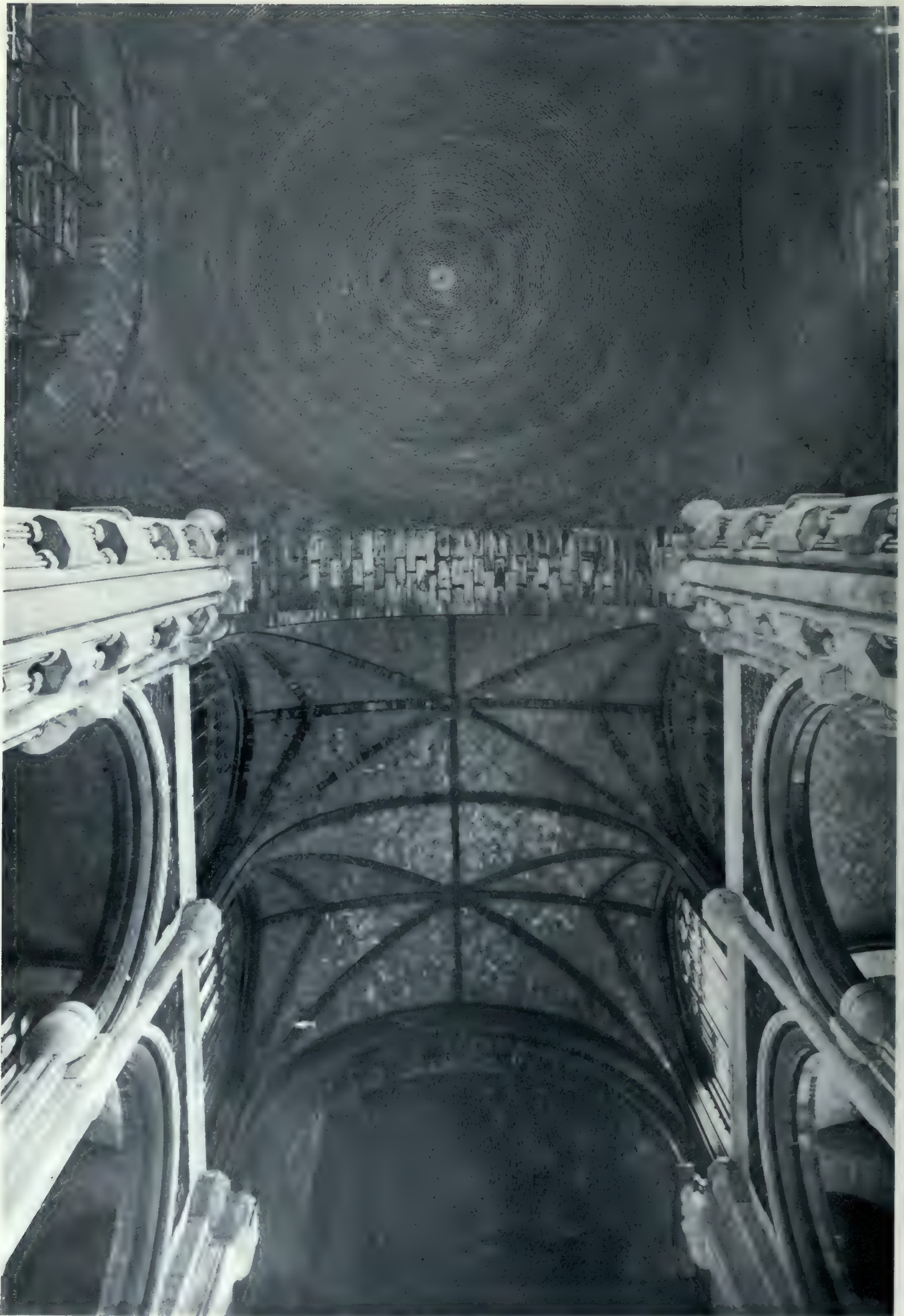
View of dome and vaulting over retrochoir, Cathedral of St. John the Divine, showing the detail of Columns, arching and groin work.
