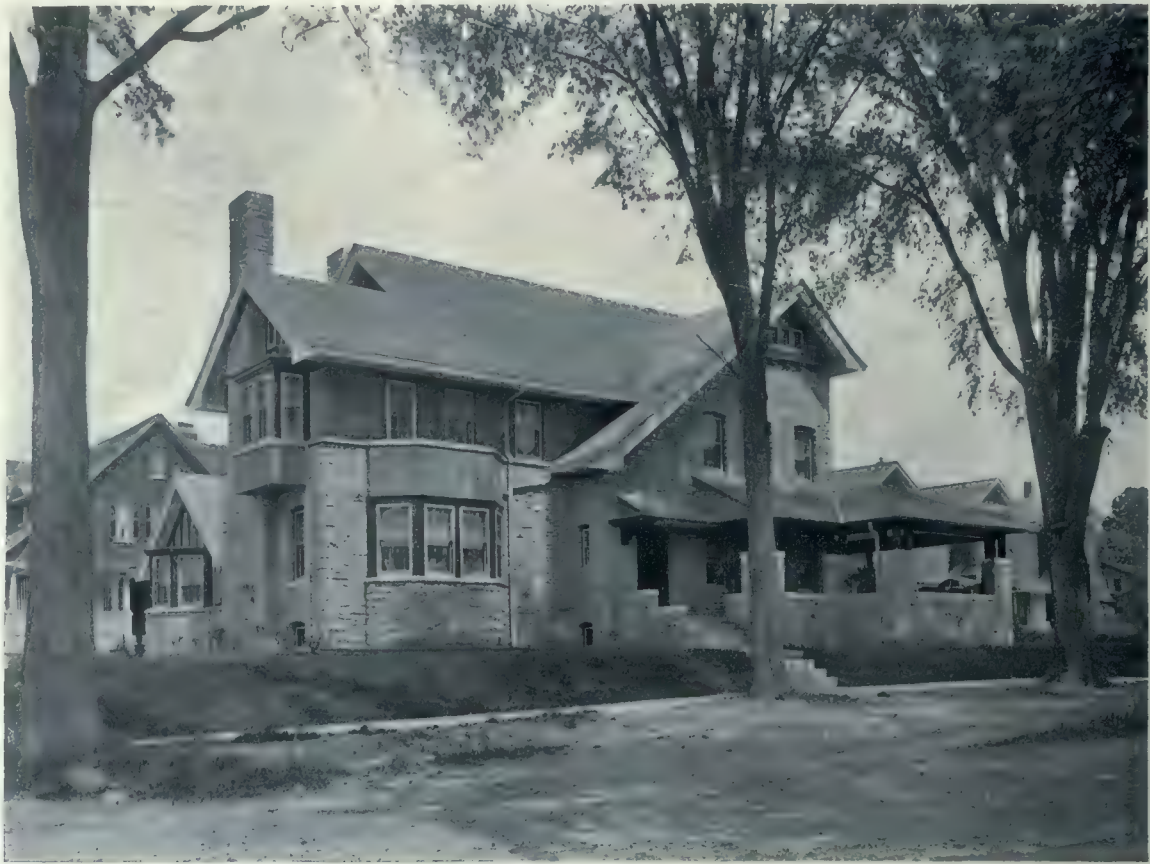
Home of A. W. Taylor, St. Catharines, Ont. Built of Credit Valley Broken Ashlar, with Cement Stucco Above the Second Storey Sills. The Roof is of Slate and the Color of the Woodwork, Brown. Bond and Smith, Architects.
