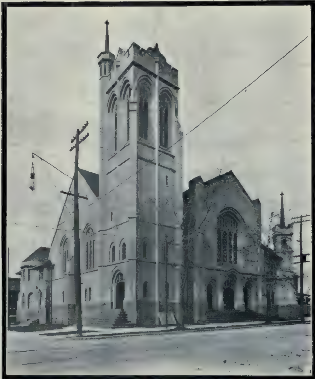
A Sand-Lime Ecclesiastical Edifice—High Park Presbyterian Church, Roncesvalles Avenue, Toronto. Smith and Gemmill, Architects.
