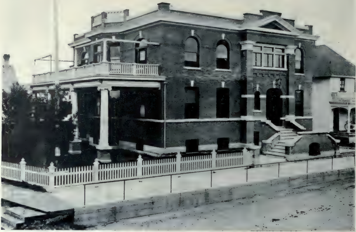
The Edmonton Club, Edmonton, Alta., which has a membership of over 200 professional and business men. This view shows the building as far as it has been completed. A large addition forming a part of the original scheme is to be built to the right of the entrance, thus making the structure one of the most commodious and best appointed club houses in Western Canada. A. M. Calderon, Architect.
