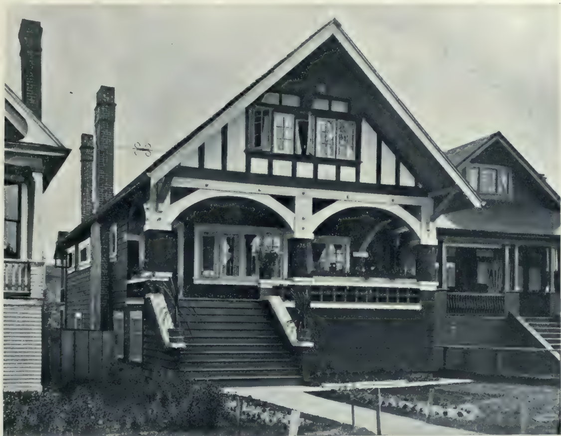
Bungalow of H. J. Simmons, Vancouver, B.C.—The Low, Broad Lines and Massiveness of the Design, make the Heavy Timber Effect and External Construction of this Dwelling Eminently Suitable. E. Stanley Mitton, Architect.
