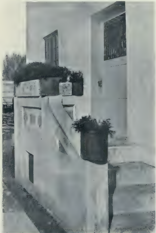
Side Entrance, Concrete Residence at Brantwood, Maryland. Milton Dana Morrill, Architect.
