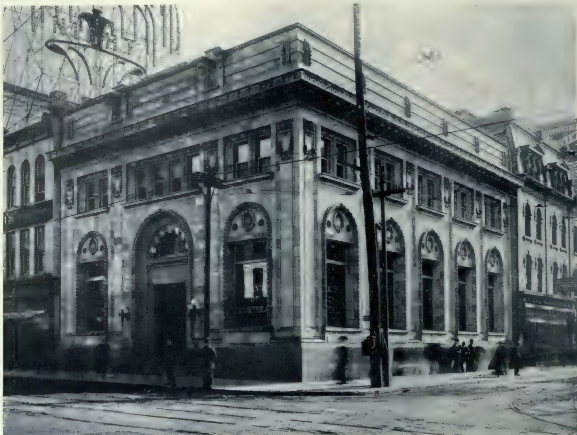
New Premises, Bank of Montreal, Yonge and Queen Streets, Toronto. A Recently Erected Building Which Shows an Interesting use of Terra Cotta in Commercial Design. Darling and Pearson, Architects.
