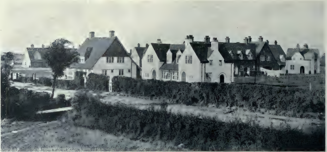
Cottages at Westholm, Letchworth. These Houses were Built by a Co-operative Tenants' Society on a Self Supporting Basis. Note the Extreme Simplicity of the Elevations and Delightful Harmony of the General Scheme. Parker and Unwin, Architects.
