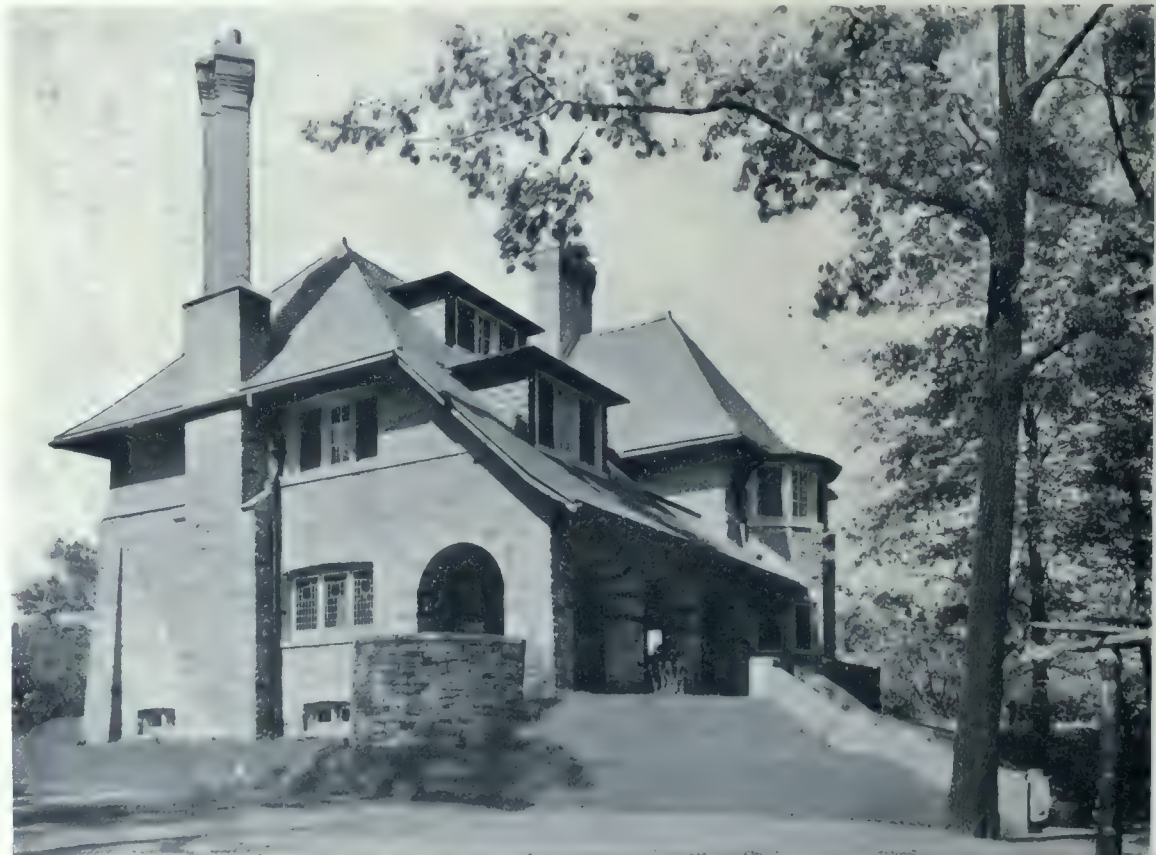
"Seven Oaks," As It is Seen from the Rear. The View Shows the Sunken Garden and the Arcade Openings and Comfortable Lines of the large South-Fronting Verandah Which Overlooks one of the Prettiest Parts of Rosedale Ravine. The Roof Lines have a Picturesque Quality and the Over-hang of the Eaves a Sheltering Sense that Renders the Whole Both Private and Restful. Chadwick and Beckett, Architects.
