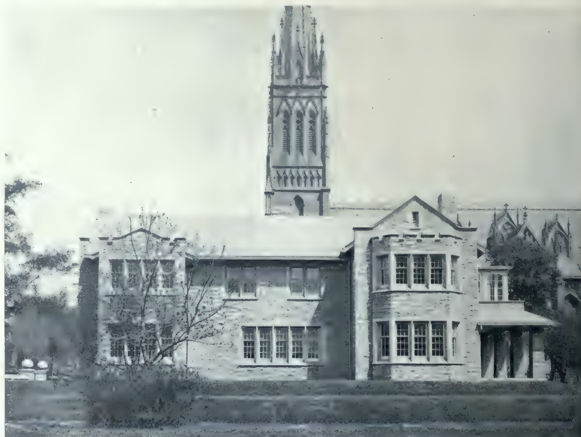
South Wall of Parsonage, Metropolitan Church, Showing St. Michael's Cathedral in the Background. This Residence was Designed in the Elizabethan Style to Harmonize with the two Gothic Churches, Between Which it Stands. Sproatt and Rolph, Architects.
