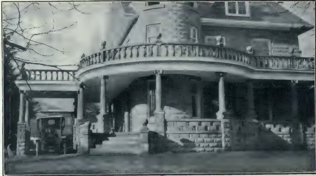
Residence of F. A. Fraser, Bowmanville, Ont., built entirely of concrete blocks.
