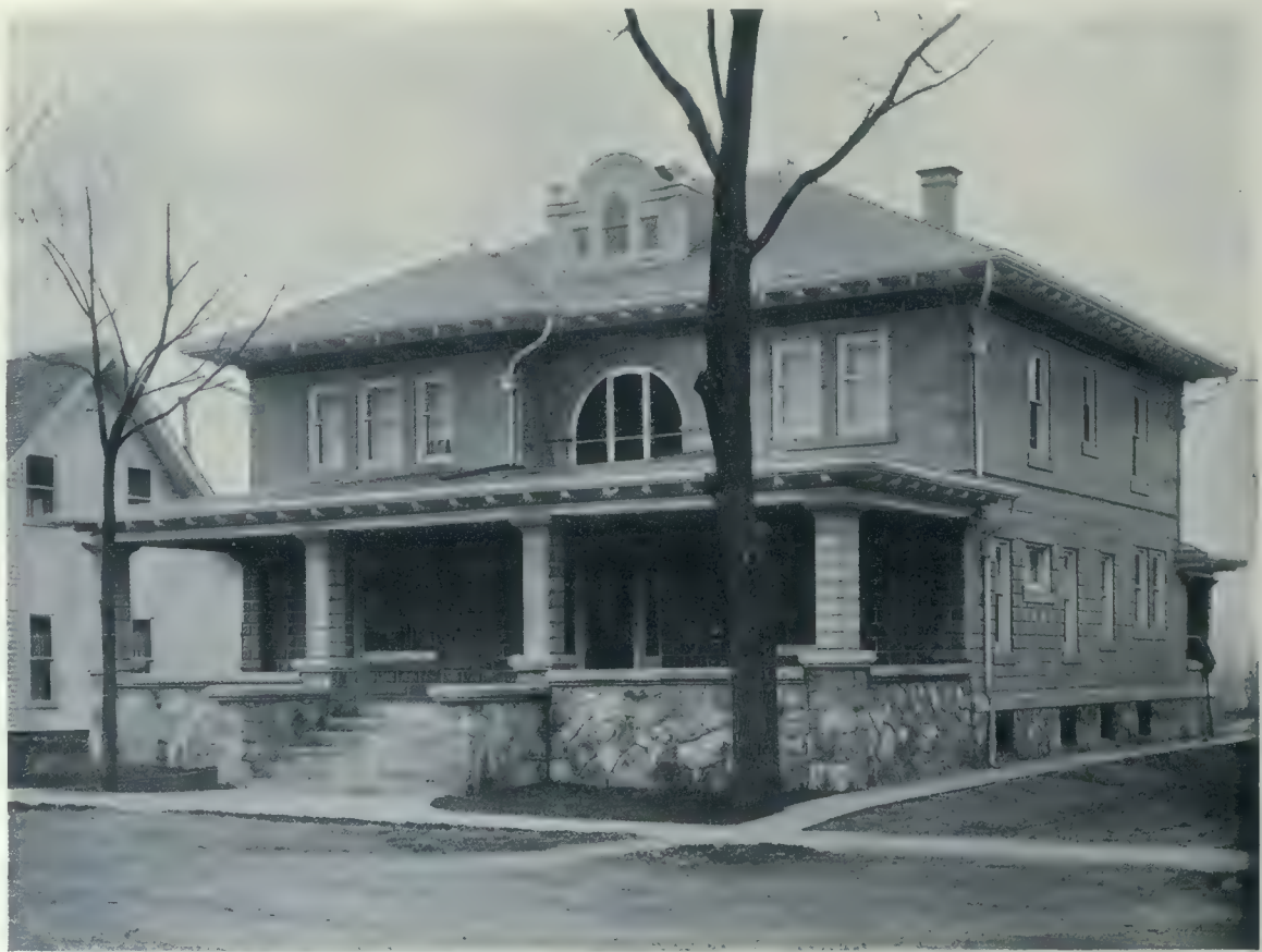
Residence of A. H. Brown, Leesburg, Indiana. Built of Bevel and Plain Cement Blocks. Note the Arched Window over the Verandah, and the Perfect Adjustment of the Material at all Wall Openings. Cosmo C. Elwood, Architect.
