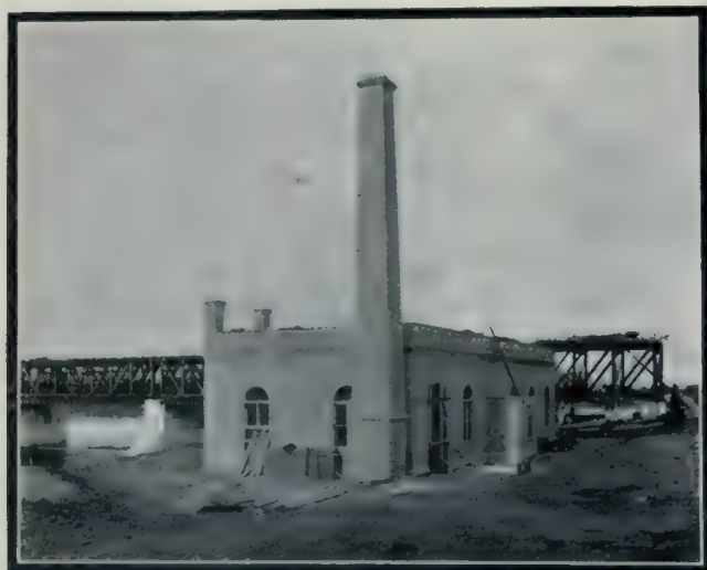
Power House, Built of Sand-Lime Brick, St. Andrew's Rapids Dam, Manitoba. H. E. Vautelot, Consulting Engineer.
