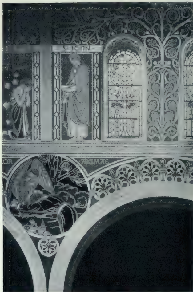
South Wall of All Saints' Church, Ennismore Gardens, London, showing the further possibilities of Sgraffito.
