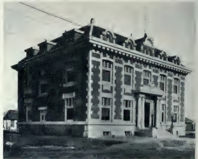
Court House, Saskatoon, built at a cost of $45,000. The walls are of red sand mould brick, with Tyndall stone trimmings, and the interior is finished throughout in quarter-cut oak. Storey & Van Egmond, Architects.
