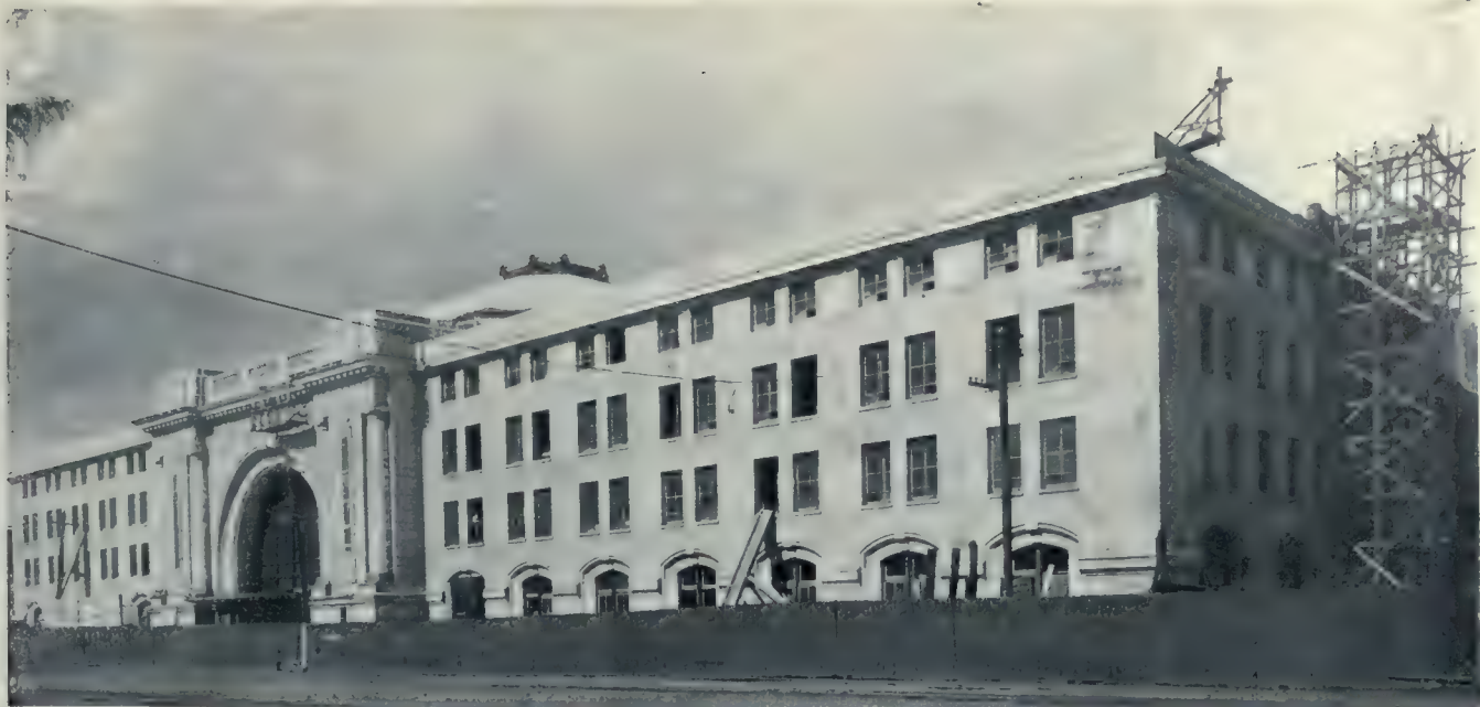
Fort Garry Station, Winnipeg—A $4,500,000 Terminal Building in Which the Only Bricks of the Vast Quantity Used, are of Sand-Lime Manufacture. Warren and Wetmore, Architects.
