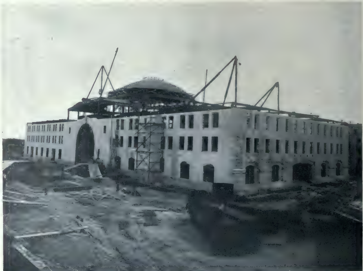
Fort Garry Station, showing the work well under way. When completed, Winnipeg will have the most modernly equipped terminal on the American Continent, if not in the entire world. Warren & Wetmore, Architects and Engineers.
