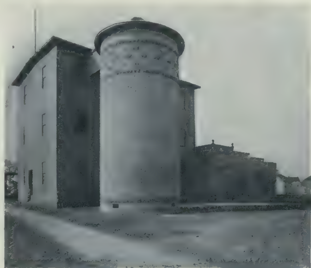
Grain Bin Erected at Marlon City, Michigan. Type of Building in which Concrete Block Construction, Owing to its Durable and Fireproof Qualities, is Being Extensively Employed.
