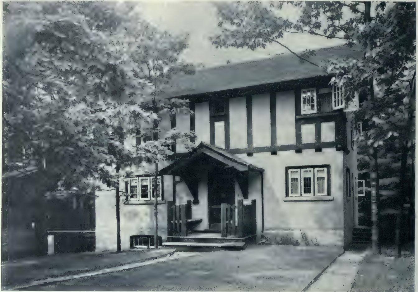
Residence of W. F. Temple, 106 Balsam Avenue, Toronto. An Attractive Small House Which Shows in an Interesting Manner the Use of Cement Stucco in External Construction. E. G. Wilson, Architect.
