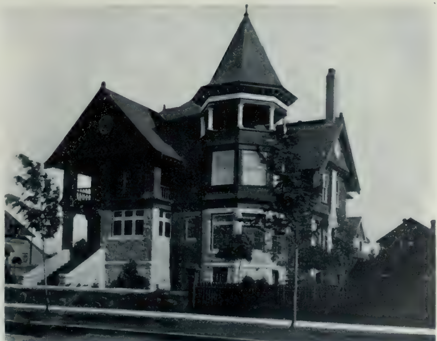
Residence of Mr. George Snyder, Victoria, B.C. An attractive Dwelling House of Frame and Stone Construction—a Combination of Materials Which is Quite Common in Residential Work Throughout the Extreme Western Section. Thos. Hooper, Architect.
