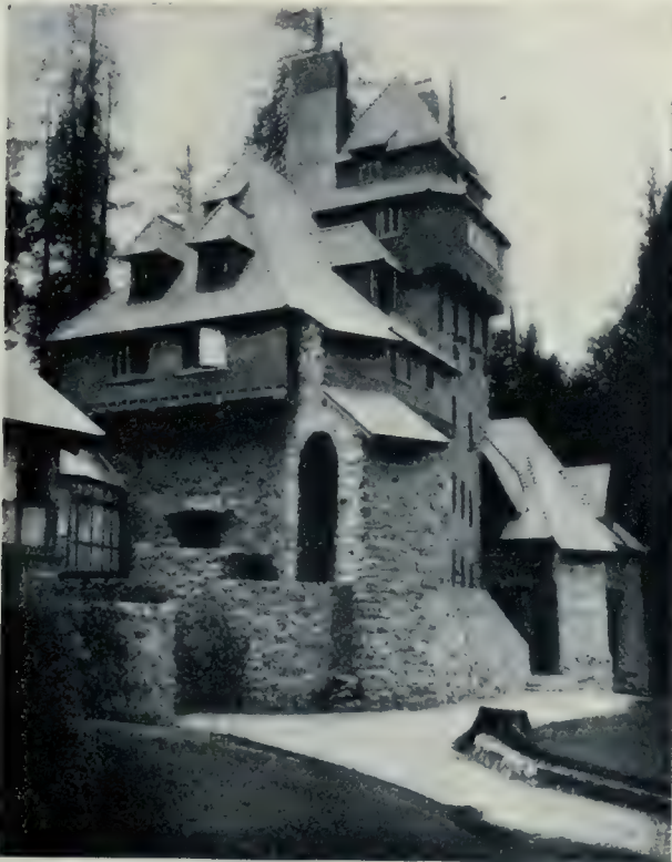
"Mytoon"—The Chief Feature of the Exterior is the Central Tower which is Seventy-five Feet High.
