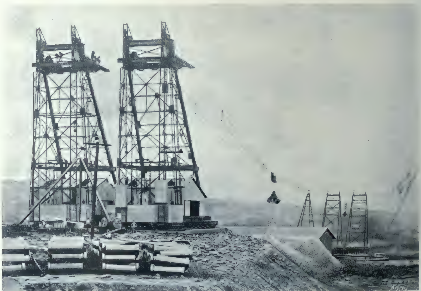
The Five High-speed Lidgerwood Cableways which are Handling, from Barges to the Storage Heaps, the 2,000,000 cu. yds. of Broken Stone and 1,000,000 cu. yds. of Sand Required to Build the Gatun Locks at Panama Canal.
