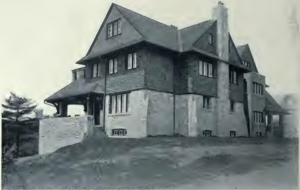
Residence of Howard Bovell, 50 Western Avenue, Toronto. An Interesting South-Fronting House in Which the Main Rooms are Arranged to Obtain the Advantage of a Picturesque Ravine Which the Site Overlooks. The Lower Walls are of Fleming Quarry Stone, and the Upper Portion and Roof of Brown Stained Shingles. Chadwick and Beckett, Architects.
