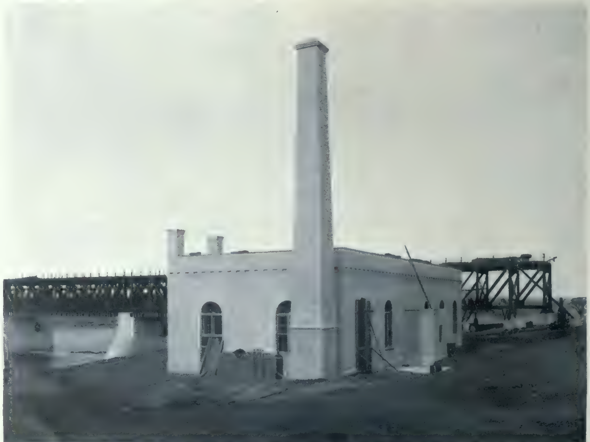
View of Power House, St. Andrew's Rapids Dam, in which the power used for operating the dam is generated. H. E. Vautelet, Consulting Engineer.
