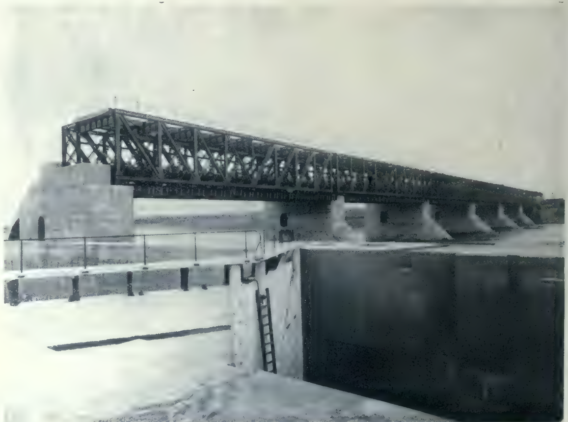
View of St. Andrew's Rapids Dam, showing the steel superstructure with curtain frames raised, as they will appear during the Winter and early Spring. The lock gates around the west end are shown in the foreground. H. E. Vautelet, Consulting Engineer.
