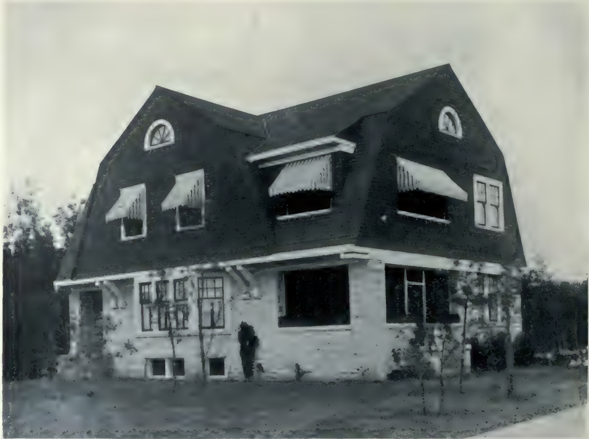
Home of Dr. K. C. Campbell, Ruskin Row, Winnipeg, an interesting example of a mansard-roof residence in which Tyndall stone and stained shingles are attractively combined. J. D. Atchison, Architect.
