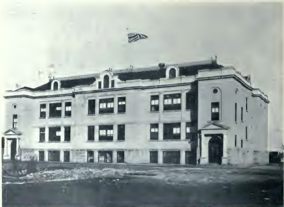
Lord Selkirk School. Another of Winnipeg's new school buildings. This structure was built simultaneously to the King Edward School, and cost $53,000. The walls of both buildings are lined with hollow tile, to which the plaster is directly applied.
