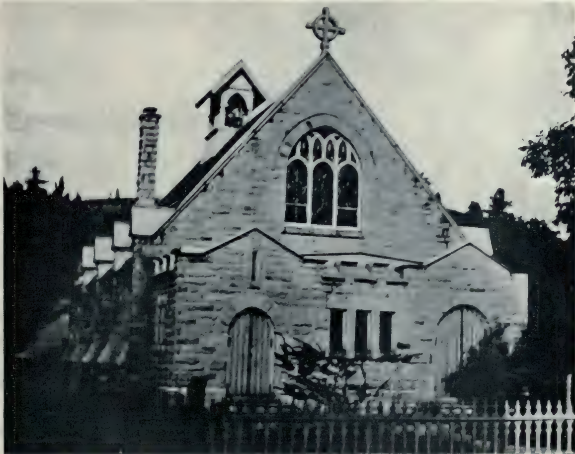
St. Alban's Episcopal Church, Glen Williams, Ont. F. S. Baker, F.R.I.B.A., Architect.
