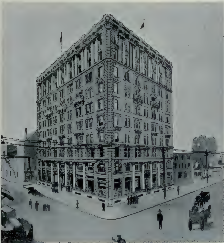
Perspective View of Ten Story Fireproof Office Building now in Process of Erection at the Corner of Hastings and Howe Streets, Vancouver, for the Dominion Stock and Bond Company. It will be of Steel Frame Construction Encased in Concrete, with Granite Exterior Walls. Thos. Hooper, Architect.
