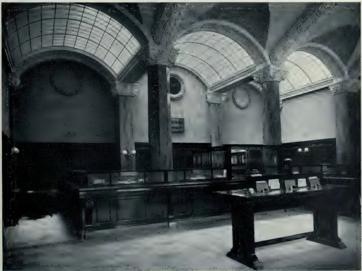
Banking Room, New Premises, Bank of Montreal, Queen and Yonge Streets, Toronto. Showing the Arched Skylights and the Treatment of Side Walls and Ceiling. Darling and Pearson, Architects.
