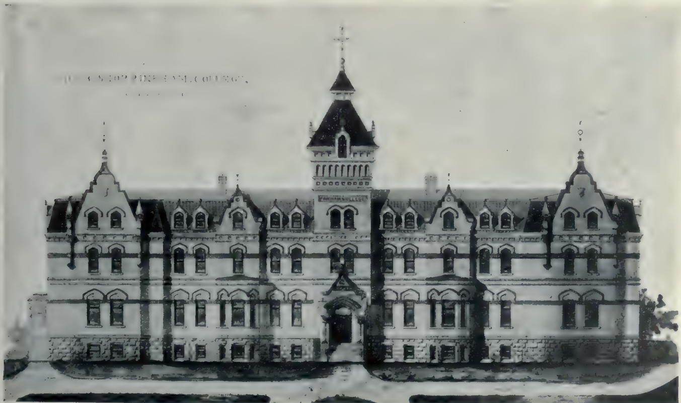
The Bishop Pinkham College, one of Calgary's architectural assets in the way of an educational institution. Hopkins & Wright, Architects.
