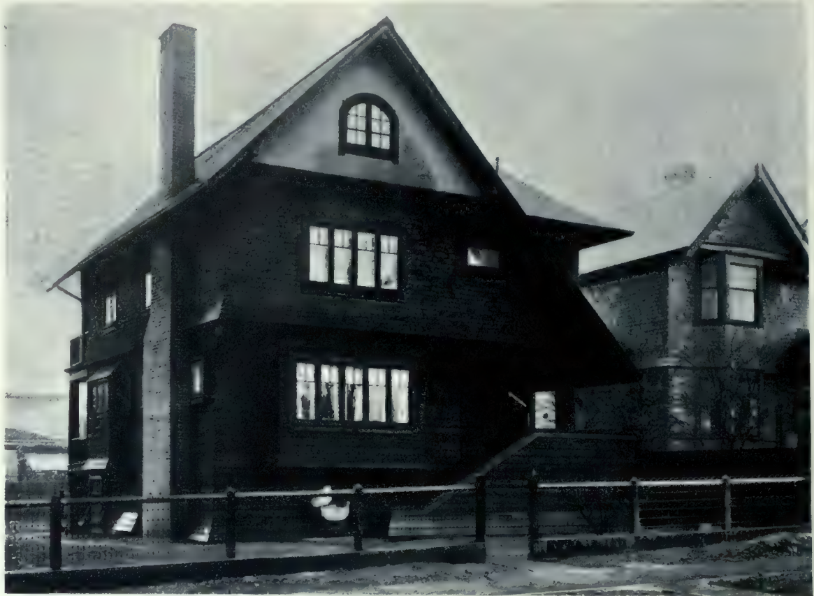
Residence of H. D. Hulme, Vancouver—A Clapboard and Shingle House, which Typifies the Construction Usually Prevalent in British Columbia for Small Moderate Priced Dwelling Structures. E. Stanley Mitton, Architect.
