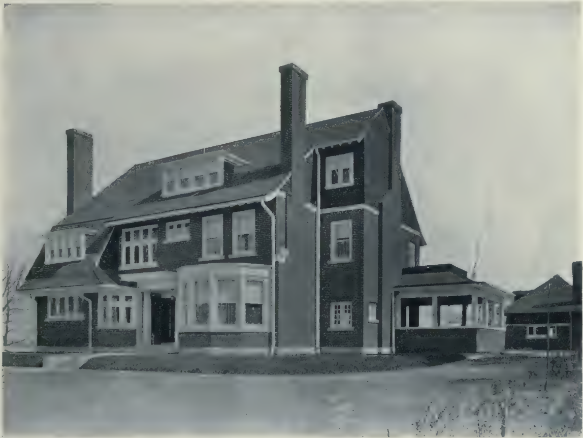
Residence of S. F. May, 81 Binscarth Road, Toronto. Spacious Grounds and a Magnificent View down the Don Valley renders this Attractively designed House Particularly Adapted to the Character of the Site. Wickson and Gregg, Architects.
