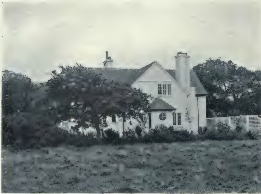
House at Bromborough, Cheshire. A Most Commendable Little Structure Whose Charm and Beauty lie in the Simplicity of Its Design and Color Scheme. The Walls are of Brick, Roughcasted and Limewhited, and the Roof is of Tile. P. Morley Holder, F.R.I.B.A., Architect.
