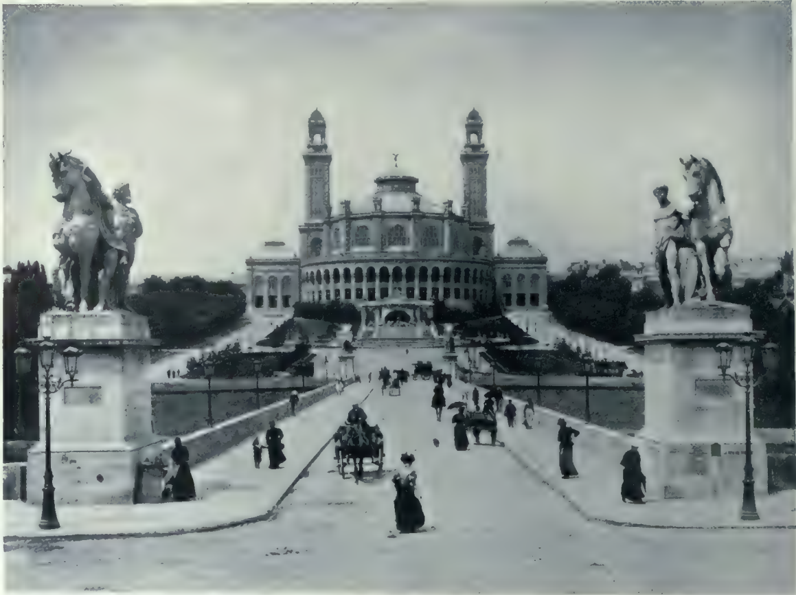
Font d'Iena—Showing the Continuous Roadway Effect, Which is a Prominent Feature of Parisian Bridges.
