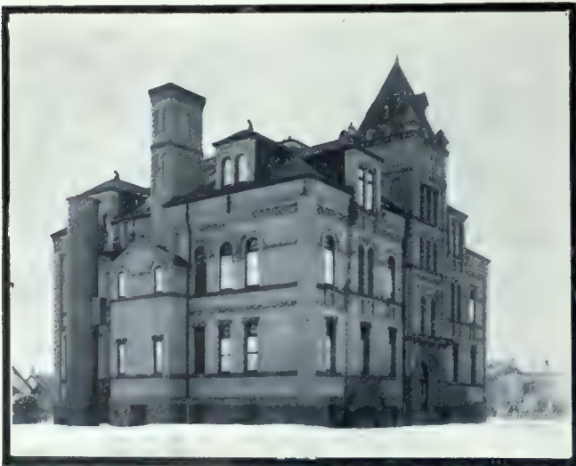
Dufferin School, Which, Together with Other Buildings of Similar Character Illustrated on this Page, Shows the Extent to Which Sand-Lime Brick is used in Winnipeg Schools. Designed by Commissioner of School Buildings J. B. Marshall.
