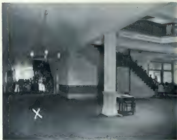
The main corridor of the Ogden School, Toronto, showing the course taken by the children in their fire drill. "X" marks the location of the boilers under the main corridor.
