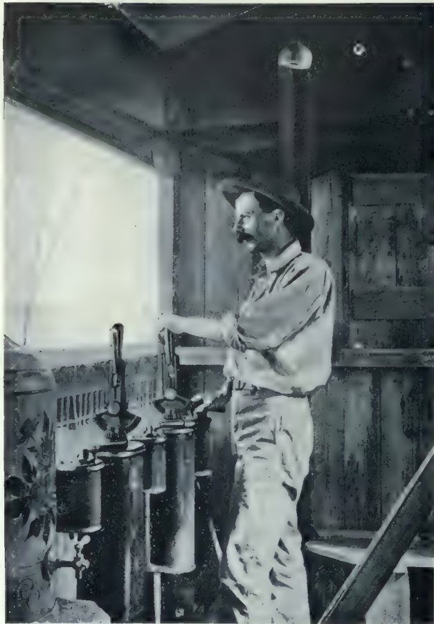
One of the Cableway Operators in His Booth, Showing the Simple Apparatus with which He Controls the Operation of the Bucket and Carriage.
