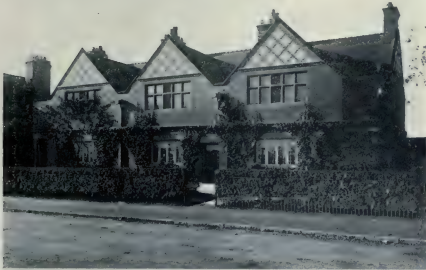
New Chester Road, Port Sunlight. Brick Walls Relieved with Stone Trimmings, Constitute the Outer Garb of this Interesting Series of Dwellings. The Gables, Executed in Dark and Light Brick, add a Decorative Touch, both Simple and Effective.
