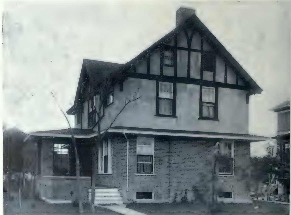
Home of C. D. Shepard, Winnipeg. A noteworthy moderate sized dwelling with red brick and cement stucco walls and half timbered gables. Herbert B. Rugh, Architect.
