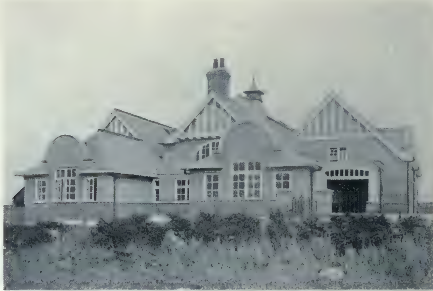
School House built at Westerhope, Eng., by the Northumberland County Council. Note the general architectural treatment, so decidedly in contrast with the average rural school building in Canada.
