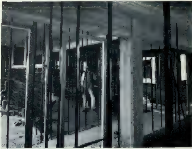
Fireproof partitions in "Men's Own" Building, Winnipeg. John D. Atchison, Architect.
