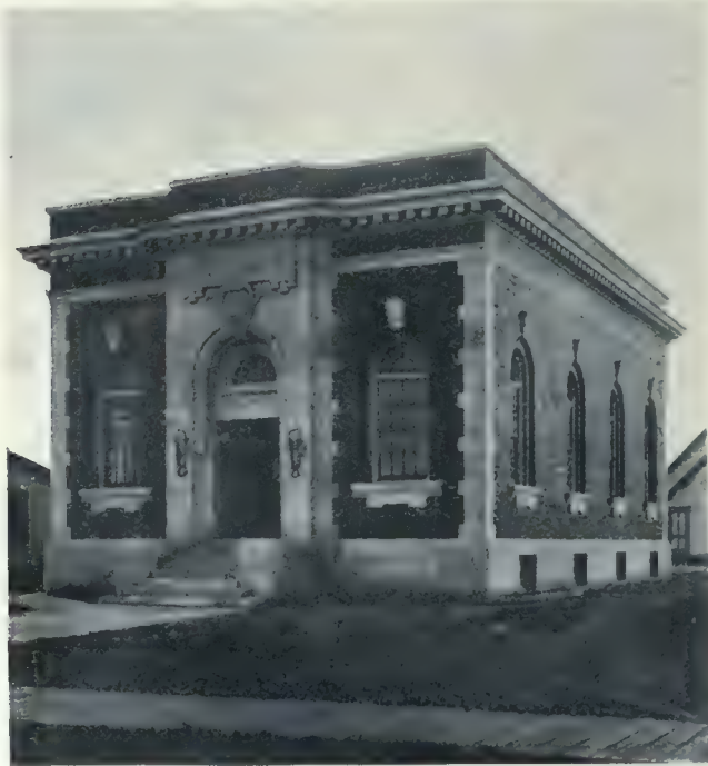
Land Titles Building, Saskatoon, said to be the most thoroughly built fireproof structure in Western Canada. It is constructed of dark brown clinker brick, with Tyndall stone trimming, the floor and roof being concrete, the partitions hollow tile, and the doors and windows of the most approved fire-resisting type. Storey & Van Egmond, Architects.
