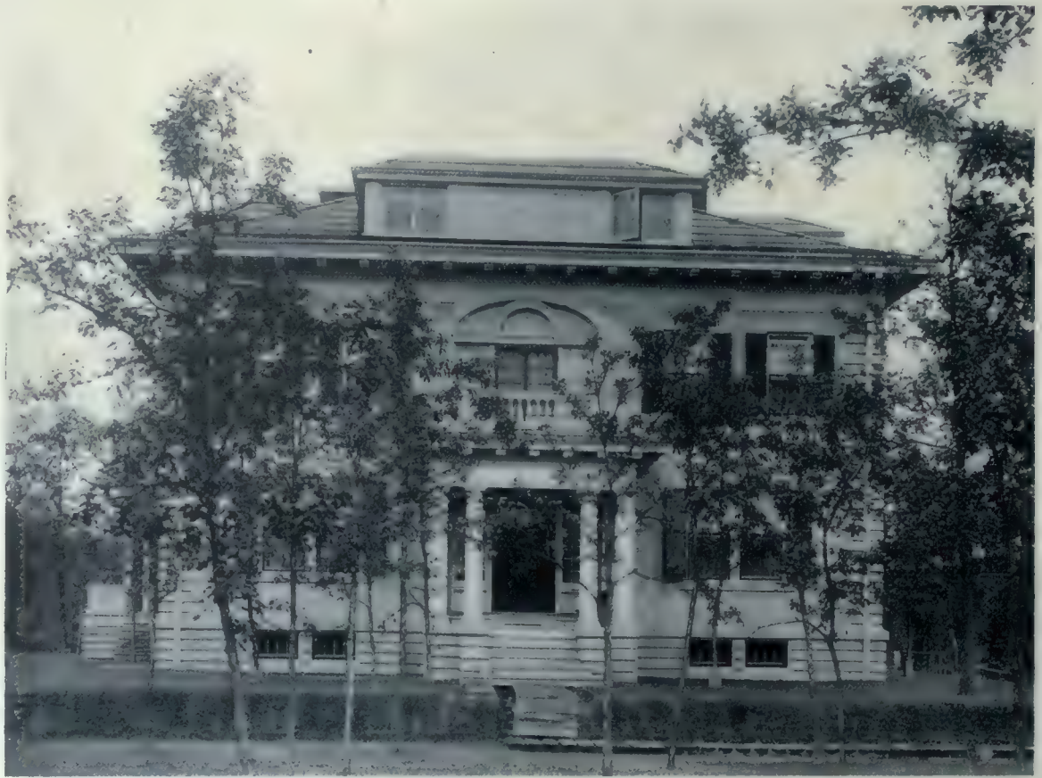
Home of J. Y. Reid, Winnipeg, a concrete residence in modern Colonial design, the stone, which is made of white Portland cement, ground stone, white sand and marble dust, being hollow, tool faced, and of the color and texture of natural stone. Herbert B. Rugh, Architect.
