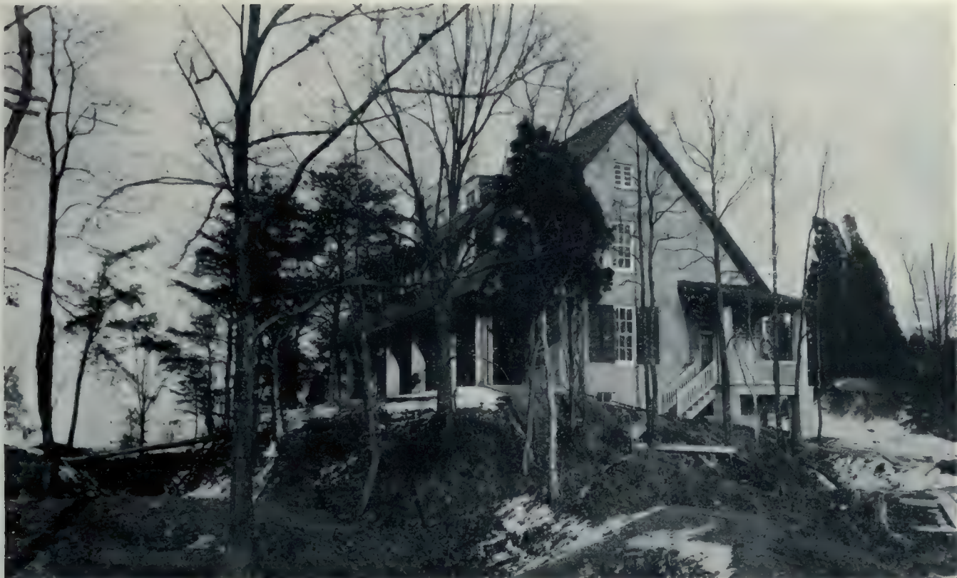
An attractive reinforced concrete residence with a red tile roof and a picturesque setting. Milton Dana Morrill, Architect.
