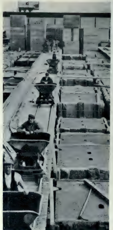
BLOCKS WAITING TO BE PLACED IN POSITION.
