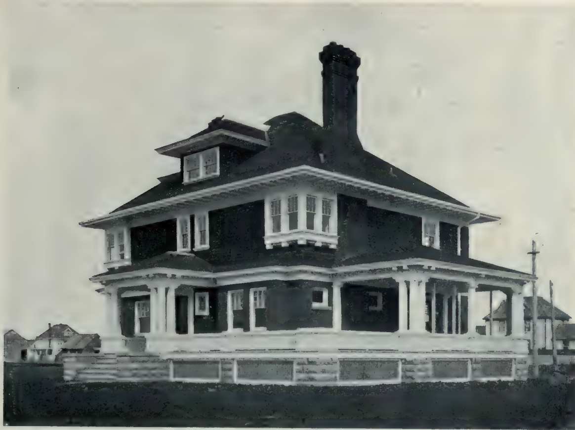
Residence of Joseph Campbell, Regina. Comfortable lines and pleasing color scheme serve to make this home an attractive abode. The walls for the first storey are red brick, with dark brown shingles above, the roof being green and the woodwork white. J. H. G. Russell, Architect.
