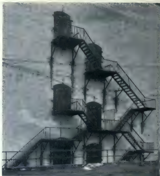
The system of outside stairways with which the Royal Alexandra Theatre is equipped. If theatre-goers are entitled to this fire protection, we ask why our school children should not receive some consideration.
