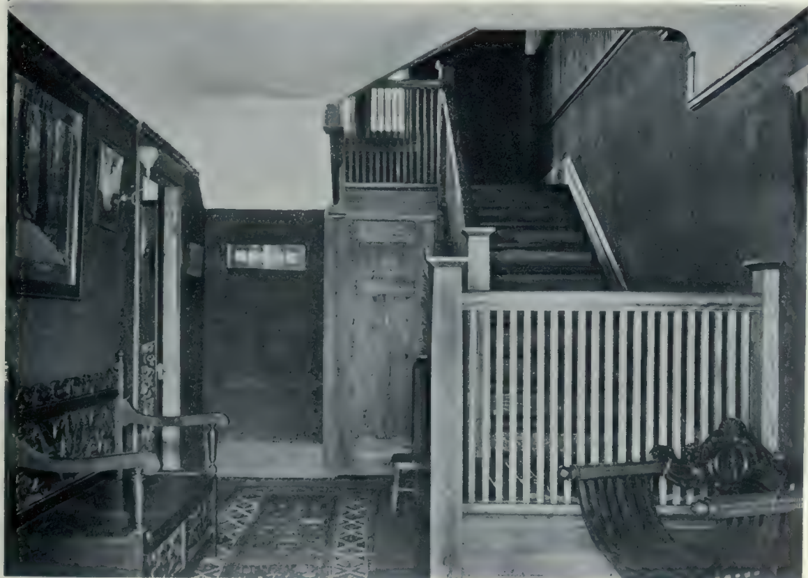
Hallway, Residence of C. Cambie, 34 Poplar Plains Road, Toronto. Finished in Hardwood, Stained a Silver Grey, with harmonizing Wall Treatment. Bond and Smith, Architects.
