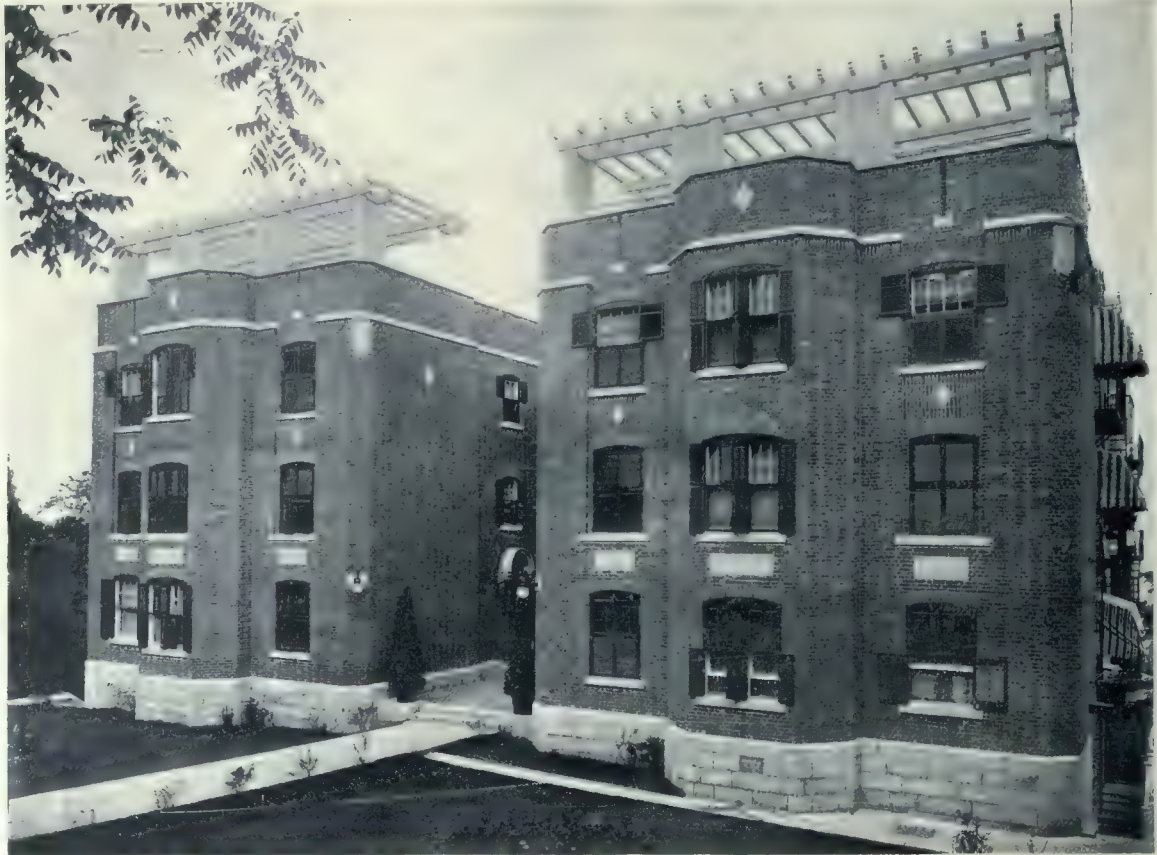
An Unusual Adjunct of the "Travancore" is a Roof Pergola an Excellent View of which is Obtained Herewith. This Innovation Suggests Certain Possibilities in "Roof Gardening" which Might Well be Considered by Architects in Providing Outdoor Advantages, Especially where the Ground Dimensions are Restricted on All Sides.
