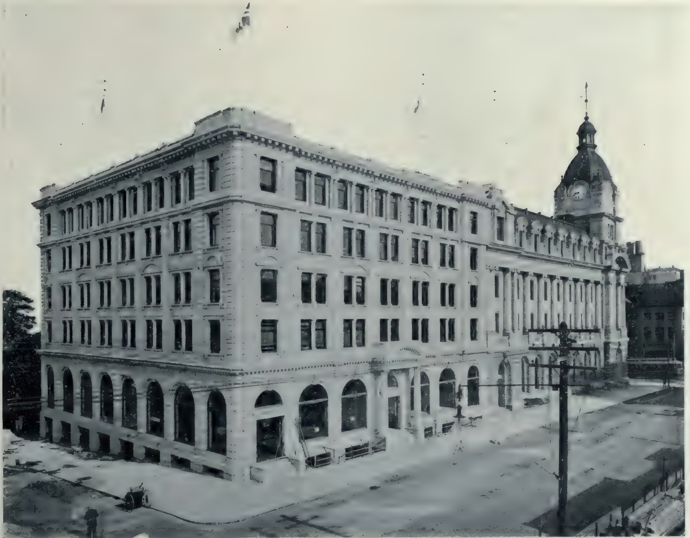
The new Winch Building, Corner Hastings and Howe Streets, Vancouver, B.C. A Handsome and Substantial Commercial Structure Recently Erected in the Centre of the City's Business District. It is Designed to Carry Two Additional Storys and is of Fireproof Construction Throughout. On the Other Corners of this Intersection are to be Built Three Ten Story Office Buildings, One of Which is Now Well Under Way. Hooper and Watkins, Architects.
