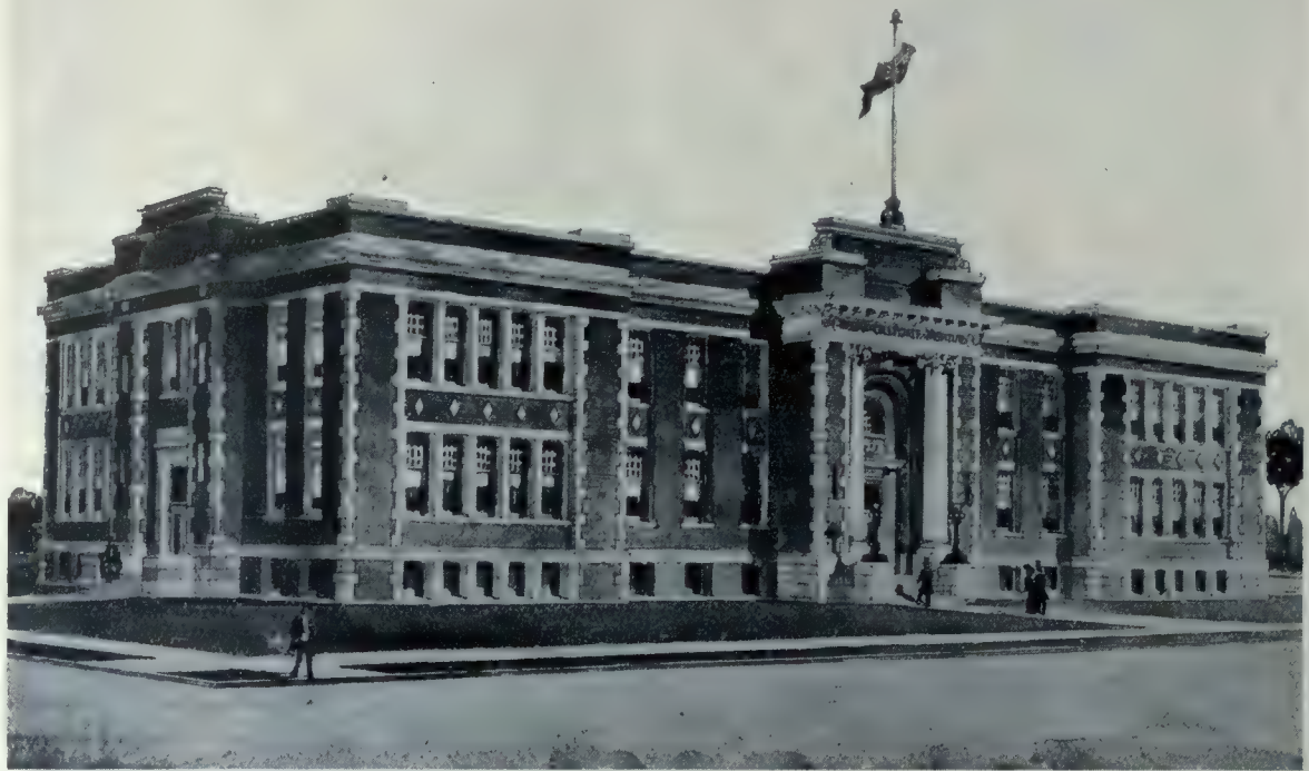
Regina's new Collegiate Institute, built at a cost of $110,000. An evidence of the safe and substantial manner in which the West provides for the housing of her school children. The building is practically fireproof, the walls being of buff brick and Tyndall stone, the floors of reinforced concrete and the partitions of the metal stud and metal lath type.
