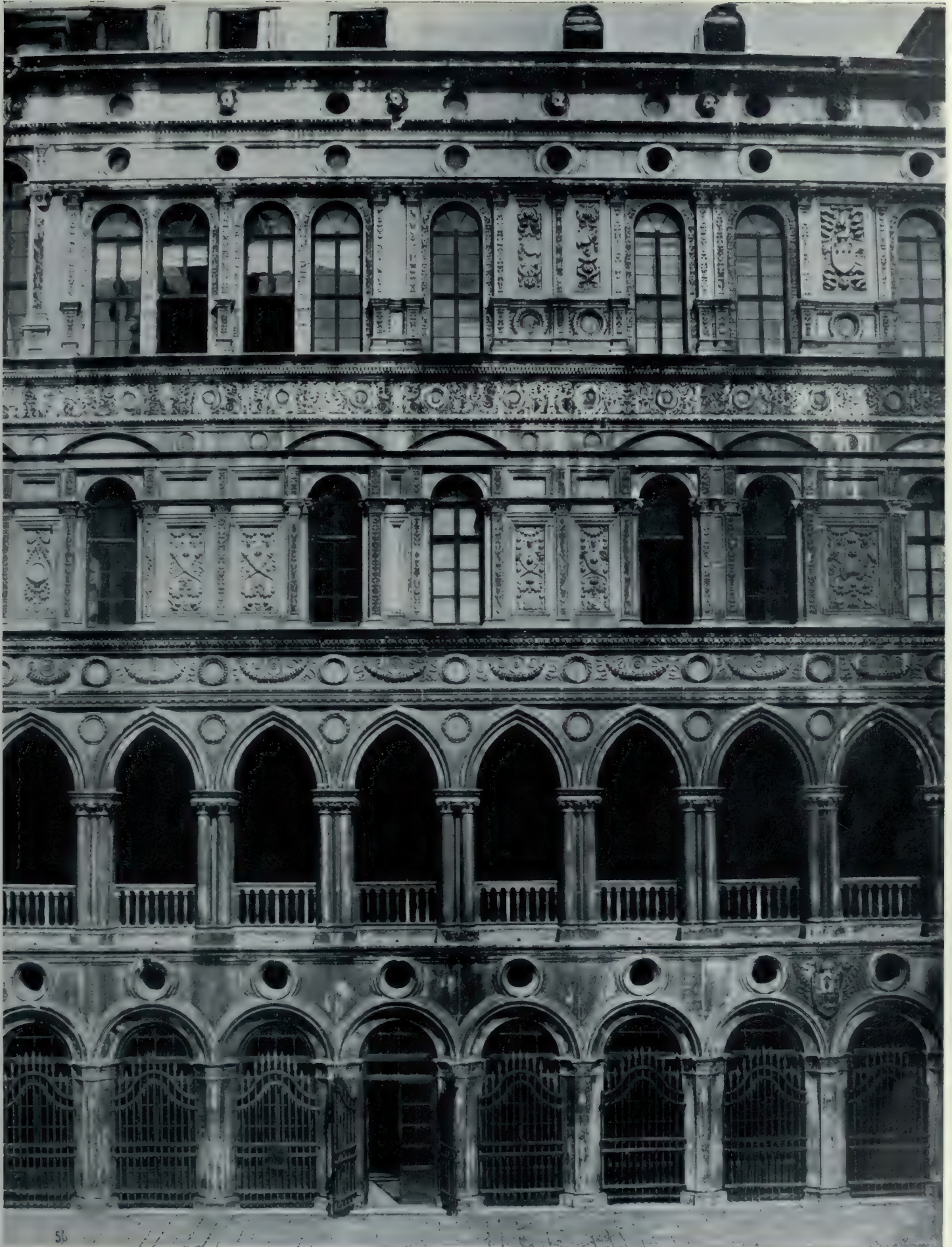
Section of Elevation in Court, Ducal Palace, Venice, showing the Decorative Enrichment of the Walls, and the General Arrangement of the Windows in the Upper Stages.
