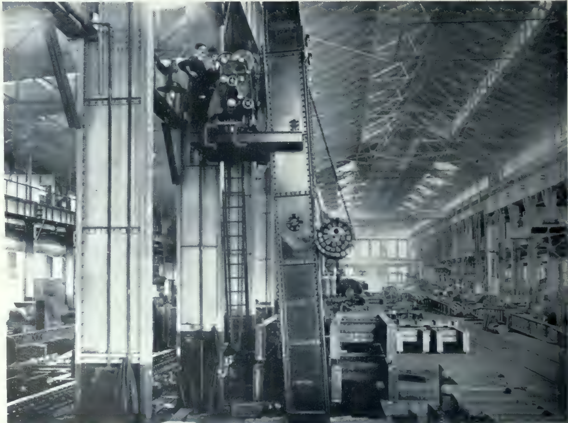
St. Andrew's Rapids Dam. View showing method of assembling and operating curtains in the shops before shipment. H. E. Vautelet, Consulting Engineer.
