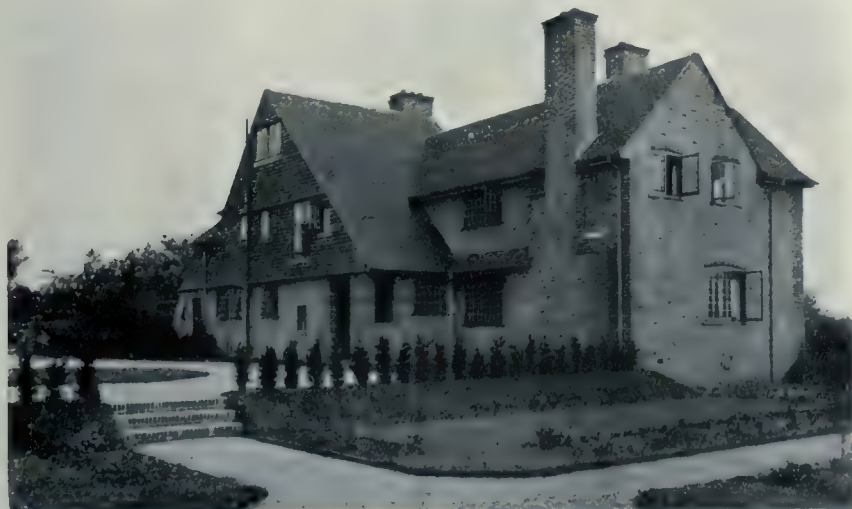
Rear View, House at Walton Heath. Accidental Varieties in the Coloring of the Grey Brick, Together with Flat Laid Tile Courses and the Red Tile Roof, Make the External Composition of this House Unusually Attractive. P. Morley Horder, F.R.I.B.A., Architect.
