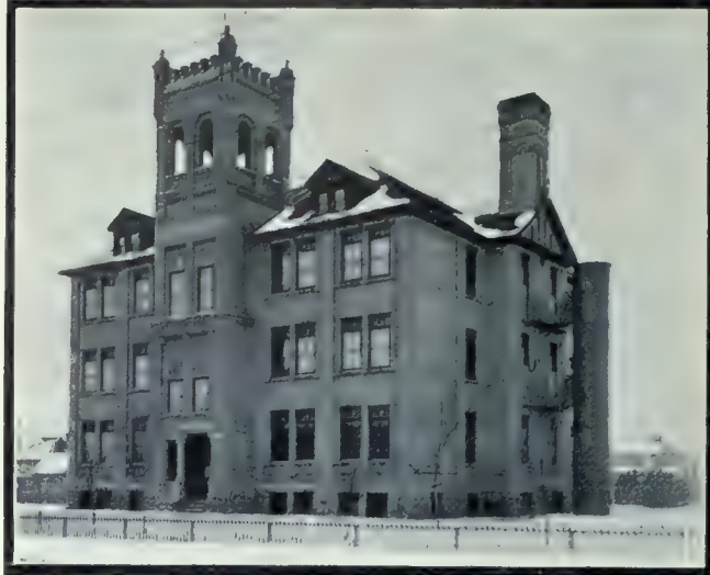
Somerset School—Another of Winnipeg's Sand-Lime Brick School Structures. Designed by Commissioner of School Buildings J. B. Mitchell.
