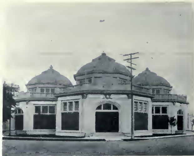
Railway Exhibit Building, Canadian National Exhibition Grounds, Toronto. A structure that is unique in design and arrangement, being in the form of a trefoil and removed from the conventional style of Exhibition buildings. Mr. Geo. W. Gouinlock, Architect.
