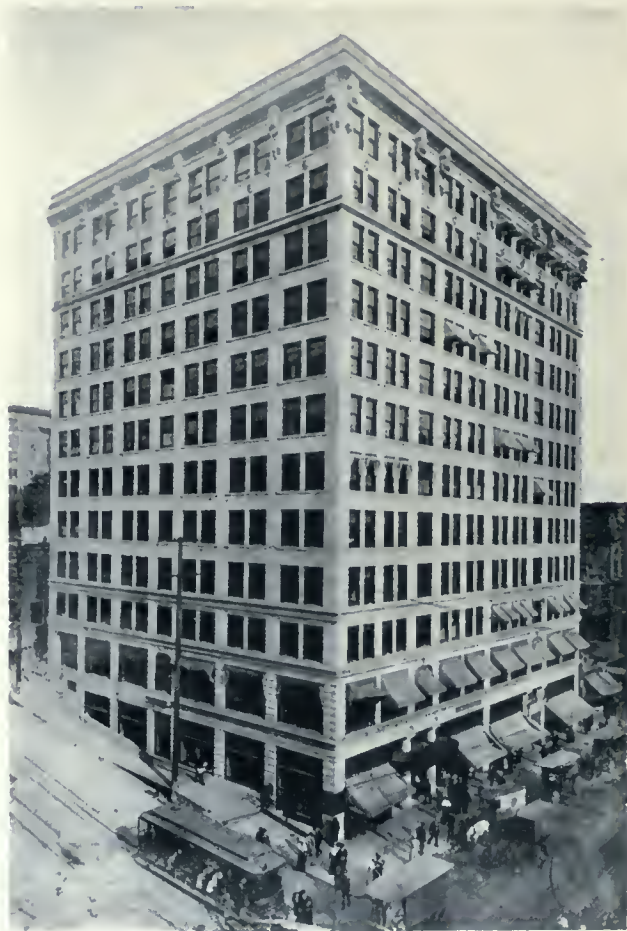
EMPIRE BUILDING, SEATTLE. A. WARREN GOULD, ARCHITECT. ANOTHER EXAMPLE OF HIGH OFFICE BUILDING CONSTRUCTION OF WHICH THE ENTIRE FRAMEWORK IS OF REINFORCED CONCRETE CONSTRUCTION.
