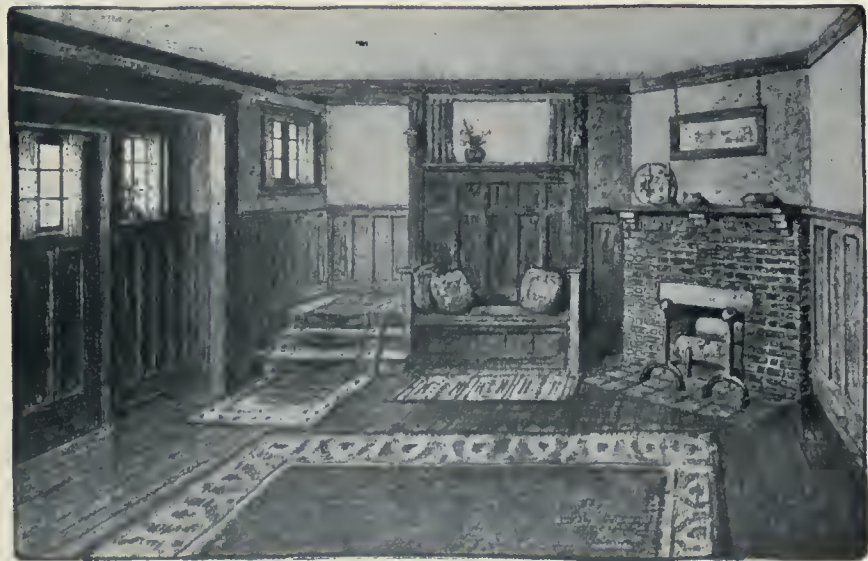
Fireplace and stairway in living room of Design No. 5. The fireplace is built of red brick, being thrown diagonally across the corner and carried up to the height of the wainscot, where a stone lintel forms a projecting shelf.
