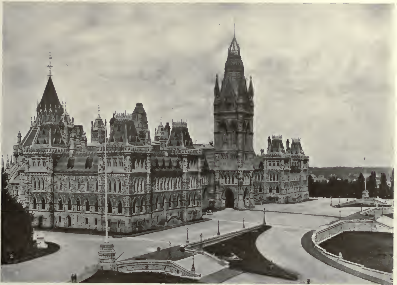
PLATE VI. THE CENTRAL OR PARLIAMENT BUILDING ON A WIDE TERRACE, SHOWING THE NUMEROUS, AND PARTLY CONTINUOUS, WINDOWS, WITH DEEP MOULDED JAMBS, AND EFFECT OF SOLID WALL WITH RICH HORIZONTAL DECORATION.
