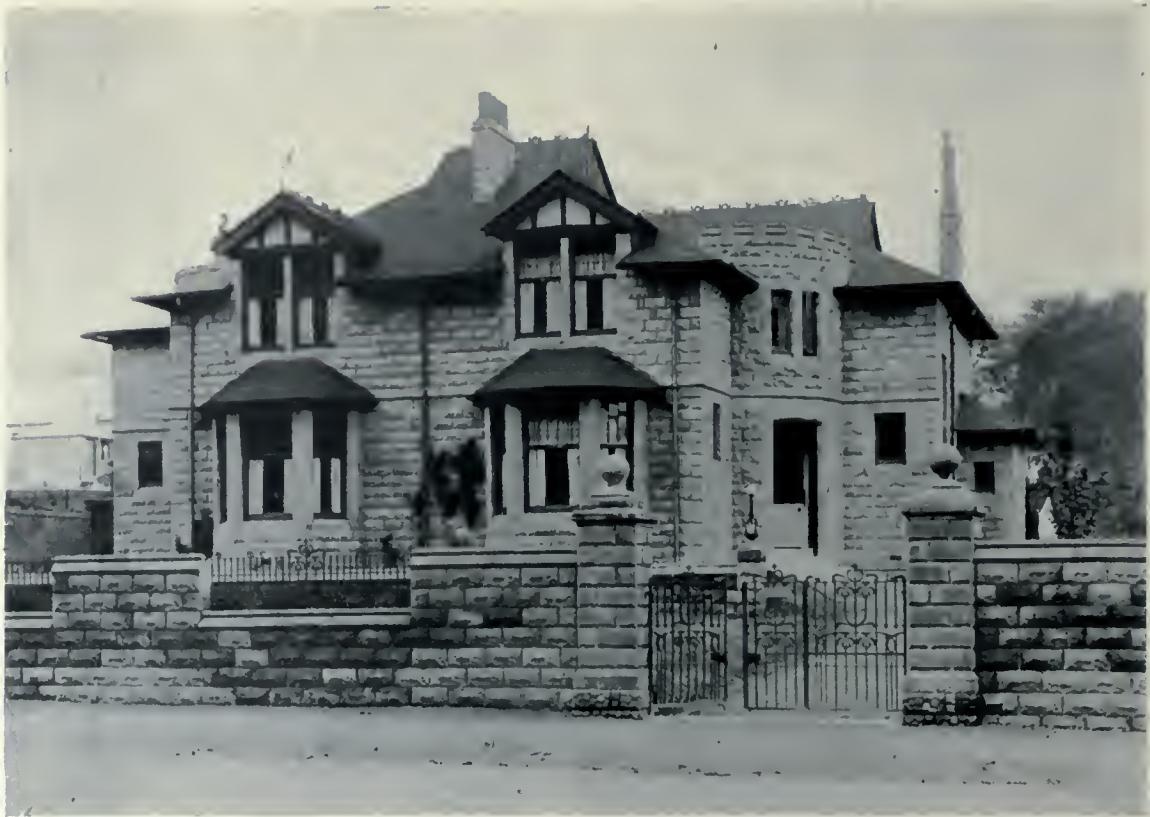
This house shows the introductory use of concrete blocks in Scotland. It is a two-family dwelling located on the main Glasgow Road, Paisley, and was the first concrete block house built at that place. Note how carefully the architectural and constructive detail has been considered and the thorough manner in which the work has been executed.
