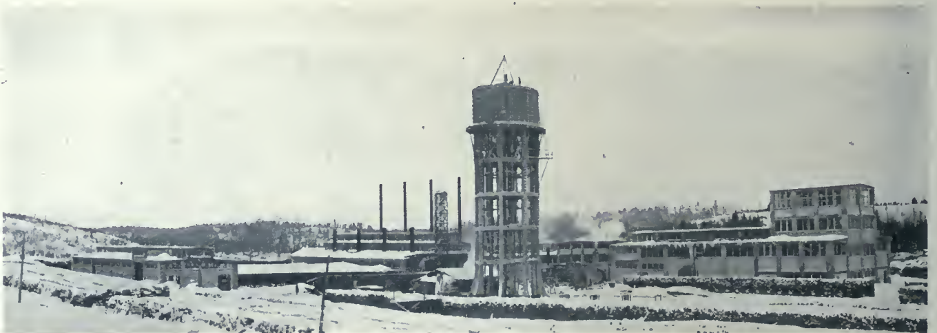
Panoramic view of new plant of Wood Product Company, Dysart, Ont., taken from the west, Dec. 15th, '08, showing the plant completed with the exception of the water tower, which remain only to be stripped. E. D. Pitt, designing and constructing engineer.
