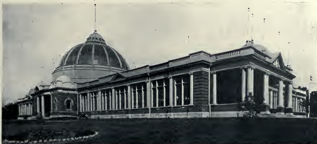
Horticultural Building, Canadian National Exhibition Grounds, as seen from the main approach. One of the most successfully designed buildings in the entire Exhibition group. It is of red pressed brick construction, with gray stone trimmings, trussed steel roof and concrete floors, and cost, complete, $97,000. Mr. Geo. W. Gouinlock, Architect.
