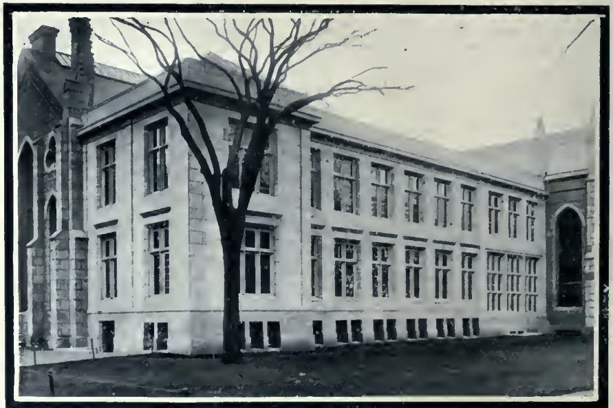
Gore Hall (Library Building) Harvard University, showing concrete addition in the foreground. The surface of the concrete in which the selected aggregates are revealed, has the appearance of Quincy Granite and strongly simulates the natural stone used in the original building.
