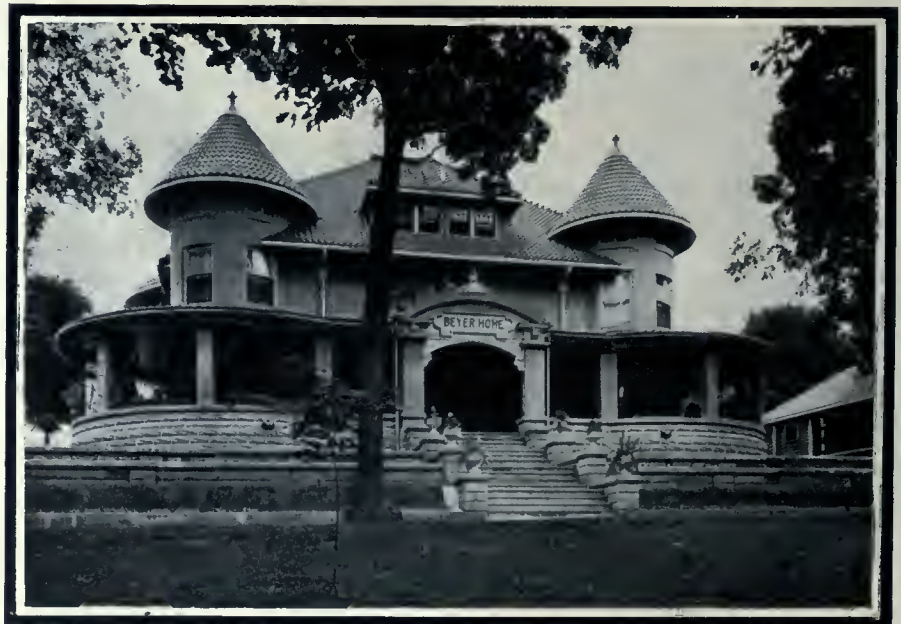
Summer residence of Beyer Bros., at Winona Lake, Indiana, erected at a cost of $13,000. The first story consists of alternating courses of 8-inch and 4-inch rock face blocks, while the second story and towers are built of plain blocks.
