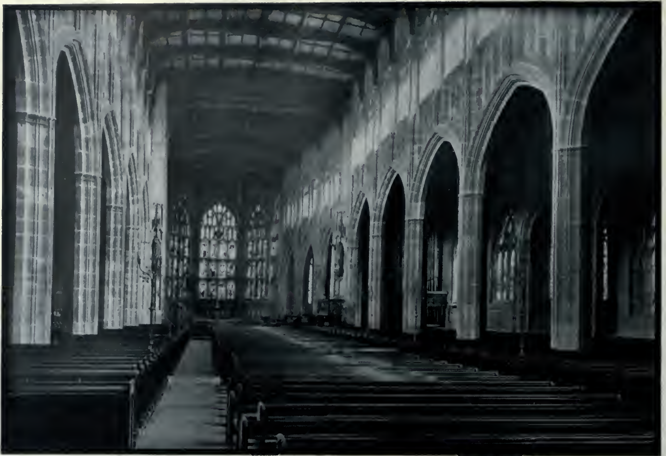
INTERIOR VIEW ST. MICHAEL'S COVENTRY, SHOWING THE OPEN TIMBER ROOF WITH BRACED ARCHES WHICH DATES FROM THE PERPENDICULAR PERIOD, AND THE BEAUTIFUL EFFECT IT HAS PRODUCED.
