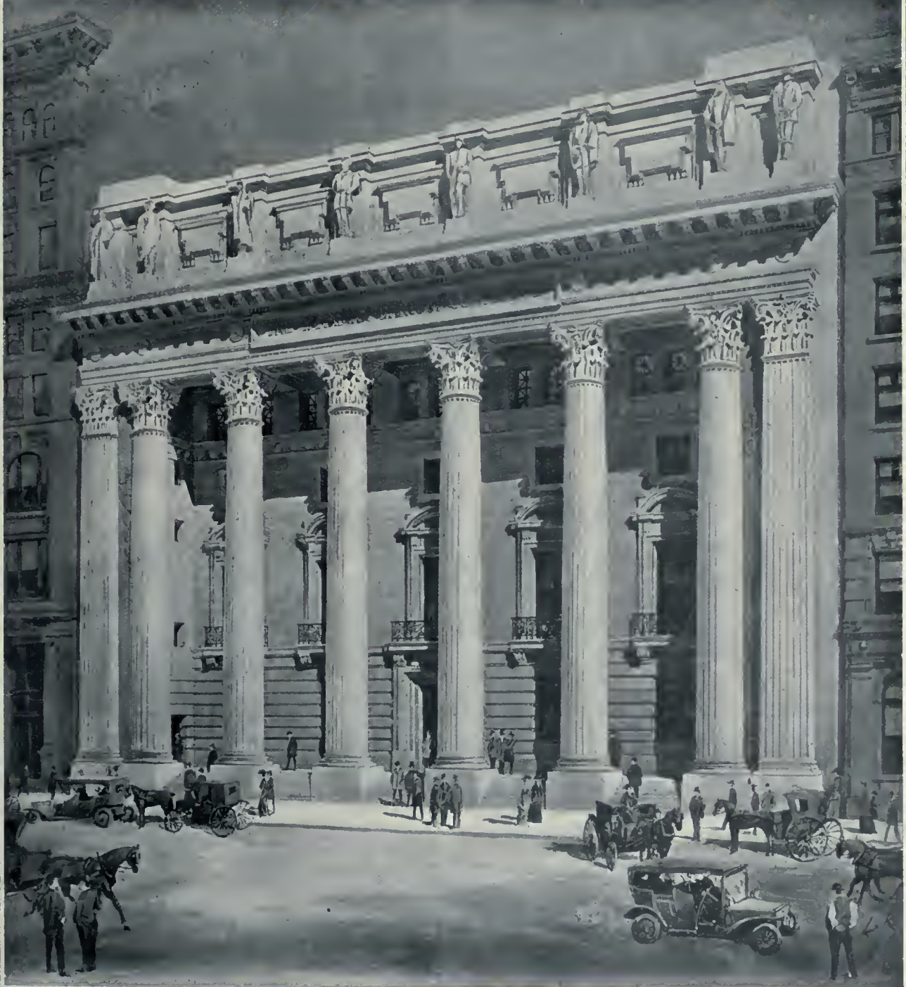
New Canadian Bank of Commerce Building, Montreal—Darling & Pearson, Architects.
