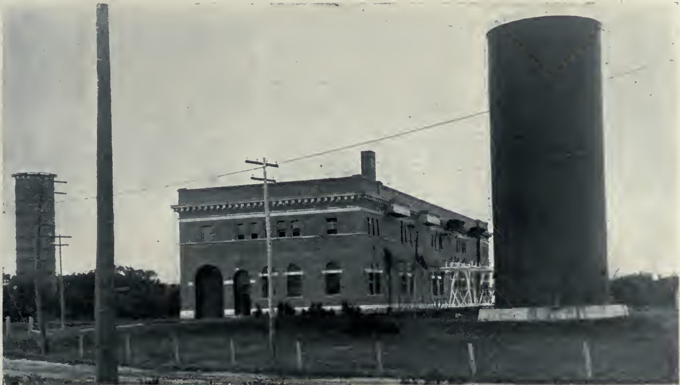
Transformer Station, plant of the Electrical Development Company, Niagara Falls, Ont. E. J. Lennox, Architect.
