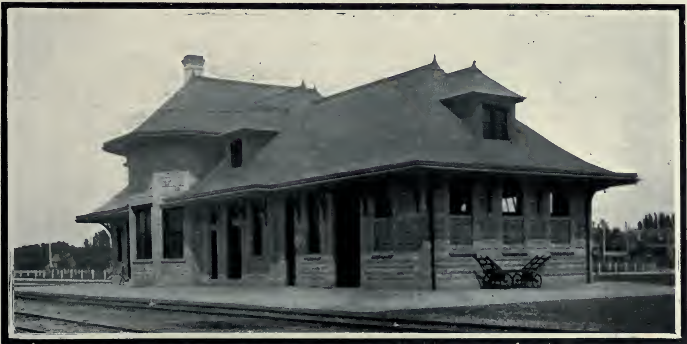
Passenger Depot, O. S. L. Railway, Payette, Idaho. A highly acceptable design carried out in concrete blocks with buff brick trimmings.
