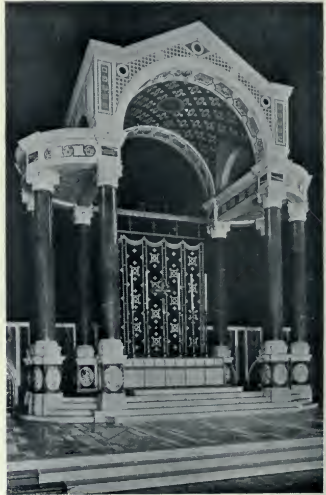
The Baldachino, New Catholic Cathedral at Westminster, London. An exquisite canopy of white marble, carved, paneled and inlaid with lapis-lazuli, and supported by eight monolith marble columns. The Altar beneath is a solid block of granite weighing fourteen tons. Every marble column in the building is a monolith. Mr. John Francis Bentley, Architect.
