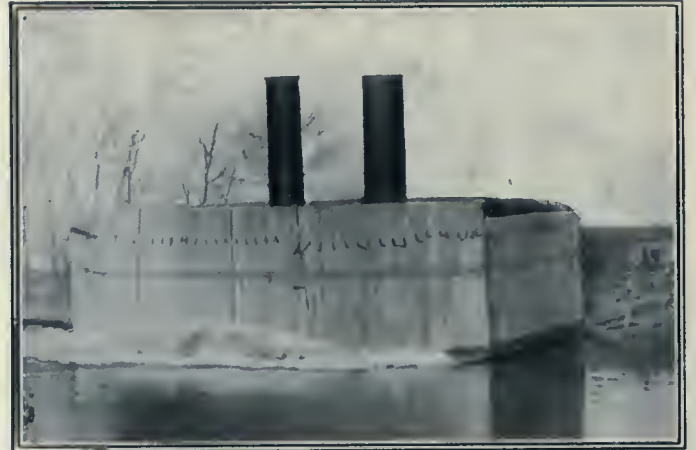
LAUNCHING A CAISSON FOR RIVER WORK.
