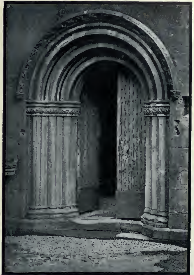
RECESSED DOORWAY, A GRACEFUL EXAMPLE IN EARLY WORK OF THE ROUNDED ARCH.
