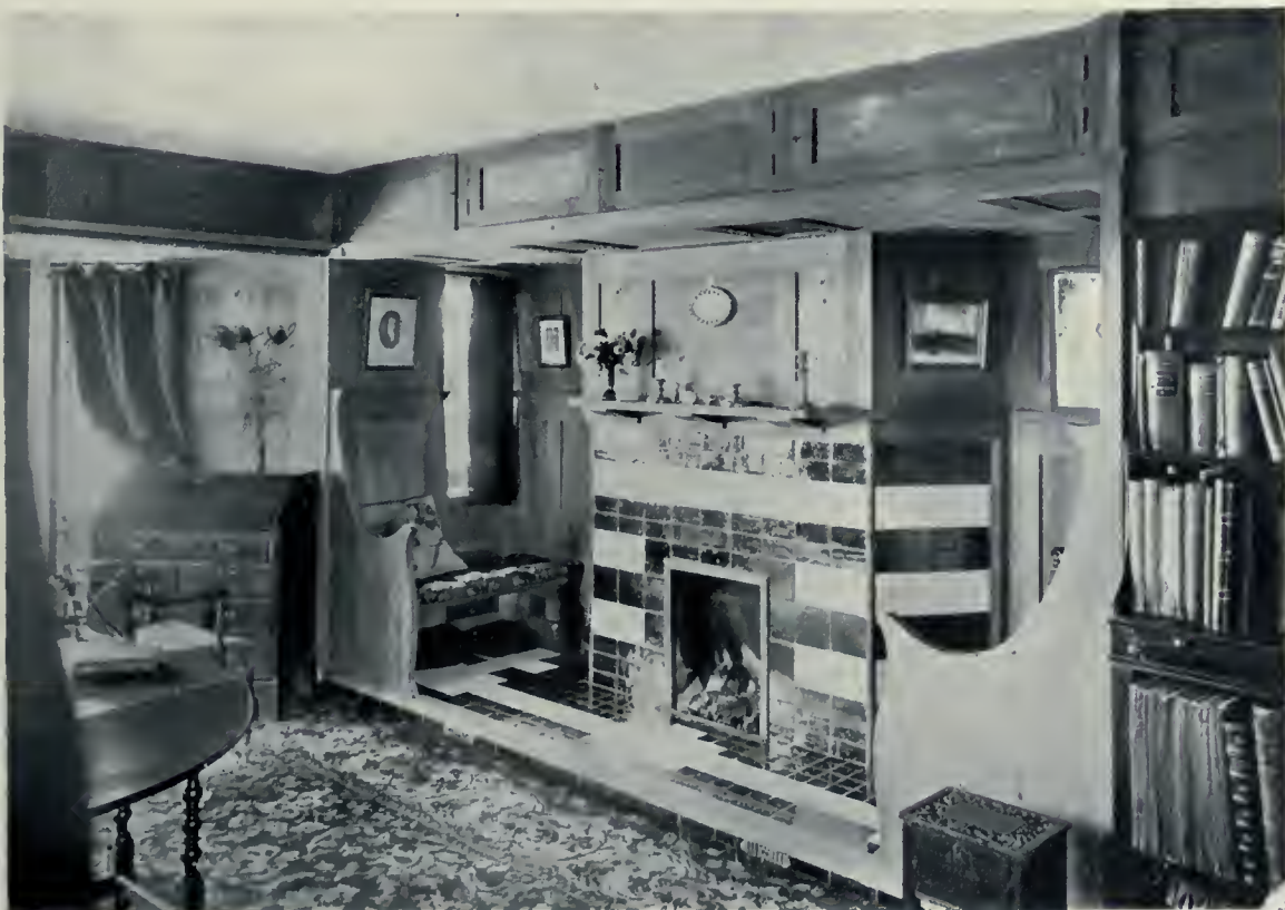
Dining Room, House at Biddenham. Among the distinctive features of this interior is the extreme simplicity of the woodwork. The fire-place seats and the panelling of the walls are most unique in both design and finish, the built-in cupboards around the top of walls being a most commendable innovation. Mr. C. E. Mallows, Architect.
