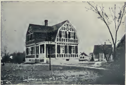
One of a group of cottages covered roof sides with our roofing.
