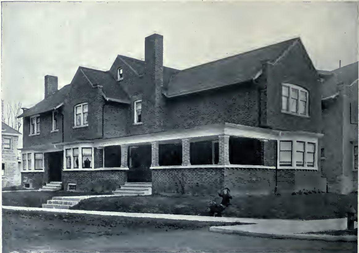
Semi-detached residence, cor. Ontario and Lake Streets, St. Catharines, Ont. While the exterior and interior of each dwelling apartment varies in elevation and plan, the whole unites into a most successful architectural composition in a two-family dwelling. Mr. A. E. Nicholson, Architect.
