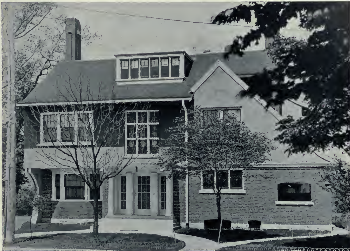
"Altmore," home of J. McLenehan, Lamport Avenue, Toronto. A residence of noteworthy design, built of red brick for the first story, with cement stucco above. At the back it overlooks a deep ravine, and takes in a fine perspective of the picturesque bit of country stretching out toward the north beyond. Messrs. Wickson and Gregg, Architects.
