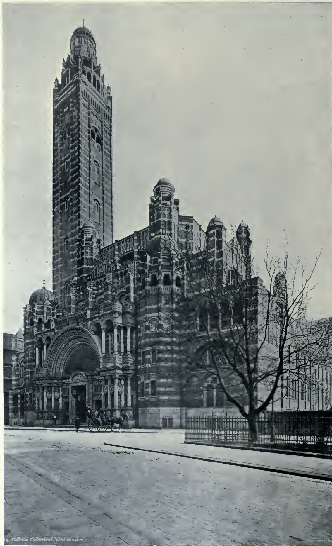
The West Front, New Catholic Cathedral at Westminster, London. A striking facade essentially Byzantine in character. Note the enormous arch, wider than that of St. Marks, Venice, and the somewhat excessive detail and decoration. Restrictions of "Ancient Lights" limited the architect to a low elevation, increasing the difficulties of treatment. Mr. John Francis Bentley, Architect.
