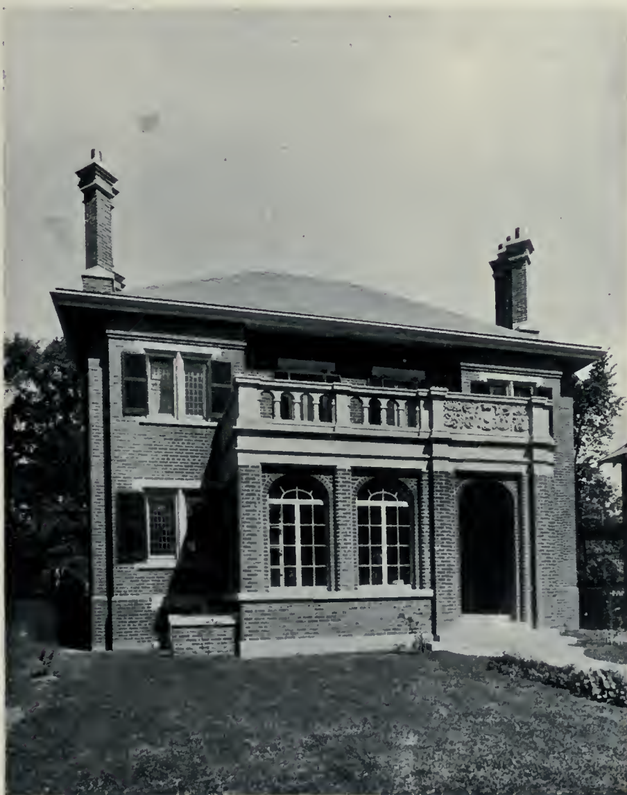
Residence of Mrs. W. P. R. Street, 10 Mackenzie Ave., Toronto, as seen from inside the garden wall. W. A. Langton, Architect.
