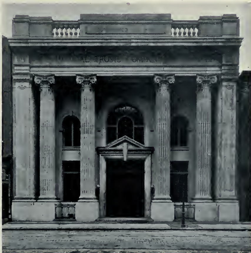
New building of the Imperial Trust Company, Toronto. Note the general detail of the facade, which is built entirely of manufactured stone. Messrs. Chadwick and Beckett, Architects.
