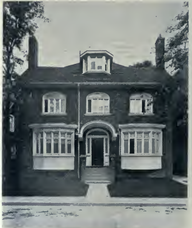
Home of R. L. Cowan, Rowanwood Avenue, Toronto. A clinker-brick residence of attractive design, which derives its chief charm from the variegated surface of its walls, and the simply decorative effect imparted by its doors and windows. Messrs. Chadwick and Beckett, Architects.
