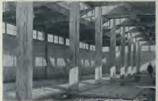
PLANT OF WOOD PRODUCTS COMPANY—INTERIOR VIEW OF CHARCOAL HOUSE IN FINISHED CONDITION. NOTE THE MONITOR ROOF RAISED ON THE INNER THIRD POINTS OF THE MAIN GIRDERS. E. D. PITT, DESIGNING AND CONSTRUCTING ENGINEER.
