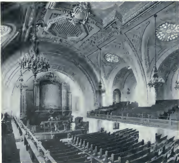
First Church of Christ (Scientist), Central Park West and Ninety-sixth Street, New York, designed by Carrere & Hastings. A costly church building in the Modern French style, with notably rich and elaborate decorations, verging on the Baroque.
