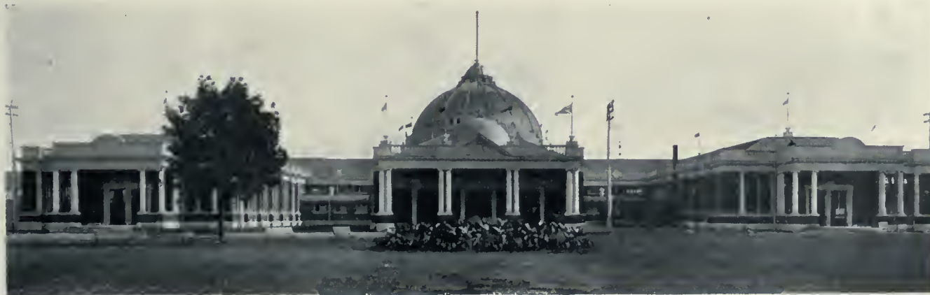
Horticultural Building, Canadian National Exhibition Grounds, Toronto, showing the projections which give its plan the form of a double U, and which provide separate sections for the agricultural, horticultural and floricultural exhibits. The building, over all, is 253 feet long, by 155 feet wide. Mr. Geo. W. Gouinlock, Architect.
