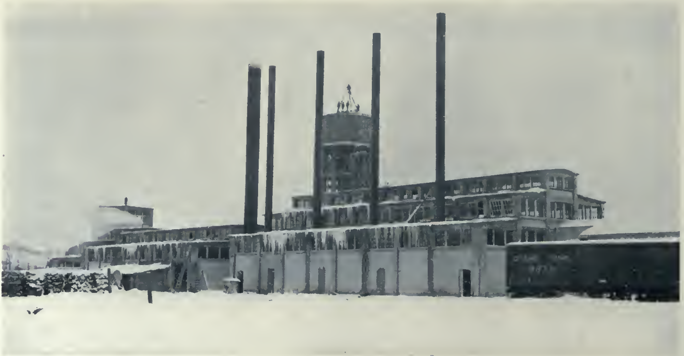
PLANT OF WOOD PRODUCTS COMPANY—REAR VIEW OF OVEN HOUSE AND BOILER HOUSE, SHOWING THE STILL HOUSE IN THE DISTANCE. E. D. PITT, DESIGNING AND CONSTRUCTING ENGINEER.
