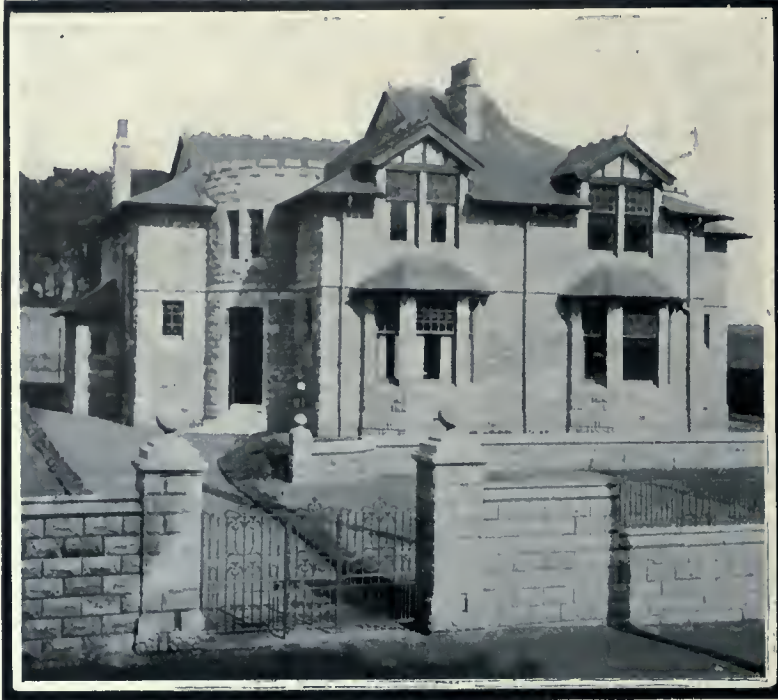
A concrete two-family block villa, designed and erected by the owner, David Brown, Jr., at Paisley (near Glasgow), Scotland. The total cost of this building was $3,360.
