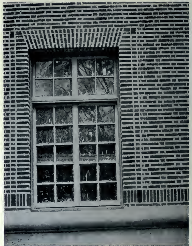
Fig. 3.—Detail of window of house illustrated in Fig. 2, showing the uniform manner in which the brick work flanks the window on either side.
