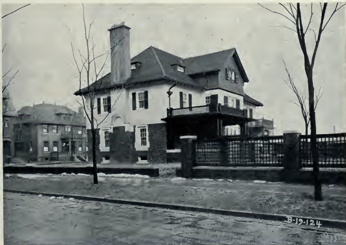
Front and side views, residence of Architect Albert Kahn, cor. Rowena and John's Streets, Detroit (Mich.). A thoroughly fireproof building that is not only commendable in design, but exceedingly interesting from a constructive standpoint. It is built in skeleton form, the structural frame being reinforced concrete, and the floors and walls a combination of reinforced concrete and hollow tile.
