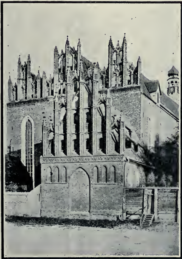
Franciscan Monastery of the Trinity, Dantsic, Germany.—A splendid example of Gothic architecture, 300 years old, in which the wall construction, including the arching, cornice and panel work, is entirely executed in brick.
