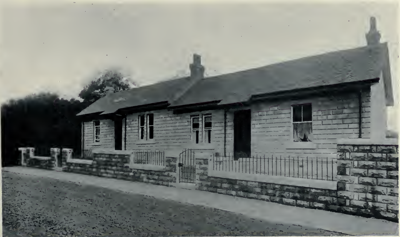
Two family cottage at Dumbarton, Scotland. A simply and pleasingly designed small double dwelling, executed in concrete block, the front of the building being of panel blocks, while the remaining portion of the walls is carried out in blocks of the rock-faced type.
