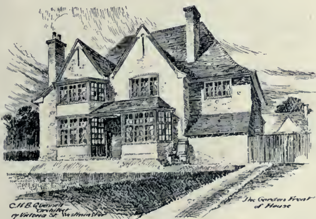
Small House at Purley. A recent adaptation in domestic work, built in an exposed situation on the Downs, and executed in red brick with red tile roof and wood casements. Mr. C. H. B. Quennell, Architect.
