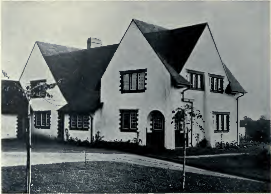
Home of W. E. Steers, at Caterham, Surrey, as viewed from the south-west. This house demonstrates the successful results which can be obtained from plain surfaces and uniform roof lines. The only decorative work to be observed is in the skillful treatment of the windows, and it is more to its perfect symmetry and balance, than to anything else, that this dwelling owes its exquisite home-like charm and character. Messrs. Unwin and Parker, Architects.
