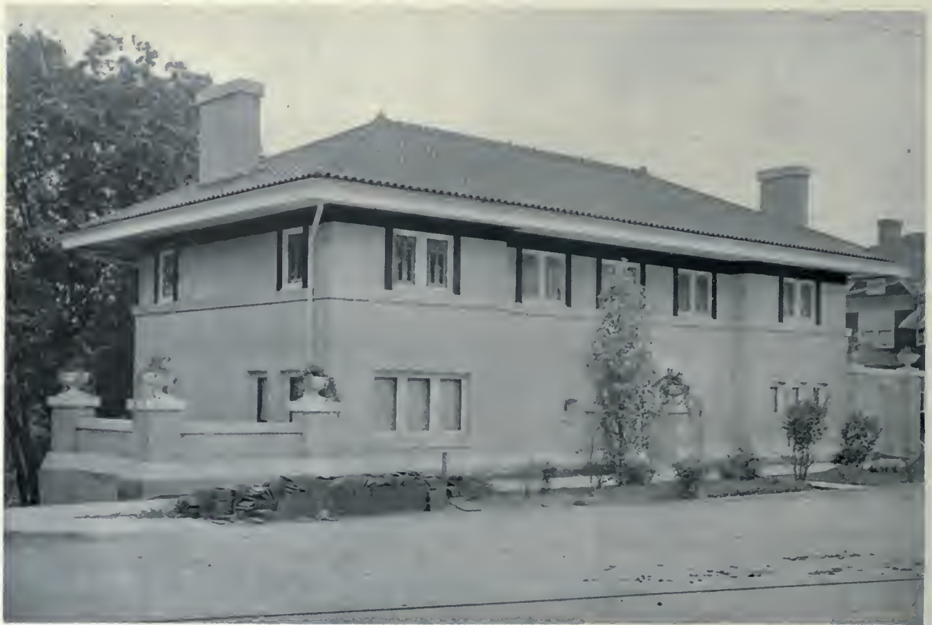
Fireproof residence of Dr. George E. Harter, Elkhart, Indiana. An adaptation of the Mission style of architecture, built of concrete blocks with cement stucco exterior.
