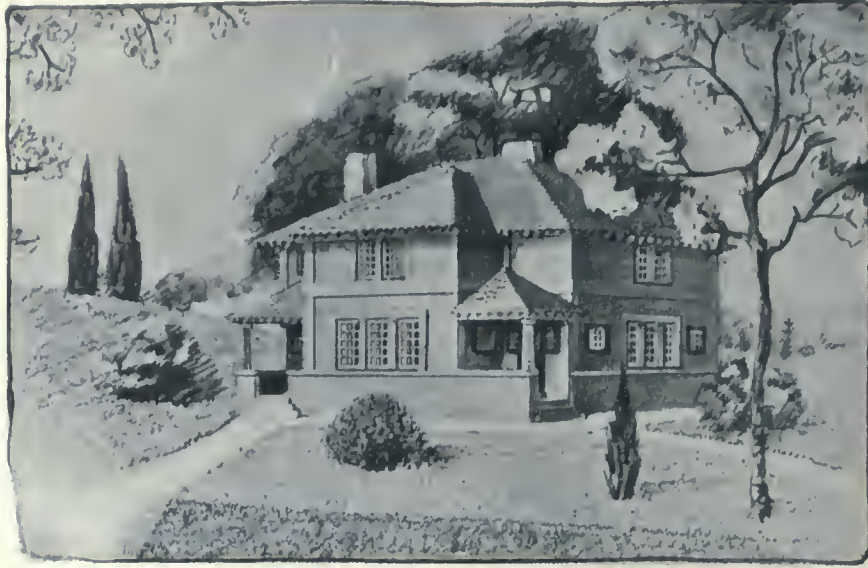
Design No. 6. A cottage which will readily adjust itself to any locality where an ample site and a few natural advantages are provided. It is built of concrete brick, being shaped like a cross, which gives opportunity for the maximum allowance of light and air and for large, well-placed rooms.
