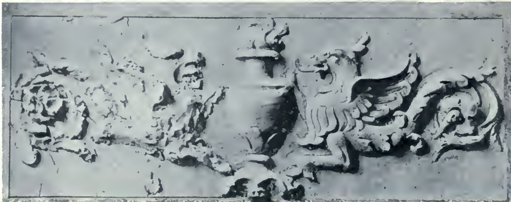
Ornament for the panels of porch. Detail of decorative work, Edison concrete house.
