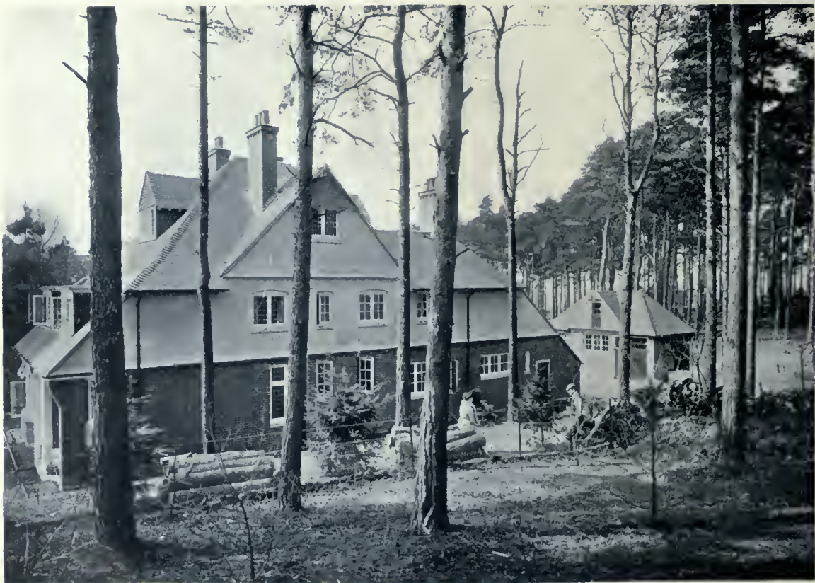
House at Camberley, as seen from the front and side. This home is built in the midst of a pine woods, a rather unusual site for an English house, but nevertheless one of a decidedly picturesque character. The building itself is a successful treatment carried out in red brick with rough-cast above, and a tile roof. One of its most striking features, and one which has greatly enhanced it from a viewpoint of design, is the interesting and architectural treatment of the windows and doorways. Mr. C. H. B. Quennell, Architect.
