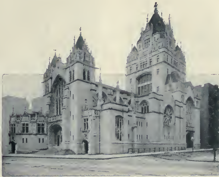
The Broadway Tabernacle (Congregational), Broadway and Fifty-sixth street, New York, designed by J. Stewart Barney. While thoroughly ecclesiastical in character, this church is remarkable as combining, on a limited site, a large auditorium and a twelve-story office building for parish work.
