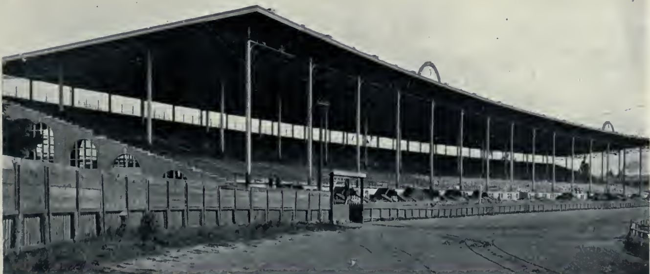
New Grand Stand, Canadian National Exhibition Grounds, Toronto. A steel and reinforced concrete structure which is capable of comfortably seating, in chairs, 17,000 people. The immensity of its size can be imagined from the fact that it is 725 feet long and 100 feet wide. It was erected at a cost of $240,000, and is the largest covered and most complete fireproof grand stand in the world. Mr. Geo. W. Gouinlock, Architect.
