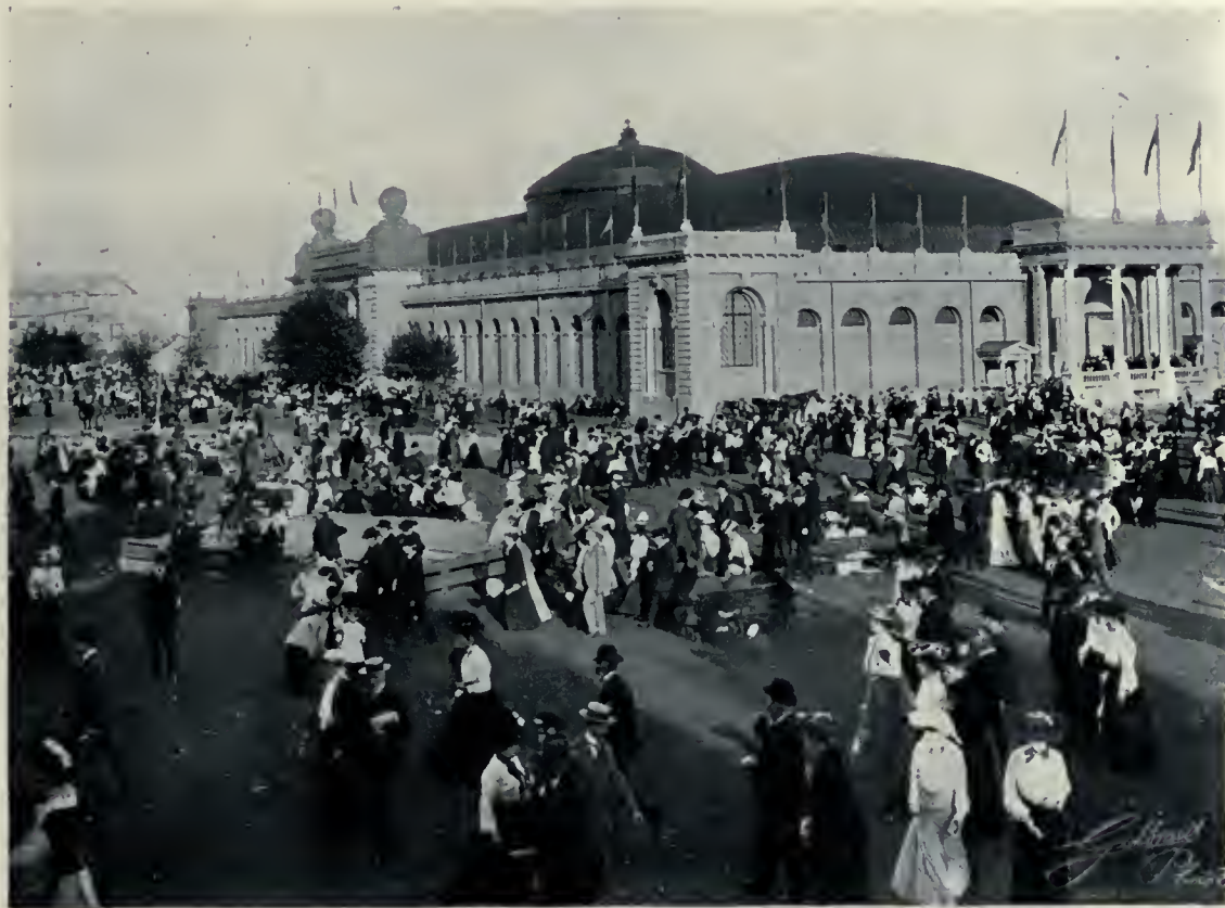
Manufacturers and Liberal Arts Building, Canadian National Exhibition Grounds, Toronto. Constructed of brick and steel, and having large arched trusses spanning the central portion. It is 450 feet long by 250 feet wide, and is utilized for exhibiting the finer class of manufactured goods. The cost of this building was $110,000. Mr. Geo. W. Gouinlock, Architect.
