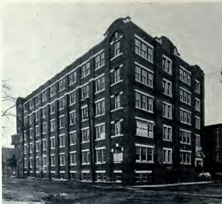
New Southam Press Building, recently erected at Toronto. A simple designed, well proportioned, reinforced concrete structure with brick curtain walls. Messrs. Sproatt & Rolph, Architects.
