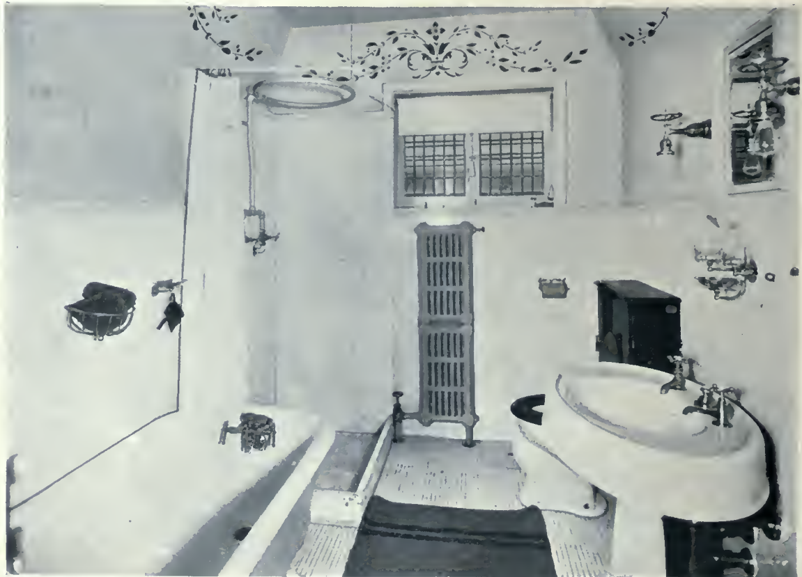
Bath-room, residence of Architect Wm. F. Sparling, Toronto. A compact but conveniently arranged and refreshing interior, equipped with the most approved sanitary fixtures and carried out with consistency of decorative detail.
