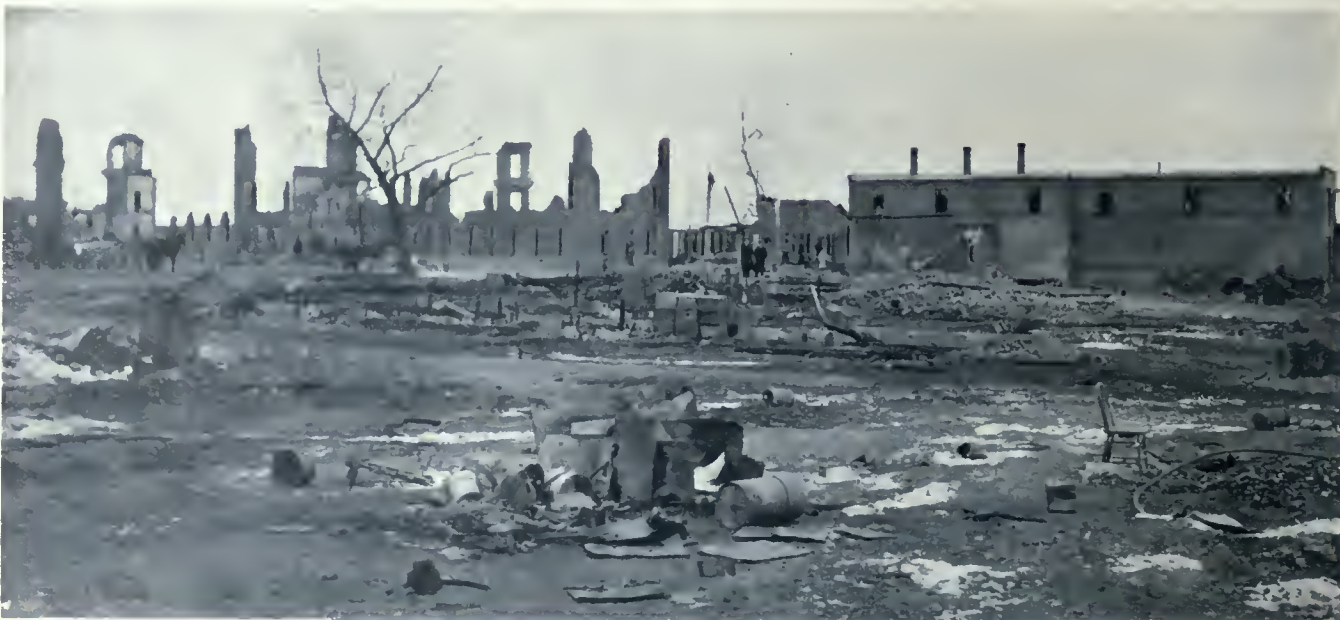
VIEW OF DISTRICT RECENTLY SWEEPED BY FIRE AT PEMBROKE, ONT., SHOWING THE CONCRETE BLOCK CARRIAGE AND WAGON FACTORY OF ALEXANDER BARR WHICH WAS THE ONLY BUILDING THAT SUCCESSFULLY STOOD THE ONSLAUGHT OF THE FLAMES.
