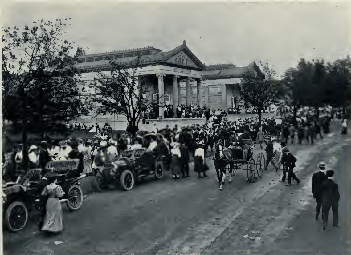
Art Gallery, Canadian National Exhibition Grounds, Toronto. An absolutely fireproof building, with walls of brick and stone, and floors and roof of reinforced concrete. Erected at a cost of $40,000. It is 120 feet long by 82 feet wide, constructed in quadrangular form, and will readily permit of future extensions. Mr. Geo. W. Gouinlock, Architect.
