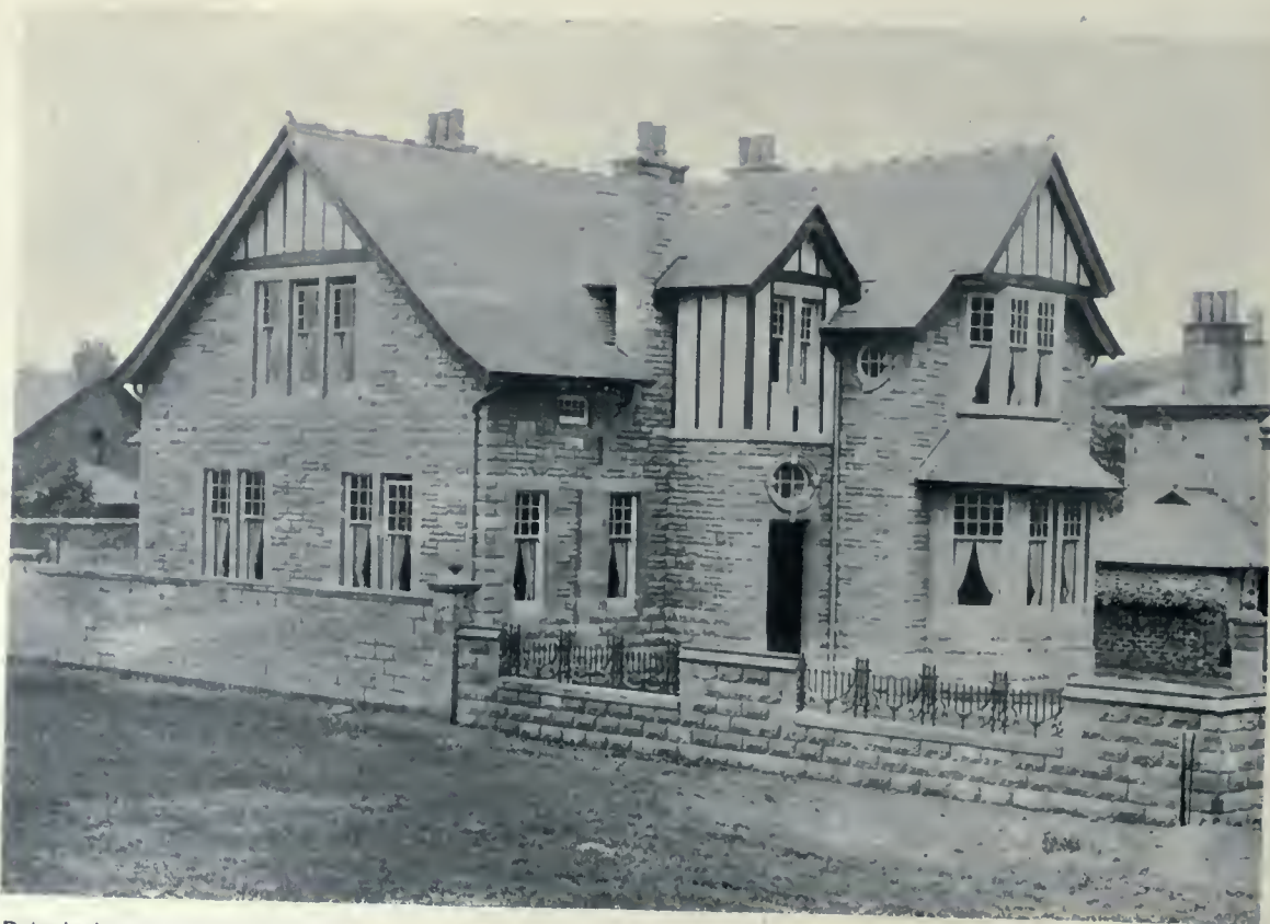
Detached concrete block residence, Paisley, Scotland. Note the ashlar effect, with panel trim at corners and plain trim around windows and doors.
