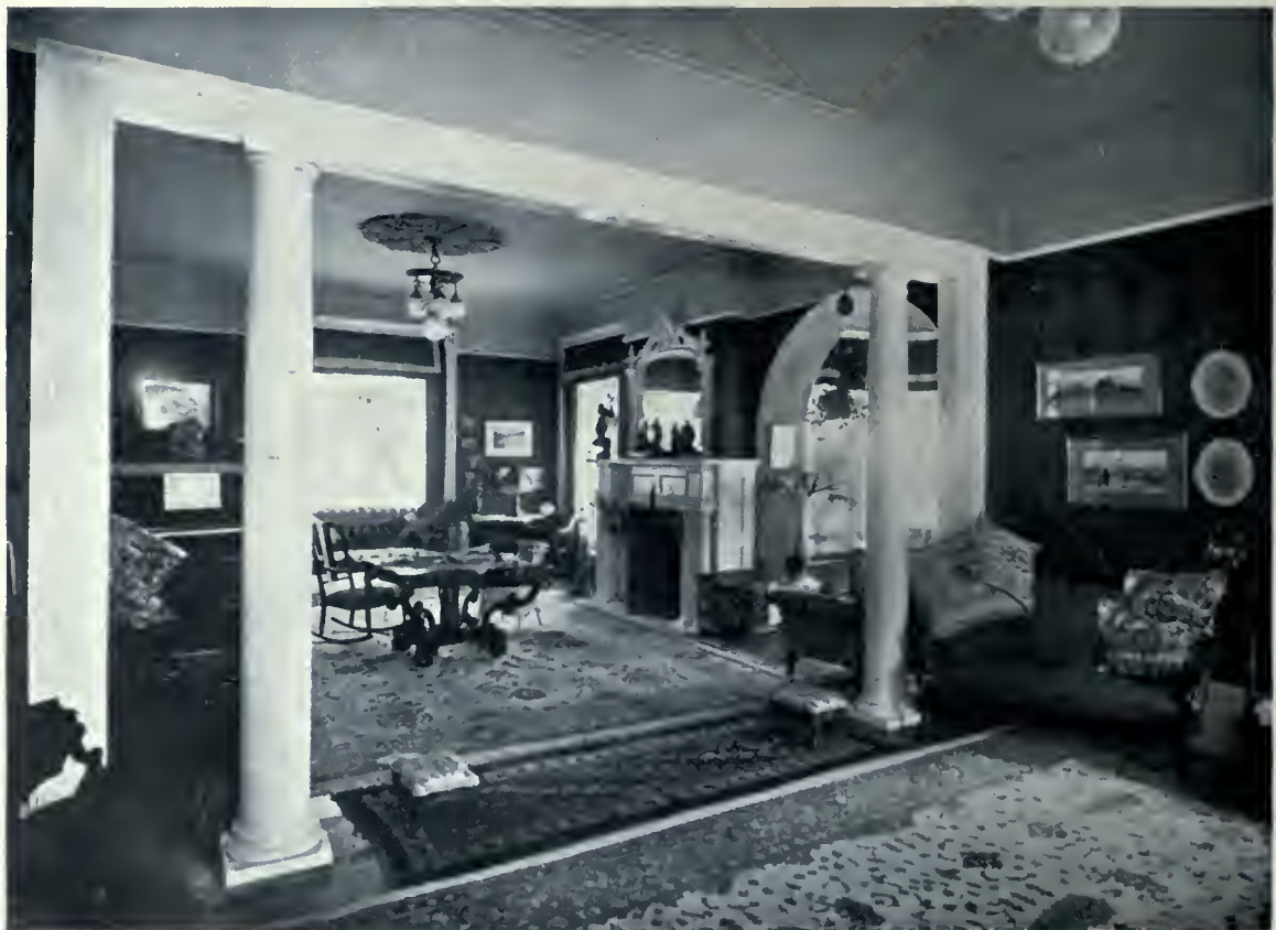
Living Room, Home of Mr. H. T. Bush, Port Hope, Ont., looking towards the rear and showing arched opening to bay window or sun parlor on the right. This is practically two rooms which have been formed into one by means of a large square-arched opening, with a large column on either side.
