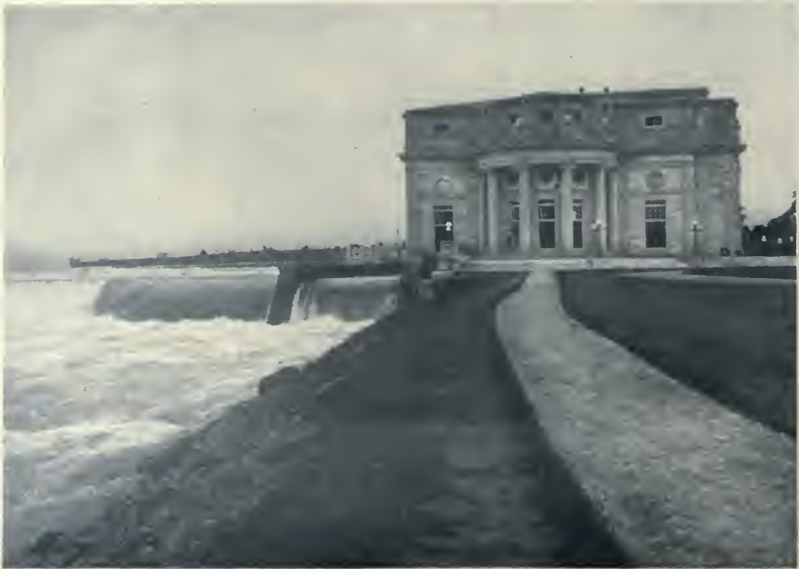
End view of Power House, Electrical Development Company, Niagara Falls, Ont., showing the onrush of water which is utilized in developing electric power and energy to operate Canadian manufactories and industries. E. J. Lennox, Architect.
