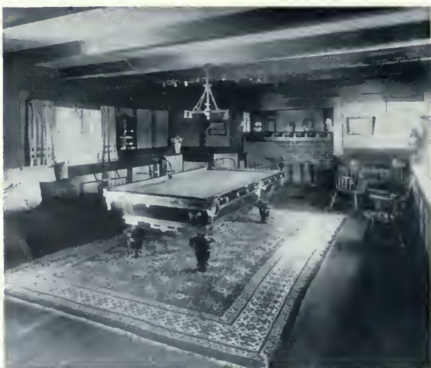
BILLIARD ROOM, COUNTRY HOME OF MR. JAMES RYRIE. BURKE AND HORWOOD, ARCHITECTS.
