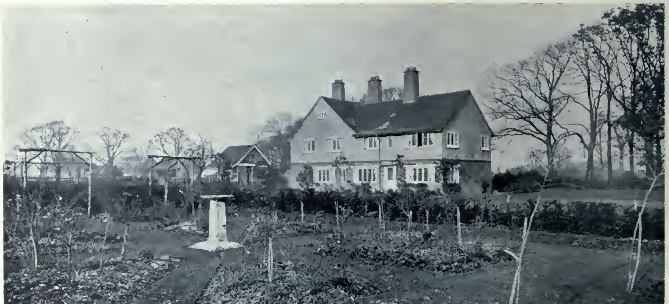
House at Biddenham, as viewed from the garden at the rear. The simple yet skillful manner in which this home is designed, has imparted to it a pronounced individual domestic character, that renders it unusually attractive. It is built of red brick, with the upper portion cement plastered, and a hand-made tile roof. Against this background, the white painted woodworks of the door and windows stand out in a pleasing contrast. Mr. C. E. Mallows, Architect.
