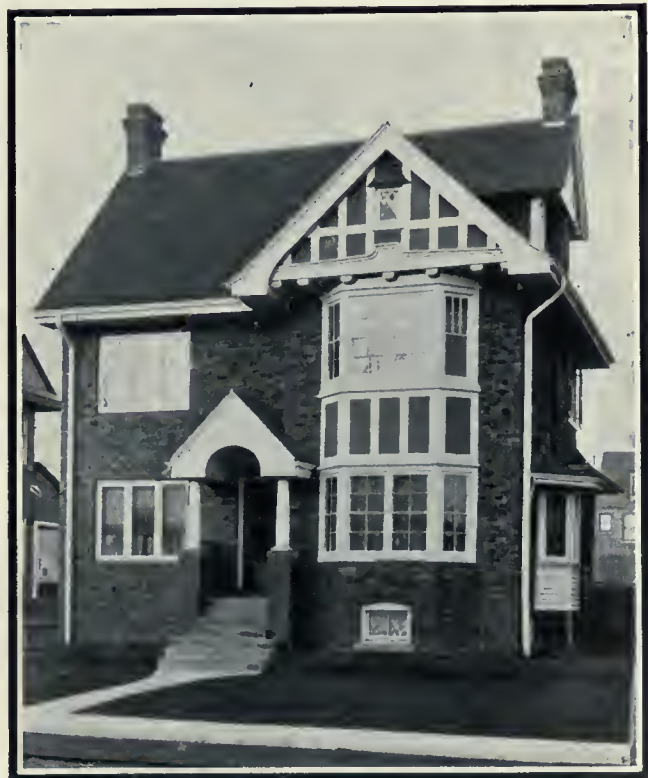
Residence of John M. Bowman, Toronto, an example of clinker brickwork in domestic architecture.
