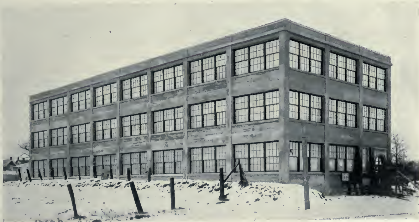
THREE-STOREY FACTORY BUILDING RECENTLY BUILT ON CARLAW AVENUE, TORONTO, FOR A. A. BARTHELMES, IN ACCORDANCE TO THE MUSHROOM SYSTEM OF REINFORCED CONCRETE. CLARKE & MONDS, DESIGNING AND ERECTING ENGINEERS.
