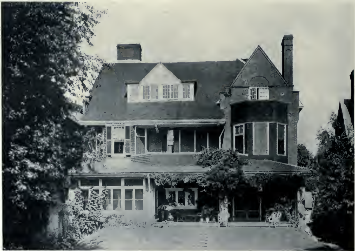
REAR VIEW, RESIDENCE OF MR. JOHN MARTIN, TORONTO, SHOWING THE VERANDA AND CONSERVATORY WITH BALCONY ABOVE, ALL OF WHICH OVERLOOKS A WELL KEPT TERRACE AND LAWN. MESSRS. EDEN SMITH & SON, ARCHITECTS.
