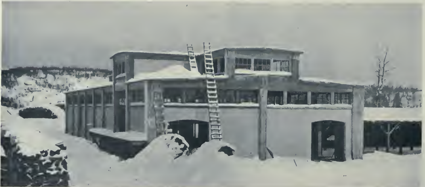
PLANT OF WOOD PRODUCTS COMPANY—VIEW OF CHARCOAL HOUSE, TAKEN FROM THE SOUTH, SHOWING THE SAND LIME BRICK CURTAIN WALLS. E. D. PITT, DESIGNING AND CONSTRUCTING ENGINEER.
