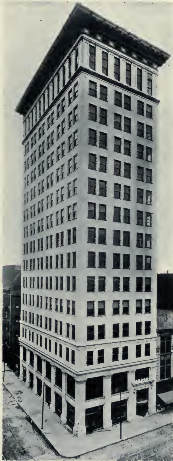
INGALLS BUILDING, CINCINNATI, OHIO, DESIGNED BY ELZNER AND ANDERSON. A SIXTEEN STOREY OFFICE BUILDING OF REINFORCED CONCRETE SKELETON CONSTRUCTION, WHICH SHOWS HOW THIS MATERIAL IS BEGINNING TO COMPETE WITH STRUCTURAL STEEL IN THE SKYSCRAPER FIELD.
