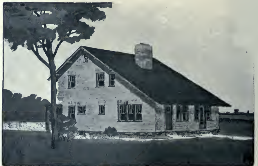
Rear view of Design No. 4 of suburban house, showing the broad sweep of roof. Note the slight projection in the shingled wall that forms a cap over each window or group of windows. This not only affords protection, but is a very interesting feature of the construction.
