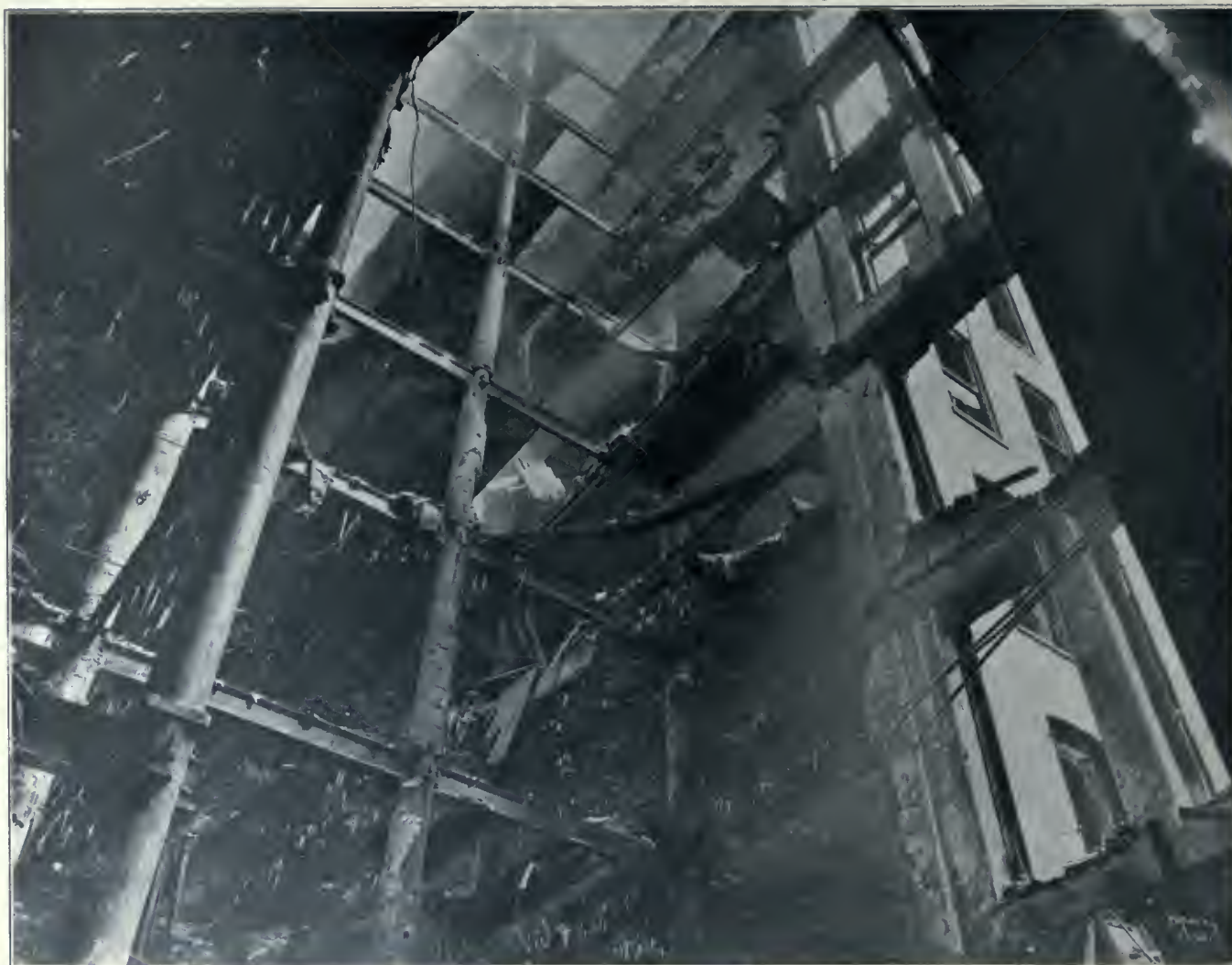
VIEW OF DESTROYED BUILDING, SHOWING HOLE BURNED FROM BASEMENT TO THE ROOF.
