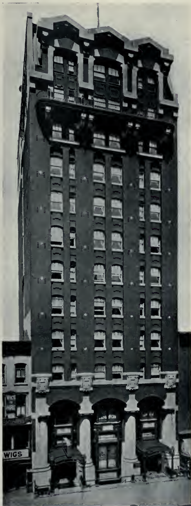
Fig. 4.—Hotel building of attractive design, the facade of which is built of red pressed brick with blue toned bricks for trimmings. These are laid up in the ordinary Flemish bond with white raked-out mortar joints of an appropriate thickness.
