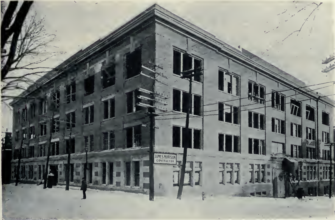
AMES-HOLDEN BUILDING, MONTREAL. ROSS & MACFARLANE, ARCHITECTS. AN INTERESTING INSTANCE OF FLOOR SUSTAINING EXTERIOR WALLS IN REINFORCED CONCRETE CONSTRUCTION.
