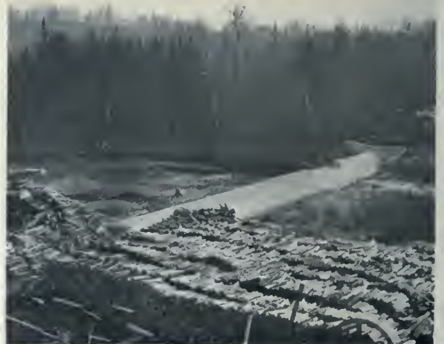
PLANT OF WOOD PRODUCTS COMPANY—VIEW OF COMPLETED DAM FOR STORAGE PURPOSES—214 FEET LONG OVER A NORMAL HEAD OF 9 FEET. E. D. PITT, DESIGNING AND CONSTRUCTING ENGINEER.
