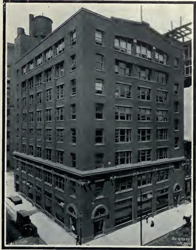
Light manufacturing and office building, showing the satisfactory and unpretentious brick exterior of a steel frame structure.
