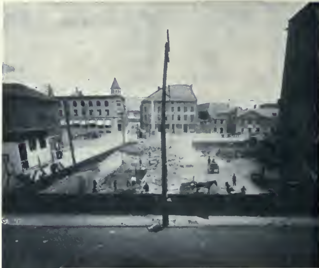
View Taken June 1st, 1908, when Excavation was Completed
