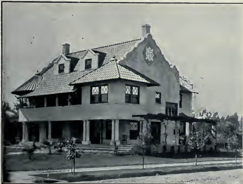
A Southern Cement Stucco Residence, Plastered outside and inside on "EXPANDED METAL LATH."
