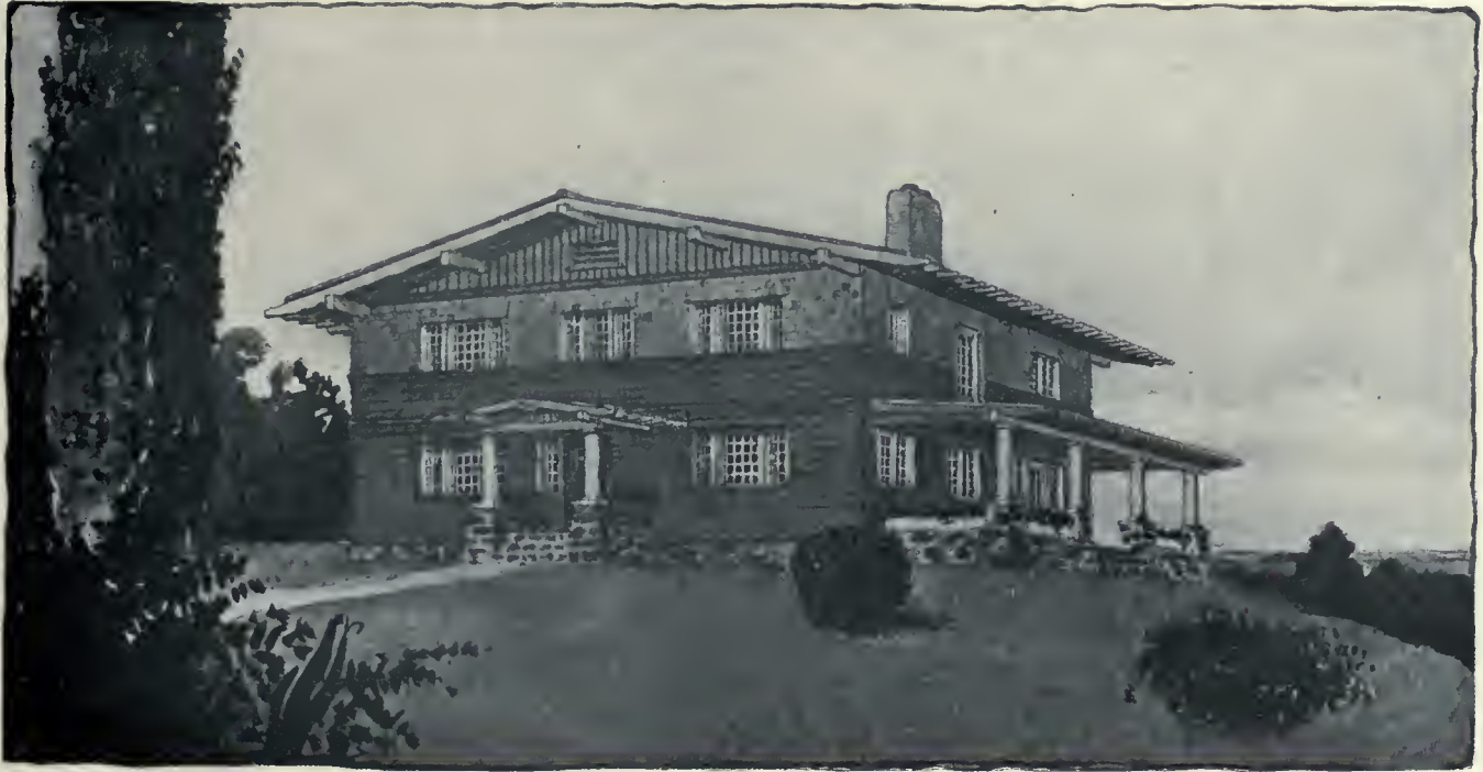
Design No. 1—A country house especially adapted to a site which is slightly elevated and the immediate grounds somewhat open. It is built entirely of wood on a foundation of field stone. The lower story, and part of the second is covered with eight-inch weather boarding \frac{7}{8} of an inch thick; the shingles are of the rived kind and the vertical gable boards V-jointed. The three belt courses, stained a darker tone than the rest of the walls, materially assist to give the house its low, bungalow like appearance.
