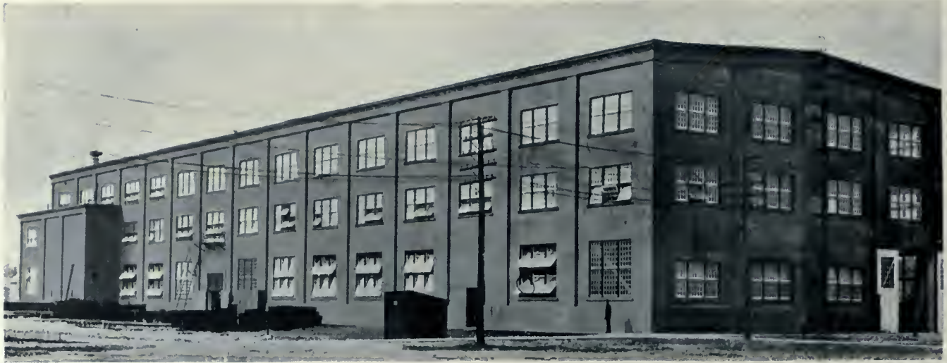
CANADIAN GENERAL ELECTRIC COMPANY'S TRANSFORMER HOUSE, PETERBORO. A STEEL FRAME STRUCTURE, WITH CONCRETE WALLS AND FLOORS.
