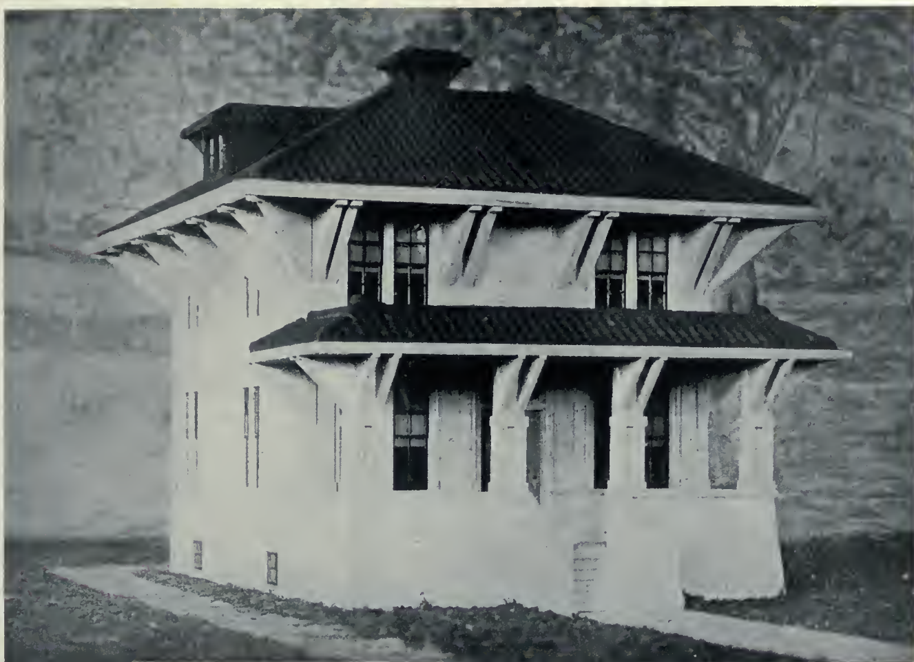
Front view of new model for Mr. Edison's $1,200 concrete, fire-proof workingman's house, the practicability of which the inventor claims he is about to demonstrate.
