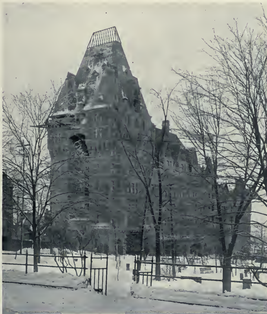
NEW ADDITION TO CHATEAU FRONTENAC, QUEBEC CITY. VIEW TAKEN FROM REAR OF THE NEW PORTION, LOOKING TOWARDS THE OLD, SHOWING THE MANNER IN WHICH THE ARCHITECT SUCCEEDED IN PROVIDING FOR A FIRE ESCAPE WITHOUT MARRING THE ARCHITECTURAL BEAUTY OF THE BUILDING, THE FIRE ESCAPE BEING PLACED IN THE DEEP RECESS TO BE SEEN IN THE FOREGROUND OF THE PICTURE. W. S. PAINTER, ARCHITECT.
