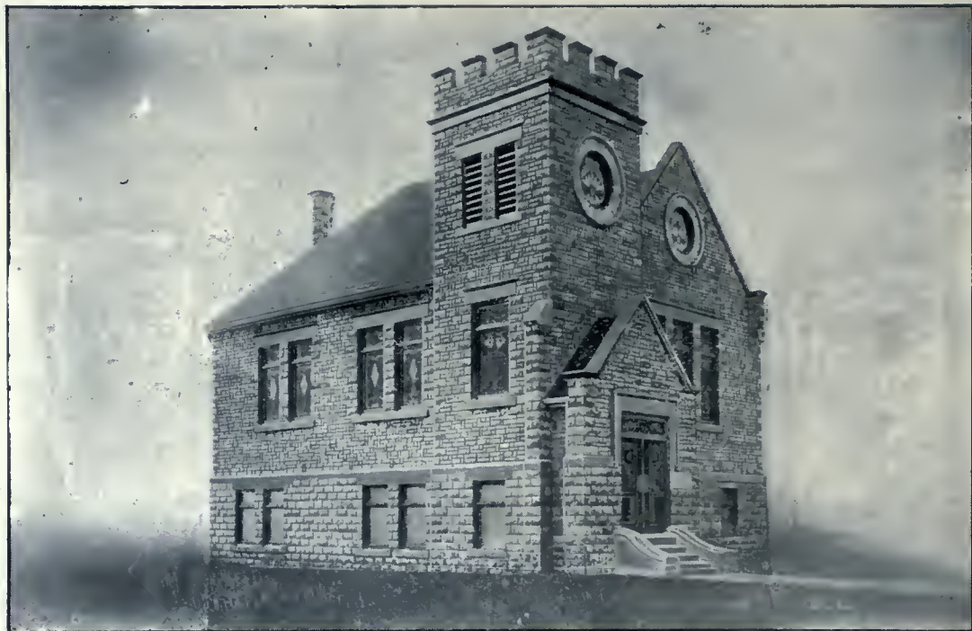
SALEM METHODIST CHURCH, DERWENT, ONT., BUILT OF CEMENT BLOCKS. THE STRUCTURE WAS DESIGNED BY H. POCKOCK, ARCHITECT AND PRESIDENT OF THE LONDON CONCRETE MACHINERY COMPANY, LONDON, ONT.
