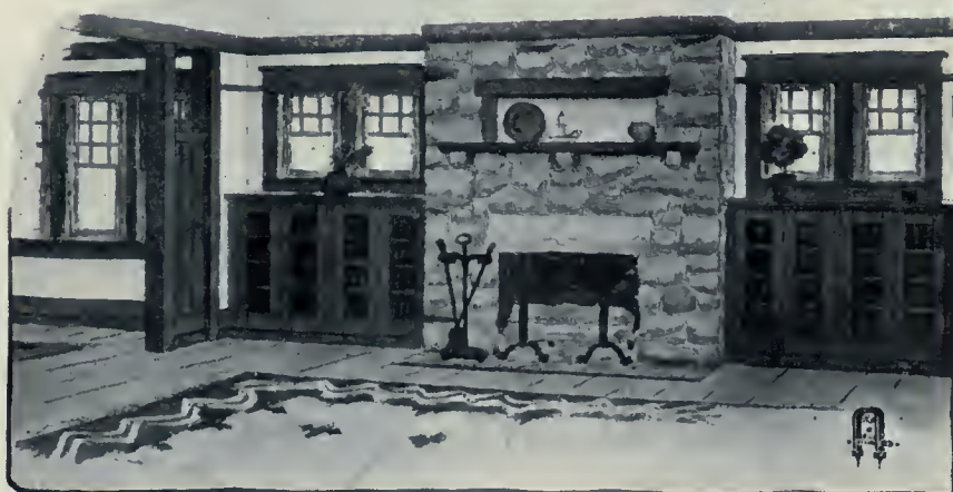
Fireplace and bookcases in living room of Design No. 3. This fireplace is built of field-stone, laid in black cement, and runs clear to the ceiling. Note the bookcases built in on either side of the fireplace, above which are two small double-hung windows.
