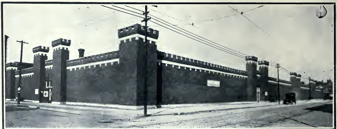
Central Market, located in the West Side District, Chicago. A simple, but effective treatment of brick work in wall, tower, and parapet design.
