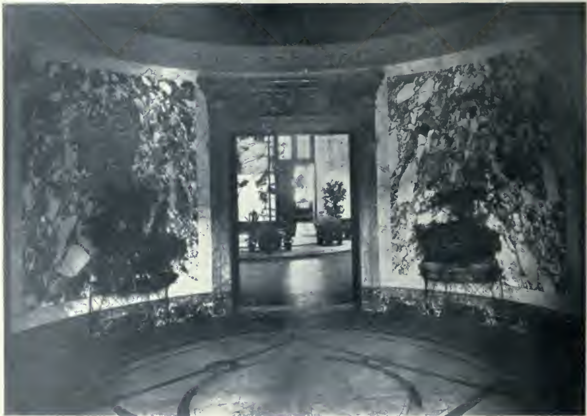
Rotunda, looking towards Generator-room, Power House, Electrical Development Company, Niagara Falls, Ont. A rich interior, circular in shape and executed in high-grade marbles. The panels of the wall are in Breche violet with a stile of English veined Italian, the sub-base being Jaune Fleuri and the door trim consisting of Rouge Jasper and Jaune Fleuri. The floor has a field of White Italian inlaid with Red Numidian, the border being composed of Rouge Jasper, Sienne, Verde Antique with Sylvian Green squares. E. J. Lennox, Architect.
