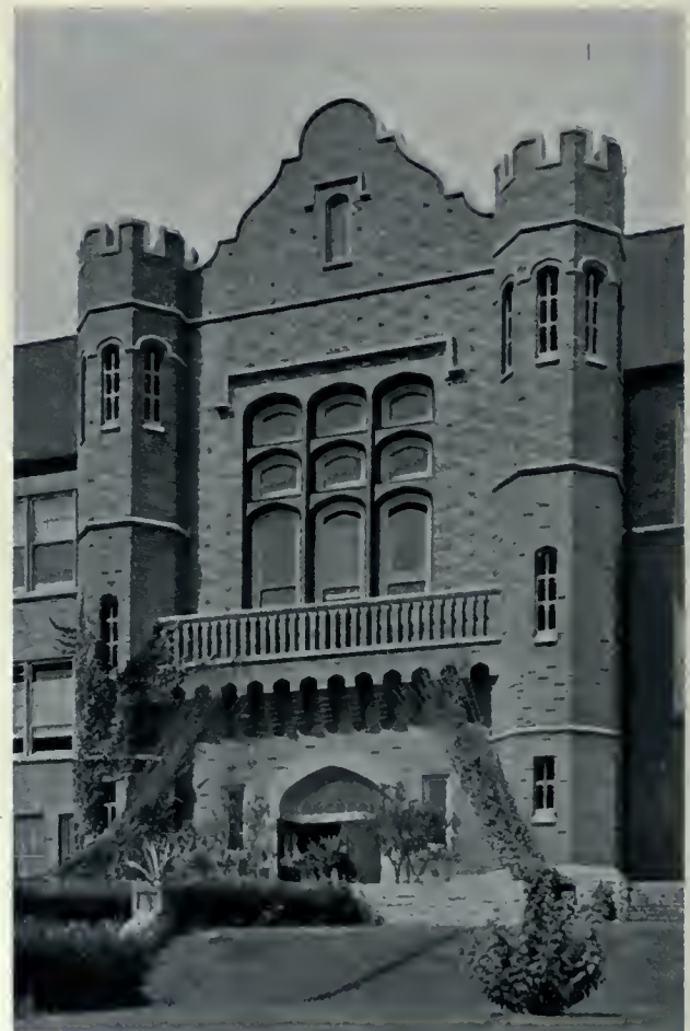
Main Entrance of Edward Wyman School, St. Louis, Mo.—A commendable architectural treatment expressed in hard and red brick, mixed as to color, and laid in up with a Flemish bond. Note the simple details of the towers and the arcading under balcony over doorway.
