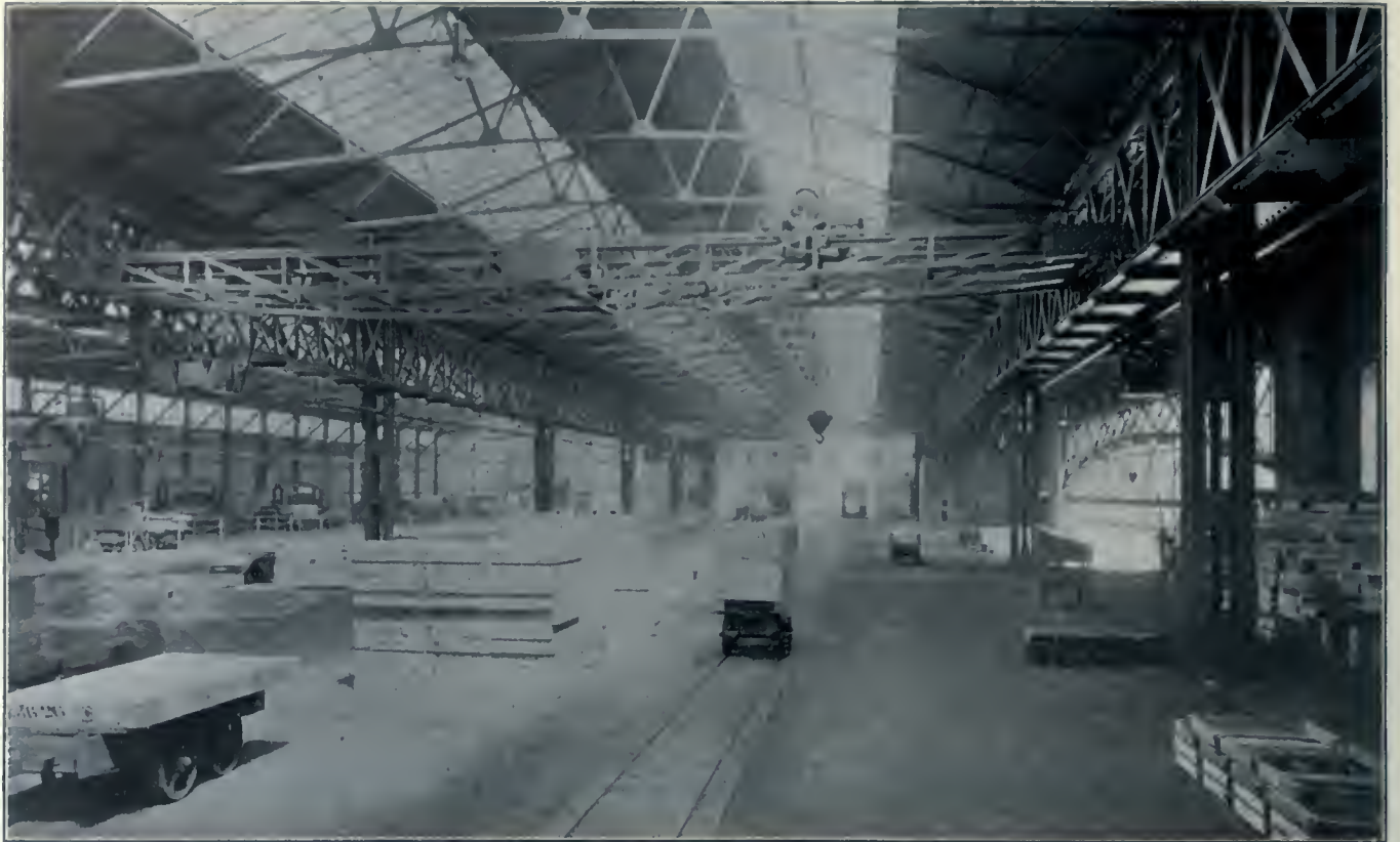
View of Packing and Shipping-Room for galvanized sheets of the plant of John Lysaght, Limited, at Bristol, Eng.
