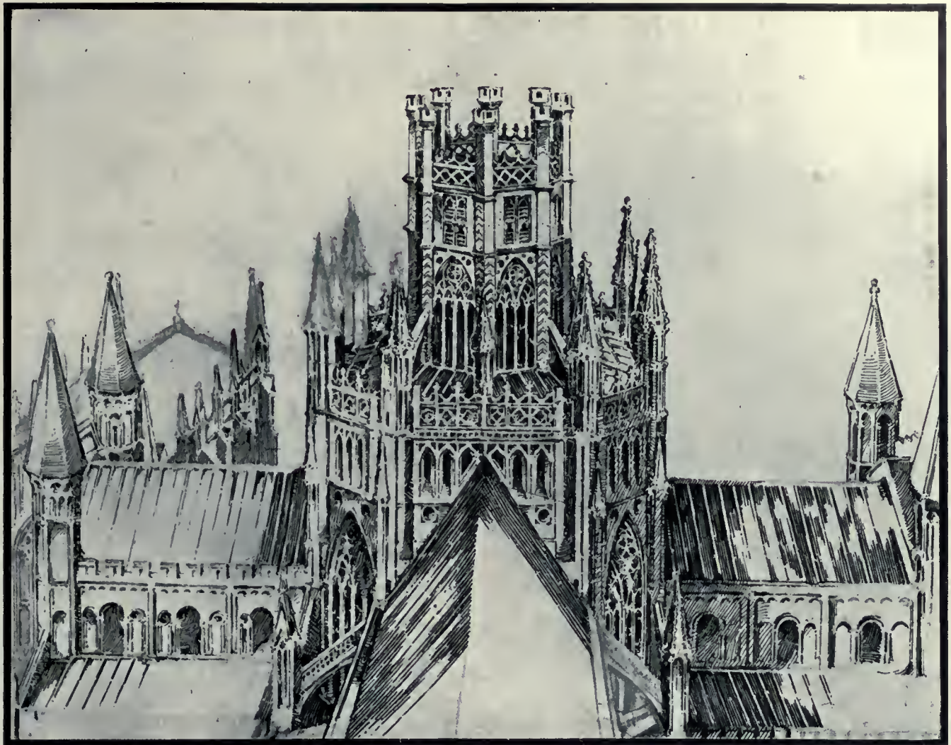
OCTAGONAL LANTERN OF ELY CATHEDRAL,—“ST. ANDREY’S CROWN,”— A PRODUCTION OF THE DECORATED PERIOD, EXECUTED IN STONE AND WOOD, WHICH IS THE MOST PERFECT EXAMPLE OF THIS TYPE OF WORK EXTANT. REPRODUCED FROM PEN DRAWING (UNFINISHED) MADE AT TOP OF WEST TOWER.
