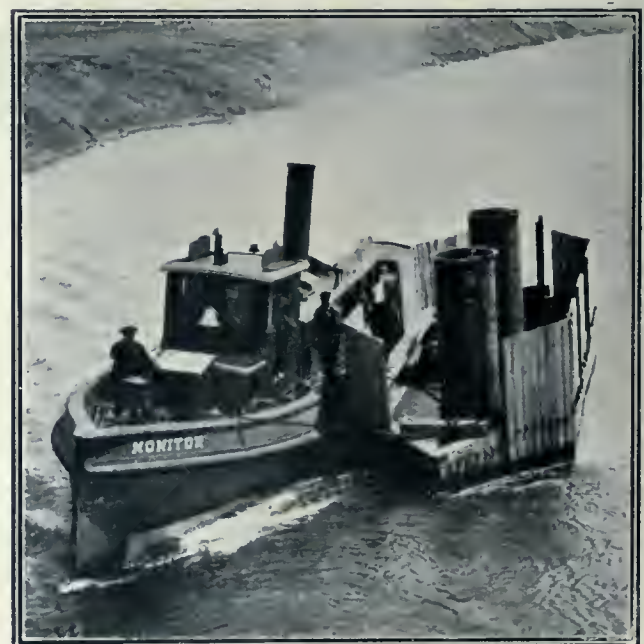
TOWING A CAISSON TO POSITION.
