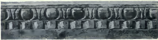
Detail of the two exterior ornamental bands, Edison concrete house.
