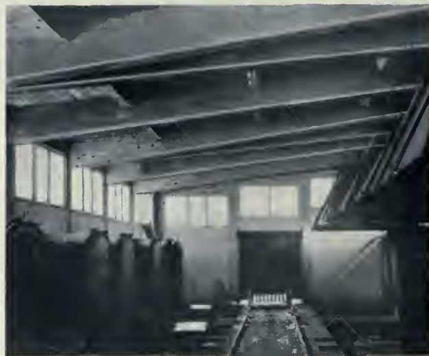
PLANT OF WOOD PRODUCTS COMPANY—INTERIOR VIEW OF OVEN HOUSE, SHOWING DIVIDED BEAMS WHICH CENTRE AT ONE END ON A SINGLE COLUMN. THE DETAIL OF THIS ARRANGEMENT MAY BE SEEN IN THE ROOF PLAN OF THIS BUILDING, PUBLISHED HEREWITH. E. D. PITT, DESIGNING AND CONSTRUCTING ENGINEER.
