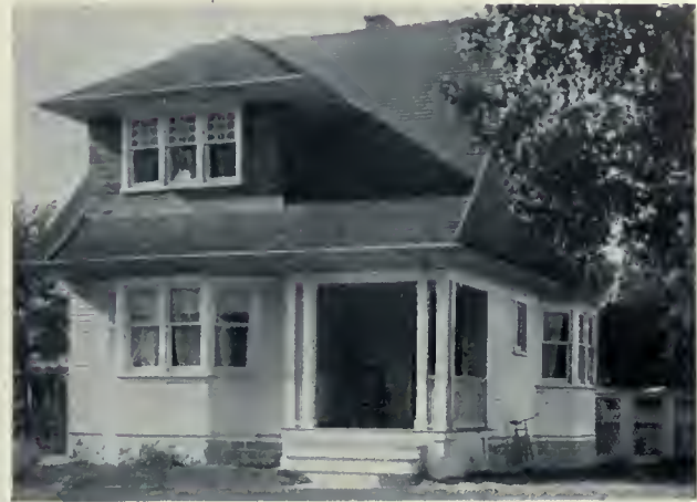
Frame cottage, Welland Avenue, St. Catharines, Ont., a small house with exceptionally good lines. Mr. C. E. Nicholson, Architect.
