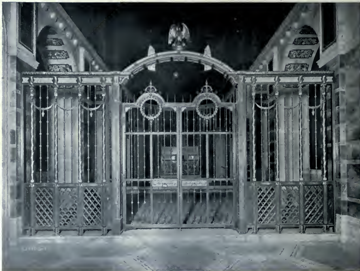
Chapel of Blessed Sacrament, New Catholic Cathedral at Westminster, London, showing the Screen and Gates. A fine example of modern metal work, the design being beautiful and the execution perfect. Mr. John Francis Bentley, Architect.
