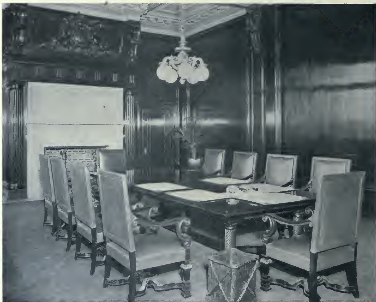
BOARD ROOM, NEW ROYAL BANK BUILDING, MONTREAL.—H. C. Stone, Architect.
