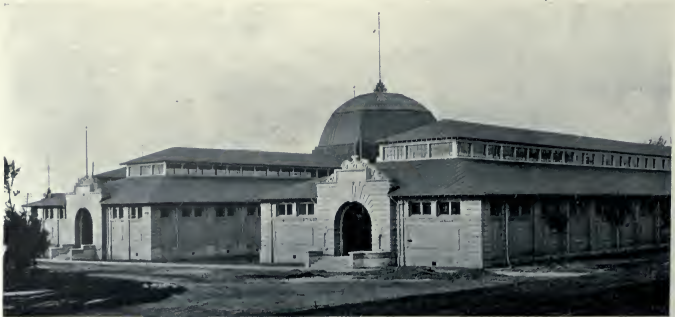
Industrial Building, Canadian National Exhibition Grounds, Toronto. This building is in the form of a double H, and is 231 feet long by 340 feet wide over all. Access to the interior is obtained through eight separate entrances, the central one being elaborated with a columned portico. The structure is built of cement concrete, brick and stone, with steel trussed roof having a large dome at centre. It contains 74,000 superficial feet of floor space, and cost, complete, $95,000. Mr. Geo. W. Gouinlock, Architect.
