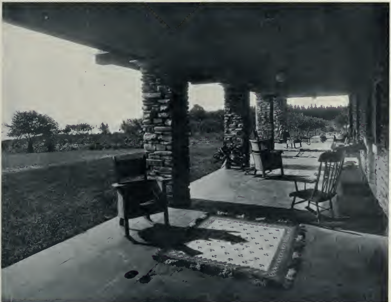
SPACIOUS VERANDAH, COUNTRY HOME OF MR. JAMES RYRIE, SHOWING THE LAKE STONE PIERS SUPPORTING THE UPPER FRONT PORTION OF THE HOUSE. BURKE AND HORWOOD, ARCHITECTS.
