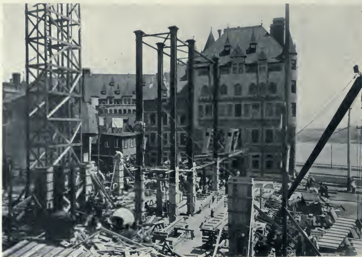
NEW ADDITION TO CHATEAU FRONTENAC, QUEBEC CITY. VIEW SHOWING THE TEN STRUCTURAL STEEL COLUMNS AND STEEL TRUSSES USED IN THE BUILDING, AND THE PROGRESS OF THE WORK MADE UP TO JULY 22ND. W. S. PAINTER, ARCHITECT.
