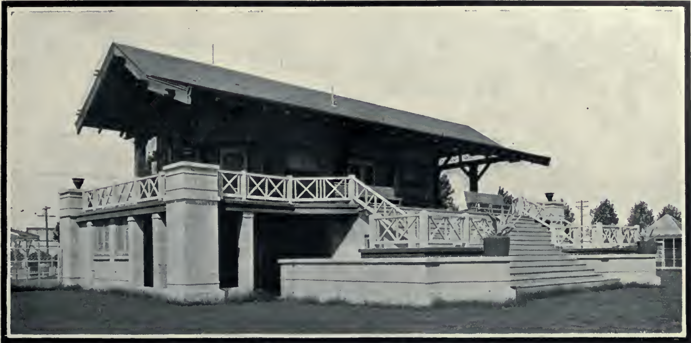
Club House, Dallas Driving Association, Dallas, Texas. An attractive structure of concrete block, cement stucco, and half-timber construction.
