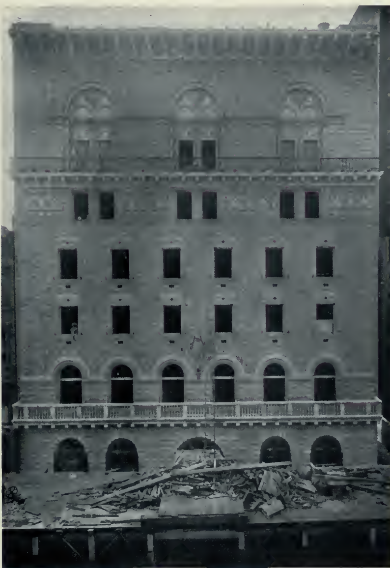
Fig. 1.—Facade of Club Building, showing an interesting treatment in diaper work. The bricks, 12 x 2½ x 4 inches in size, and of a rough texture, are laid up with a gray raked mortar joint, three-quarters of an inch in thickness, the bond being of a special character. The color tones are a soft warm gray tinged with brown, and white headers and special moulded bricks, on a smooth brown ground.
