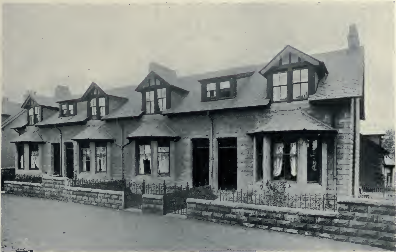
Four family cottage, built of concrete blocks, at Paisley, Scotland, where this form of construction is coming much into evidence.
