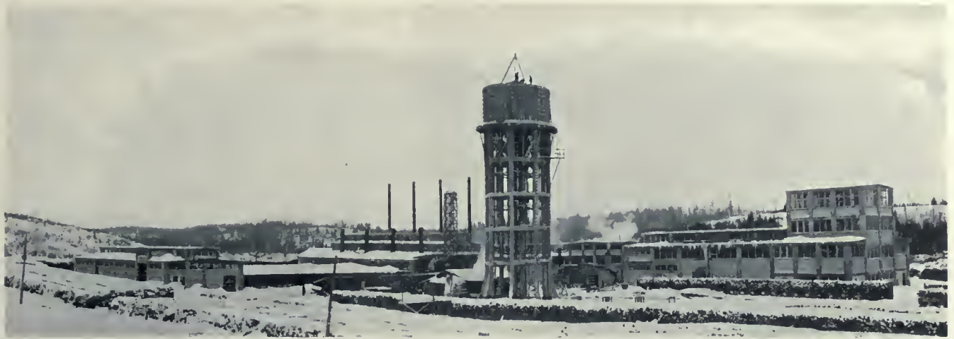
PANORAMIC VIEW OF NEW PLANT OF WOOD PRODUCT COMPANY, DYSART, ONT., TAKEN FROM THE WEST, DEC. 15TH, '08, SHOWING THE PLANT COMPLETED WITH THE EXCEPTION OF THE WATER TOWER, WHICH REMAINS ONLY TO BE STRIPPED. E. D. PITT, DESIGNING AND CONSTRUCTING ENGINEER.
