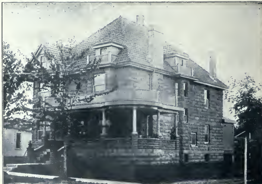
A $2,400 RESIDENCE. ALL THE BLOCKS USED WERE MADE ON THE CONCRETE BLOCK MACHINE MANUFACTURED BY THE LONDON CONCRETE MACHINERY COMPANY, LONDON, ONT.
