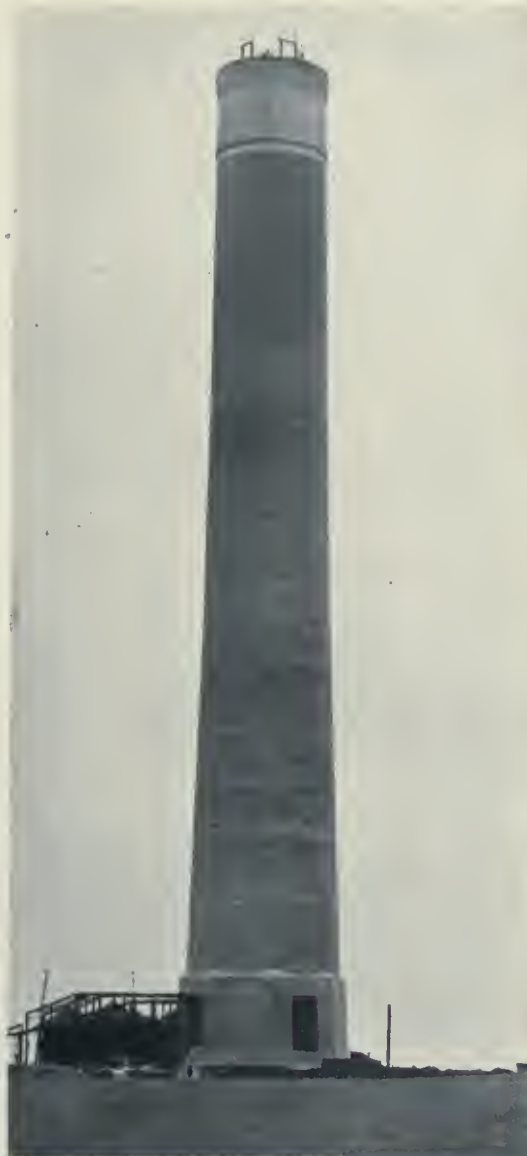
GIGANTIC CHIMNEY ERECTED AT THE SMELTING WORKS OF THE BOSTON AND MONTANA CONSOLIDATED COPPER AND SILVER MINING COMPANY, GREAT FALLS, MONTANA. FROM FOUNDATION TO CAP IT IS 506 FEET HIGH.
