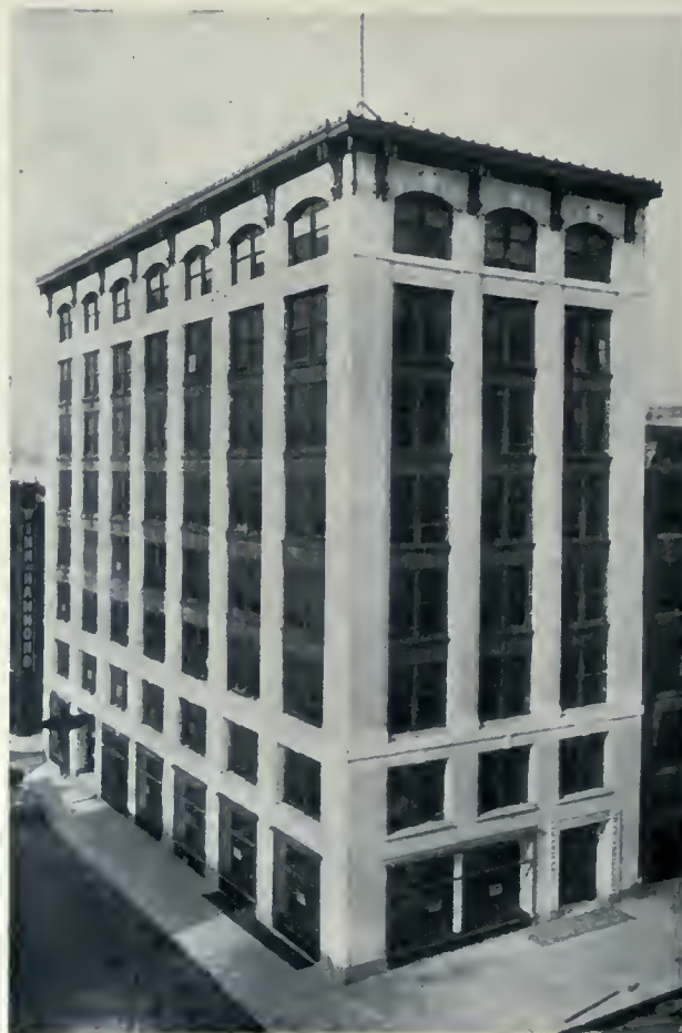
KAHN BUILDING, DETROIT, BUILT BY THE TRUSSED CONCRETE STEEL COMPANY, IN ACCORDANCE TO THE SYSTEM WHICH NAME IT BEARS. IT IS AN ALL CONCRETE STRUCTURE WITH THE EXCEPTION OF THE EXTERIOR WALLS. MR. JULIUS KAHN, ARCHITECT.
