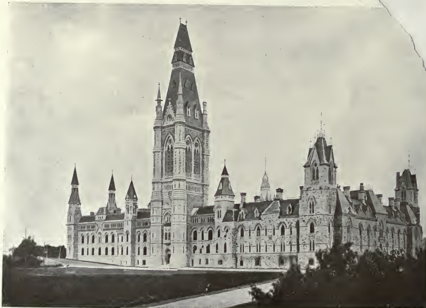
PLATE XVI. WESTERN BLOCK WITH ADDITION BY THE MACKENZIE GOVERNMENT. BETTER LIGHTED THAN OLD PART; BUT ROW OF SMALL WINDOWS IN ATTIC NOT SCALED SUCCESSFULLY WITH STOREYS BELOW. ALL DETAIL POORER.
