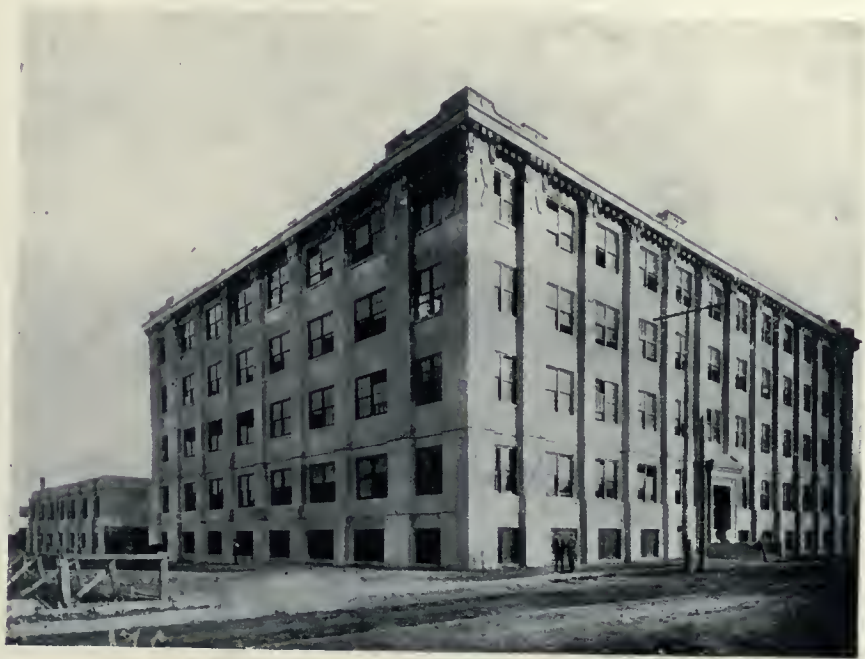
IMPERIAL TOBACCO COMPANY'S BUILDING, MONTREAL. A TYPICAL EXAMPLE OF AN ALL CONCRETE STRUCTURE. NOTE HOW SATISFACTORILY THE CONCRETE HAS ASSIMILATED THE ARCHITECTURAL LINES. MR. ROBERT FINDLAY, ARCHITECT.
