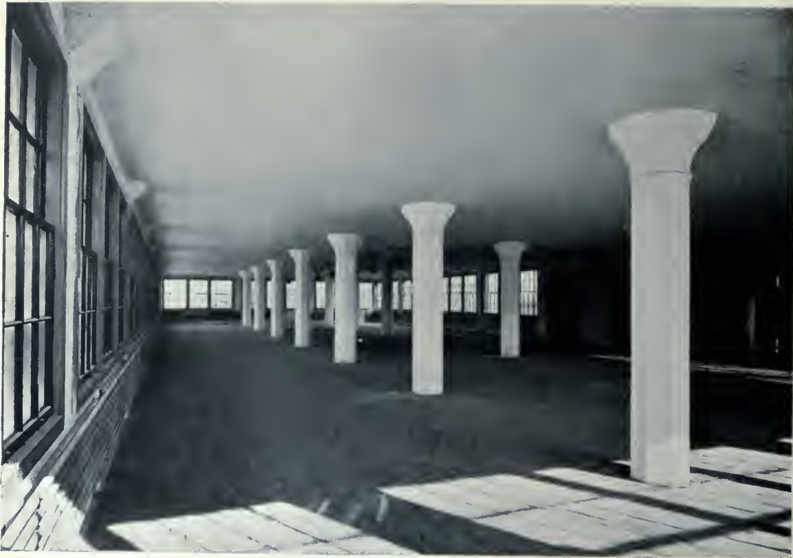
INTERIOR VIEW OF A. A. BARTHELMES' NEW FACTORY, TORONTO, SHOWING THE OCTAGONAL COLUMNS WITH SLIGHTLY FLARED HEAD, TOGETHER WITH WINDOW ARRANGEMENT. NOTE THE ABSENCE OF BEAMS BETWEEN INTERIOR COLUMNS AND THE UNBROKEN SURFACE OF THE CEILING.
