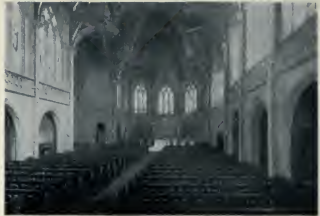
The Rhinelander Memorial Church (Episcopal), East Eighty-eighth Street, New York, designed by J. Stewart Barney. Early English timber roof, Modern English glass, Late French Gothic octagonal apse, vaulted aisles, and clear story are here combined, harmonized, and adapted to a modern city church.
