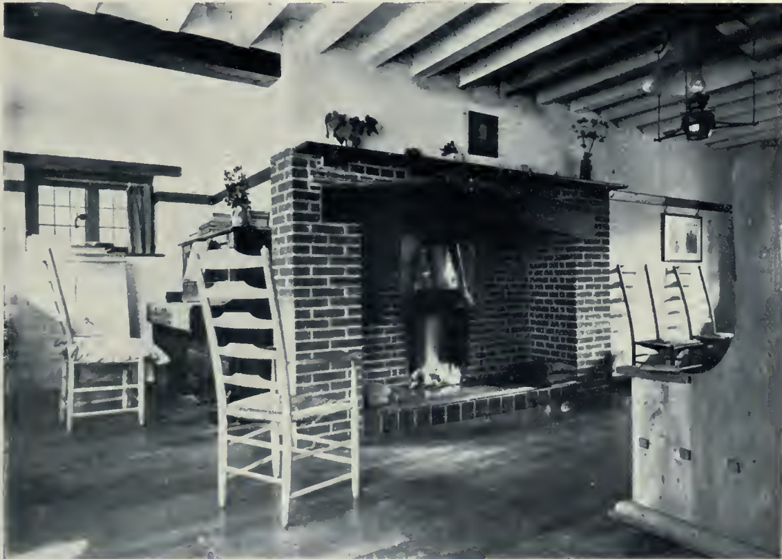
View of living room, "Laneside," the cottage to the left of the pair illustrated above. Note the delightful simplicity of this inviting little interior, with its unplastered, whitewashed brick walls, exposed ceiling joists, red brick fireplace, and the plain and severe furniture which accords so well with its surroundings. Messrs. Unwin and Parker, Architects.
