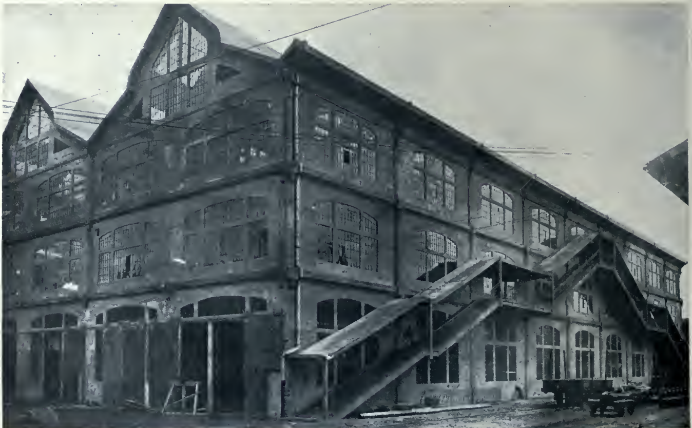
CONCRETE FACTORY, BUDAPEST, SHOWING THE OUTSIDE COVERED STAIRWAY, THE REGULATION EMERGENCY EXIT PLACED ON ALL HUNGARIAN FACTORIES, WHICH EMPLOYEES ARE REQUIRED TO USE DAILY.
