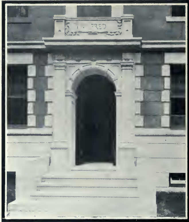
Entrance, Ivanhoe Apartments, Allston, Massachusetts. Note the excellent texture, detailed effect, and granitic appearance of the concrete.
