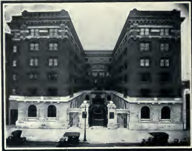
Large Modern Apartment House.—A type of building for which brick, more than any other material, is particularly well adapted.
