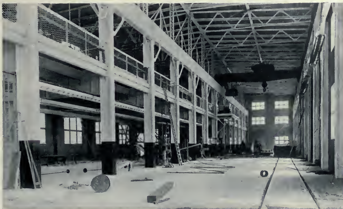
INTERIOR VIEW OF CANADIAN GENERAL ELECTRIC COMPANY'S TRANSFORMER HOUSE, PETERBORO, SHOWING THE STEEL BEAMS AND GIRDERS AND TRUSS WORK OF THE ROOF.
