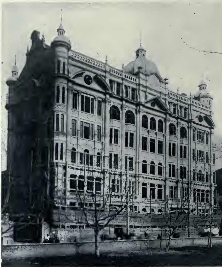
TELEPHONE BUILDING, SHANGHAI, CHINA. AN ELABORATELY DETAILED CONCRETE STRUCTURE, WHICH IS ESSENTIALLY A CARVED MONOLITH IN THAT THE EXTERIOR WAS ENTIRELY CUT BY HAND. MATHIEN & JARDIN, ARCHITECTS.
