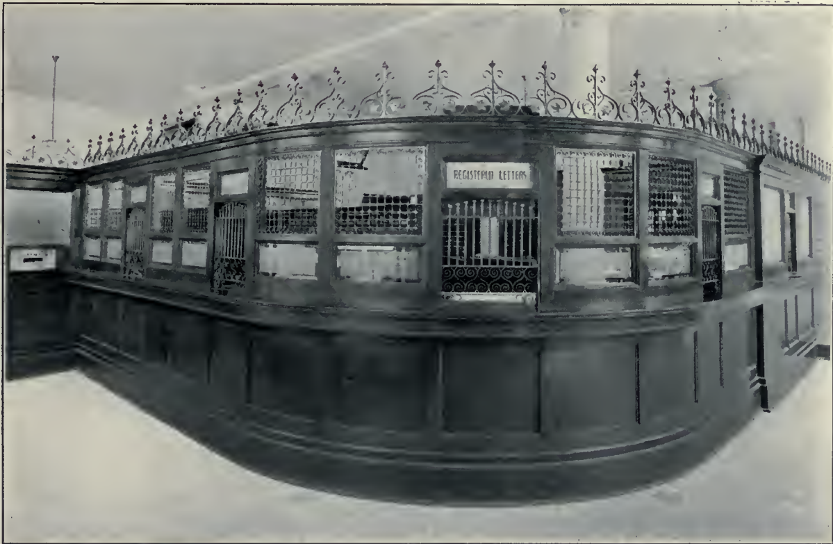
Interior of Station "F" Post Office, Corner Yonge and Charles St., Toronto
