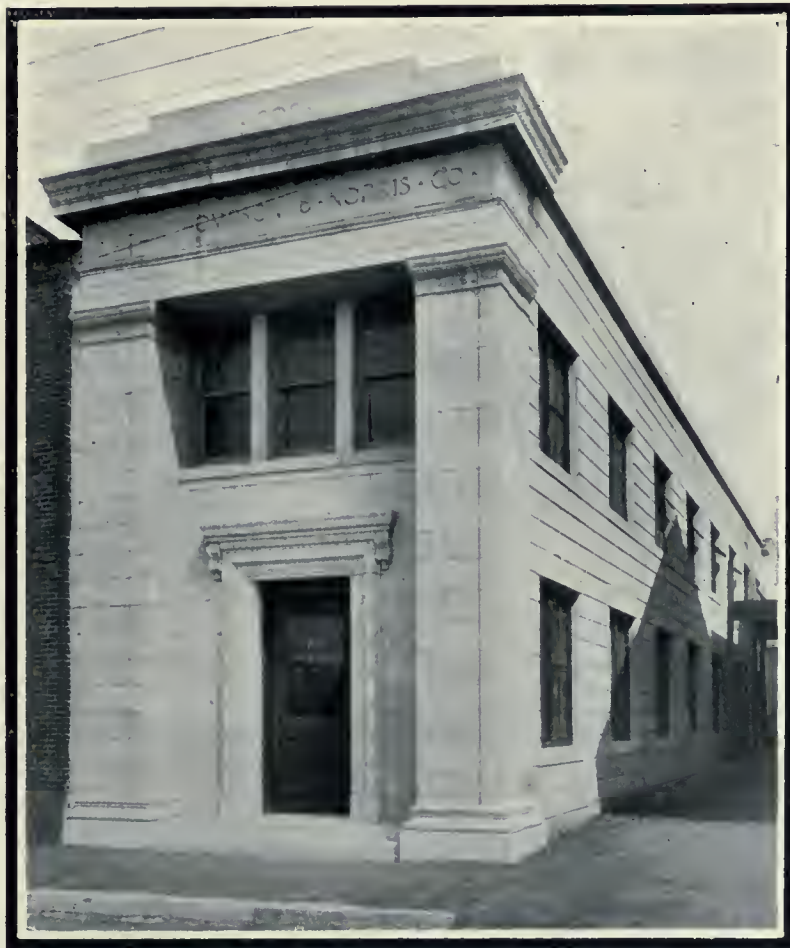
Office building, Boston. An example of artificial stone construction in which the texture of the material and the simplicity of design combine to produce a highly satisfactory and effective exterior.
