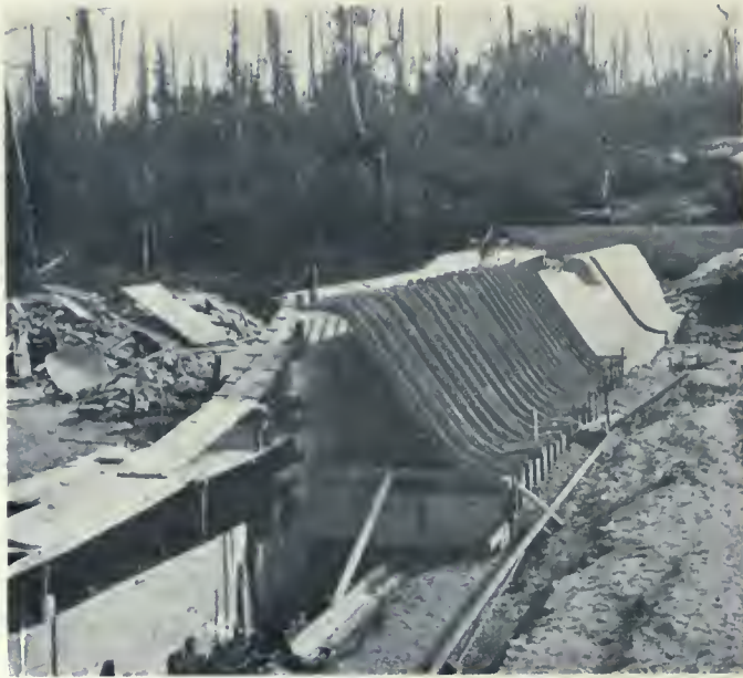
PLANT OF WOODS PRODUCTS COMPANY—DAM IN PROCESS OF CONSTRUCTION, SHOWING THE EXCAVATION INTO THE SAND FOUNDATION AT NEARLY ITS LOWEST POINT. E. D. PITT, DESIGNING AND CONSTRUCTING ENGINEER.
