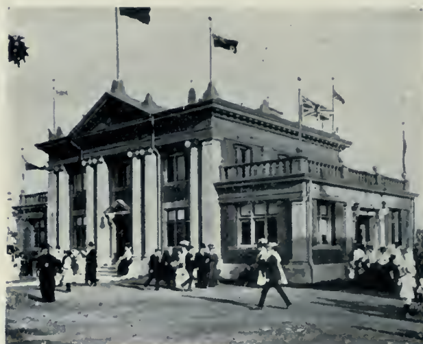
Press Building, Canadian National Exhibition Grounds, Toronto. Designed in Modern Classic and built of red pressed brick with art stone trimmings. Mr. Geo. W. Gouinlock, Architect.
