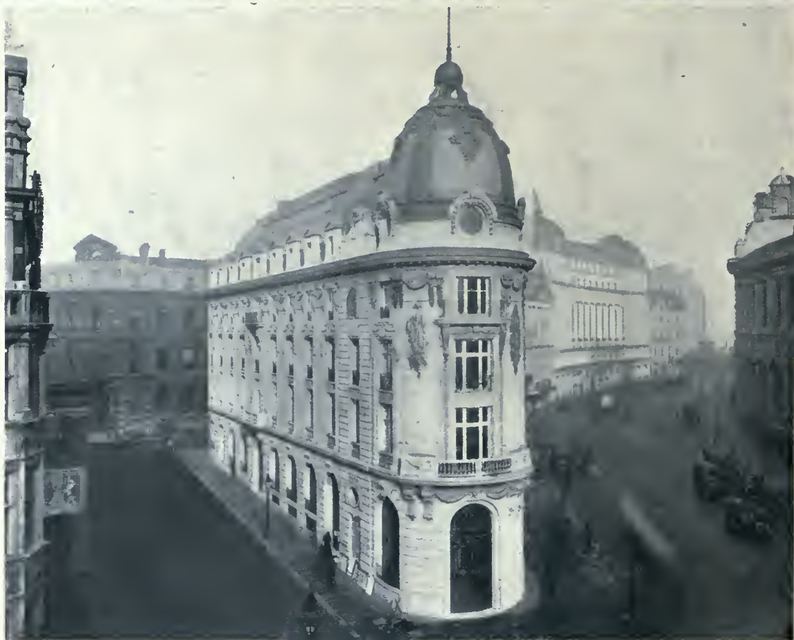
FRAME WORK AND COMPLETED BUILDING OF THE MORNING POST ON THE STRAND. THE UPPER VIEW SHOWS TO WHAT EXTENT STRUCTURAL STEEL IS BEING EMPLOYED IN THE ERECTION OF SOME OF THE MODERN BUSINESS BUILDINGS IN LONDON. MESSRS. MEWES & DAVIS, ARCHITECTS.
