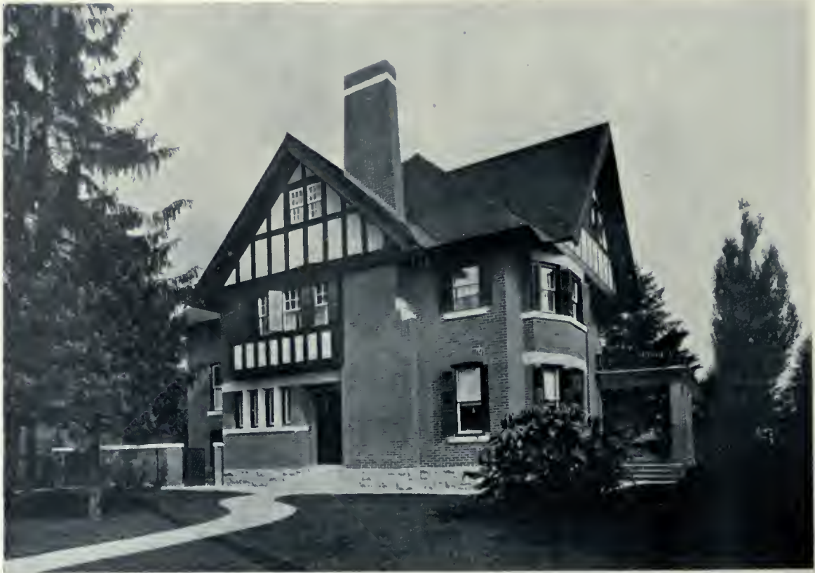
Residence of F. C. T. O'Hara, Wurtemberg Street, Ottawa. This house, which is situated on the high bank of the Rideau River, is built of common red brick, with white joints, limestone trimmings and half timbered gables. The large main chimney in the position it is placed suggests solitude and comfort, as well as adding interest to the whole scheme. Mr. C. P. Meredith, Architect.
