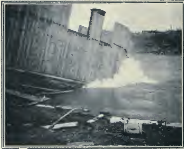
LAUNCHING A CAISSON AT FORDHAM HEIGHTS, NEW YORK.
