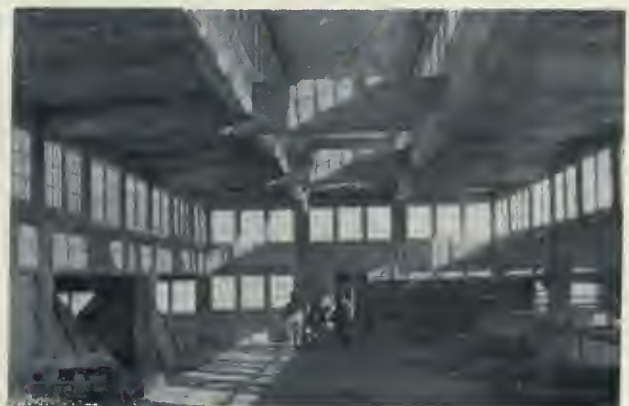
PLANT OF WOOD PRODUCTS COMPANY—ACETATE ROOM OF OVEN HOUSE WHICH STANDS OVER THE TOPS OF FOUR PAIR OF 12 CORD RETORTS AND IS USED FOR DRYING MOISTURE FROM ACETATE OF LIME. ENTIRE ROOM SYSTEM IS CARRIED ON THREE GREAT GIRDERS SHOWN IN THE FOREGROUND. DIMENSIONS 33 FT. X 107 FT. X 16 FT. HIGH. E. D. PITT, DESIGNING AND CONSTRUCTING ENGINEER.
