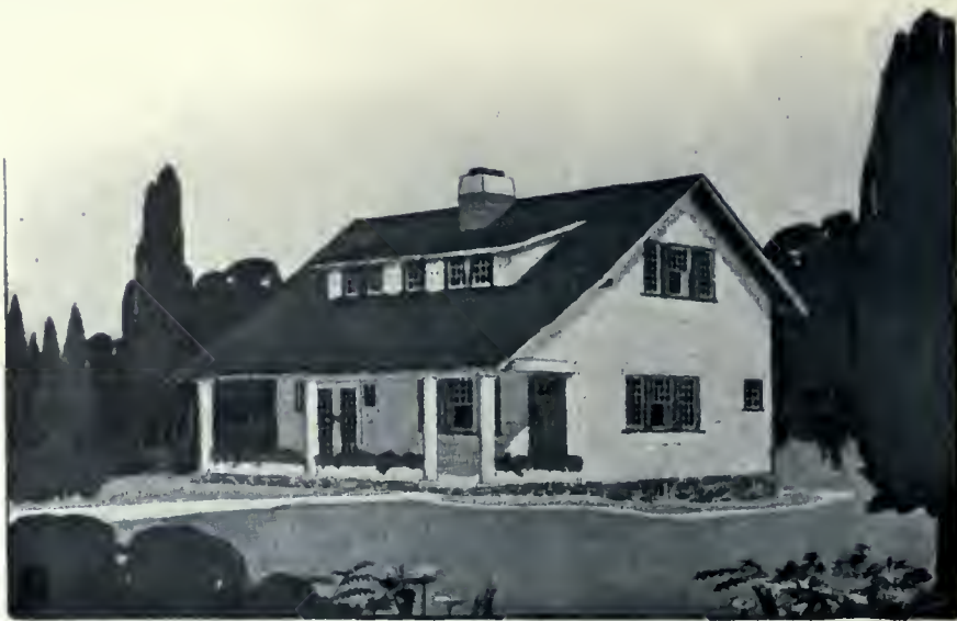
Design No. 2.—Excellent design for an inexpensive farm house, which demands the environment either of the open country or of a village where there is sufficient space to give plenty of grass and trees as its immediate surroundings. The walls are sheathed with rived cypress shingles, chemically darkened to a brown weathered tint. The foundation is of field-stone.
