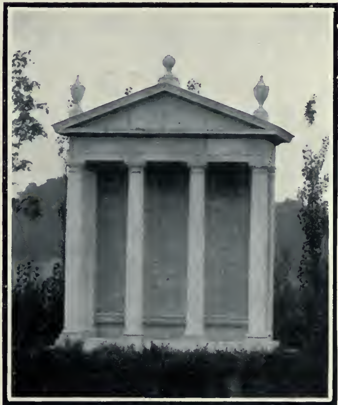
Temple in formal garden, private Estate, Massachusetts, built entirely of ornamental concrete stone.
