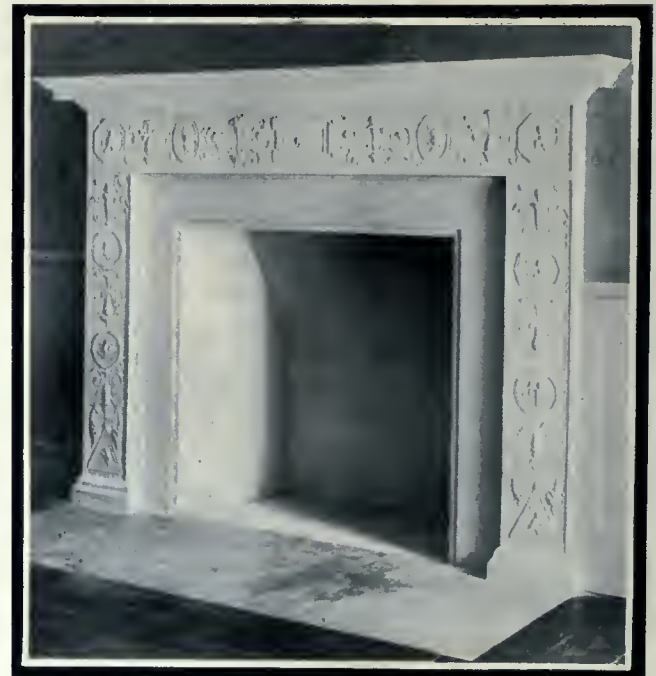
Concrete Mantel, private house, Boston. Both in design and texture of material this mantel is especially worthy of note.
