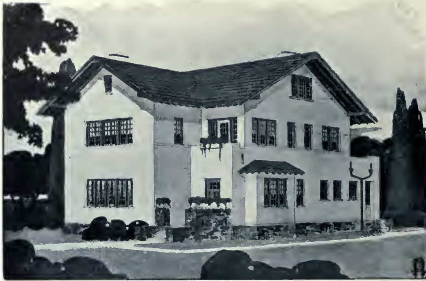
Design No. 1.—An eight-roomed cement house, suitable for a town, village or country. It is designed on simple lines, that harmonize with almost any surroundings. The walls are constructed of vitrified terra cotta blocks, directly upon which the plaster is applied, both outside and inside. The foundation is of field-stone, laid in black cement.
