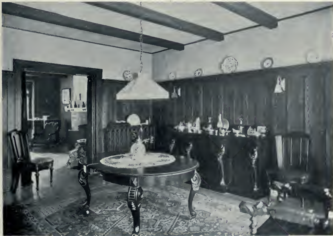
Dining Room, Home of R. L. Cowan, Toronto, looking towards the living room, and showing the effective wall panelling and beamed ceiling. The rear of this room opens on to a verandah. Messrs. Chadwick and Beckett, Architects.
