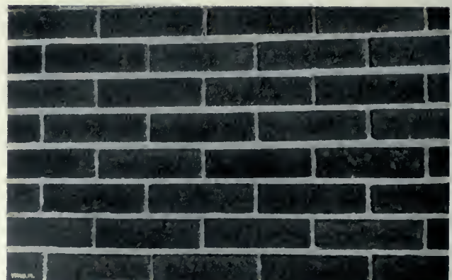
Fig. 9.—A wall of brick of ordinary size, laid up in a running bond with the conventional 3/8 inch, raked, white joints. The color scheme, however, is noteworthy, the effect being produced with bricks of clear red, and reds with finished edges.
