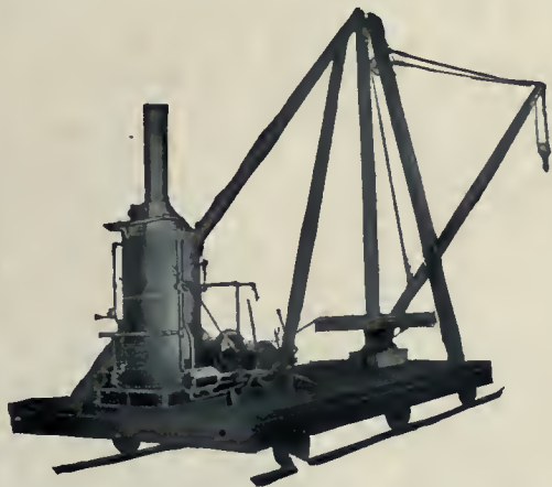
Travelling Derrick and Hoist
