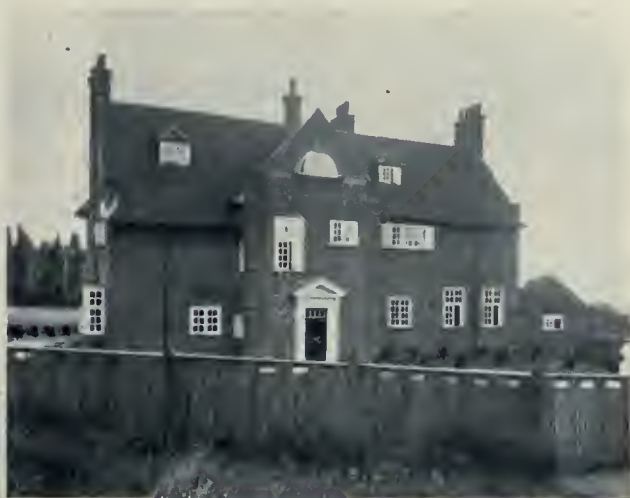
House at Elwell, looking towards the entrance. A simple, effective, brick building in which the only attempt at ornamentation is seen in the slightly emphasized quoins of the entrance bay and the arches above the windows. Mr. Guy Dawber, Architect.
