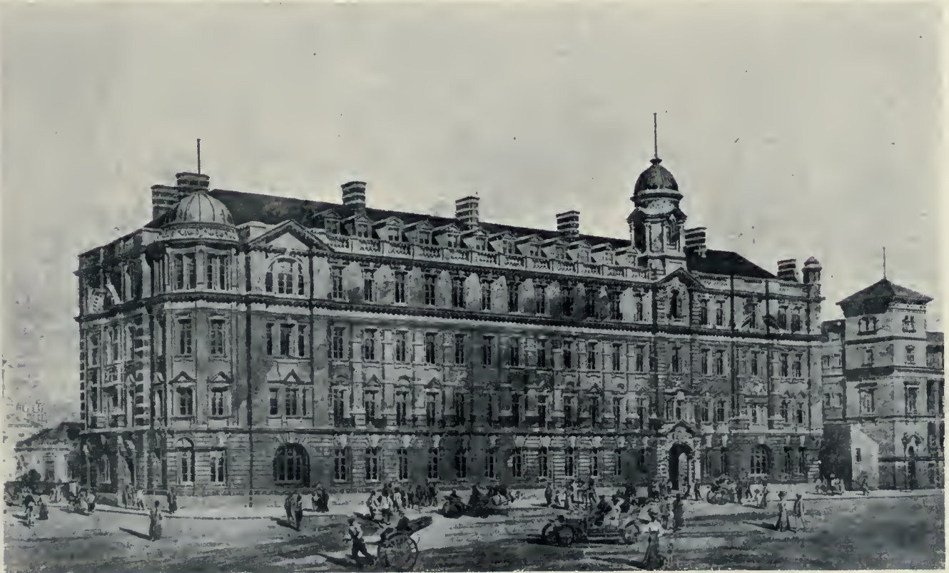
Ta Ching Government Bank, Shanghai, China. A recent example of Western World architecture in the Orient. Atkinson & Dallas, Shanghai, Architects.
