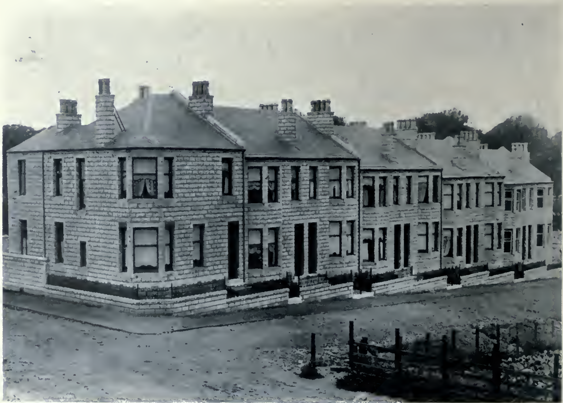
Terrace of concrete block houses at Burnside (near Glasgow), Scotland, providing accommodation for nine families. This illustration shows how well adapted this material is to meet the needs of economical and well constructed dwellings of the attached type.
