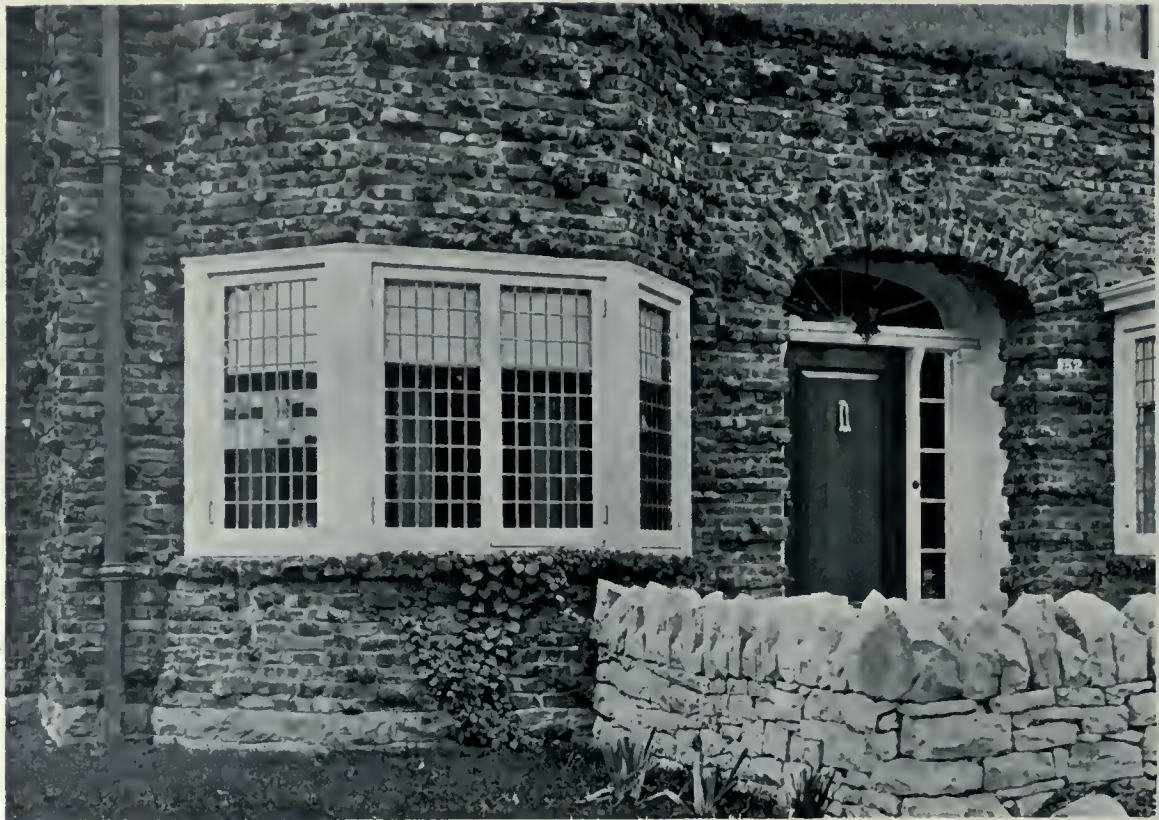
Detail of clinker brick walls and stone work, Residence of Architect Wm. F. Sparling, Toronto. Note the general ruggedness and striking rustic effect of the masonry.
