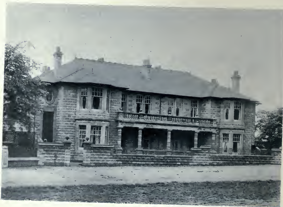
Four family concrete block house, Paisley, Scotland. Note how monotony of rock face is relieved by introduction of panel blocks and broken ashlar effects.
