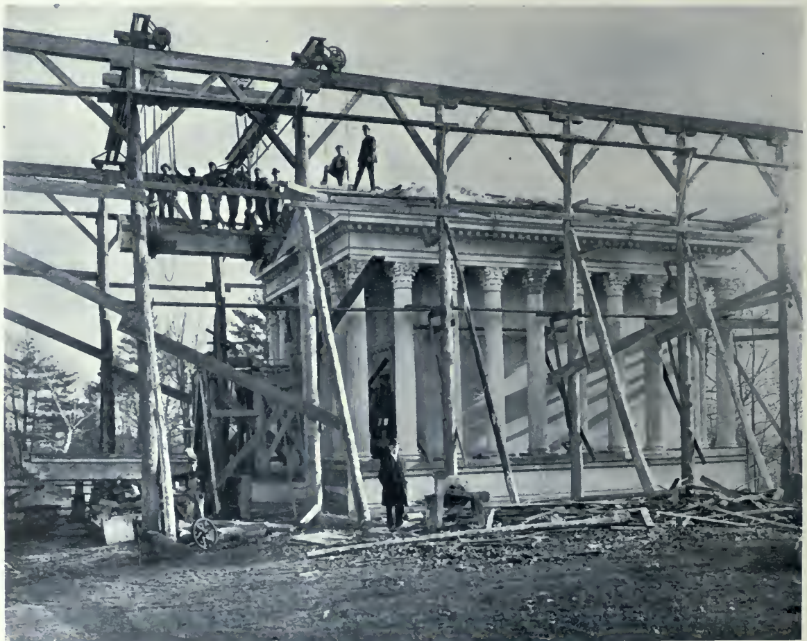
THE EATON MAUSOLEUM, MOUNT PLEASANT CEMETERY, TORONTO, SHOWING SCAFFOLDING USED IN ITS ERECTION. ARCHITECTS SPROATT AND ROLPH, DESIGNERS.
