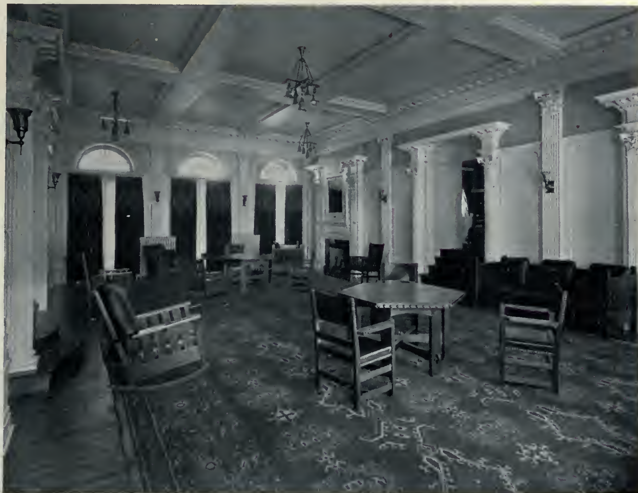
Reception Hall, Nurses' Residence, Sick Children's Hospital, Toronto.—Sproatt & Rolph, Architects.
