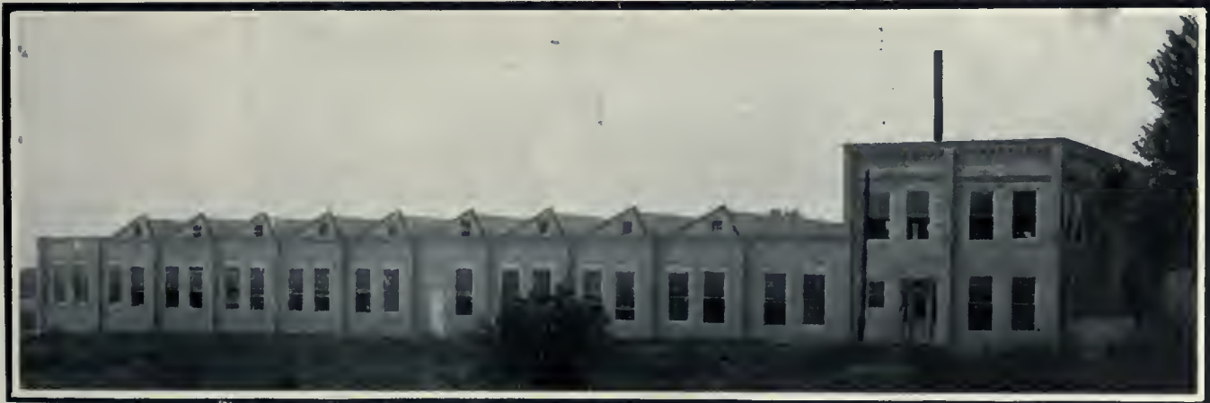
Concrete block machine shop erected for the Wolverine Motor Works, Bridgeport, Connecticut. According to the statement of the owners, who made the blocks themselves, the complete cost of this building (120 ft. by 240 ft., and 24 ft. to top of saw-tooth roof) was $2,800, the cost of blocks being six cents each.
