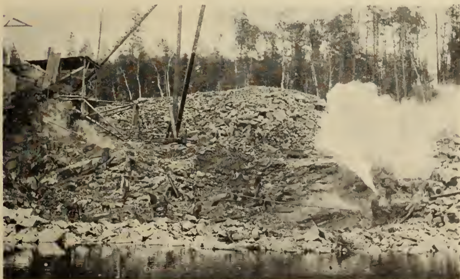
STARTING EXCAVATING FOR THE POWER HOUSE AT THE BEACH BROS. PLANT, MONTREAL RIVER
