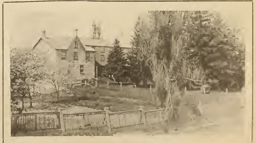
AN OLD ACADEMY—IN DIRE NEED OF RESTORATION
