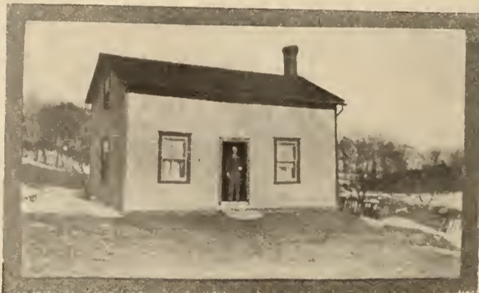
THE ORIGINAL STRUCTURE
