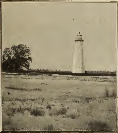
WHERE THE LIGHT-HOUSE TOWERS
