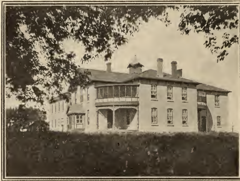
HOSPITAL BUILDING, PORTAGE LA PRAIRIE
