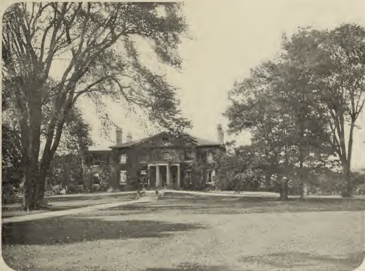
"THE GRANGE," RESIDENCE OF MR. GOLDWIN SMITH.
