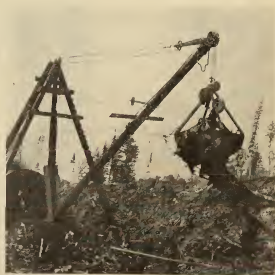
CANAL MAKING—TRAVELLING DERRICK REMOVING STUMPS
