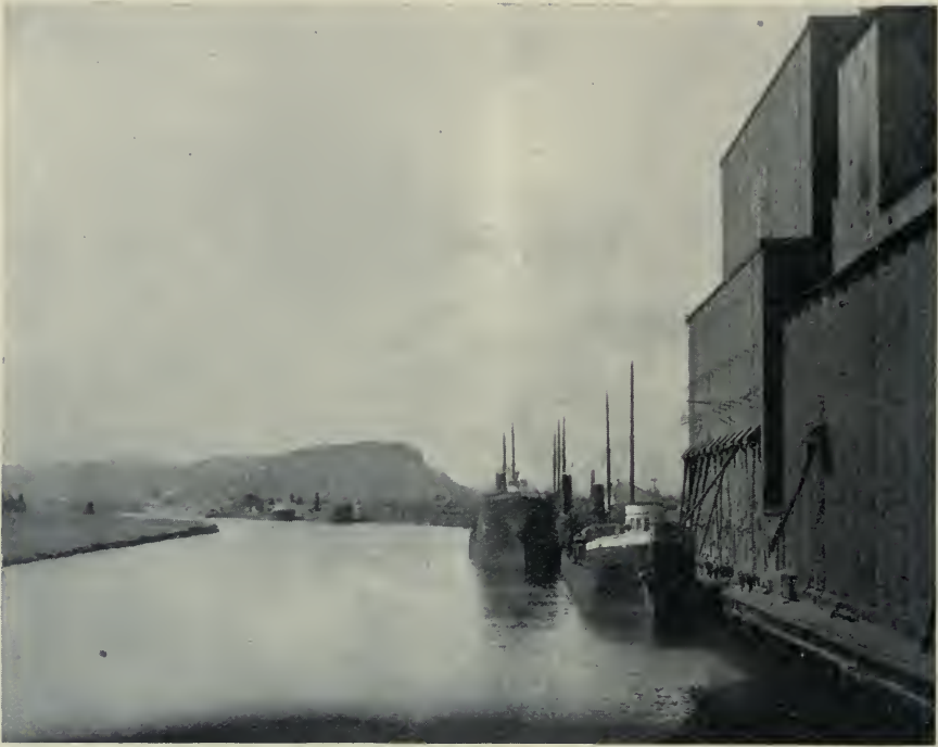
LOADING A GRAIN BOAT AT ELEVATOR "B," FORT WILLIAM
