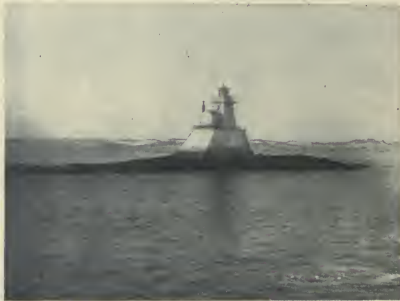
MARKING A DANGEROUS ROCK THE LIGHT ON ALGERNON ROCK, ST. LAWRENCE RIVER
