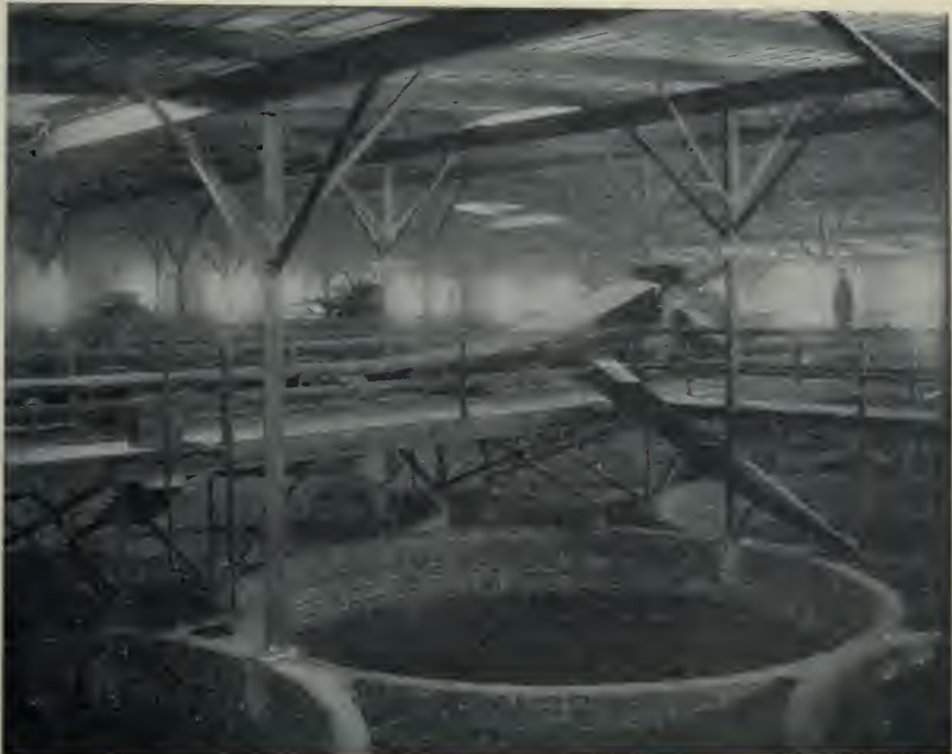
THE CIRCULAR BINS THAT HOLD THE WHEAT A SCENE IN ONE OF THE BIG ELEVATORS, LOOKING DOWN ON THE TOPS OF THE BINS
