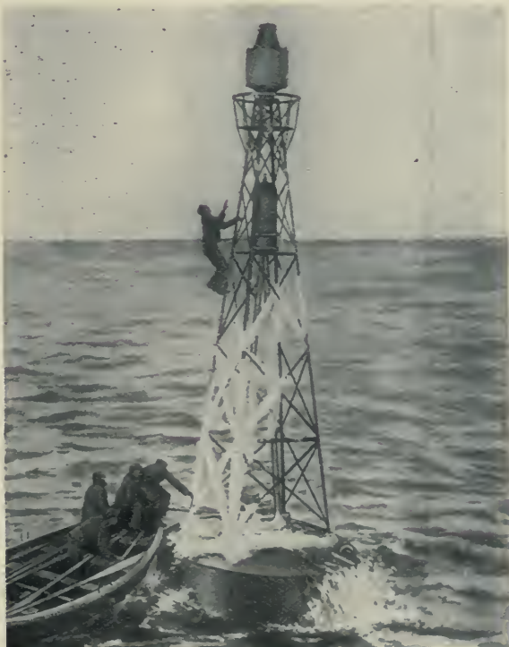
A GAS BUOY
