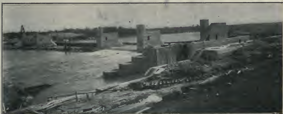
THE DAM AND ABUTMENTS AS THEY APPEARED BEFORE THE SUPERSTRUCTURE WAS PUT IN PLACE
