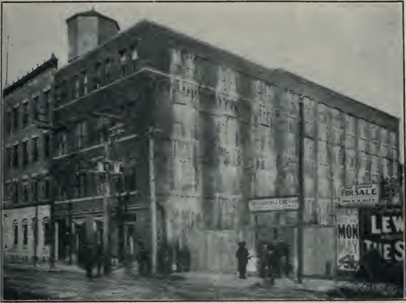
A WATER CURTAIN, IN OPERATION
