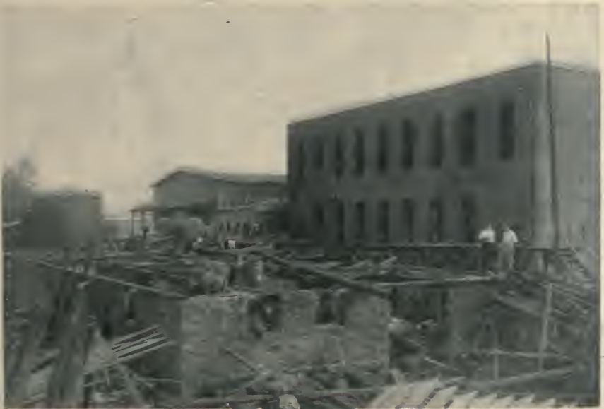
SAVED BY AUTOMATIC SPRINKLERS
