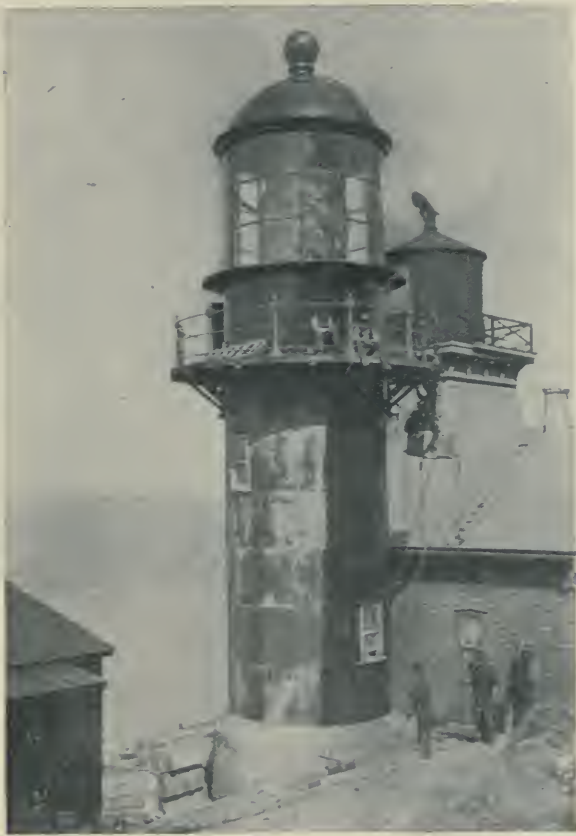
FAME POINT LIGHTHOUSE AN IMPORTANT BEACON ON THE ST. LAWRENCE ROUTE
