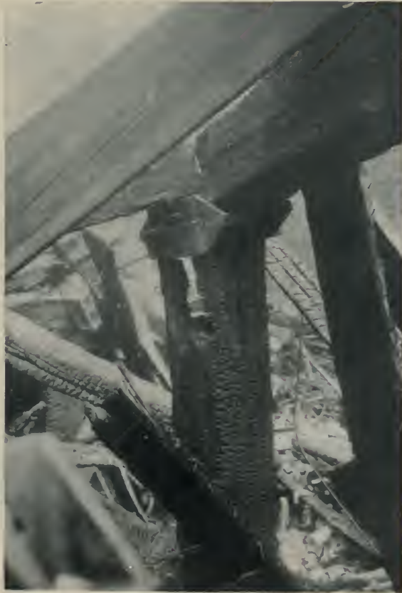
DRY ROT IN TIMBERS
