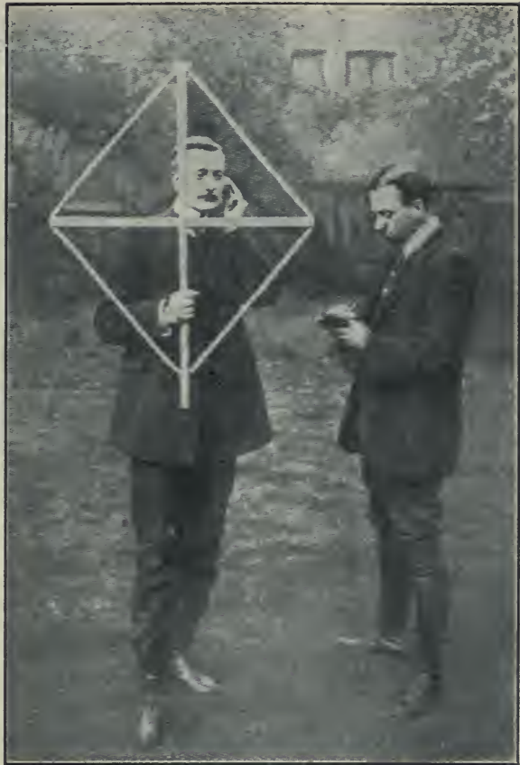
A PORTABLE WIRELESS STATION
