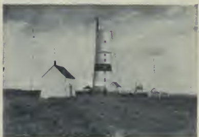
HEATH POINT, ANTICOSTI IN PROCESS OF CONSTRUCTION
