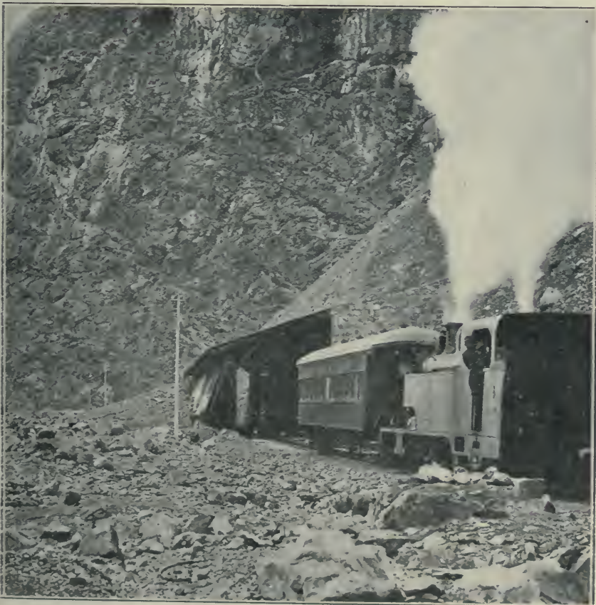
ENTERING THE ANDINE TUNNEL
