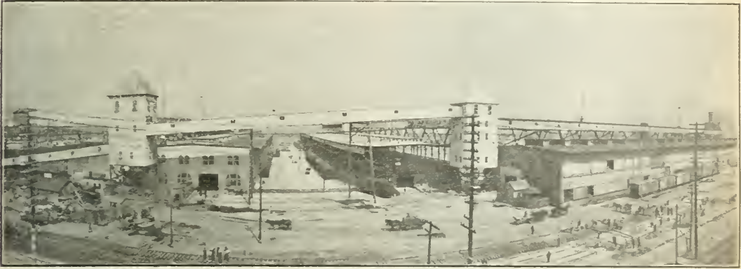
A View of the Completed King Edward Pier, Montreal.
