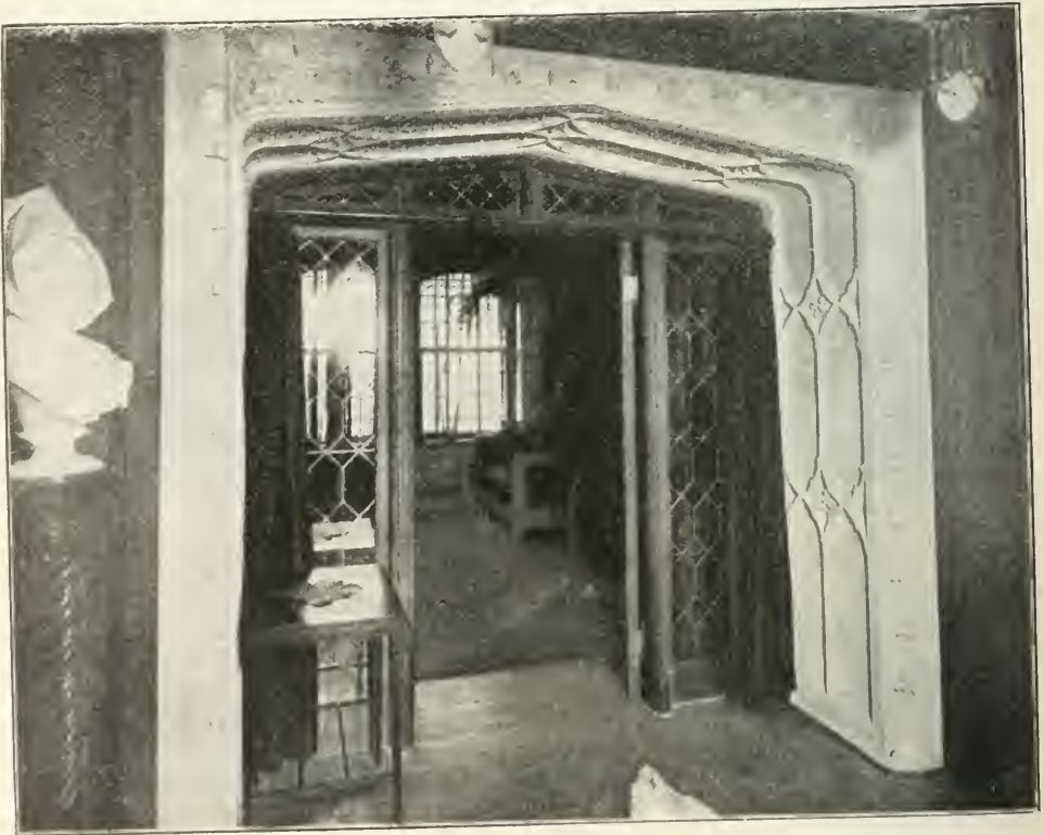
Mr. William J. Matheson's Flat Dwelling New York City, showing a Doorway in Concrete
