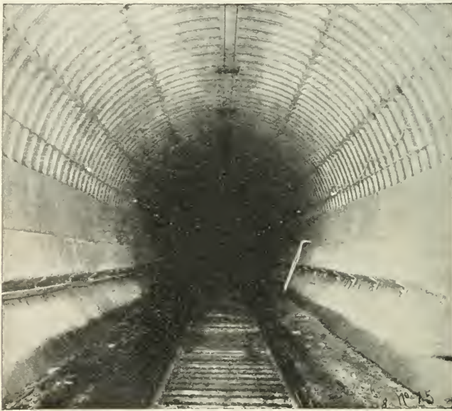
Interior of St. Clair Tunnel
