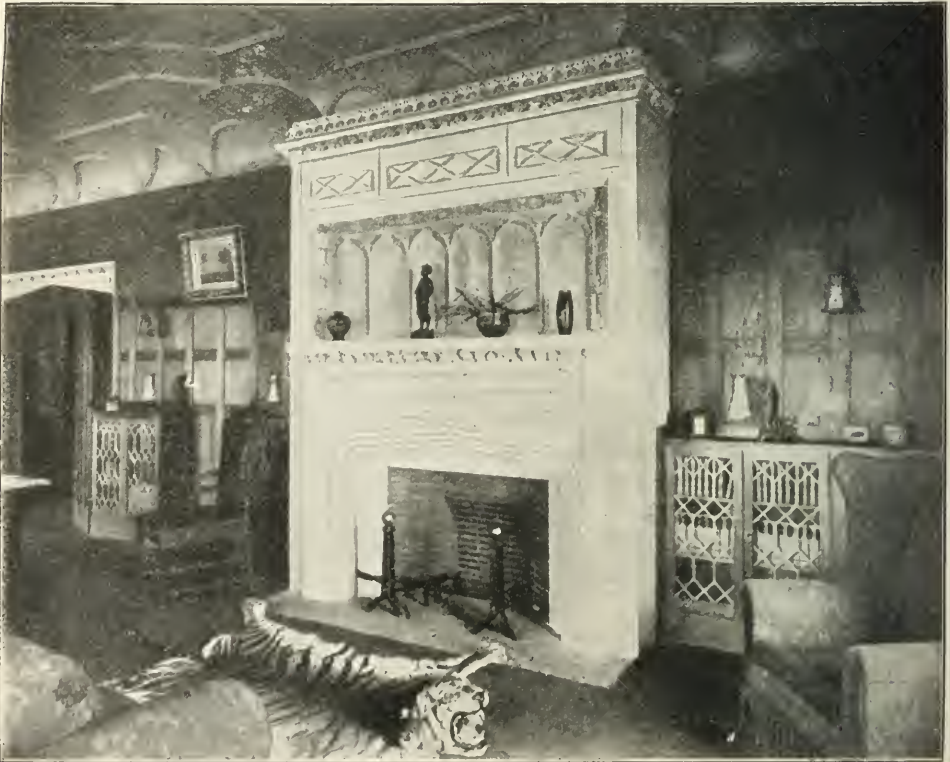
Interior of Flat Dwelling of Mr. William J. Matheson, New York City, showing the Use of Concrete for Hearth Fronts
