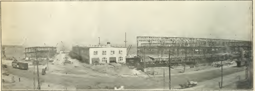
A View of the Completed Jacques Cartier Pier, Montreal.
