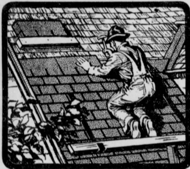
Giant Shingles are made and laid three at a time. This saves laying costs.
