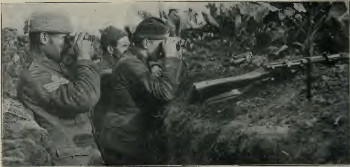
THE ENFORCED INACTIVITY OF DAYLIGHT IN THE TRENCHES IS SOMETIMES HARDER ON THE SOLDIER'S NERVE THAN HAVING TO FACE A REGIMENT OF RIFLEMEN
