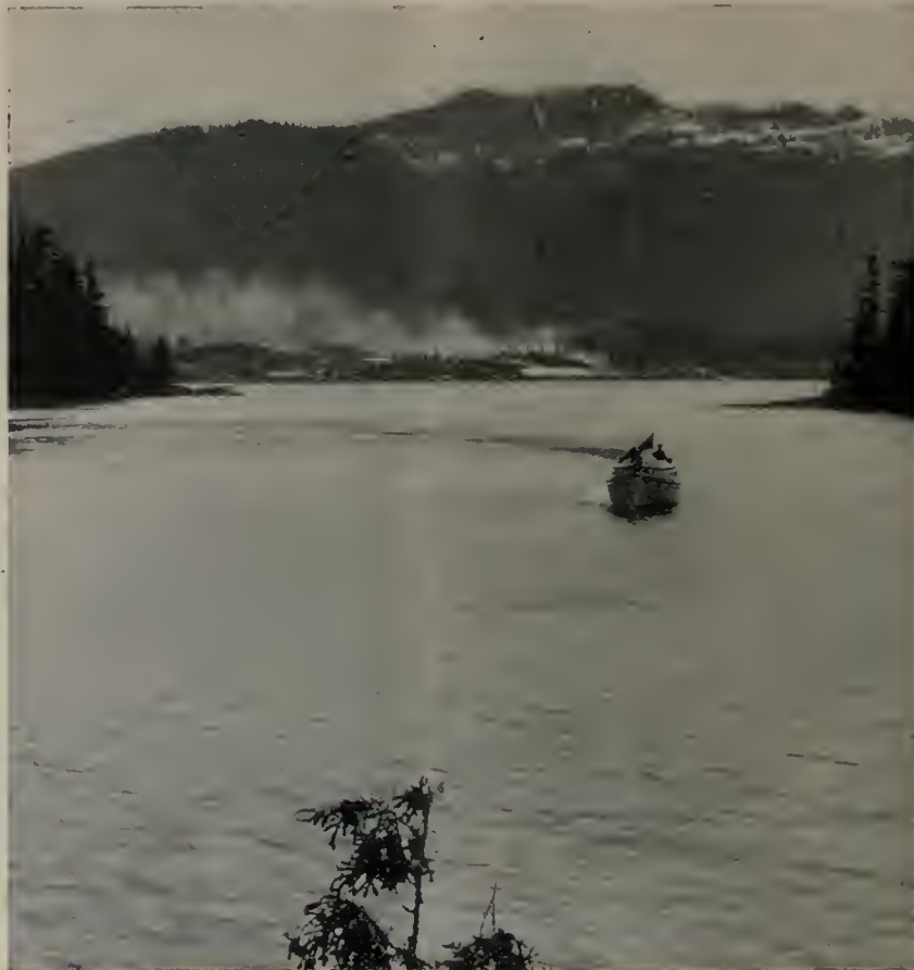
THE HARBOR ENTRANCE TO THE TERMINUS OF THE G. T. P.—THE COMPLETION OF WHICH IS JOTTED DOWN TO THE CREDIT OF E. J. CHAMBERLIN
