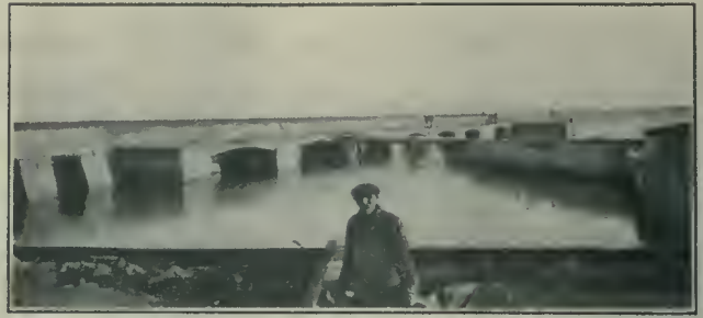
Dock at Grand Banks formed by new pier and breakwater.
