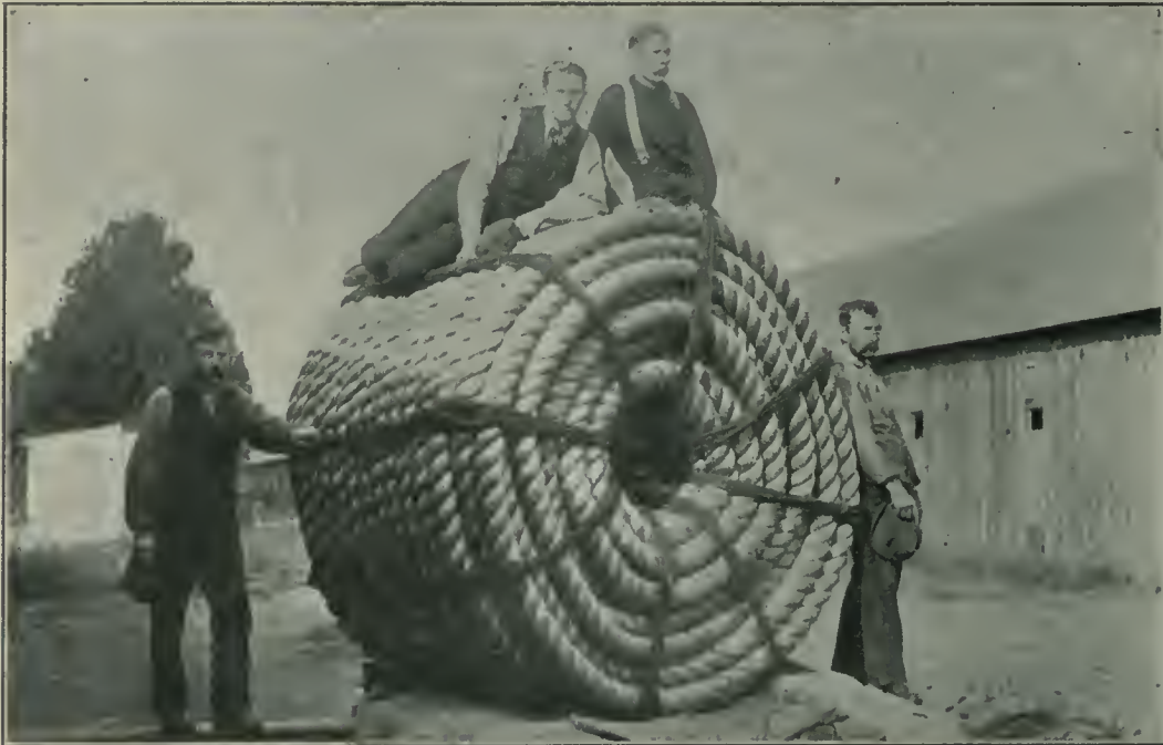
1,320 Feet of 12 Inch Manila Tow Line, Weighing 6,410 lbs., Made by The Consumers Cordage Co. Ltd., Dartmouth, N.S.
