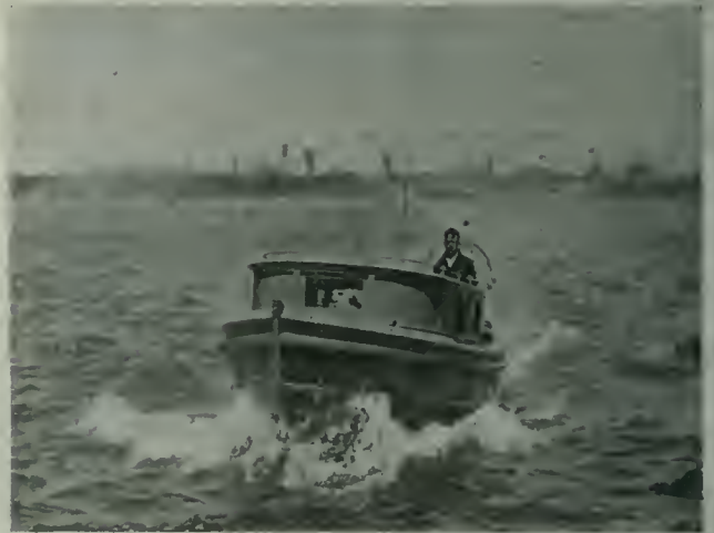
Bow View of Lighthouse Tender.
