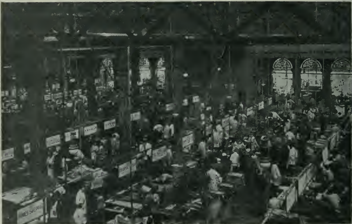
An Interior View of the Section of the Market.
