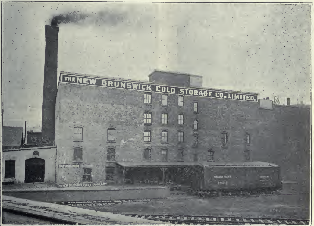
1.—The New Brunswick Cold Storage Co., Limited, St. John, N.B., main building, as seen from City Yards; Canadian Pacific Railway Fish Dept., in shadow.
