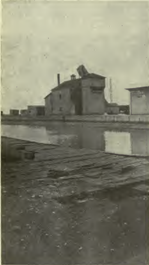
Fertilizer Plant, Port Stanley Supply Co., Port Stanley, Ont.
