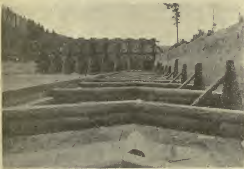
Looking up the race at Quesnel Dam, showing the construction of the fish-way on the floor of the race. The gates being closed.
