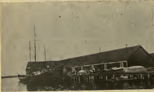
Plant of the Consumers Fish & Cold Storage Co., Ltd., Yarmouth, N.S.
