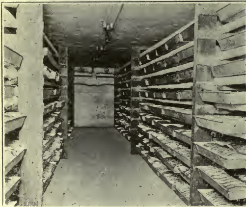
3.—The New Brunswick Cold Storage Co., Limited, St. John, N.B. One of the five sharp freezers, with pans.
