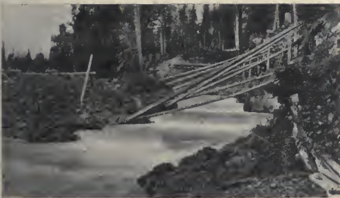
The Fish-way at Meziaden Falls, Naas River watershed, B.C. The cross timbers shown brace the retaining wall to prevent ground from filling the basins.
