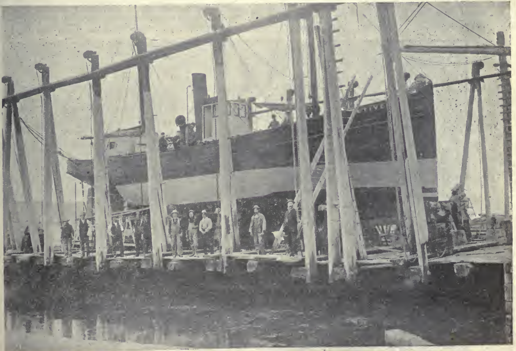
Wooden Steam Trawler "Active" on Marine Railway.
