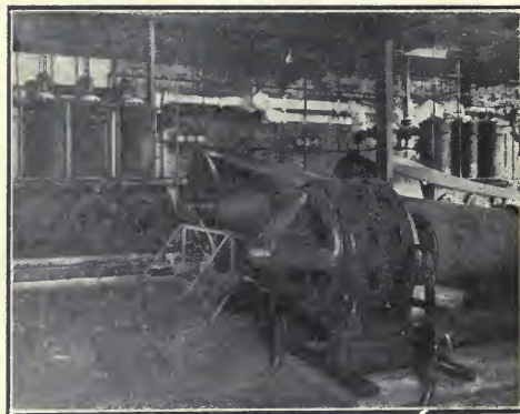
3 York Ammonia Compr. at Newfoundland Atlantic Fisheries' Plant
