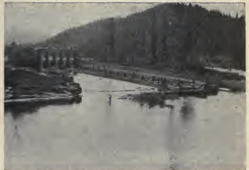
The Fish-way of Quesnel Dam, showing construction.
