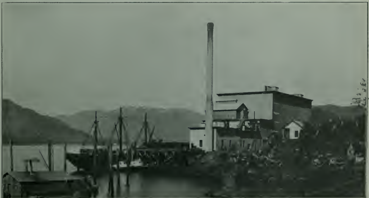
Canadian Fish and Cold Storage Plant, Prince Rupert, B. C.
