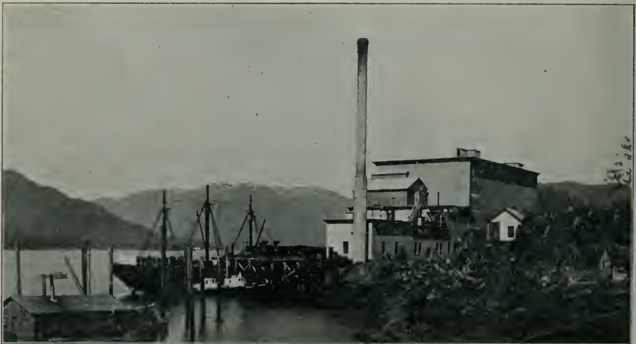
Canadian Fish and Cold Storage Company's Plant, Prince Rupert, B. C.
