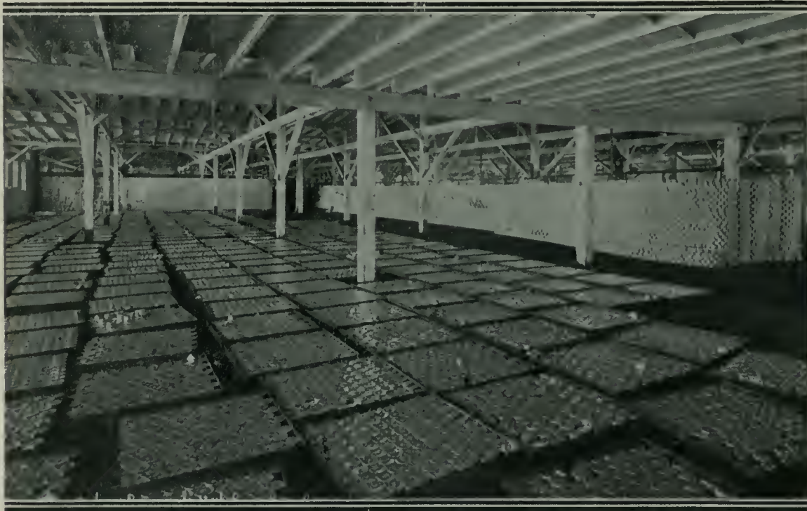
Photo, Broadbridge) COOLING ROOM, SCOTTISH CANADIAN CANNERY.
