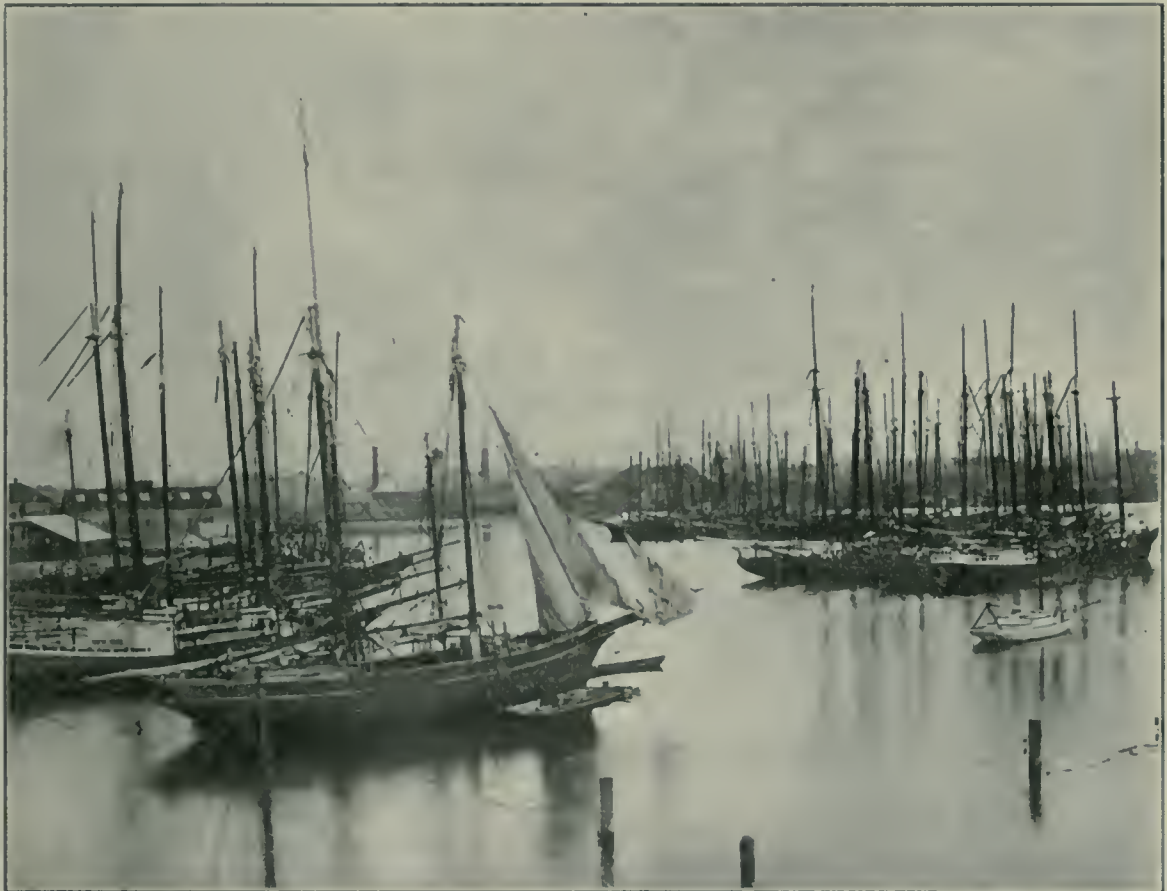
The Sealing Fleet in Victoria, B. C., when Sealing was at its height
