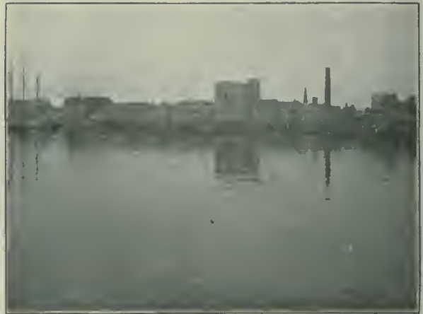
Plant and Wharves of the Lockport Cold Storage Co.
