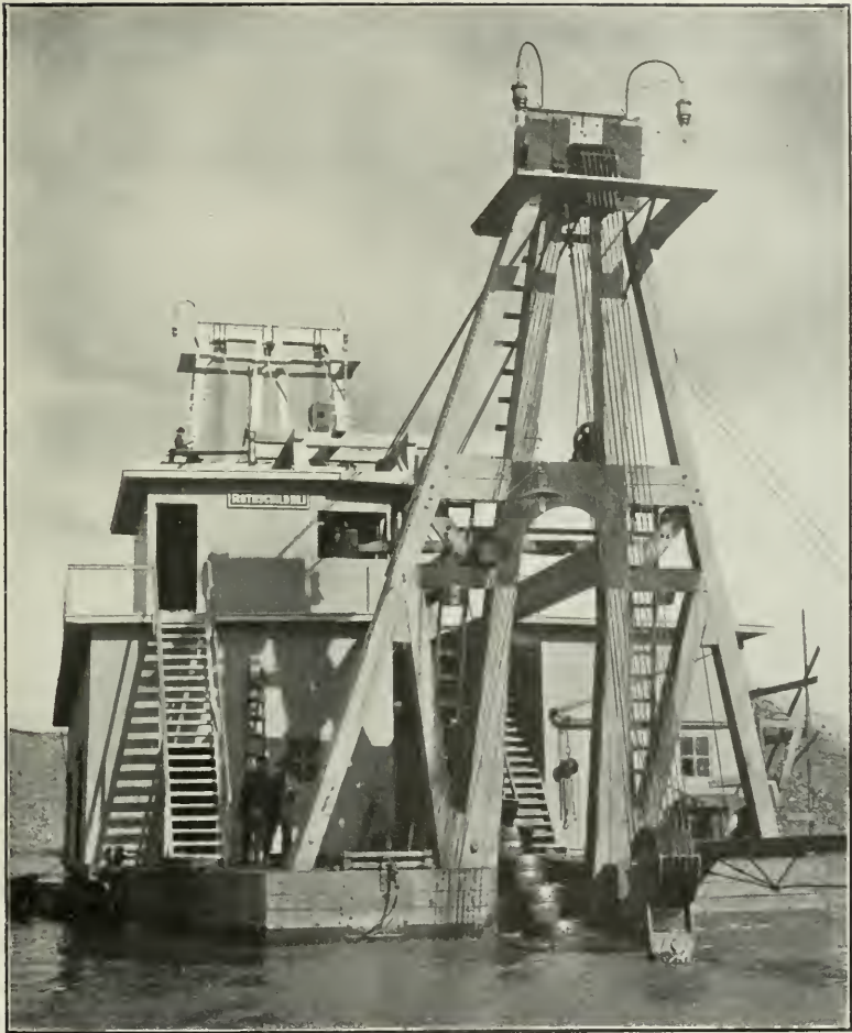
Front view of Dredge No. 1 at Bear Creek.
