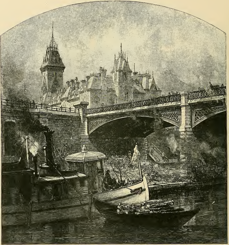
UNDER DUFFERIN BRIDGE.
