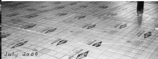
Tubing for in floor heating and insulation
