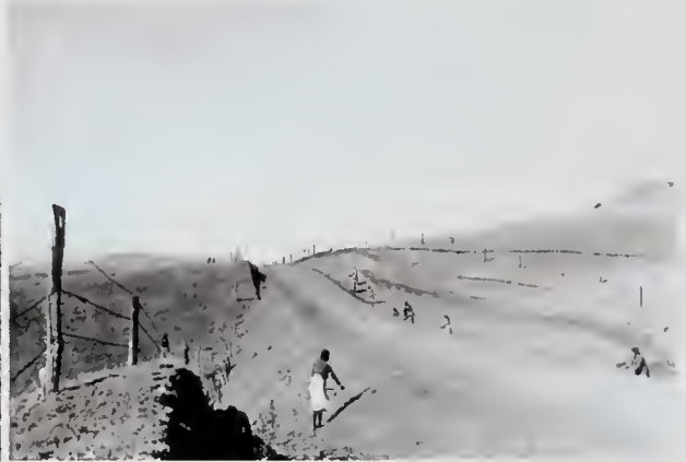
Even the women helped with construction of the roads.
