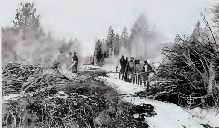
Clearing brush to build roads.
