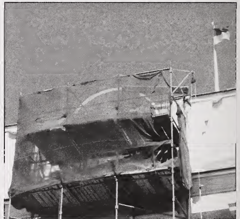
The Parliament of Ukraine with the old Soviet emblems finally being removed from the building in May 2000.
