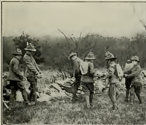
"GOOD TURN." Scouts repairing a stone wall.
