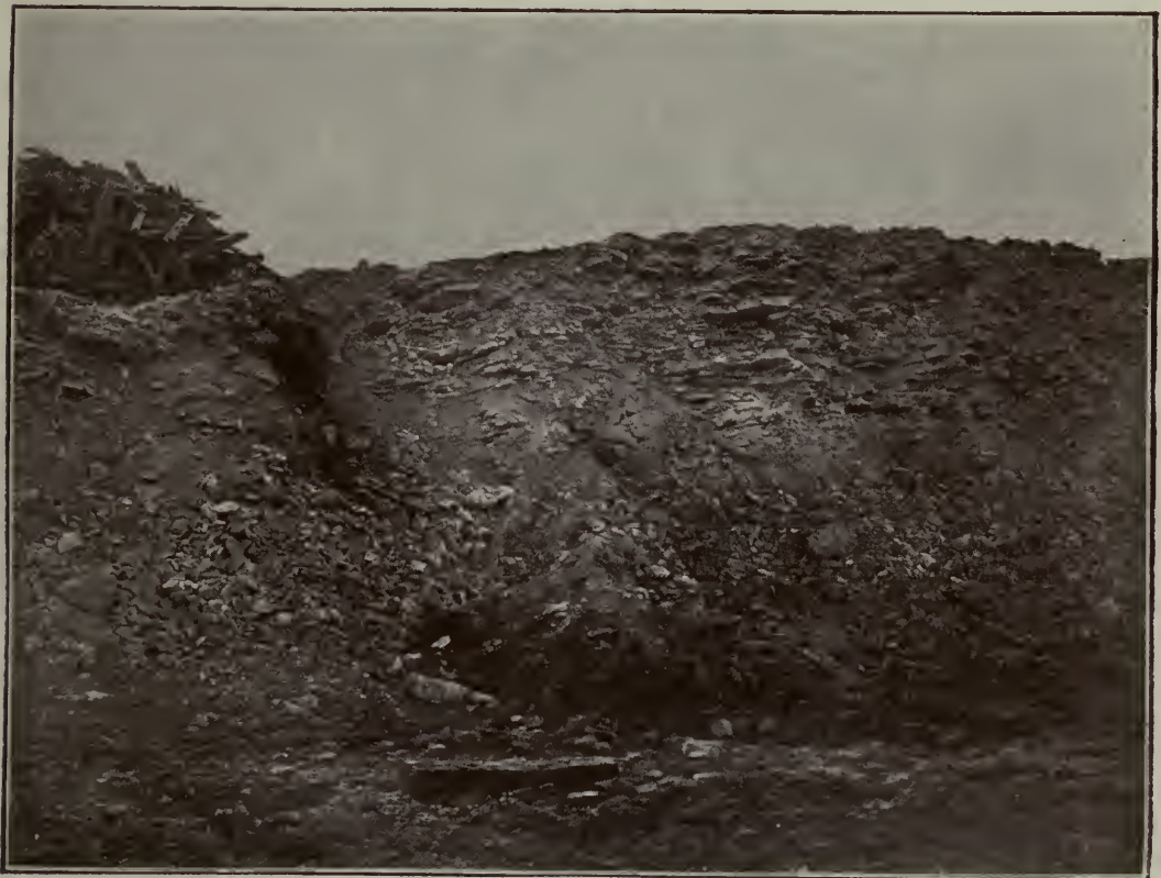
B. Face of quarry, Manitoba Gypsum Company, Gypsumville, Man. Note the bedded structure of the gypsum.
