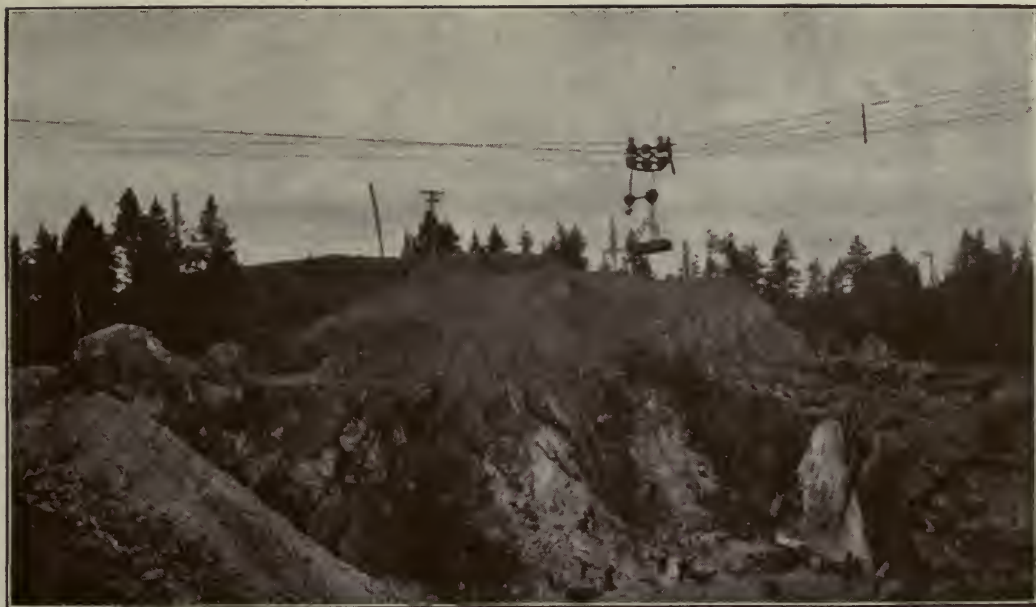
A. General view of the quarry of the Maritime Gypsum Company, Nappan, N.S., showing aerial cableway and carrier.
