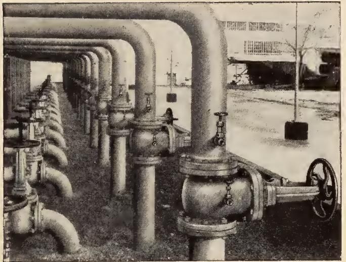
▲ **COOLING TOWER LINES** featuring Crane 200-pound W.O.G. iron body double-disc gate valves.
