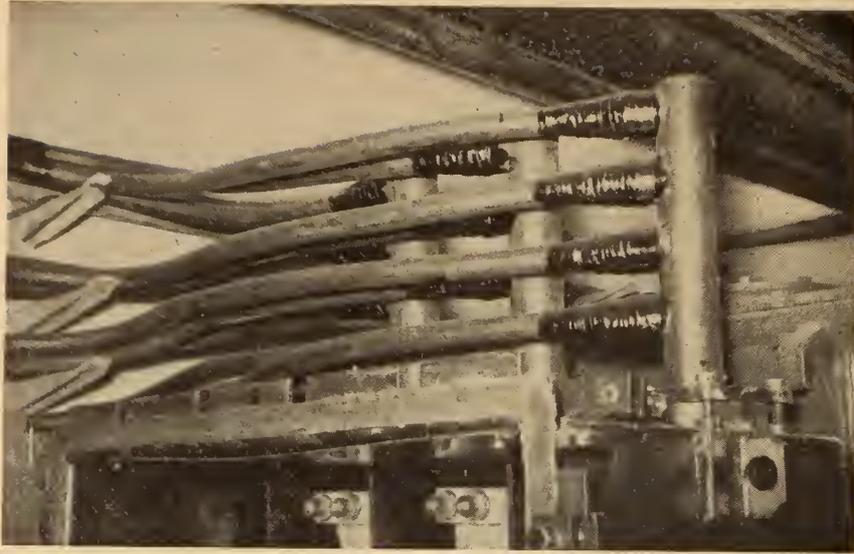
Fig. 8. Stud moles mounted on top of protector.
