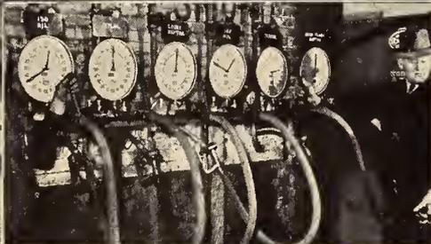
With demand for closer control pointing to positive displacement meters as the *only* accurate, dependable way to measure liquids, Neptune meters are already "proving out" with 100 different liquids. Photos at left show metering of 10 of these, including liquid soap, liquid sugar, water, acetone and corn syrup.
