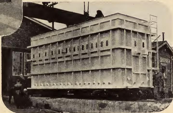
*One of 24 combustion furnace casings*
