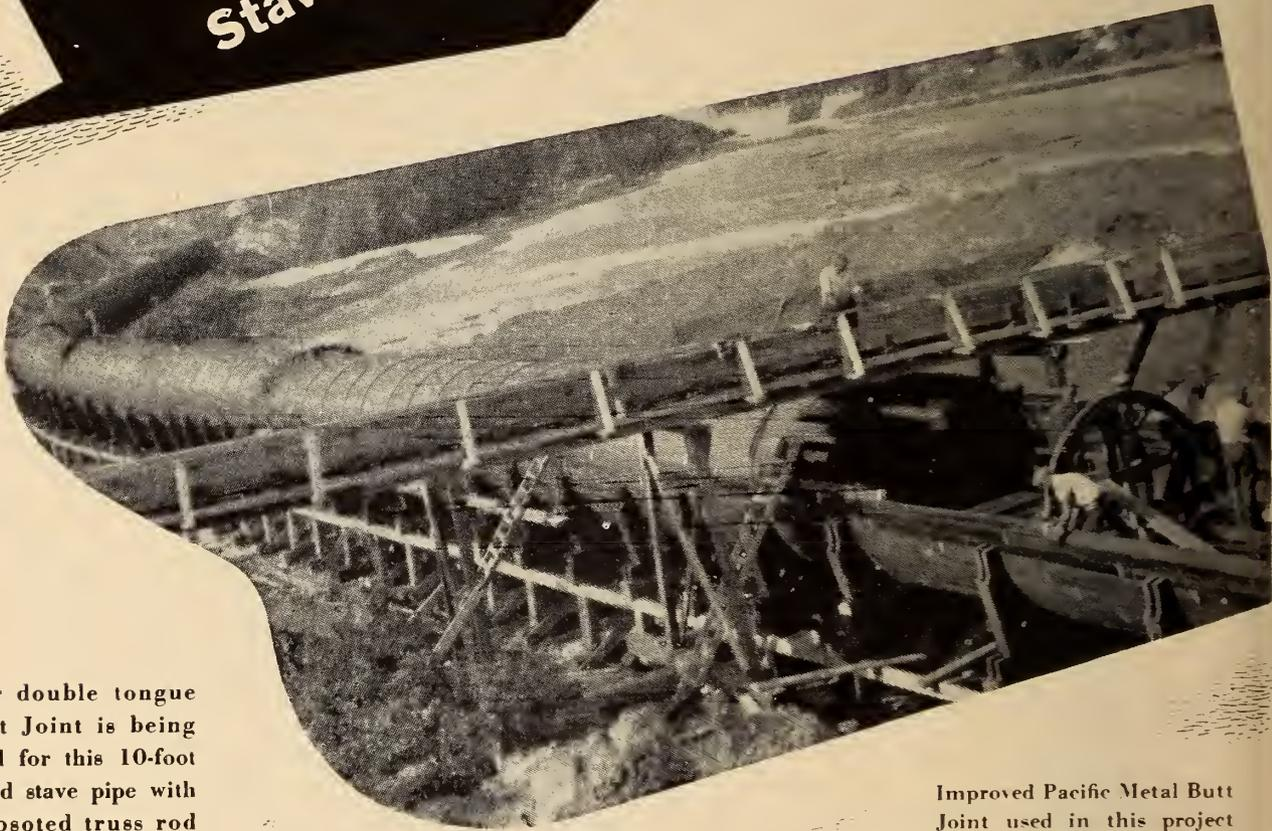
Our double tongue Butt Joint is being used for this 10-foot wood stave pipe with creosoted truss rod cradles, recently constructed in Western Ontario.
