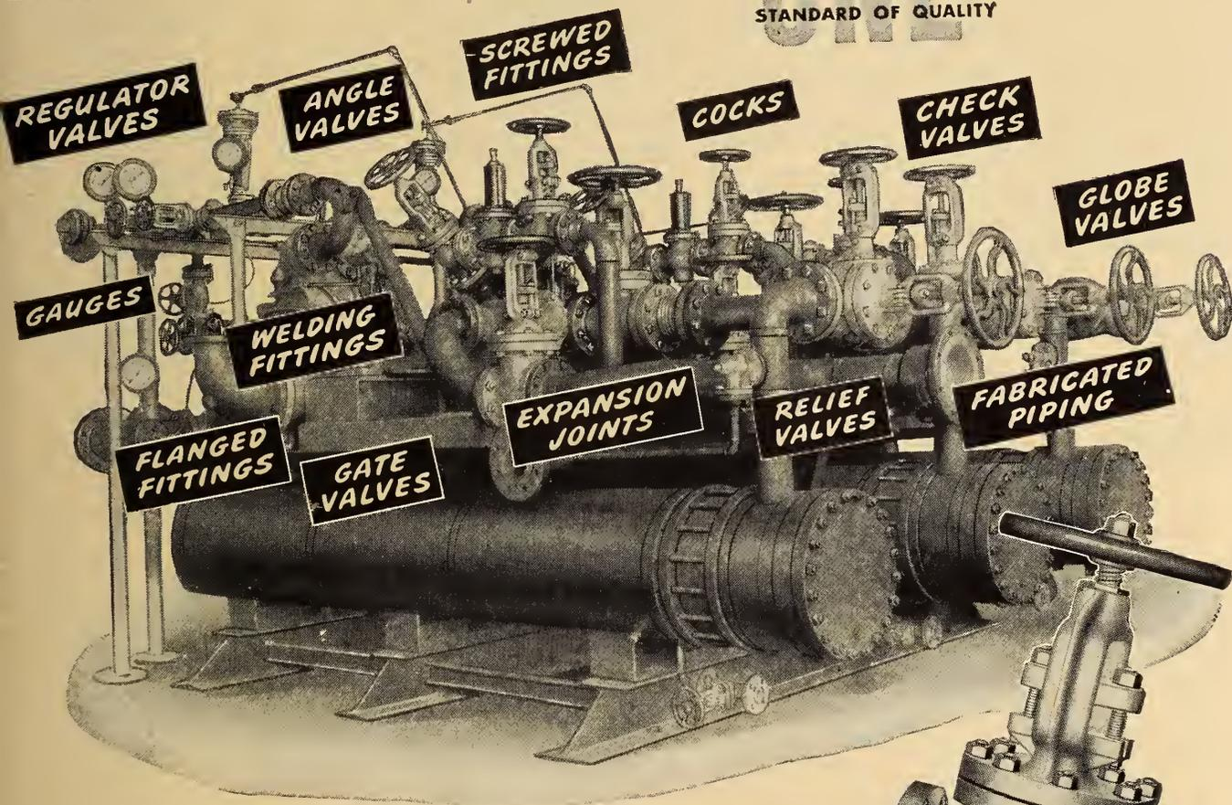
Fuel Oil Pumping and Heating Unit — equipped by Crane.
