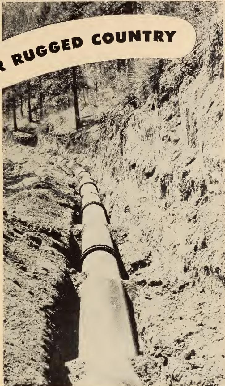
● In mountainous country like this, a water line has to be *tough*. And this Dresser-Coupled steel line can really take it. Strong, shatterproof lengths of steel pipe are connected with factory-made, factory-tested Dresser Couplings, which act as a cushion at every joint.
