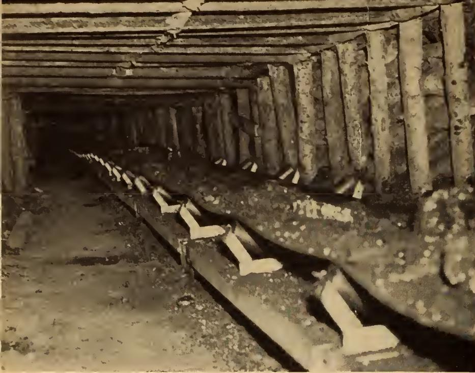
Fig. 8. View looking along main level showing belt conveyor.
