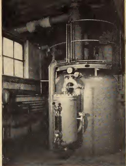
Fig. 5. Electric steam boiler of 2,000 kw., 8,000 volts, and 210 lb. per sq. in., equipped with automatic regulation of output, pressure and feed water and installed in a paper mill.
