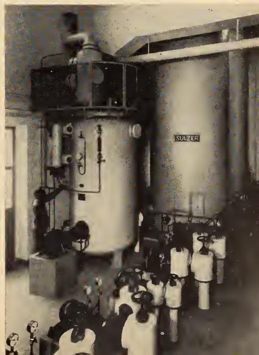
6. Combined electric-oil and electric-coal steam accumulators and steam boiler plants.
