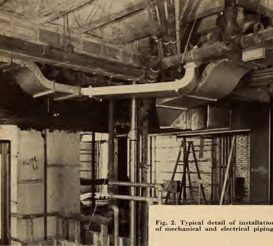
**Fig. 2. Typical detail of installation of mechanical and electrical piping.**
