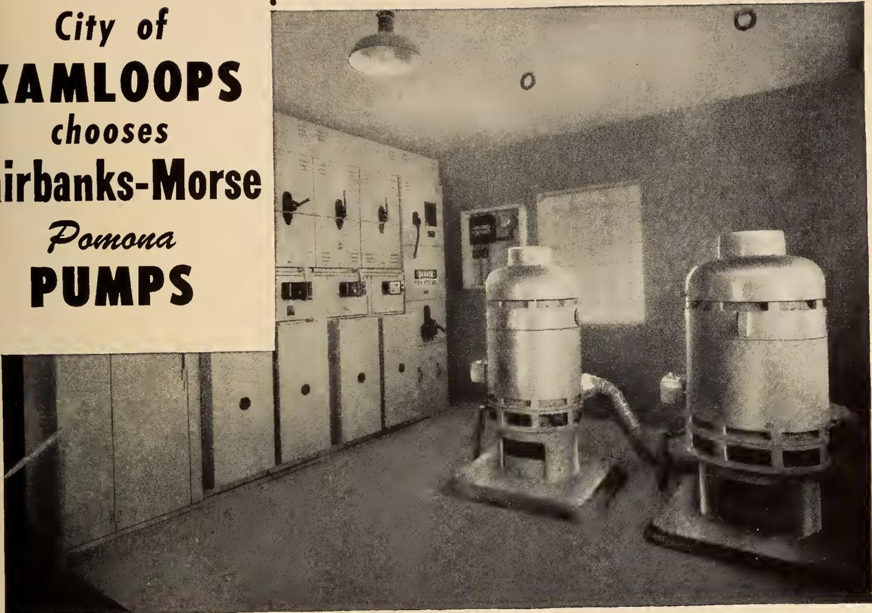
Motor floor, showing 150 HP motors and control panels for deep-well installation of two Pomona Turbine Pumps operated by the City of Kamloops, B.C.
