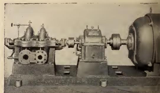
C A-C type "CM" mine pumping unit consisting of a 3" suction, 2½" discharge, 2-stage, double-suction, ball-bearing pump.
