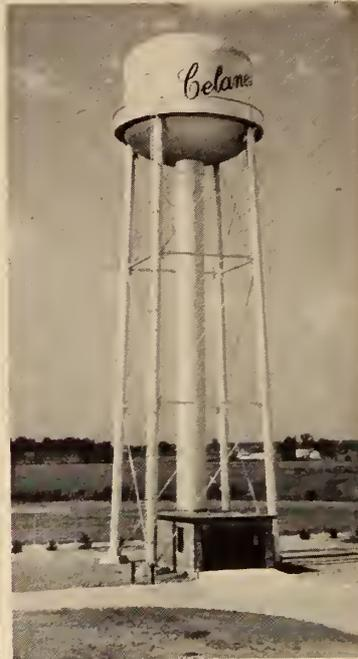
Horton elevated steel tanks are used to provide gravity water pressure for fire protection at industrial plants. The tank shown at the left is located at the Canadian Celanese Limited plant at Sorel, Quebec, and supplies water to the automatic sprinkler system throughout the plant. It has a capacity of 100,000 gallons and is 85 ft. to the bottom.
