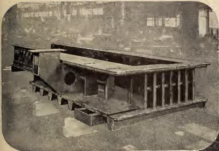
*Body for Dempster hydraulic baling press*
