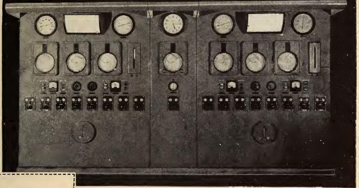
The master panel, centre, mounts the master steam pressure-recorder controller, the plant master selector valve, and all other equipment common to both boilers. The side panels mount recorders, gauges, meters, controls, push-button stations, etc., for the individual boilers.
