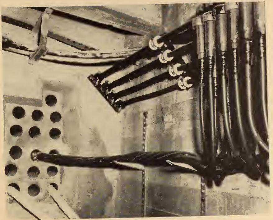
Fig. 7. Typical service manhole installation with secondary mains.
