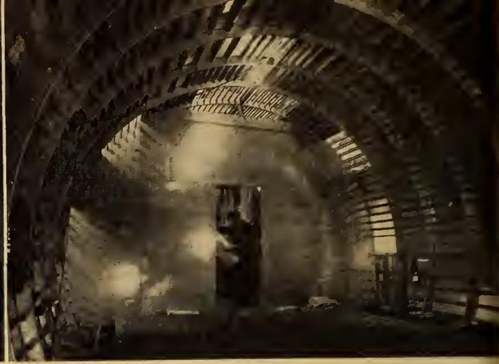
Fig. 2, above left. October 1946. Frames in way of the inner wing are complete and the inner wing spars are located in the jig. Note the tubular bracing of the interspar ribs and front spar.
