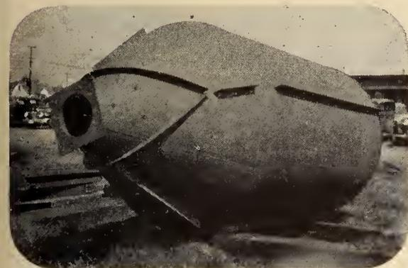
*Aggregate bin for concrete plant*
