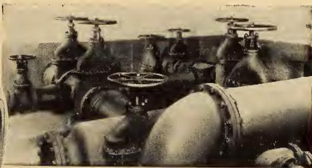
RAW WATER INLET lines in large sewage treatment plant featuring Crane low-pressure iron body double disc gate valves.
