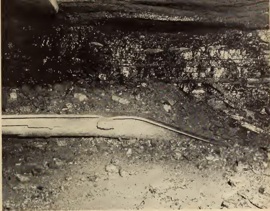
Fig. 2. Duckbill loading at face.
