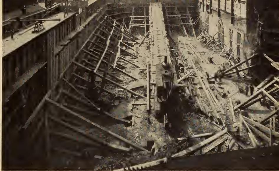
Fig. 2. Excavation, shoring, and underpinning for the foundations of the new building.
