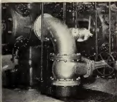
**WINE COMPRESSOR power house,** showing Crane iron double-disc gate valve, safety valve, and flanged fittings.
