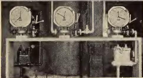
**IN PROCESS CONTROL:** For example, this meter measures liquid soap into washing process, saves soap and reduces rinsing time. Use meters also to check consumption rates.
