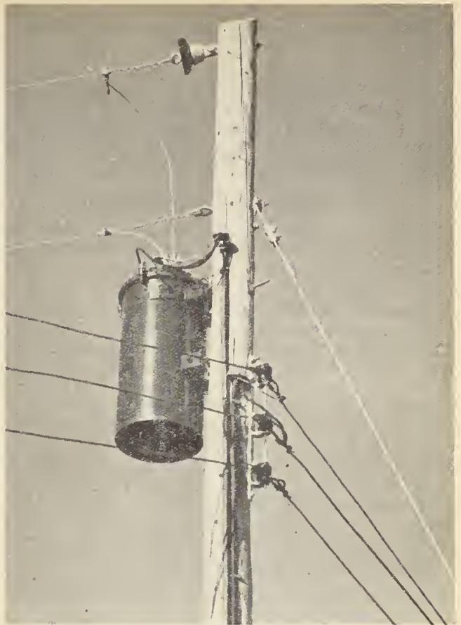
3 kva. transformer installation—6900V farm lines.
