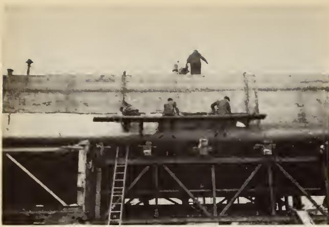
Fig. 6—The bottom of this heavily scaled barge was flame-primed and painted up to the water line, then returned to the river and completed by operators working on a small raft that held all the equipment needed.
