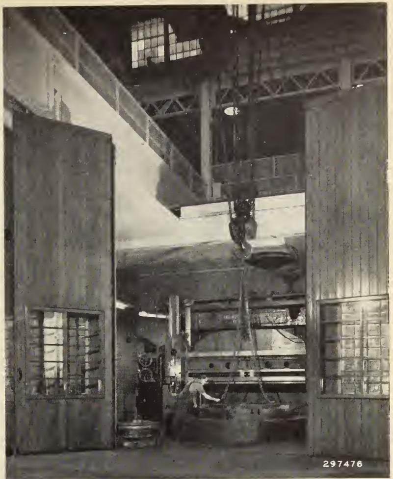
**Internal view of the air conditioned room in which thrust bearing runners are machined and finished.**
