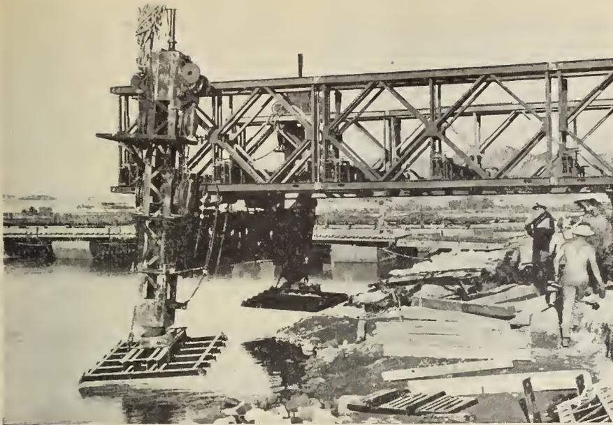
Fig. 7—Launching has begun with one trestle suspended from the end of the bridge, and rolling forward is under way.
