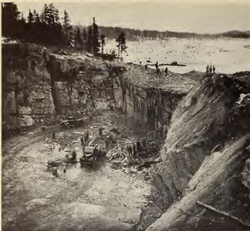
Fig. 7—The Marmion lake “plug” just before blasting.
