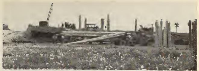
Unloading 50 ft. and 60 ft. timber piles—note transporter built specially for this task.
