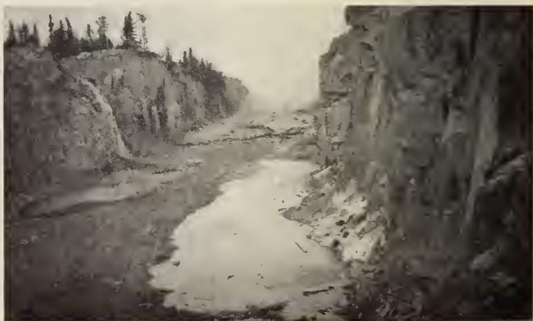
Fig. 8—Raft lake east cut; wedge-shaped wave approaching the Raft lake spillway after blasting the Marmion lake “plug”.
