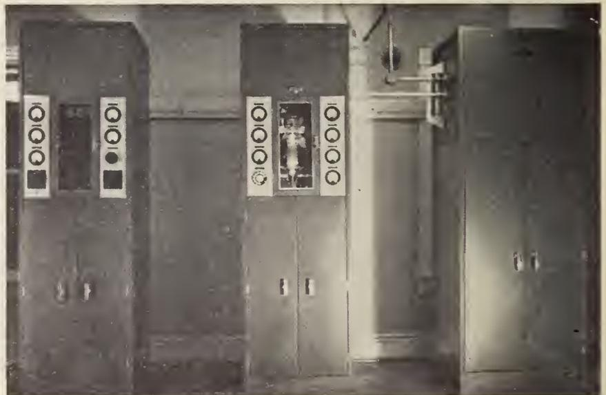
Fig. 1—Northern Electric Model 14C, 10 channel, crystal controlled transmitter used at majority of Trans-Canada Air Lines ground stations.
