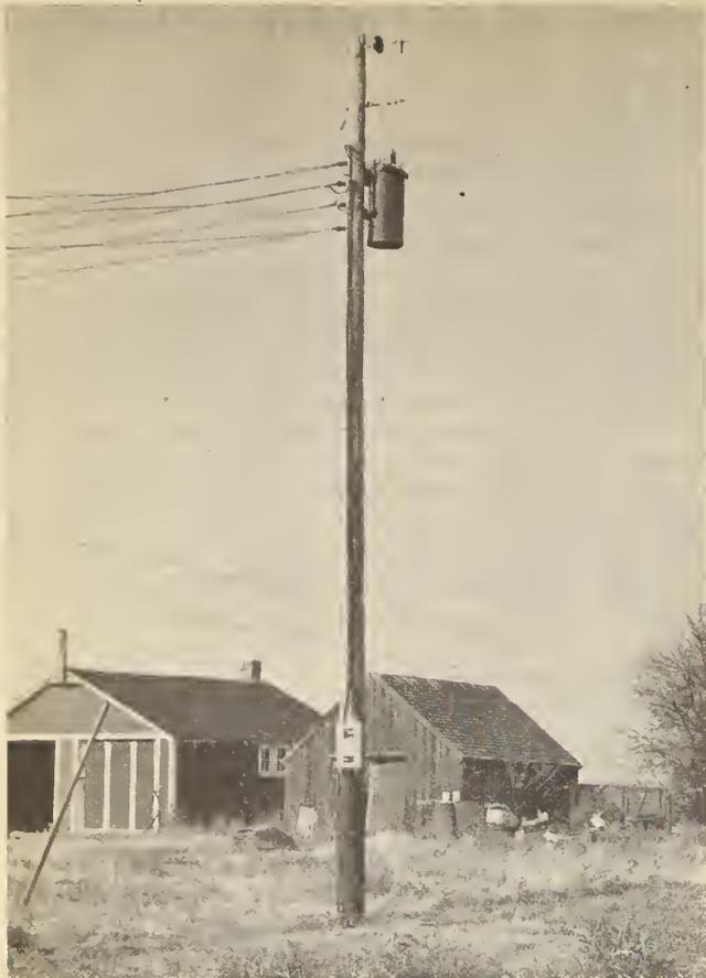
**Transformer pole showing transformer and meter box—6900V farm lines.**
