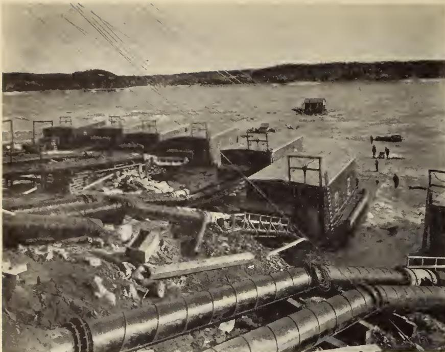
**Pumping installation, showing connection to shore and flexible couplings. Lake down 15 ft. when picture taken; now down 135 ft.**
