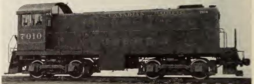
1,000 hp. Alco-G.E. Diesel-electric switching locomotive, 115 tons weight on drivers, 69,000 lbs. starting tractive effort.
