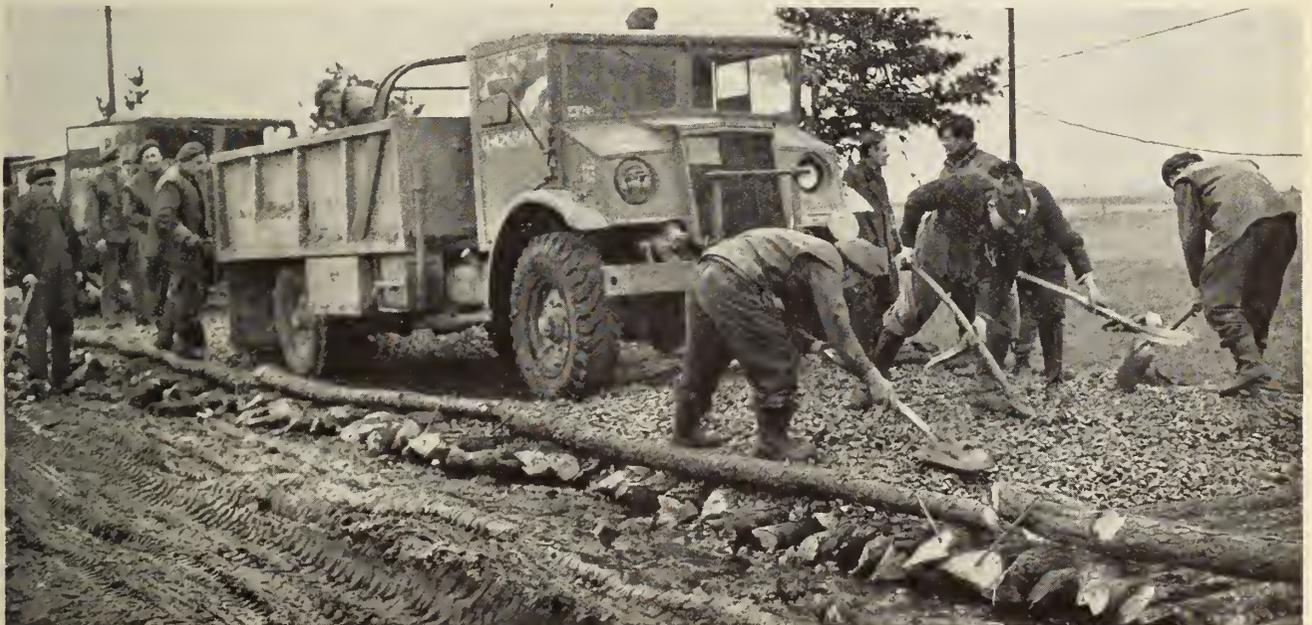
Canadian engineers, aided by Dutch civilians, spread stone on a damaged road bed—Part of reconstructural road work made necessary by heavy traffic preceding the renewed Allied offensive on the Western front.
