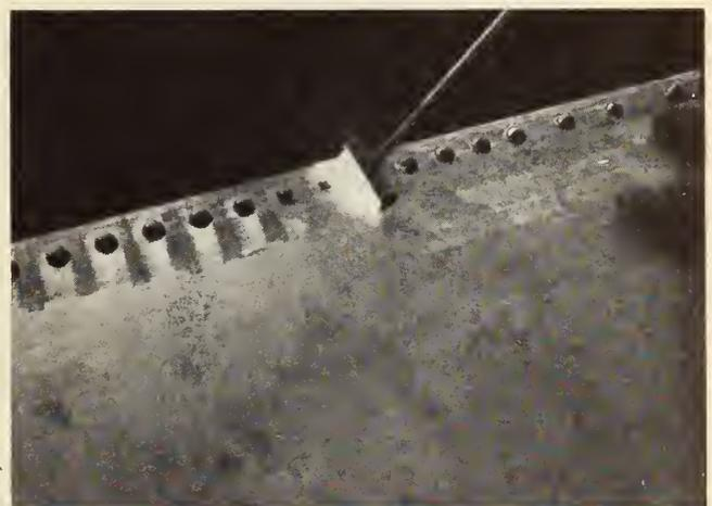
Fig. 3—Flame-priming the box girders used in the Rainbow Bridge at Niagara Falls.
