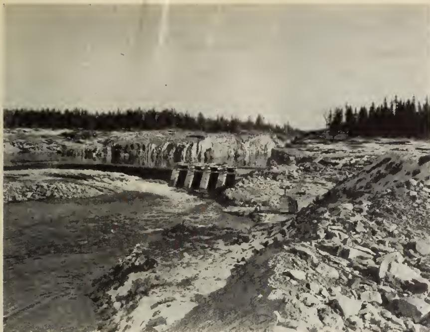
Fig. 9—Raft lake control works and spillway.
