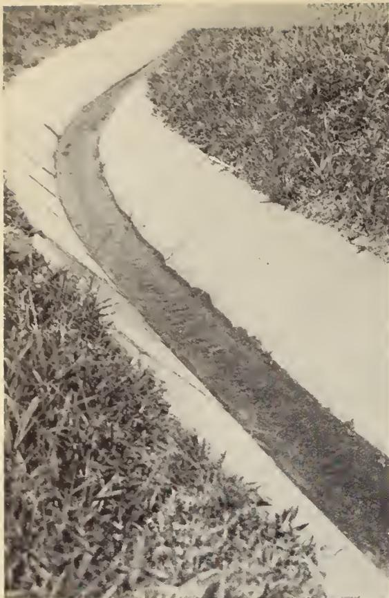
Fig. 3—Photograph of drain paved with concrete slabs.
