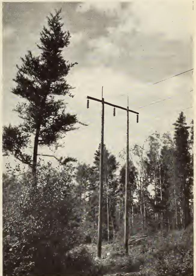
Fig. 3—Typical suspension structure—Steep Rock Line.
