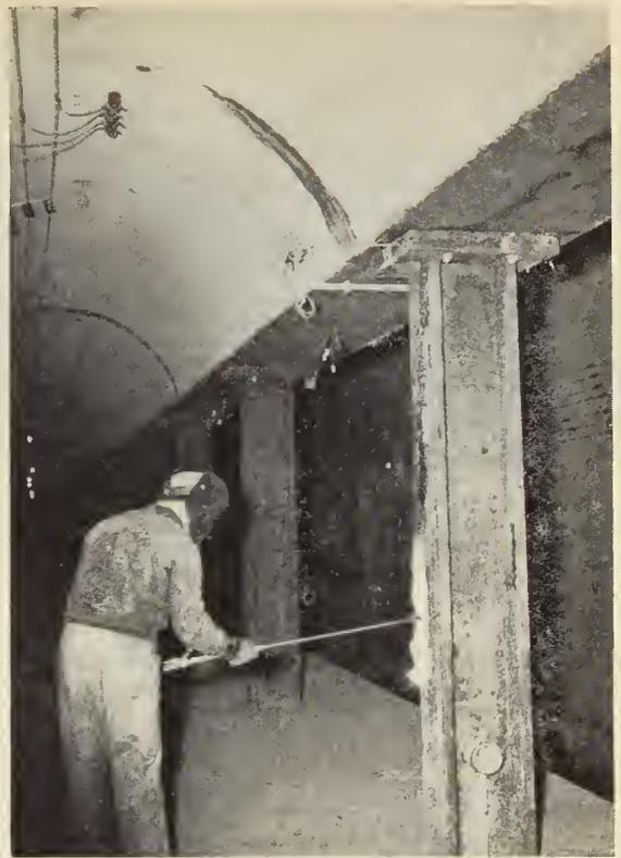
**Fig. 5—Flame-priming is practically indispensable for preparing structural steel members in subways where they must be painted after erection in a damp atmosphere. This is a view of operations during construction of the new Chicago subway.**
