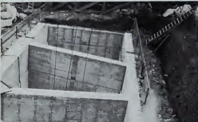
Fig. 10—South anchor-pier: completed walls of heel-block.
