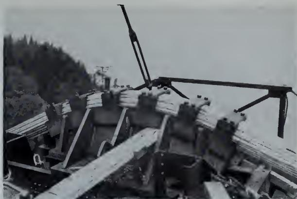
Fig. 60—Completed main saddle.
