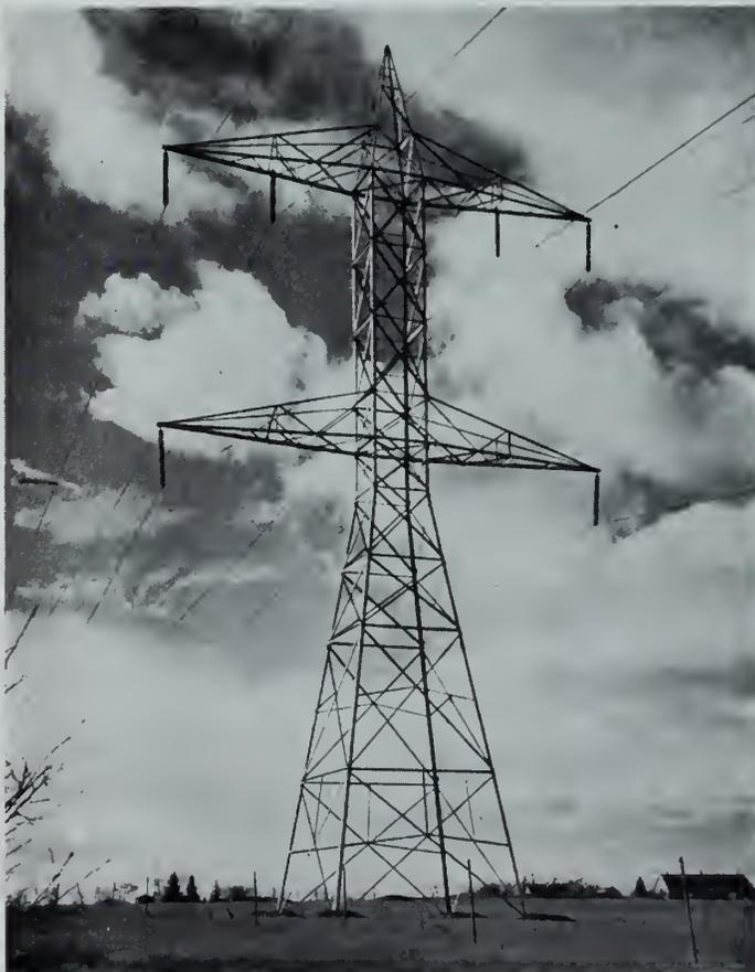
Fig. 1—Transposition tower for double circuit 220 kv. line.
