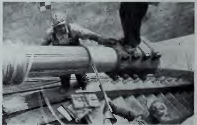
Fig. 61—Splay-casting: hand-wrapping of cable.
