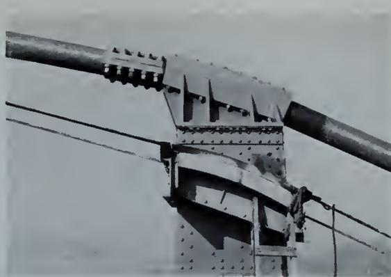
Fig. 65—Cable-saddle and keeper at cable-bend.
