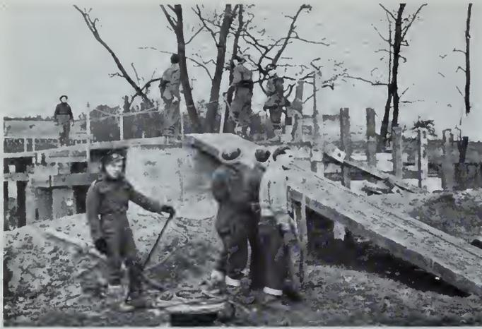
Fig. 8—Preparing to launch bridge girders.
