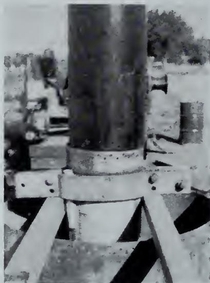
Fig. 3—Setting a 16-in. shutter screen in the 42-in. outer casing of a Layne gravel wall well.
