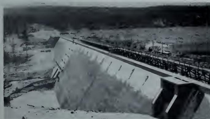
Fig. 8—Dam, looking south from mixing plant, showing conveyor trestle and diversion sluices.
