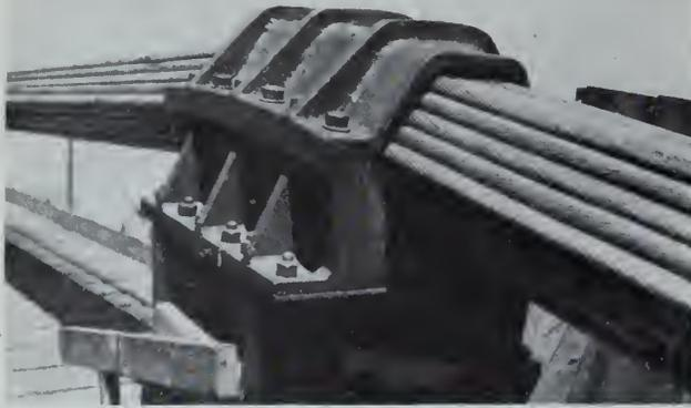
Fig. 66—Saddle at south cable-post.
