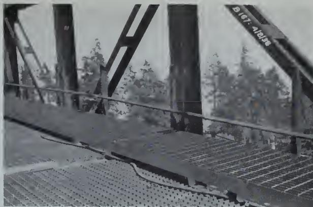
Fig. 24—Grid deck before concreting.
