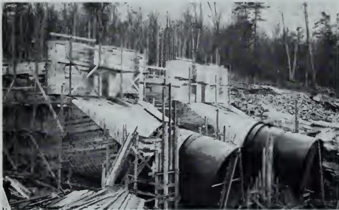
Fig. 5—Headworks gatehouse substructure and penstocks.
