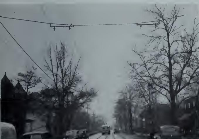
Fig. 5—Feeder span using copper feed span to support trolley wire.
