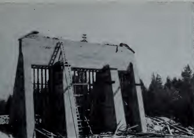
Fig. 19—Open abutment at north end of viaduct.
