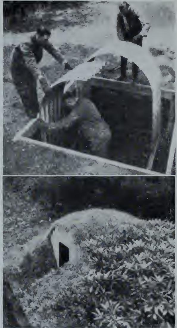
Fig. 8—Photographs showing method of erection of Anderson shelter and final appearance.
