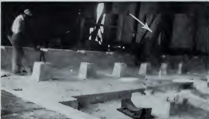
Fig. 2—Boiler foundation. Note the temporary supports for the centre building columns in the background.
