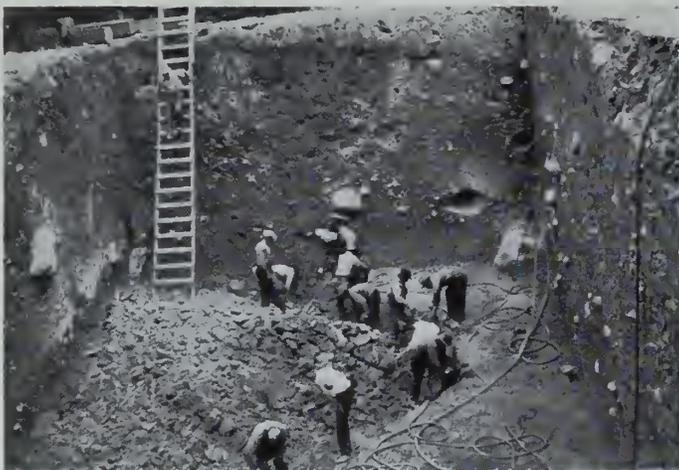
Fig. 9—South anchor-pier: excavation in stiff clay.
