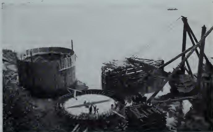
Fig. 5—South main pier: caisson-construction on shore.
