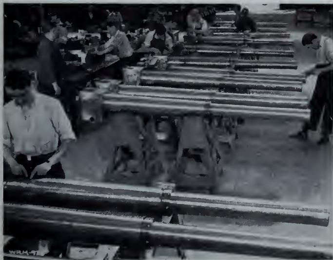
Fig. 5—Fitting breech mechanisms to gun barrels.
