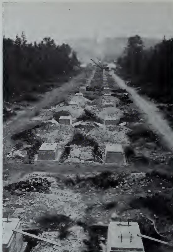
Fig. 18—Pedestals for north viaduct.
