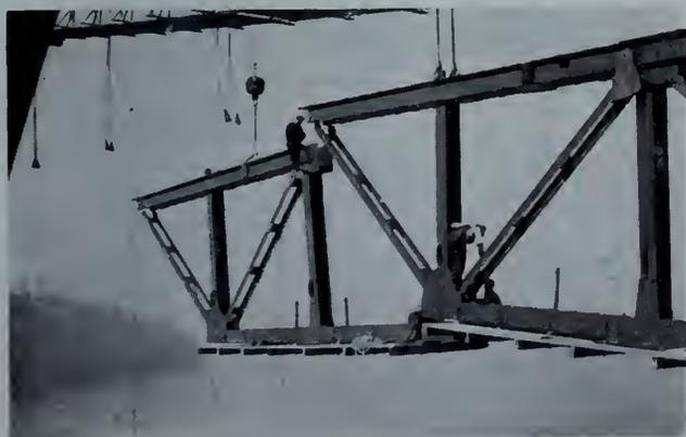
Fig. 64—Erection of truss-section, north side-span.
