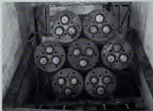
Fig. 47—Anchorage: Button-assembly.
