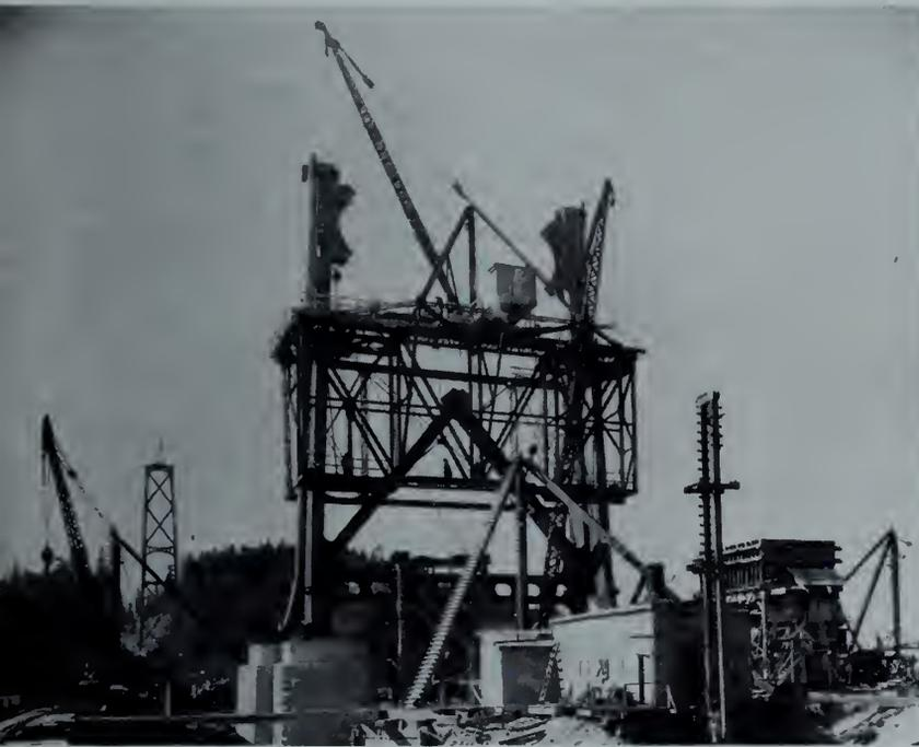
Fig. 57—Creeper-traveller erecting north tower.
