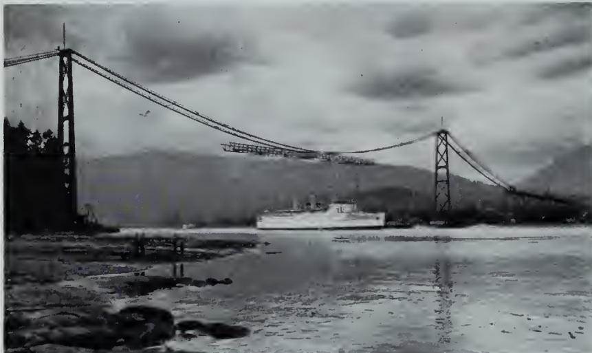
Fig. 63—Trusses partly erected, central span.
