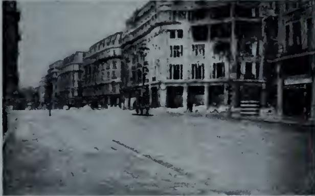
Fig. 13—Photograph of completely framed buildings still standing after severe bombing.
