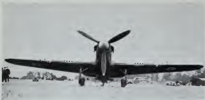
Fig. 2—The *Hurricane* II armed with twelve machine guns.
