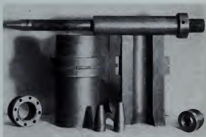
Fig. 14—Tools for 4-inch naval shell forging.
