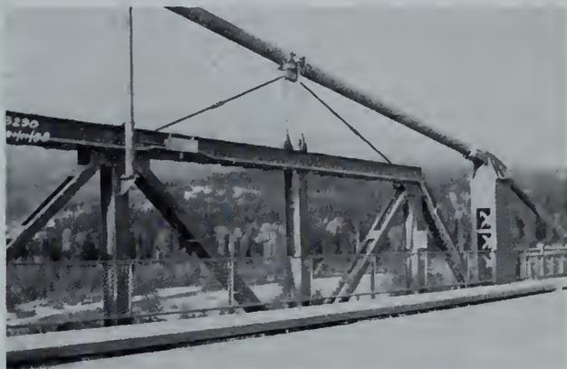
Fig. 68—Traction-rods at north end.
