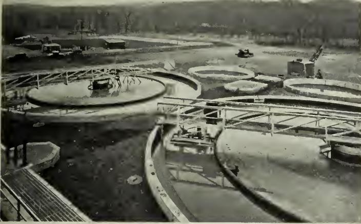
Fig. 1—Circular Sedimentation Tanks Equipped With Up-flow Magnetite Filters.
