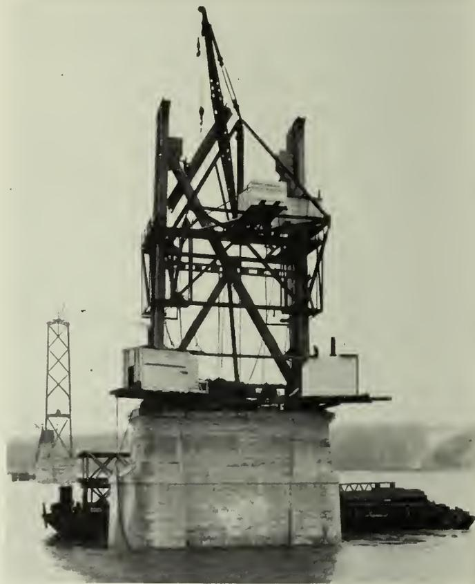
Fig. 5—Creeper Traveller Erecting Tower.
