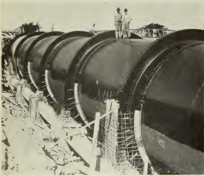
Fig. 24—Downstream Section of Steel Pipe Line. Note concrete struts and copper expansion joint strips.
