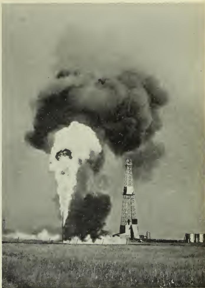
**Brown No. 2 well coming into production. The mud fluid used in drilling, saturated with oil when the productive limestone was encountered, is being blown out and burnt at the end of a 6 inch flare line.**
