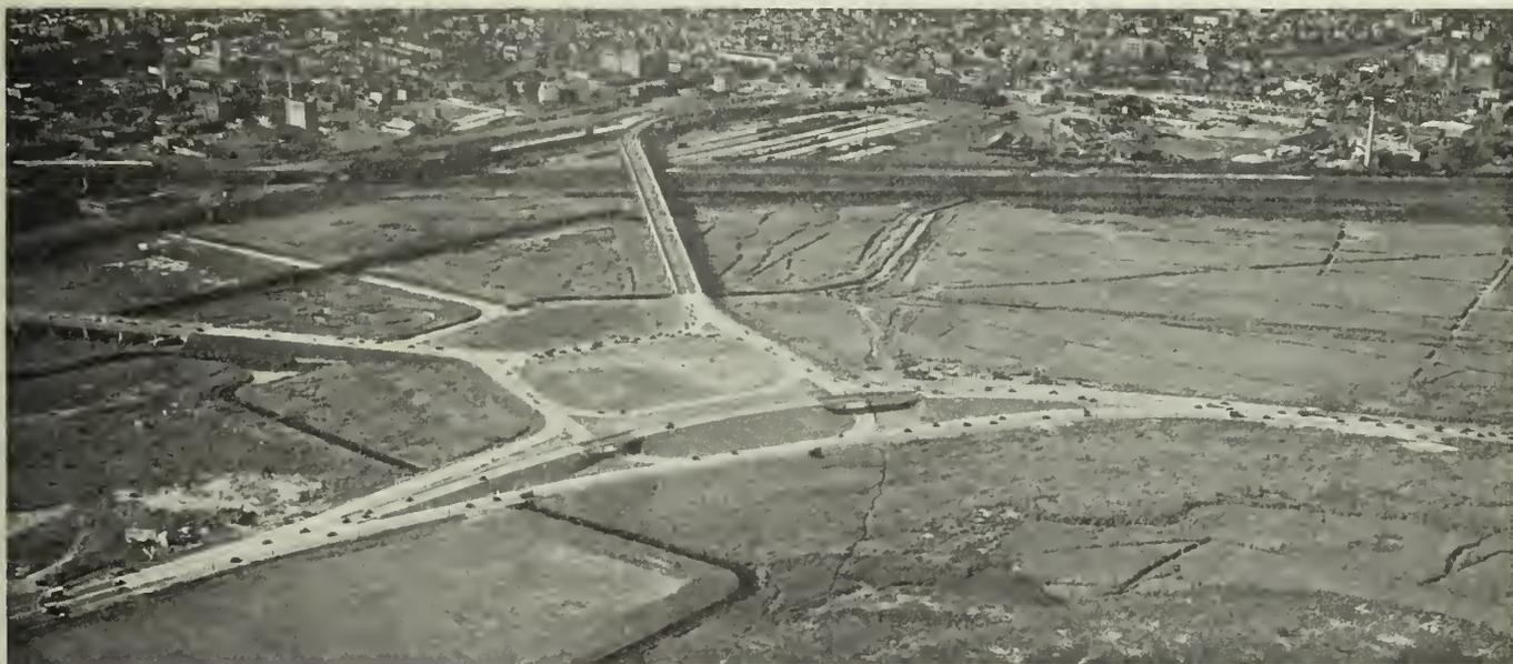
Fig. 2—Newark Junction, Essex County, N.J. State Routes No. 21, 25 and 29. Showing rotary traffic circle in connection with two grade separations.
