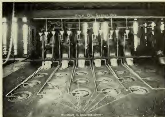
Fig. 5—Equipment for Oiling Oven Charges, Vancouver Plant.
