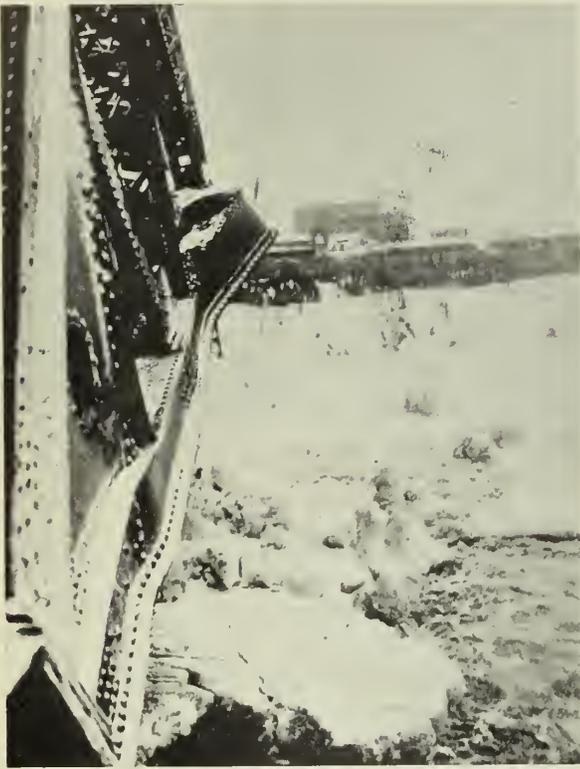
Fig. 8—Jan. 27th, a.m., Kink in Downstream Bottom Chord.
