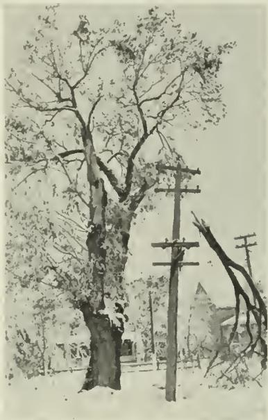
Fig. 3—Limb of tree broken off by snow and wind, short-circuiting overhead conductors.
