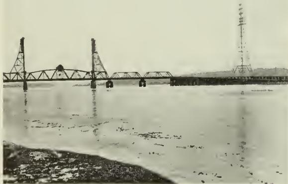
Fig. 6—Second Narrows Bridge, Vancouver, B.C., Carrying Gas Mains.
