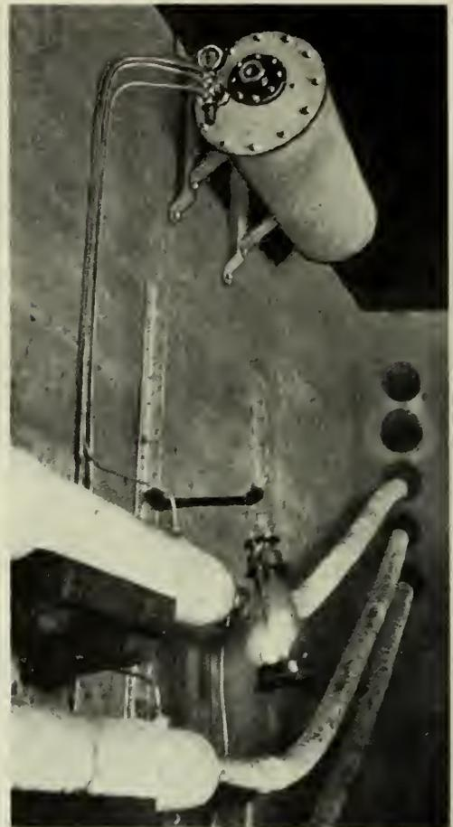
Fig. 6—Standard Underground Pressure Reservoir in Manhole.
