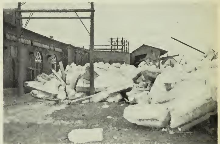
Fig. 2—Ice piled up on dam in front of power house.
