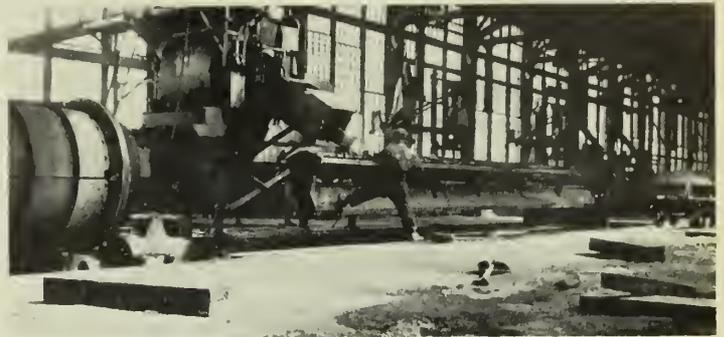
Fig. 17—Concrete Mixing, Loading and Spinning Equipment.
