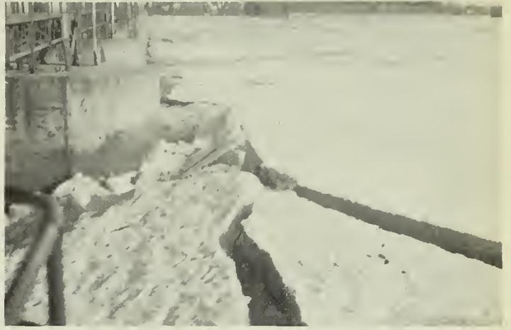
Figs. 5 and 6—Ice going through sluice gates.
