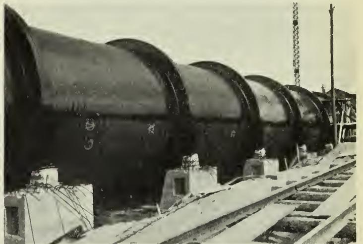
Fig. 5—Upstream Section of Steel Pipe Line Before Completion of Girder Wells.
