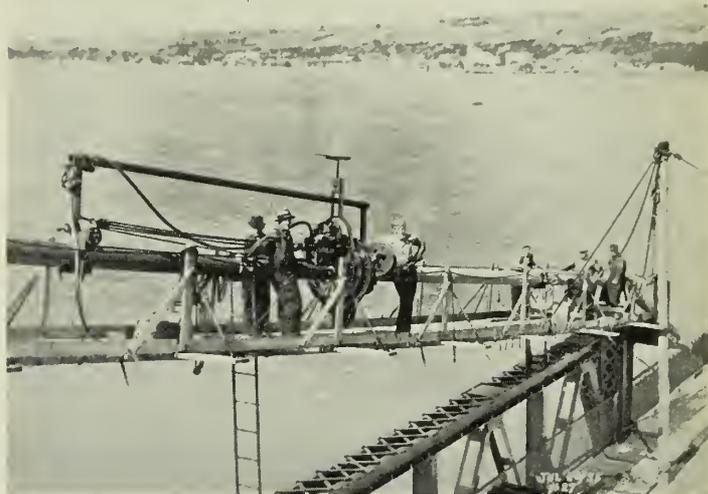
Fig. 8—Wrapping the Cable.
