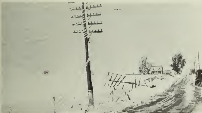
Fig. 9—Overhead telephone lines brought down by sleet.
