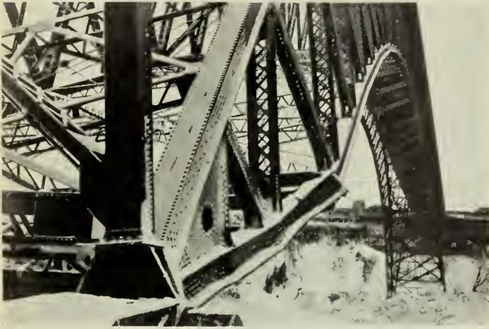
Fig. 4—Jan. 27th, 2.40 p.m., Showing Kink in Downstream Lower Chord.
