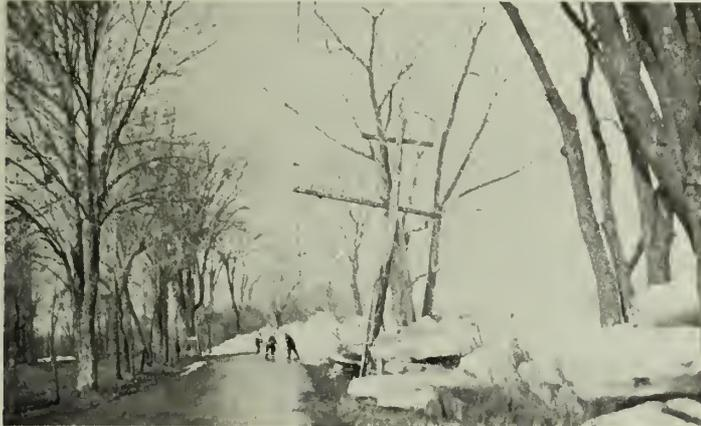
Fig. 1—Ice piled up on road breaking pole.
