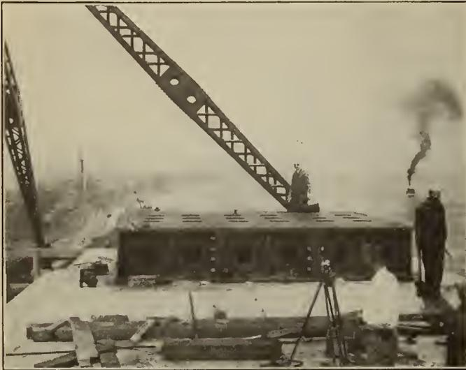
Figure No. 43.—Main Span, North Side—Setting Main Shoe Castings on Main Pier.
