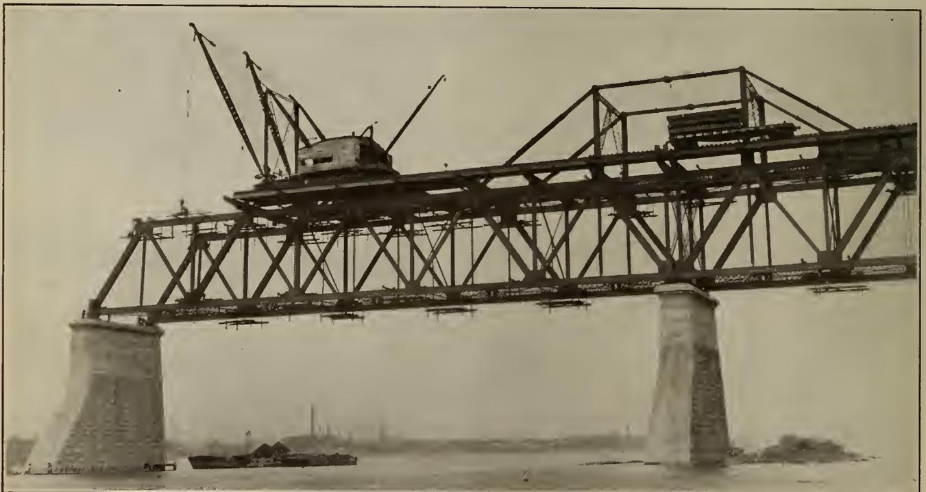
Figure No. 18.—South Approach—Cantilever Erection of 245-foot Spans—Fifth Stage.
