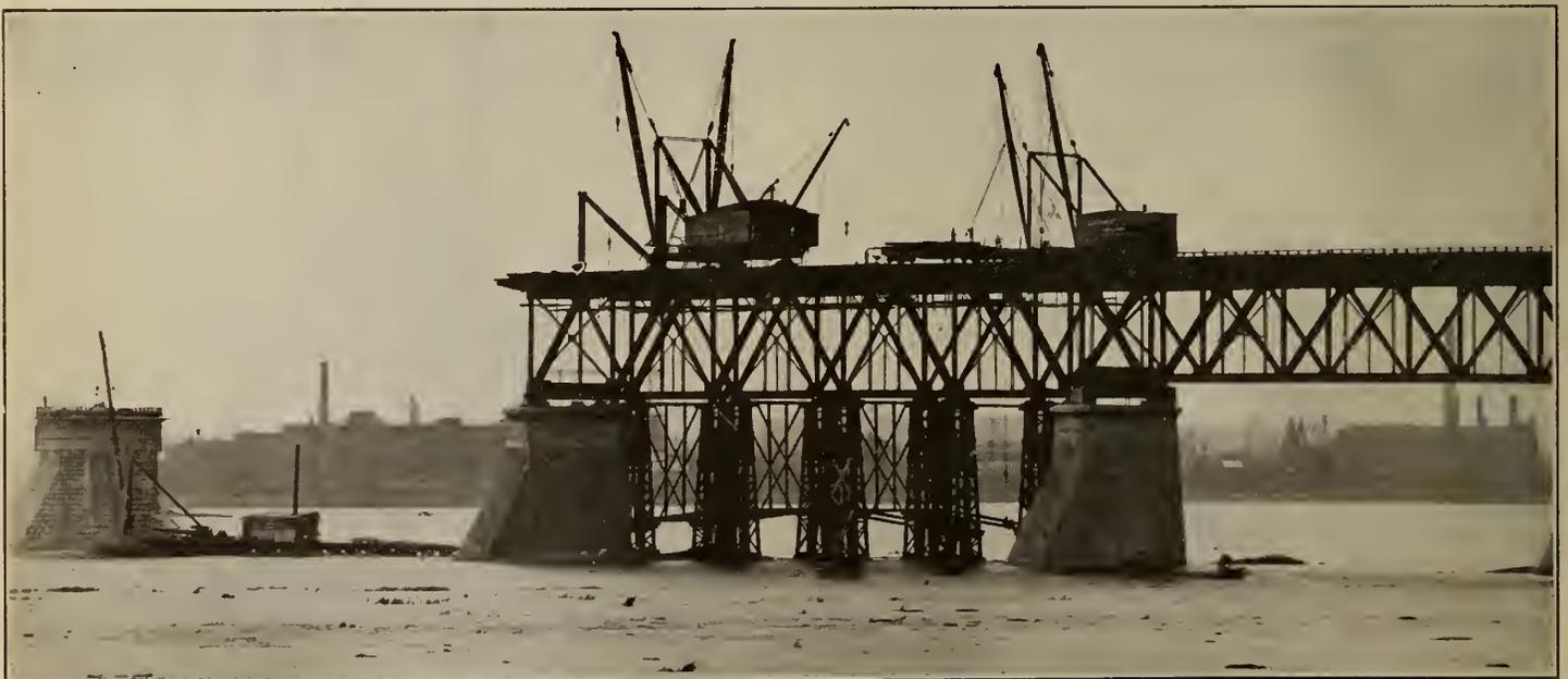
Figure No. 10.—South Approach—Timber Falsework under Span No. 10 (245-foot).
