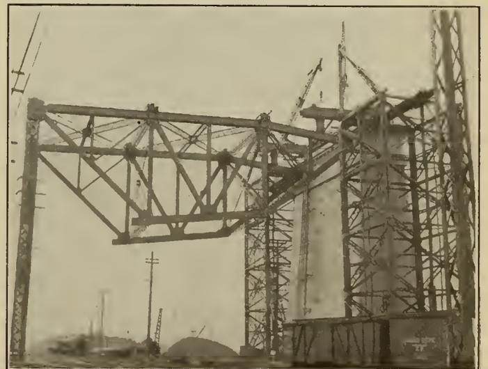
Figure No. 49.—Main Span, North Side—Placing Bottom Chord Sections of Anchor Arm—First Stage.
