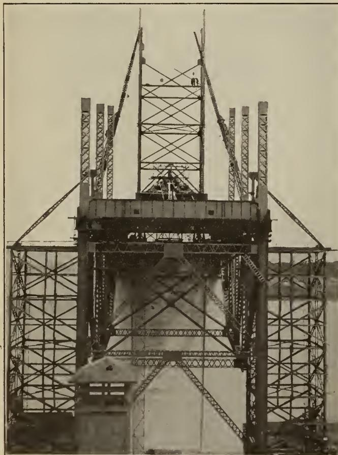
Figure No. 51.—Main Span, North Side—Erection of Traveller No. 4 on Anchor Arm—First Stage.
