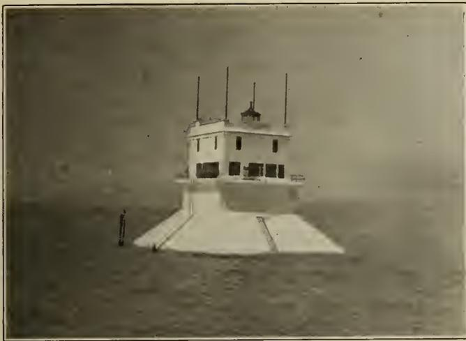
Figure No. 12.—Combined Lighthouse, Fog Alarm and Radio Beacon Station erected on South East Shoal, Lake Erie, by the Canadian Government.
