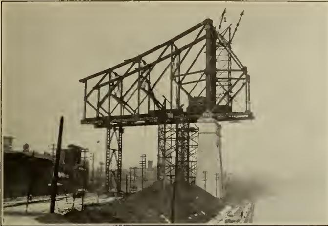
Figure No. 57.—Main Span, North Side—Erection commenced on Cantilever Arm. Progress as at December 14th, 1927.
