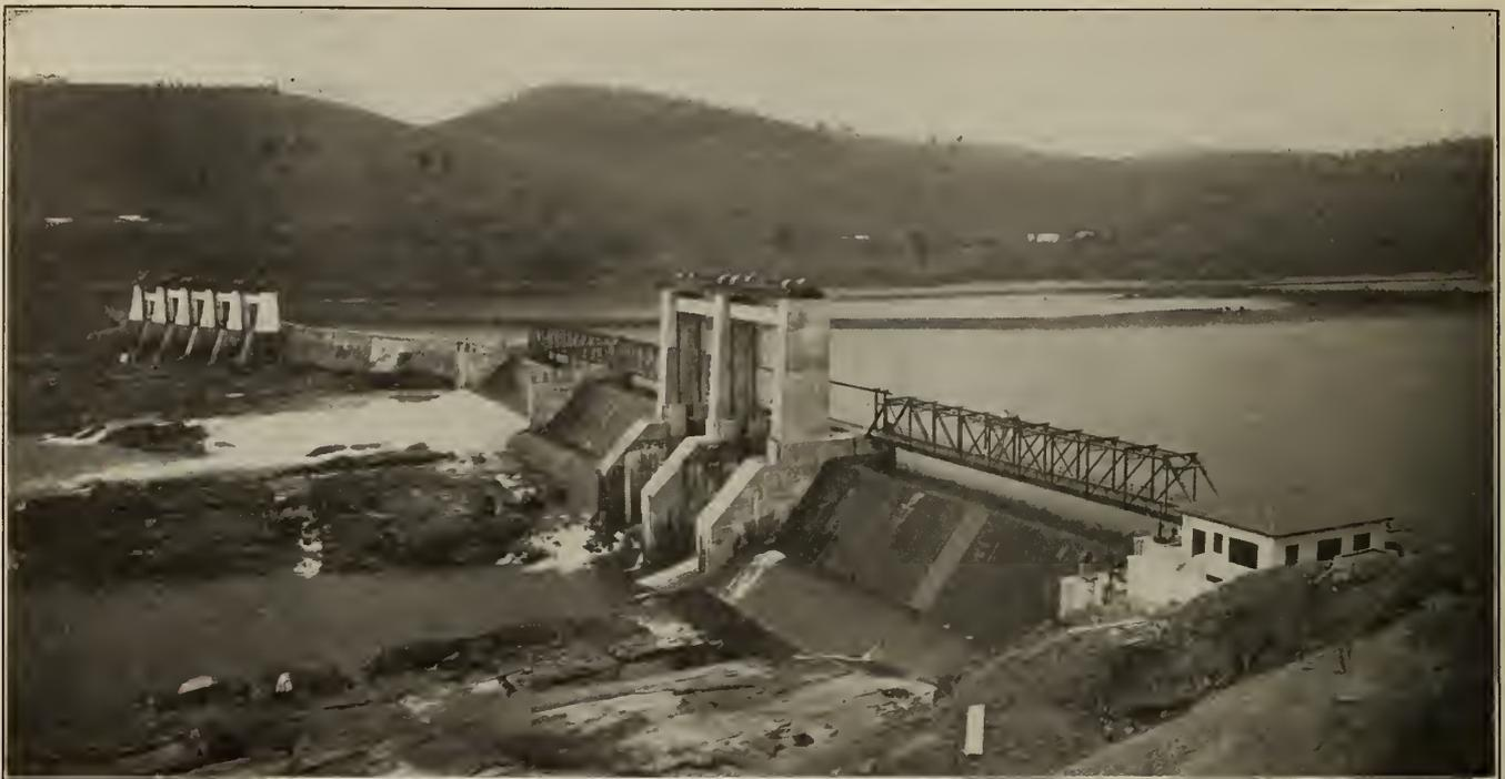
Figure No. 4.—Ilha dos Pombos Development supplying Rio. North Channel Dam looking North—South Sector No. 3 discharging Two Thousand Cubic Feet per Second
