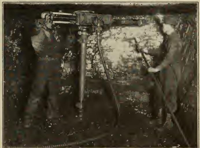
Figure No. 7.—Overcutting with a Radialaxe Type Coal Cutter.
