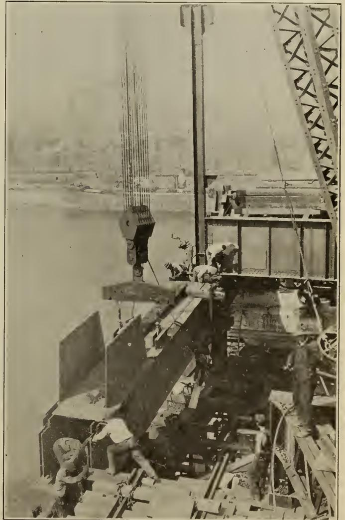
Figure No. 76.—Main Span, South Side—Placing Second Bottom Chord Section of Anchor Arm.
