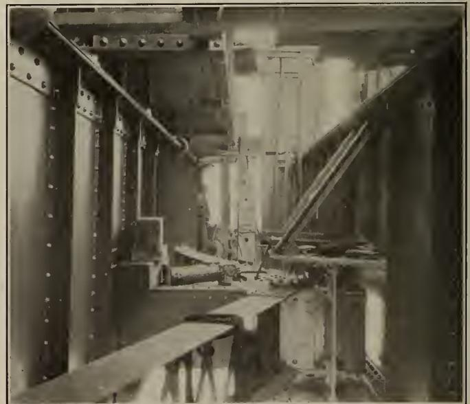
Figure No. 90.—Main Span, Centre Section—Arrangement of Floorbeams and Lateral System Connection at North End of Suspended Span.
