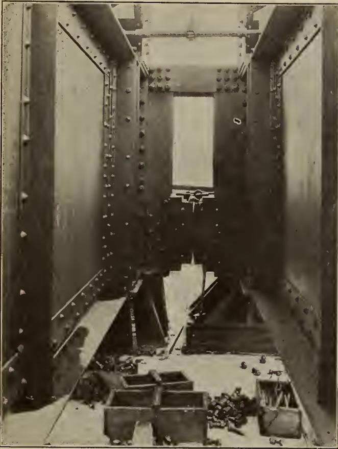
Figure No. 13.—South Approach—Cantilever Erection of 245-foot Span—Special Shoe Details.
