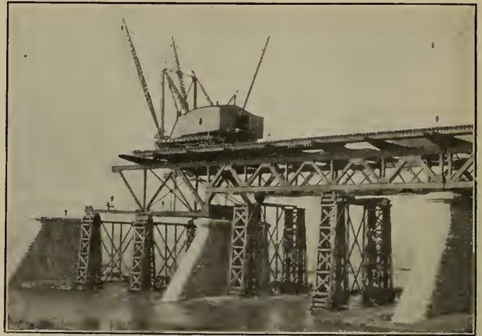
Figure No. 9.—South Approach—Timber Falsework under Short Spans.
