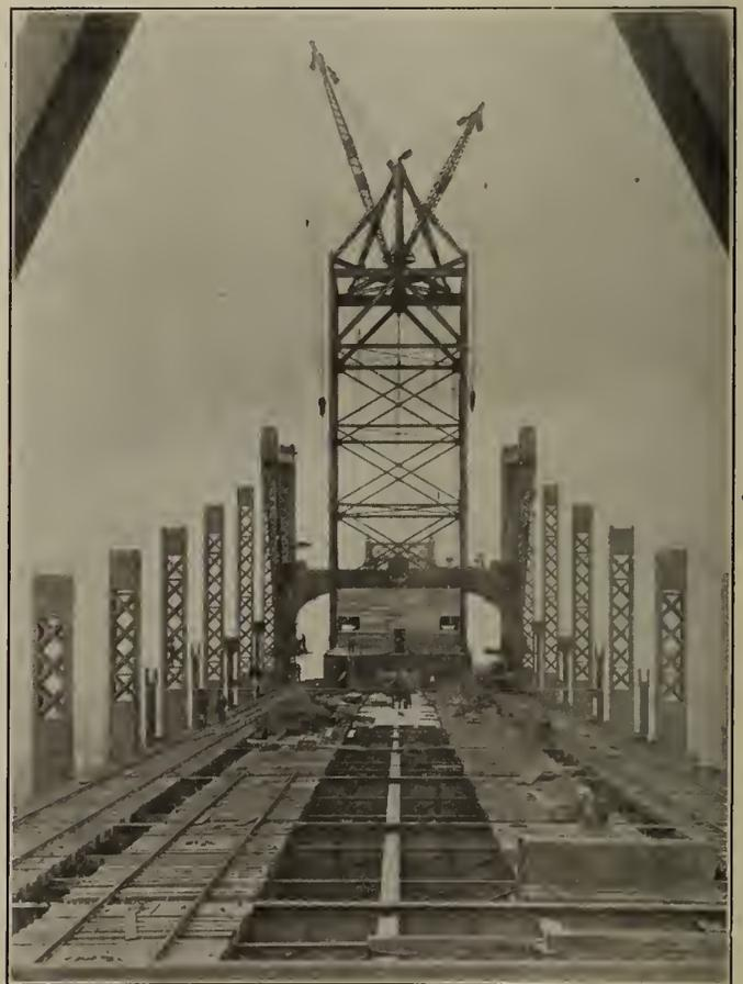
Figure No. 78.—Main Span, South Side—Rear View of Traveller No. 4 and of Deck. Erection proceeding on Anchor Arm.
