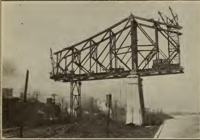
Figure No. 61.—Main Span, North Side—Erection proceeding concurrently on Anchor and Cantilever Arms.
