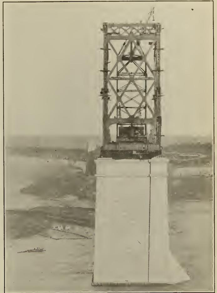
Figure No. 79.—Main Span, South Side—Front View of Main Posts and Bracing, and of Traveller No. 4.
