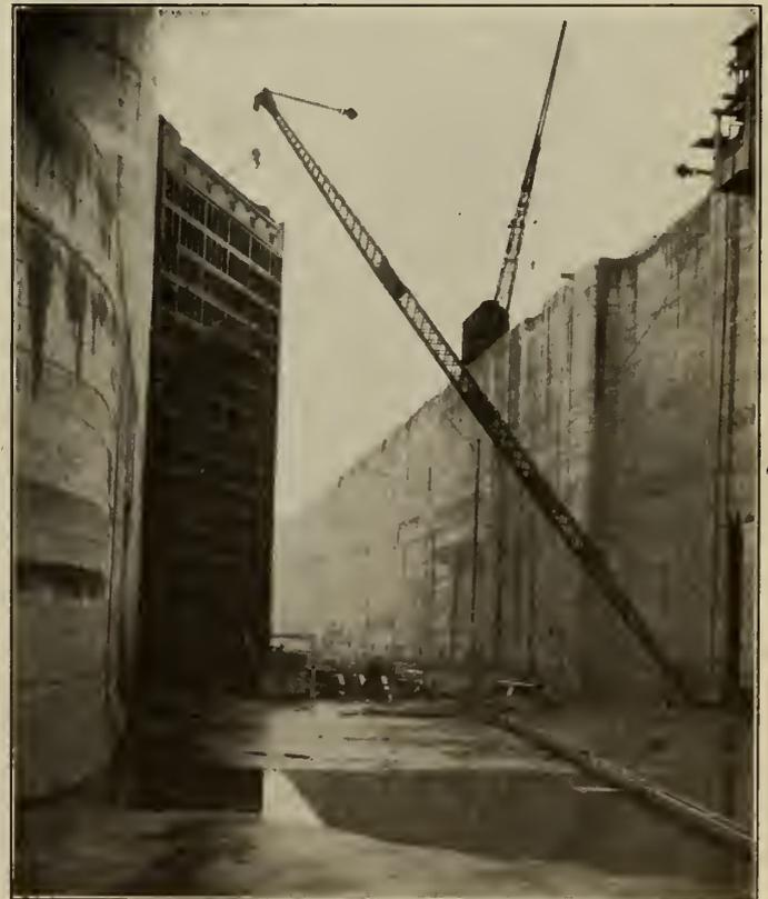
Figure No. 3.—130-foot Boom and 30-ton Crane at Lock No. 2.
