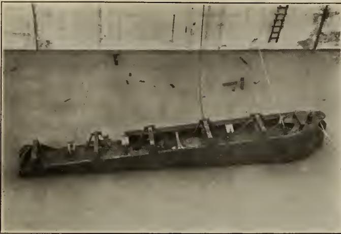
Figure No. 8.—35-foot 6-inch Leaf with Mitre End Rising as Air is Pumped In.
