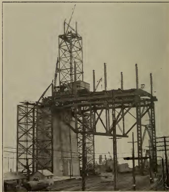
Figure No. 52.—Main Span, North Side—Erection of Traveller No. 4 on Anchor Arm—Second Stage.
