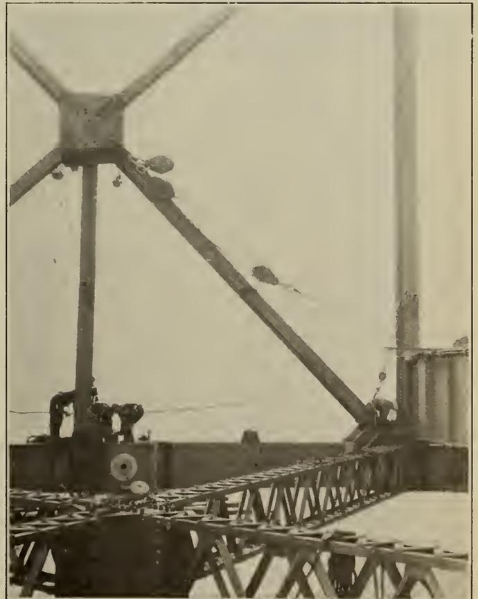
Figure No. 98.—Main Span, Centre Section—Arrangement of Adjustable Tackles in Centre Panel of Suspended Span.
