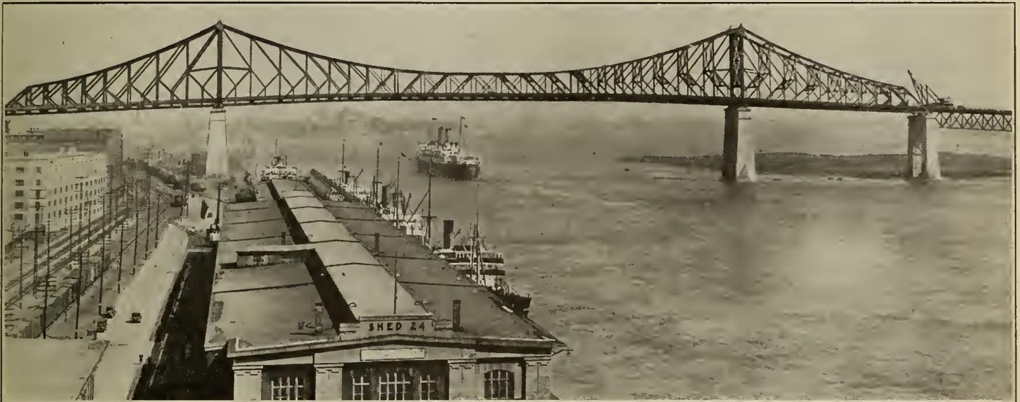
Figure No. 102.—The Main Span as at September 11th, 1929—Erection completed, Falsework Span removed and Last Equipment being dismantled.
