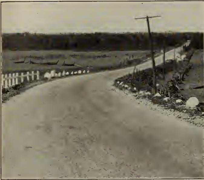
Figure No. 3.—Fenelon Falls—Lindsay Road (1929) Asphalt Mixed Macadam 6 inches Thick, 18 feet Wide.
