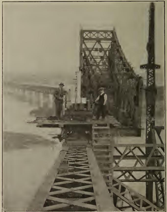
Figure No. 94.—Main Span, Centre Section—Rear View of Wedge Mechanism in Place at *CU0*.
