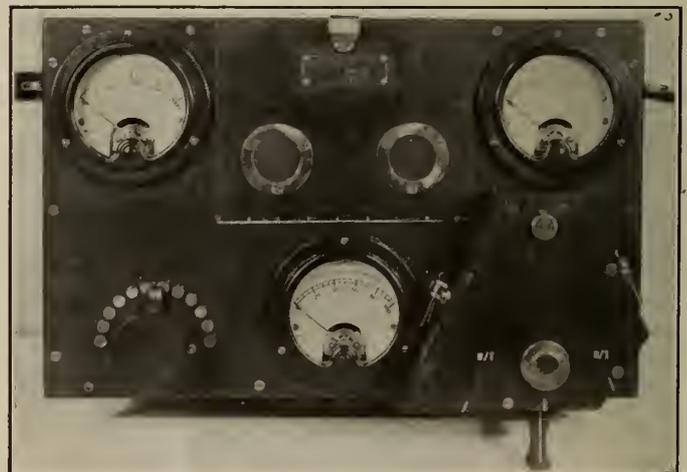
Figure No. 9.—View of Meter and Switch Panel, Aircraft Transmitter, Type CT21, developed by The Royal Canadian Signals for the Air Force.
