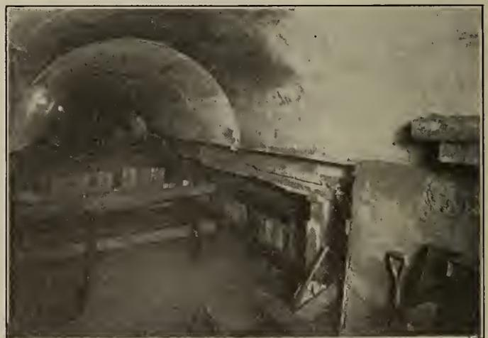
Figure No. 4.—Balliol Street Sewer showing "Flying Arch" Method of Construction.
