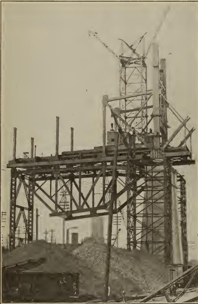
Figure No. 55.—Main Span, North Side—Erection proceeding on Main Posts and Adjacent Structure.
