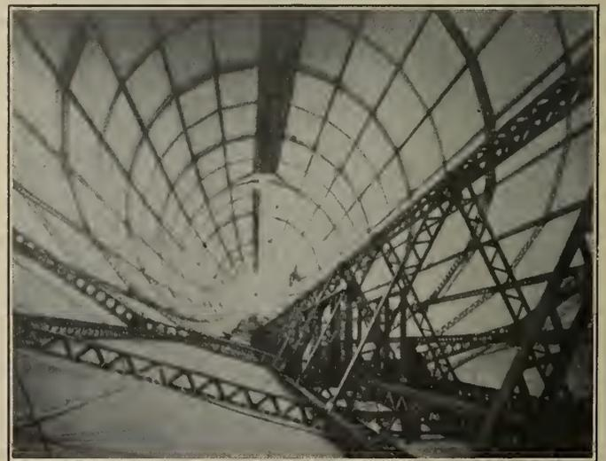
Figure No. 14.—Interior View "Schütte-Lanz Airship."
