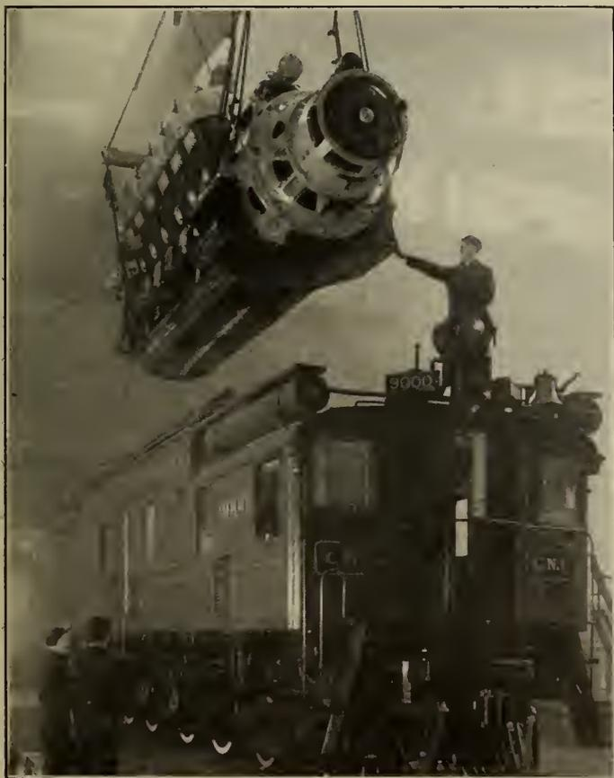
Figure No. 4.—Installation of 50,000-pound Engine in the New Oil-Electric Locomotive.
