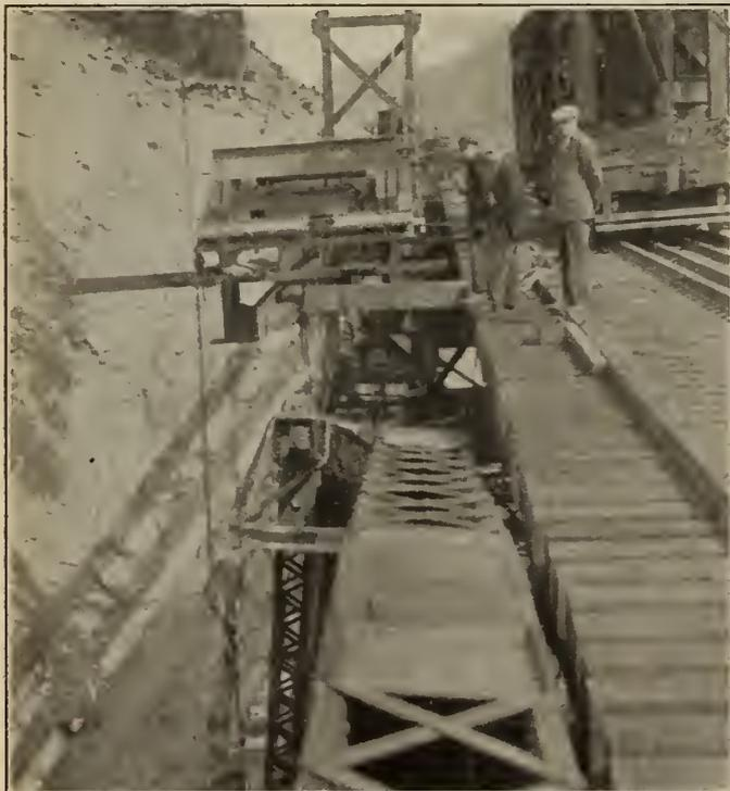
Figure No. 6.—Erecting Outer Arch by means of Cantilever Falsework without Loading Old Bridge.
