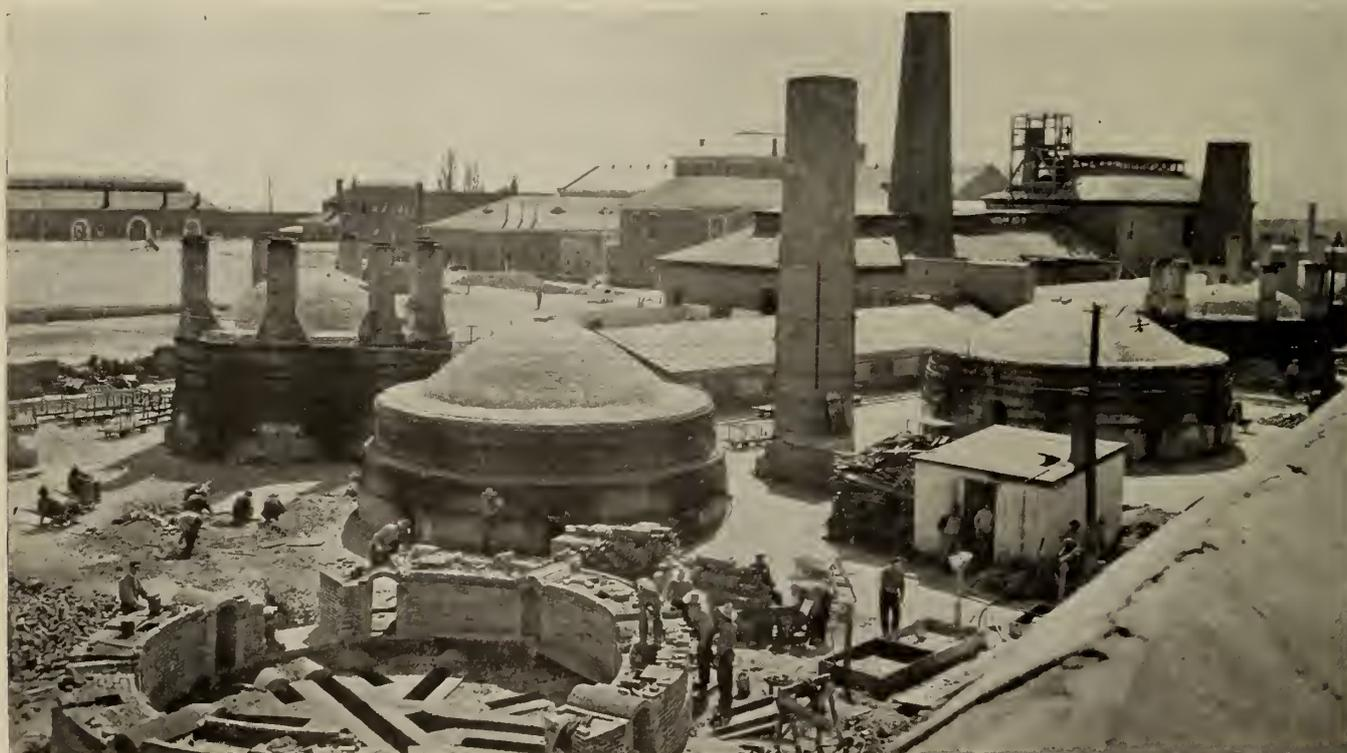
Figure No. 4.—Round Kilns of Multi-stack and Single-stack type.
