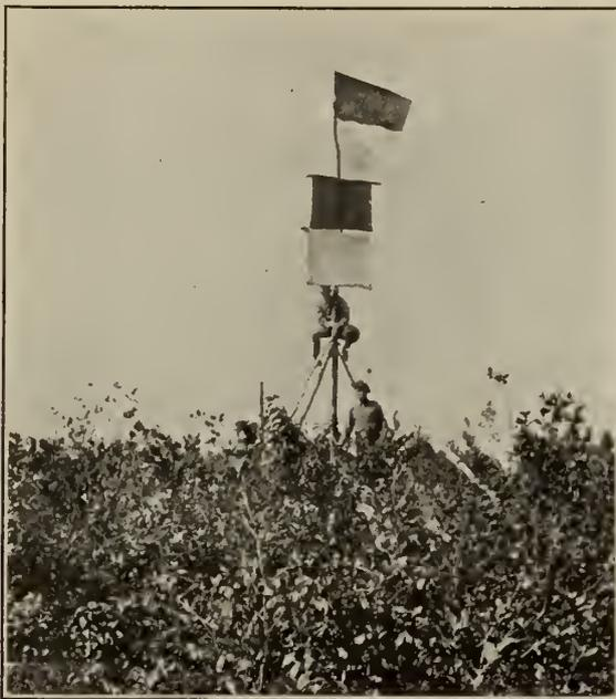
Figure No. 11.—Triangulation Control for One-Mile Mapping.
