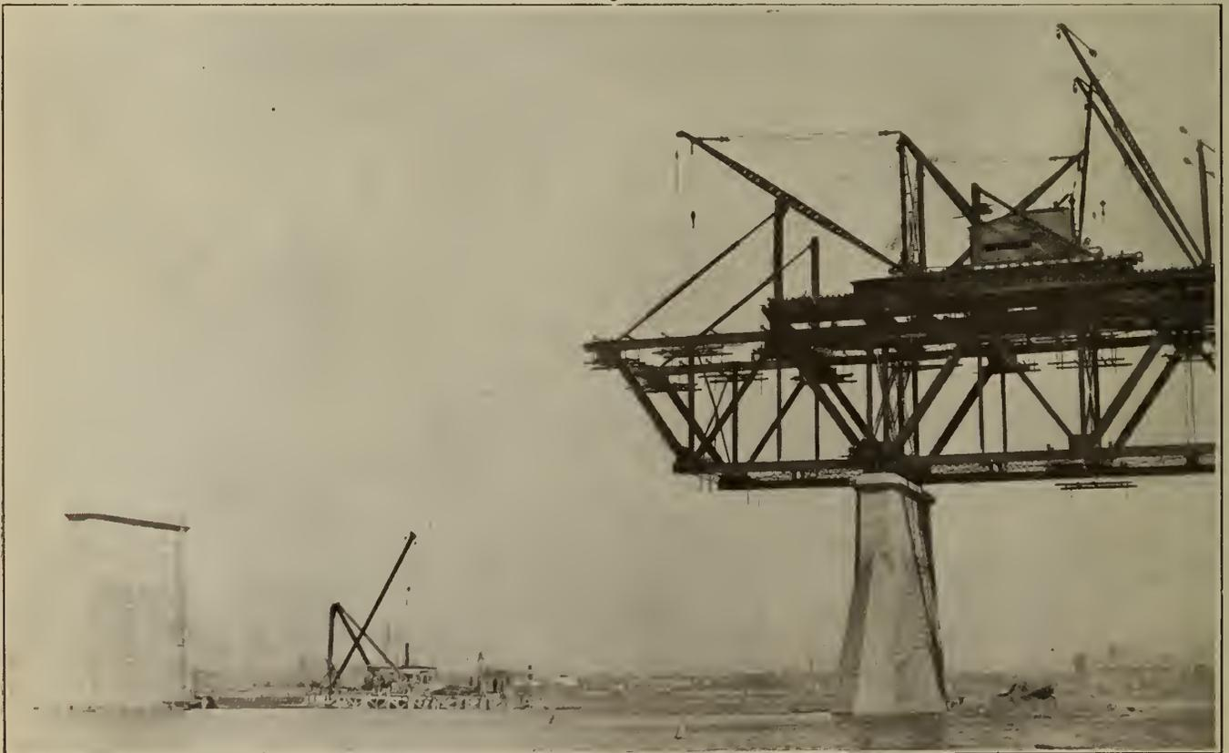
Figure No. 14.—South Approach—Cantilever Erection of 245-foot Spans—Second Stage.
