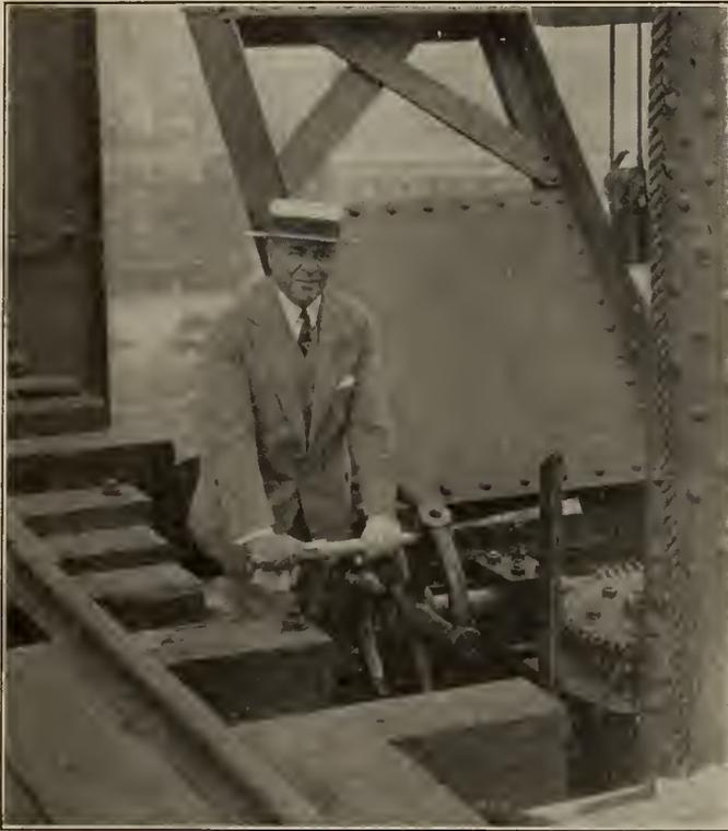
Figure No. 101.—Main Span, Centre Section—Hon. Dr. W. L. McDougald, President of the Montreal Board of Harbour Commissioners, making the Last Turn of the Wedge Mechanism which released the Suspended Span.
