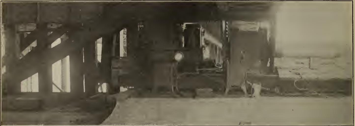
Figure No. 86.—Main Span, South Side—Arrangement for jacking at Anchor Pier.
