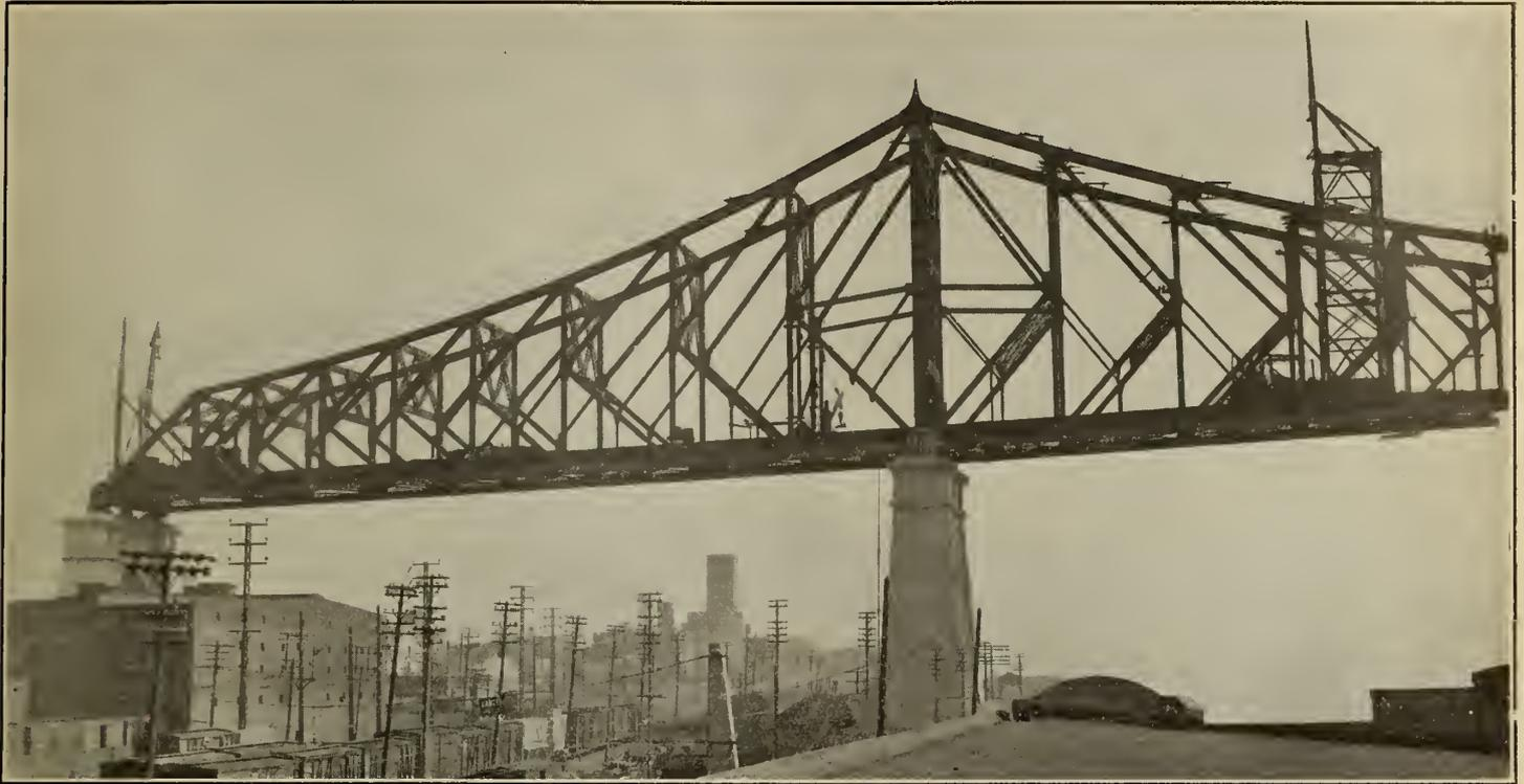
Figure No. 63.—Main Span, North Side—Stage completed. Tower at AL<sup>9</sup> removed and Traveller No. 4 being dismantled. Progress as at June 12th, 1928.
