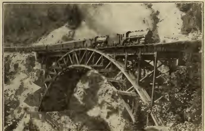
Figure No. 8.—View showing Temporary Loading of New Arch Ribs with Old Rails before attaching to Old Arch Ribs.
