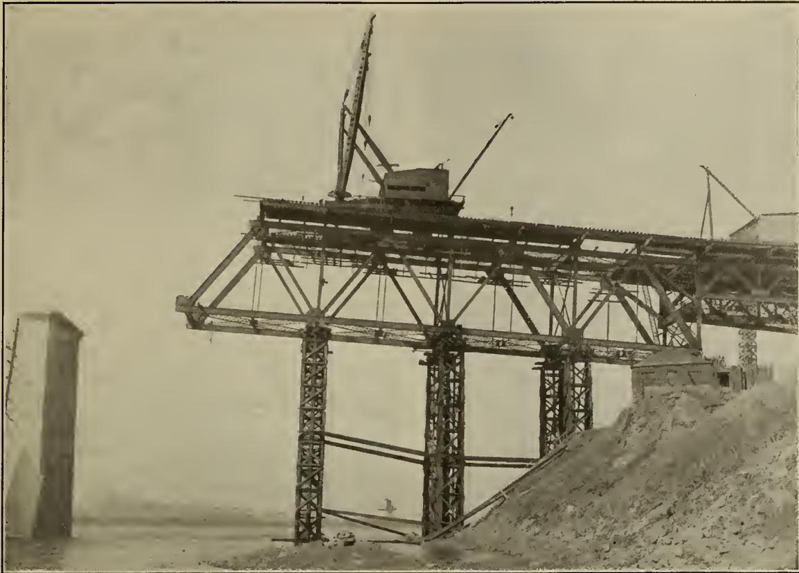
Figure No. 11.—South Approach—Timber Falsework under Span No. 22 (245-foot).
