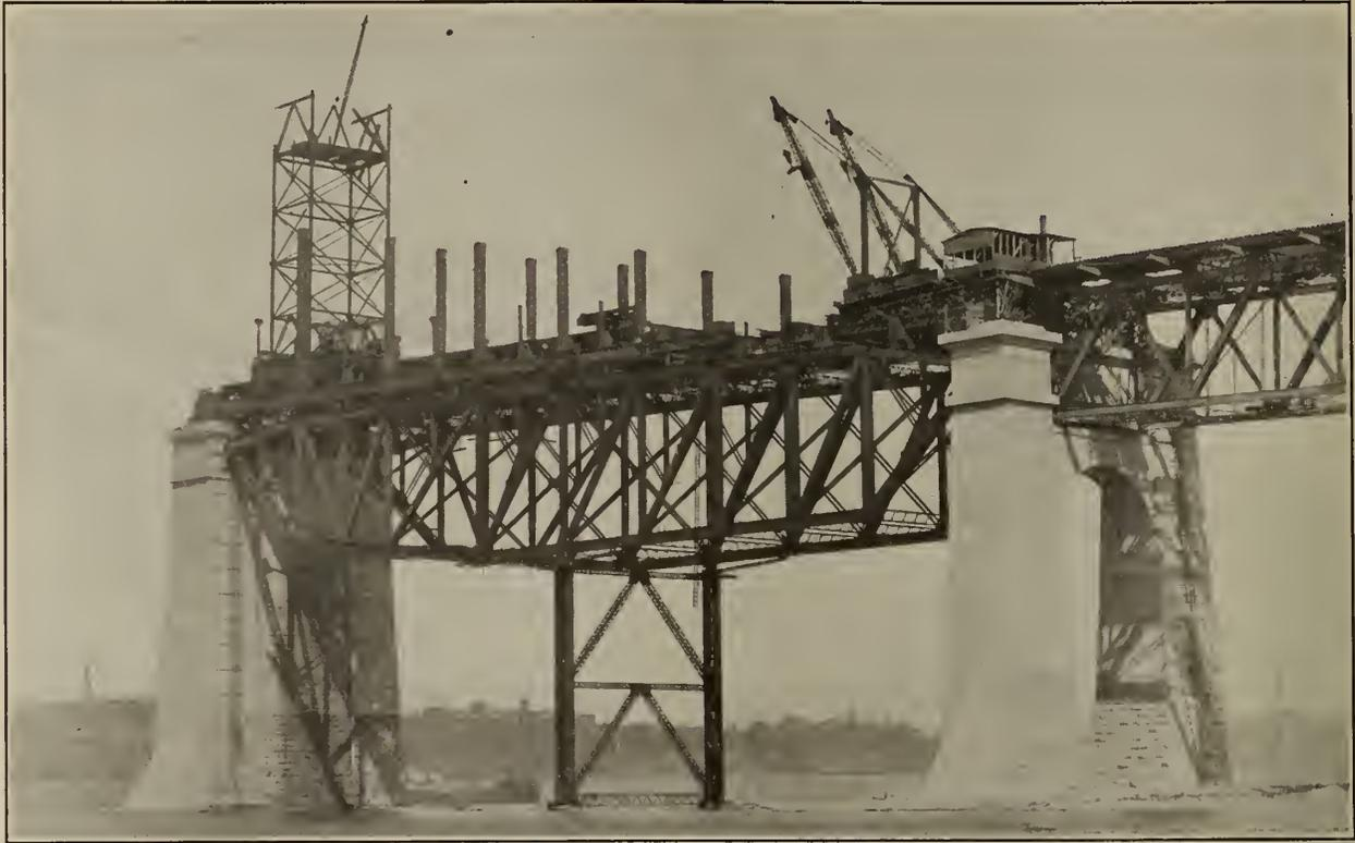
Figure No. 72.—Main Span, South Side—Erecting Bottom Chords and Floor System of Anchor Arm—Third Stage. Erection proceeding on Traveller No. 4.
