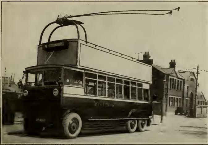
Figure No. 7.—Open Top Double-deck Trolley Bus at Hastings, England.
