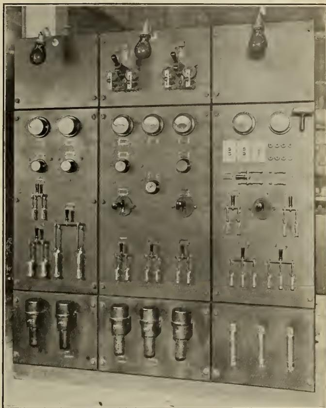
Figure No. 23.—Canadian Radio Beacon Transmitter—Power Control Panel.
