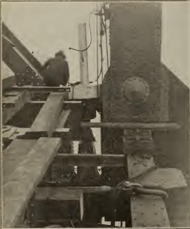
Figure No. 89.—Main Span, Centre Section—Detail at *SL0* showing Erection Wedge Mechanism in Place.
