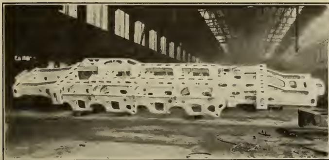
Figure No. 6.—Cast Steel Bed for Canadian National Oil-Electric Locomotive.
