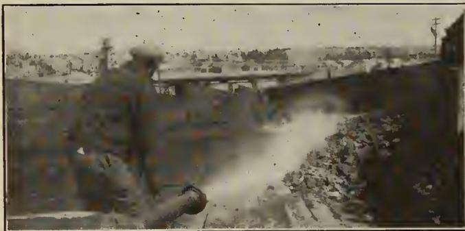
Figure No. 10.—Sluicing Operations in Hog box—Earth Fill Dam.
