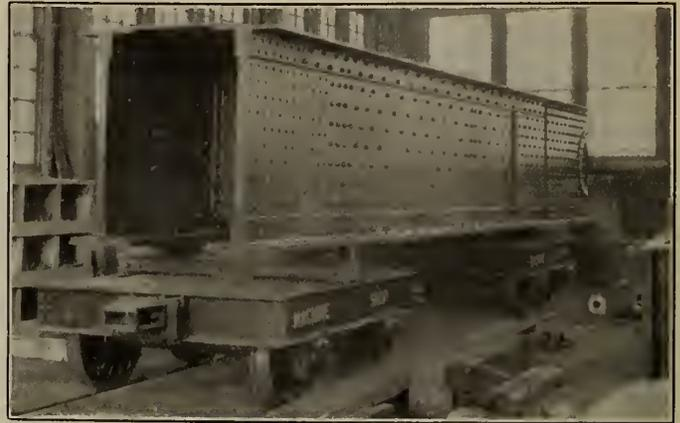
Figure No. 29.—Fabrication of Main Span—Main Bottom Chord Section—Boring of Member.
