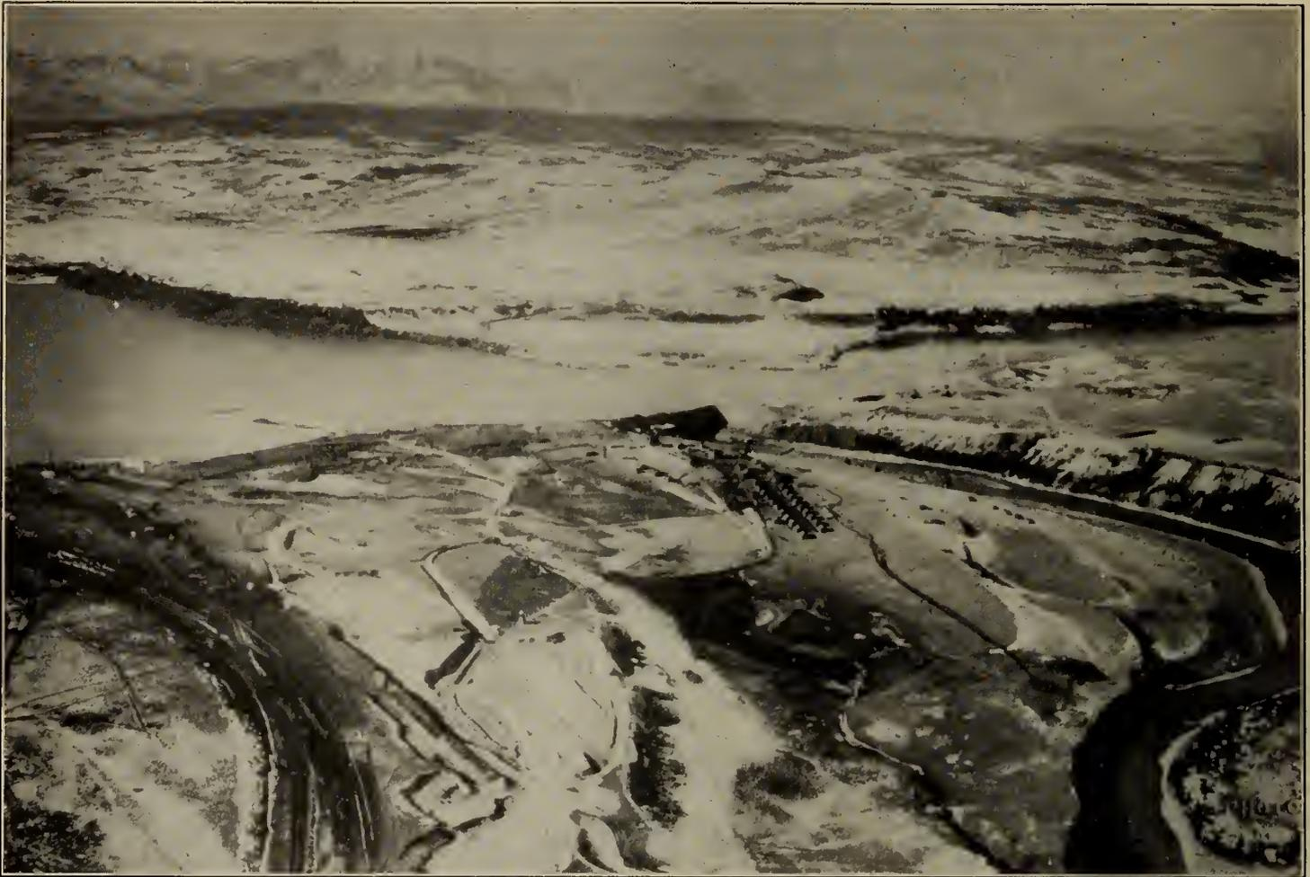
Figure No. 1.—Aerial Photograph of Dam showing Relation of Two Earth Fills to Concrete Portions of Dam.
