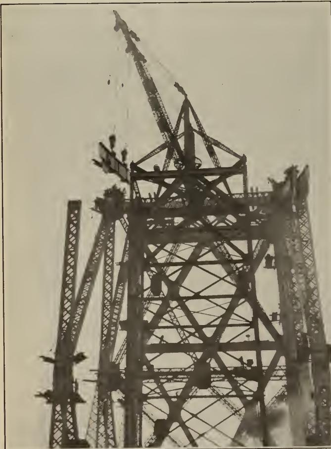
Figure No. 82.—Main Span, South Side—Erecting Top Chord Web showing Method of Handling.
