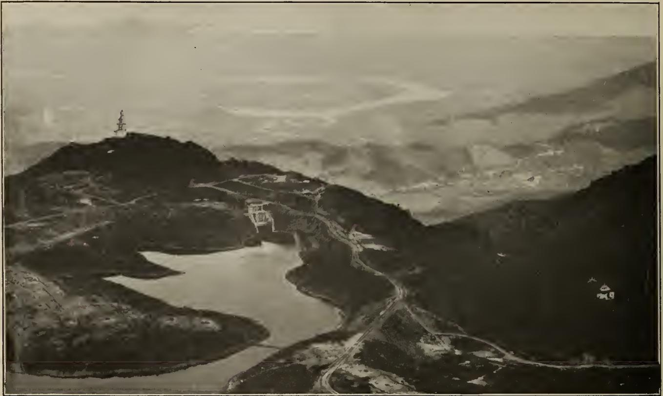
Figure No. 6.—Serra Development—Cascatinha Dike, Dam and Intake, Surge Tank, Coastal Plain and Praia Grande in Distance.
