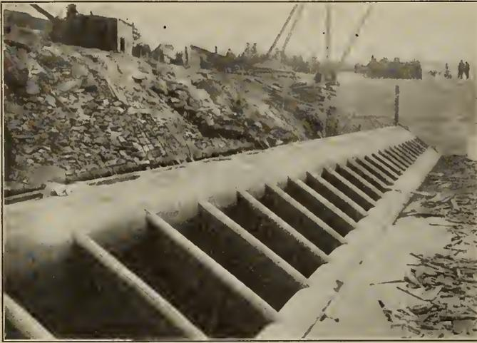
Figure No. 1.—Exterior of Intake Tube at Grand Falls Development. These Tubes, Two in Number, are  $17\frac{1}{2}$  feet in Diameter. The Vanes in the Intake Slot are set at Angles and Spaces Varied from End to End to Effect the Desired Distribution of the Draft throughout the Length of the Tube.
