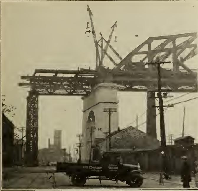
Figure No. 22.—North Approach—Typical Method of Erection—First Stage.
