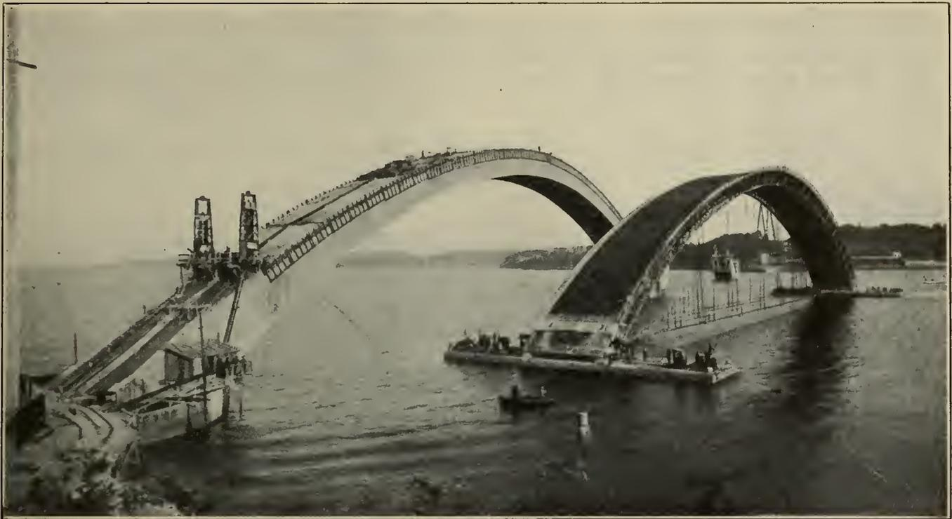
Figure No. 2.—The timber centring, originally built on shore, having been used for the first arch, has been lowered on to barges and is being moved to the site of the centre arch. In the background can be seen the pre-cast pier tops to which the centring will be secured.
