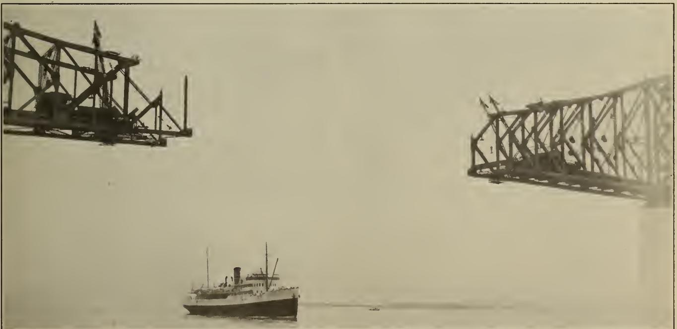
Figure No. 92.—Main Span, Centre Section—Erecting First Panel of Suspended Span on North Side—Second Stage. Erection proceeding at Outer End of South Cantilever Arm.
