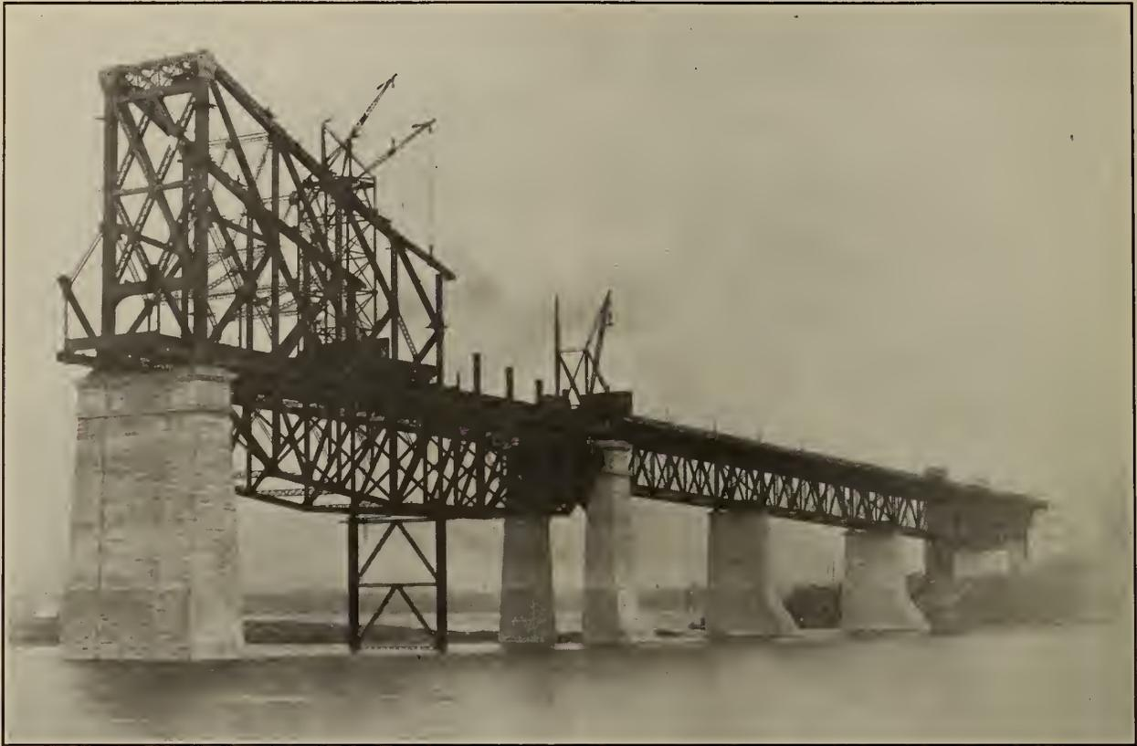
Figure No. 81.—Main Span, South Side—Erection of Anchor Arm being completed to AL7.
