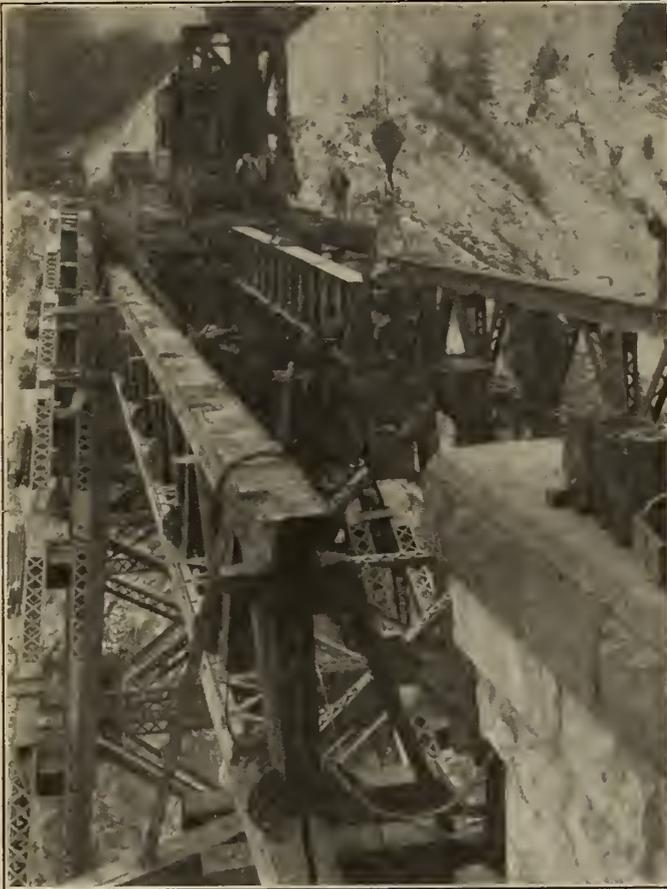
Figure No. 9.—Erecting Track Spans between Trains.
