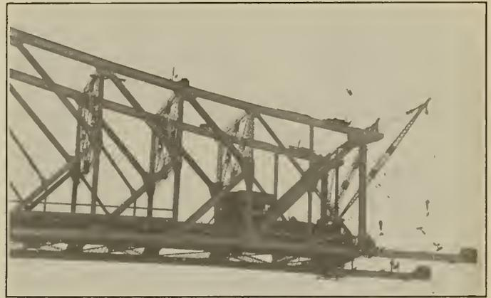
Figure No. 91.—Main Span, Centre Section—Erecting First Panel of Suspended Span on North Side—First Stage.
