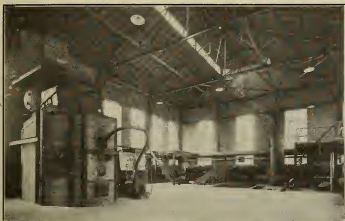
Figure No. 2.—Large Scale Testing Floor showing Pulverized Fuel Boiler Installation.
