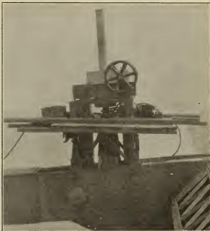
Figure No. 95.—Main Span, Centre Section—Side View of Wedge Mechanism in Place at *CU0*.
