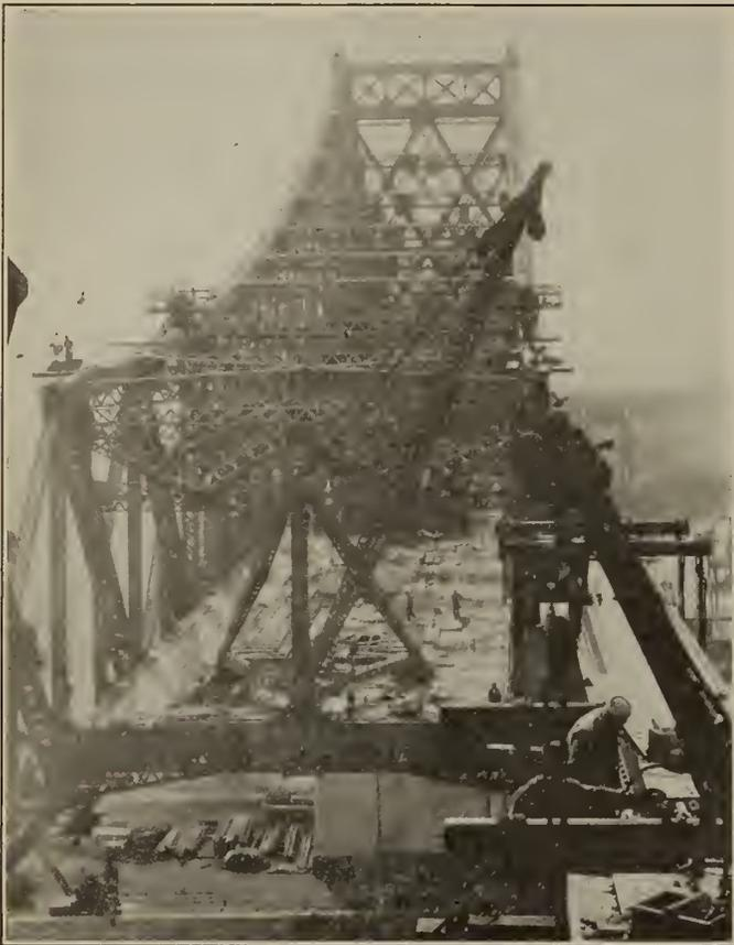
Figure No. 96.—Main Span, Centre Section—Arrangement of Moveable Derrick used in Erection of Centre Panels of Suspended Span.
