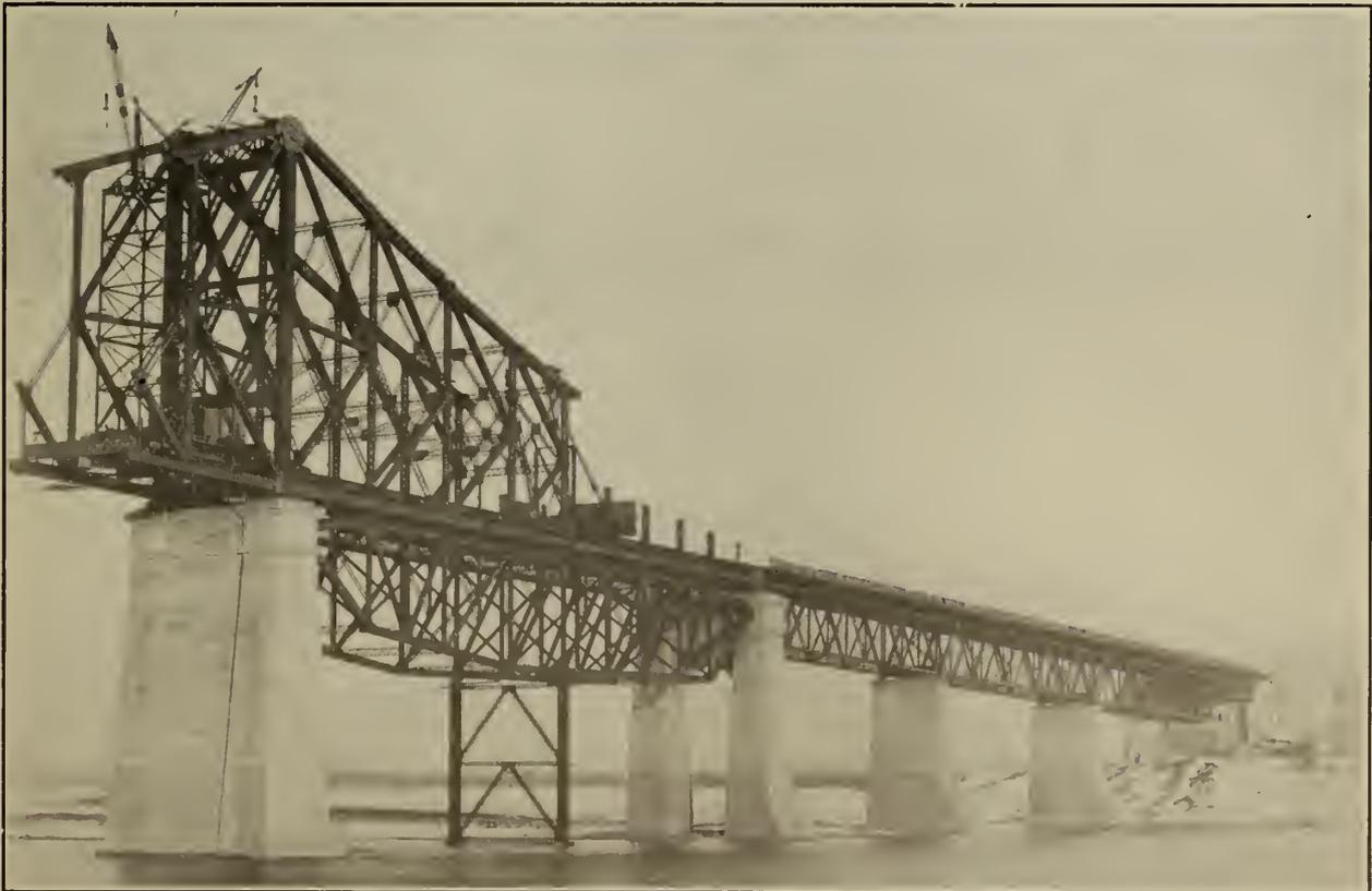
Figure No. 83.—Main Span, South Side—Erection commenced on Cantilever Arm.
