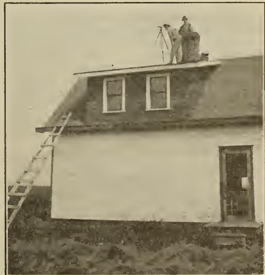
Figure No. 12.—Triangulation Control for One-Mile Mapping. An unusual triangulation station for the control of one-mile mapping in eastern Canada.
