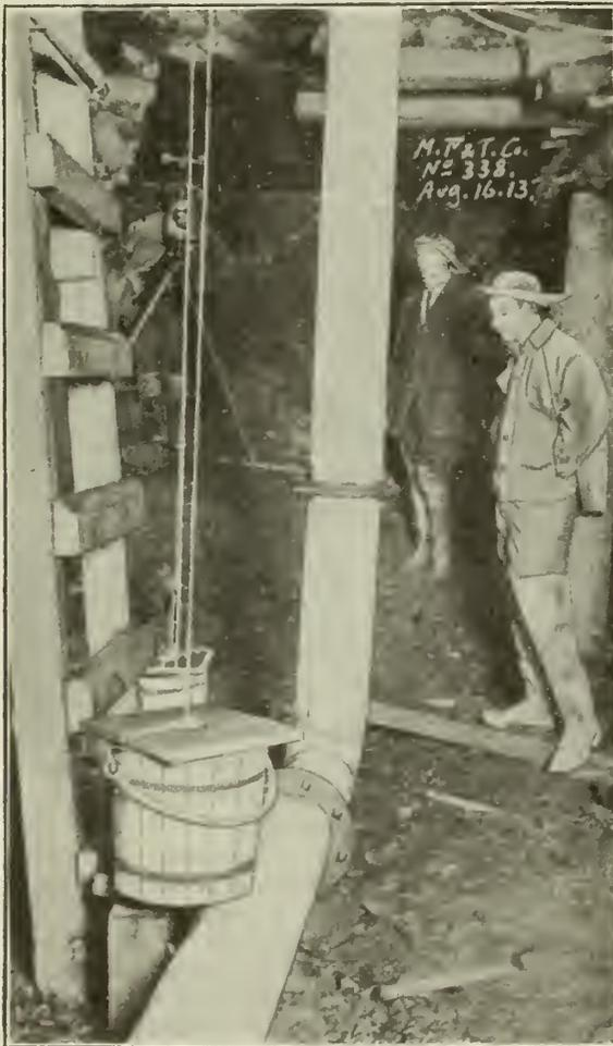
Fig. 4 Shaft Plumbing. "Bucking" into line.
