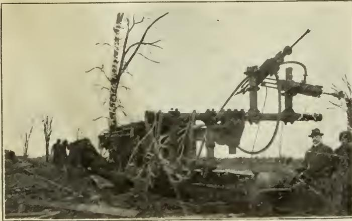
Fig. 9. Front View of Muck-Handling Drill Carriage.
