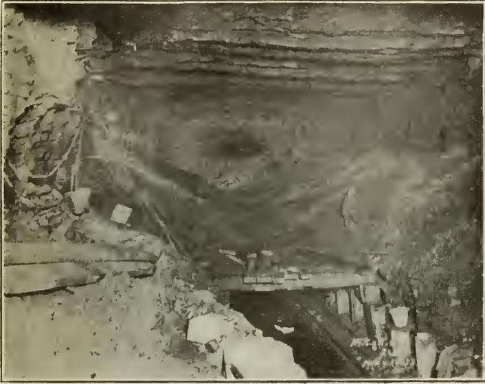
Fig. 12. Breakup showing Heading and Jumbo Timbers.
