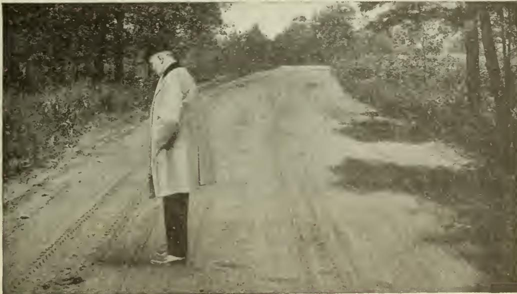
“Look at the deep tire tracks in the thick dust on this road. Dust is a sure sign of deterioration, the result of the heavy, fast moving traffic and the ravages of the elements.”
