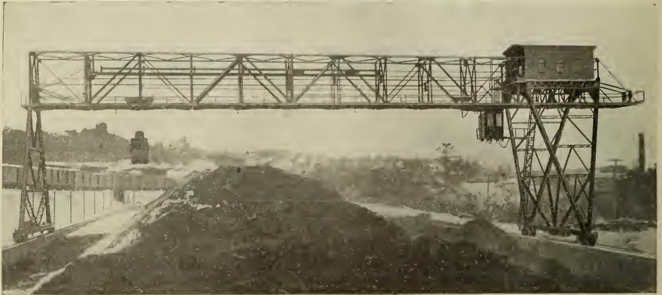
Coal Handling Conveyor—Designed and Built by Dominion Bridge Company, Limited
