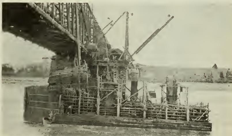
Pneumatic Caisson under air pressure in process of sinking operations.
