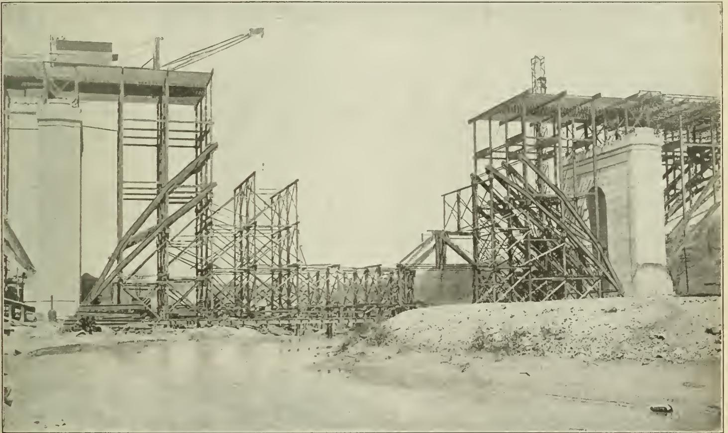
Fig. 10. 281 ft. 6 in. Span, Don Bridge, during Erection.
