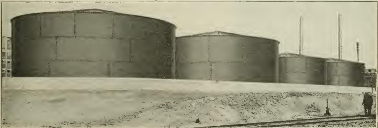
Fuel Oil Storage Installation at Dominion Steel Foundries Ltd., Hamilton, 2 tanks each 200,000 gallons capacity,
