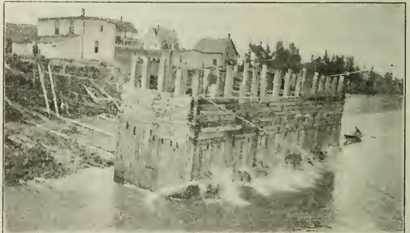
Launching Pneumatic Caisson for Moncton Bridge Foundations.
