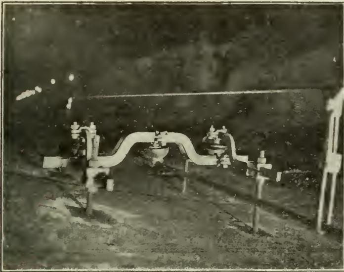
Fig. 40. Catenary Trolley Suspension in Tunnel.
