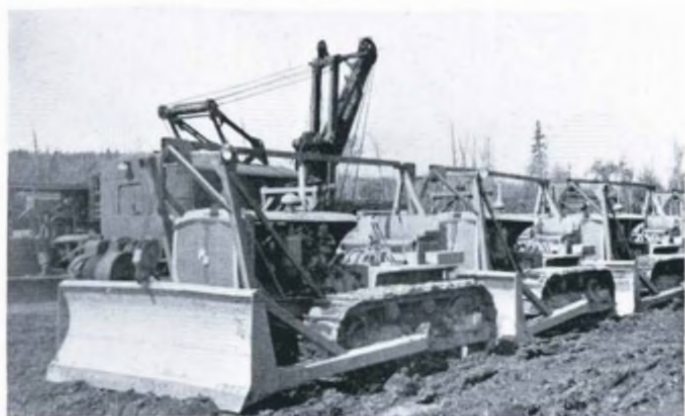
Above: A Northwest steam shovel and a group of Caterpillar diesel bulldozers lined up in the yards.
