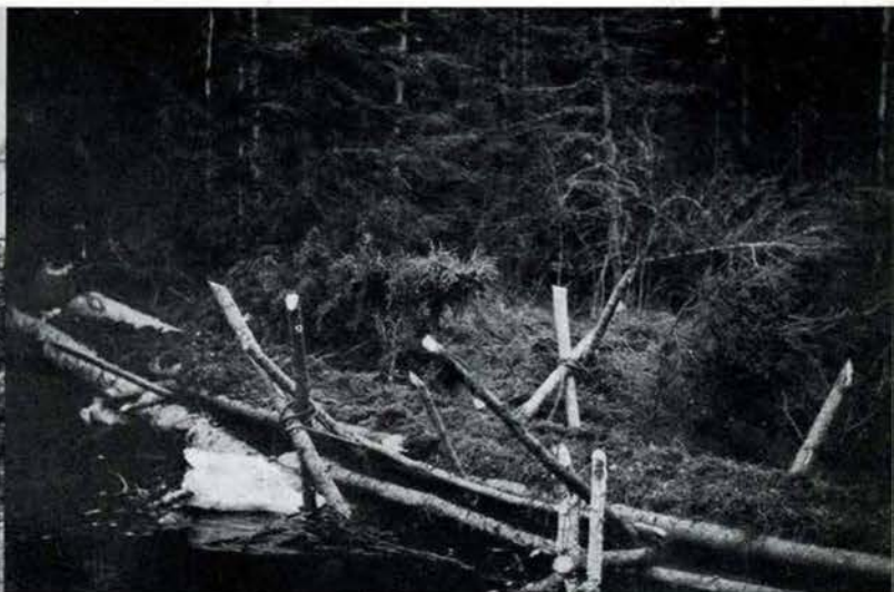
A bridge across a stream too deep to ford but narrow enough for bordering trees to span.
