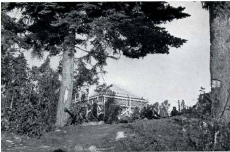
The new warehouse from the dock.
