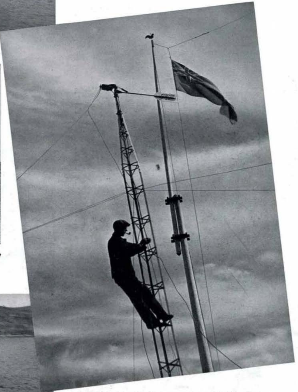
Ship's Carpenter Clem James, erecting a wind mill to charge the batteries of the radio station at Hebron.
