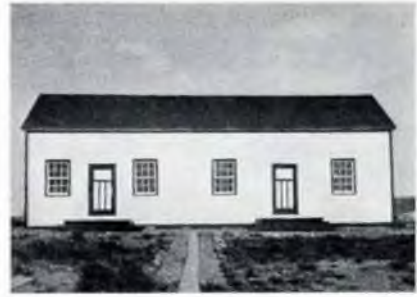
House moving at Baker Lake post. The house was cut in two, each section hauled by ninety dogs to the new site two miles away, and the two fitted together again.
