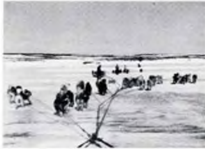
House moving at Baker Lake post. The house was cut in two, each section hauled by ninety dogs to the new site two miles away, and the two fitted together again.
