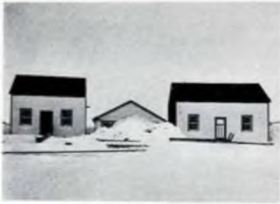
House moving at Baker Lake post. The house was cut in two, each section hauled by ninety dogs to the new site two miles away, and the two fitted together again.
