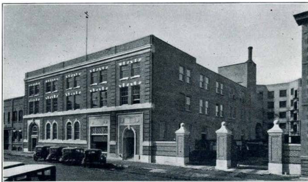
Hudson's Bay Company Edmonton Warehouse, Fur Trade District Office, Fur Trade Depot and Land Department District Office
