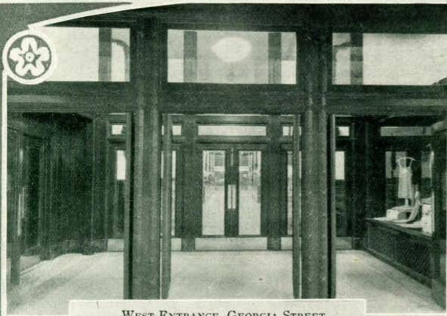
WEST ENTRANCE, GEORGIA STREET
