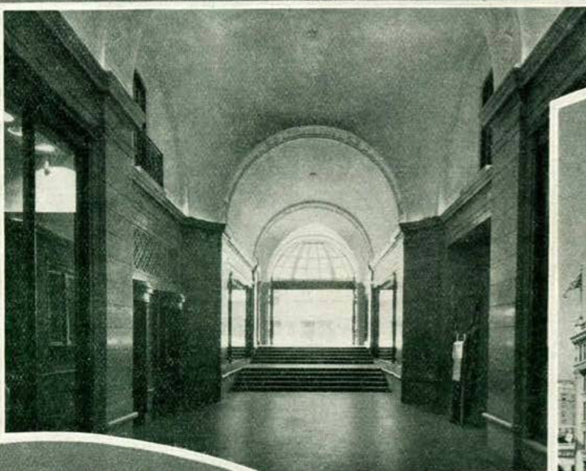
ARCADE, LOOKING WEST
