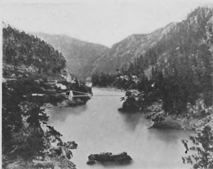
Old Cariboo Bridge Fraser Canon
