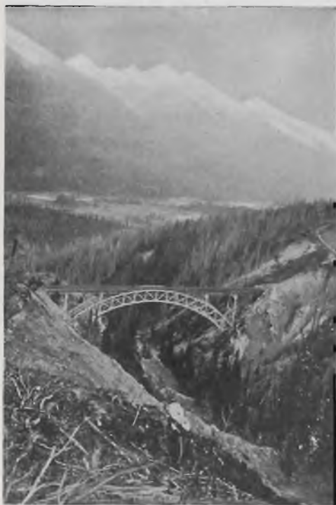
Stoney Creek Bridge
