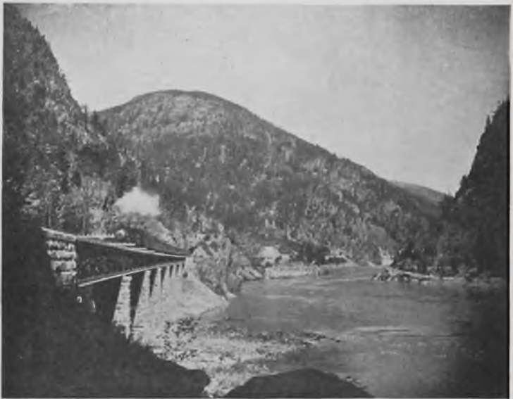
White's Creek Bridge, Fraser Canon
