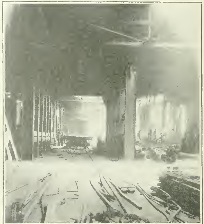
Jacking Stall for Repairing Steel Cars, Canadian Government Railways.
