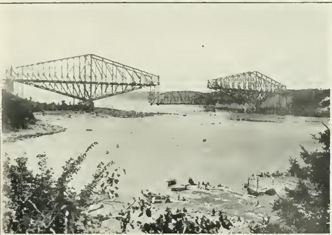
Quebec Bridge. The placing of the suspended span
