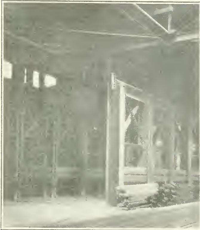
Jacking Stall for Repairing Steel Cars, Canadian Government Railways.
