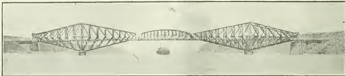
The Quebec Bridge as completed, from the Contractors' Sketch.
