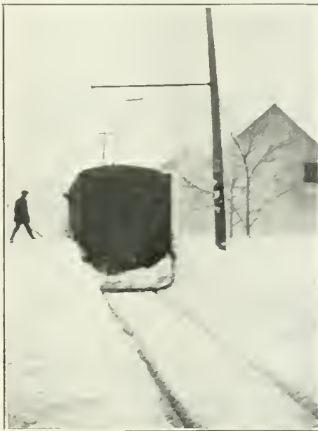
300 h.p. rotary snow plough, Levis County Ry., operating in 9 ft. of snow
