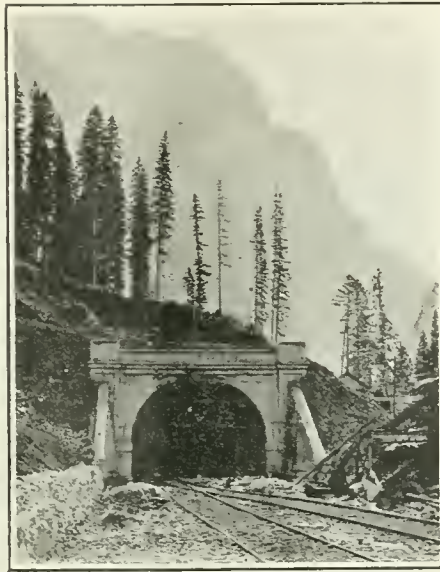
Connaught Tunnel, C.P.R., East Portal
