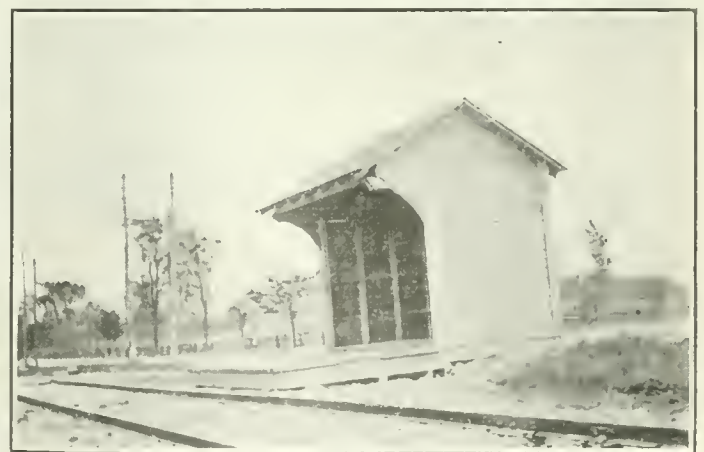
Toronto Suburban Railway, standard shelter.
