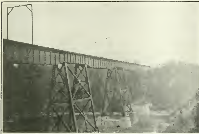
Toronto Suburban Railway, Humber River Bridge.
