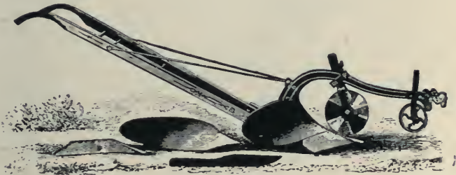
49. PLOW WITH REVOLVING COULTER.
