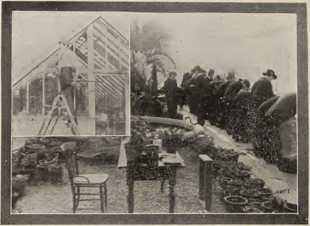
Inside and Outside the Greenhouses.
