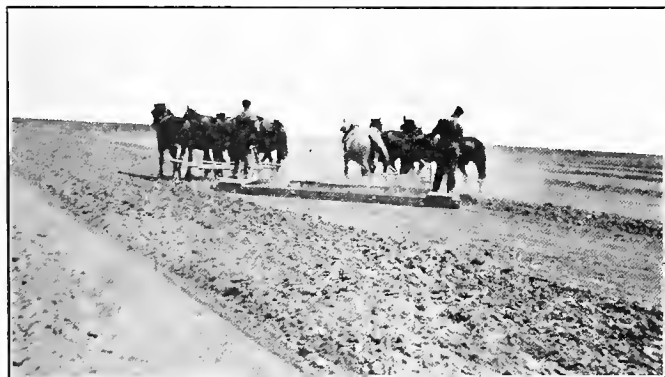
Fig. 82.—Float Levelling Land for the Border System of Irrigation.
