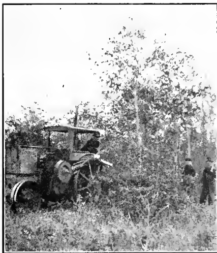
Fig. 53.—Removing Small Trees with Tractor.
