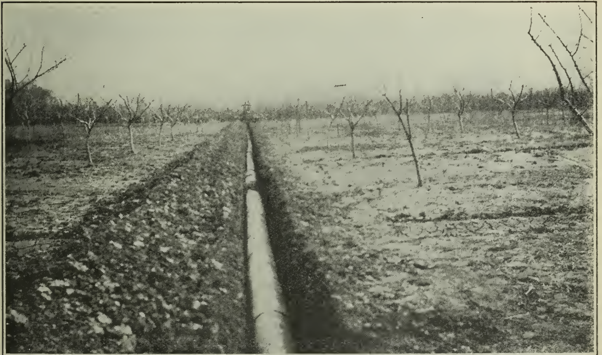
Fig. 8.—A nicely graded straight trench with tile well laid facilitates the flow of the water.
