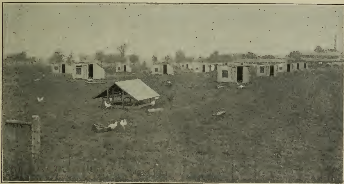
Fig. 37. Range scene with colony houses, range shelter, feed troughs and hoppers.
