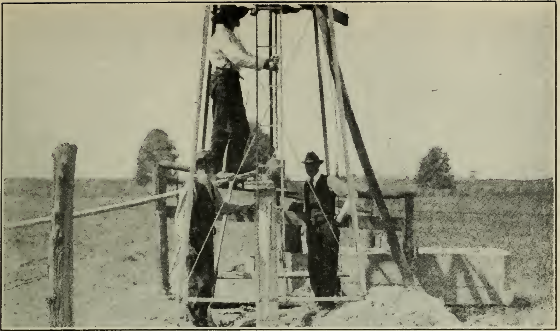
Fig. 5.—(a) Sinking the open 10-inch drive pipe.
