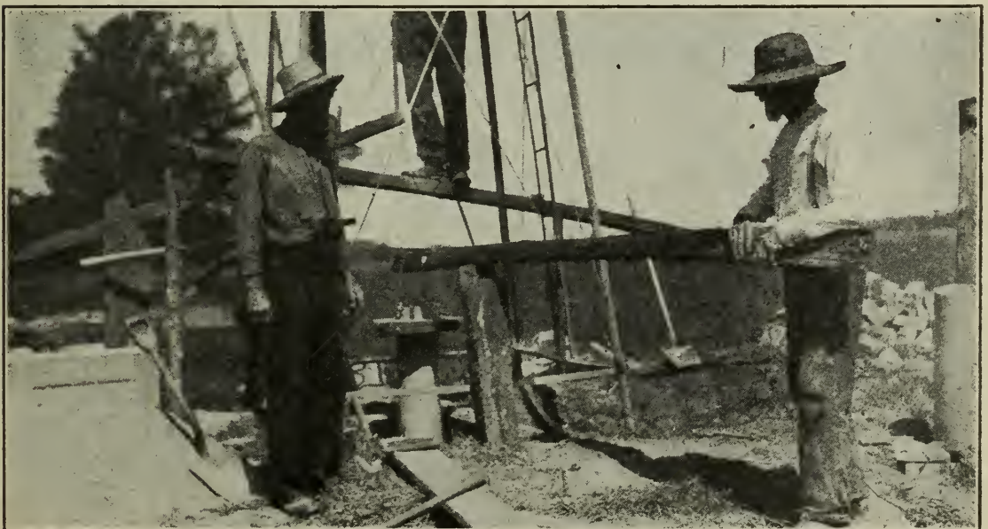
Fig. 5.—(c) Withdrawing open drive pipe.
