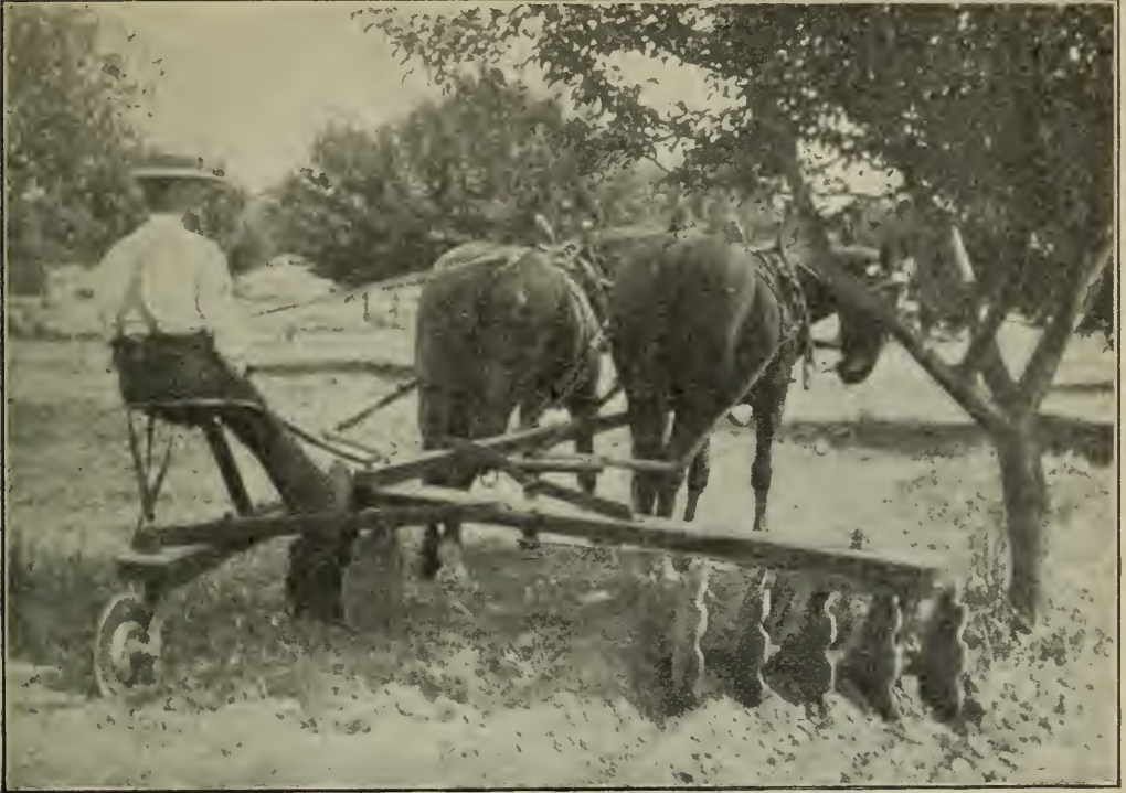
Cutaway extension disc, an improvement on the useful disc harrow.
