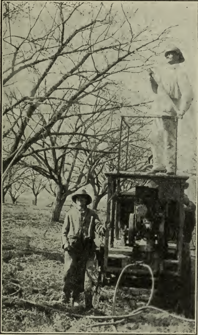
Type of gasoline spray outfit for large orchards.
