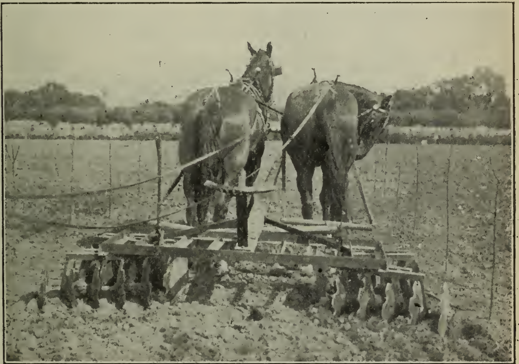
Double cutaway disc which breaks up the soil nearly as effectively as the plow.
