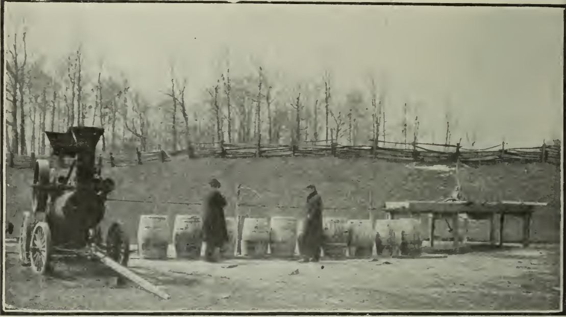
Fig. 5. Threshing engine used for boiling the wash.
