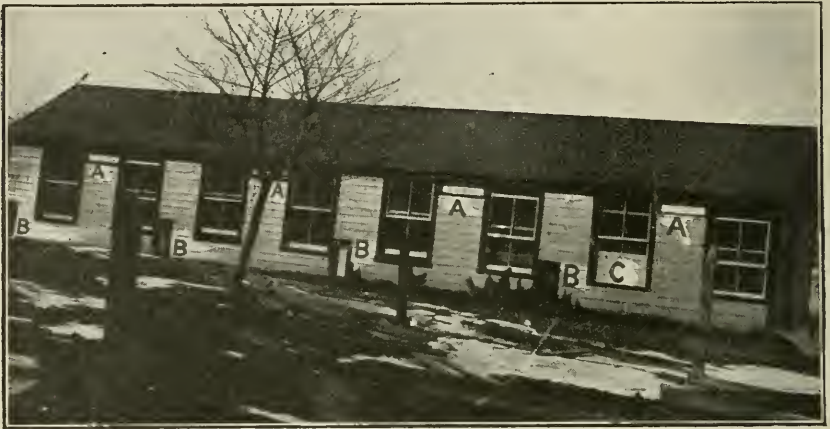
Fig. 4.—A good farm poultry house; (a) cotton screen between the windows; (b) runways; (c) frame covered with cotton for windows.
