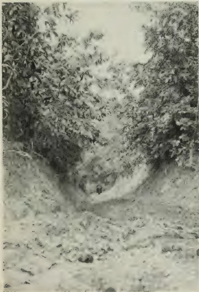
POOR ROAD-MAKING Washed out by heavy rains
