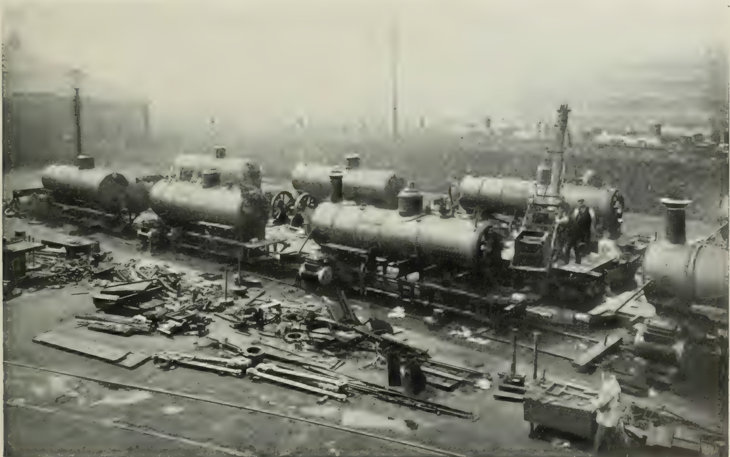
THE MIDLAND YARD IN ENGLAND The American engines are being erected in the open
